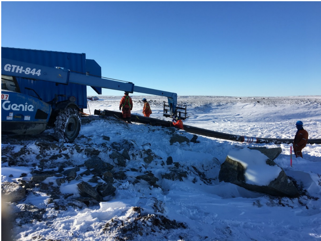
Picture 5 Telehandler pushing pipe with boom
