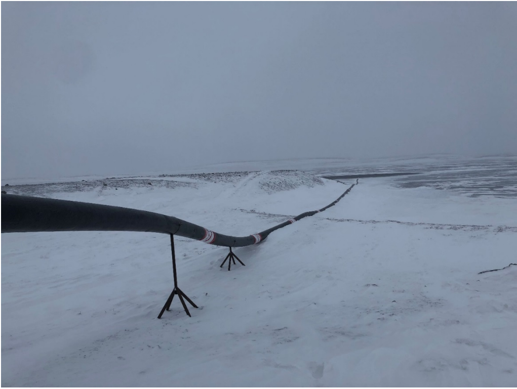
Picture 9 Final suction line installation
