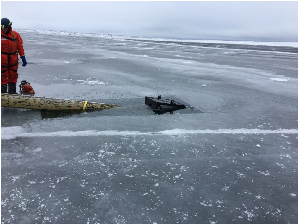
Picture 8 Suction line sinking
