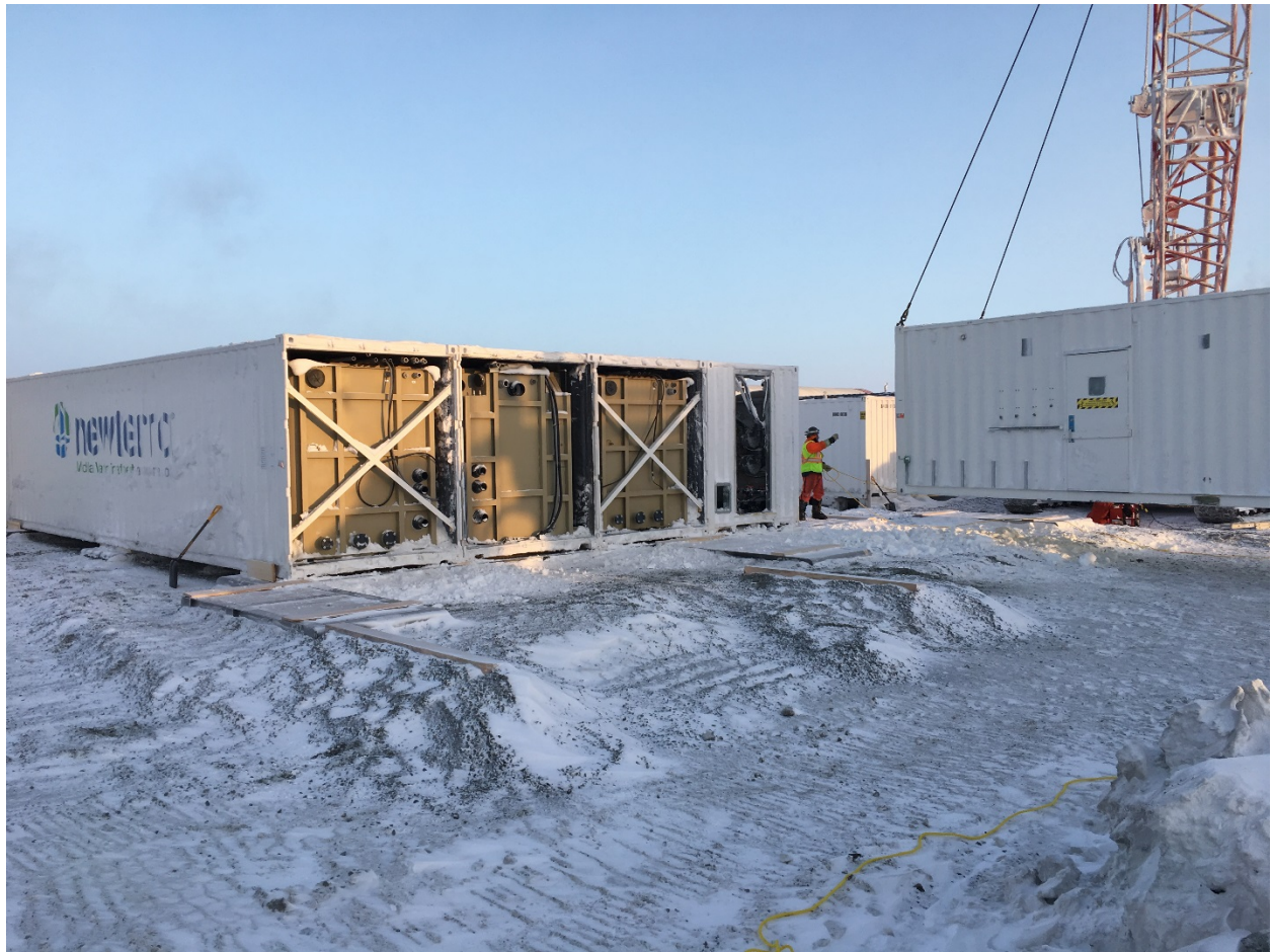
STP – Modules installation 1 of 2
