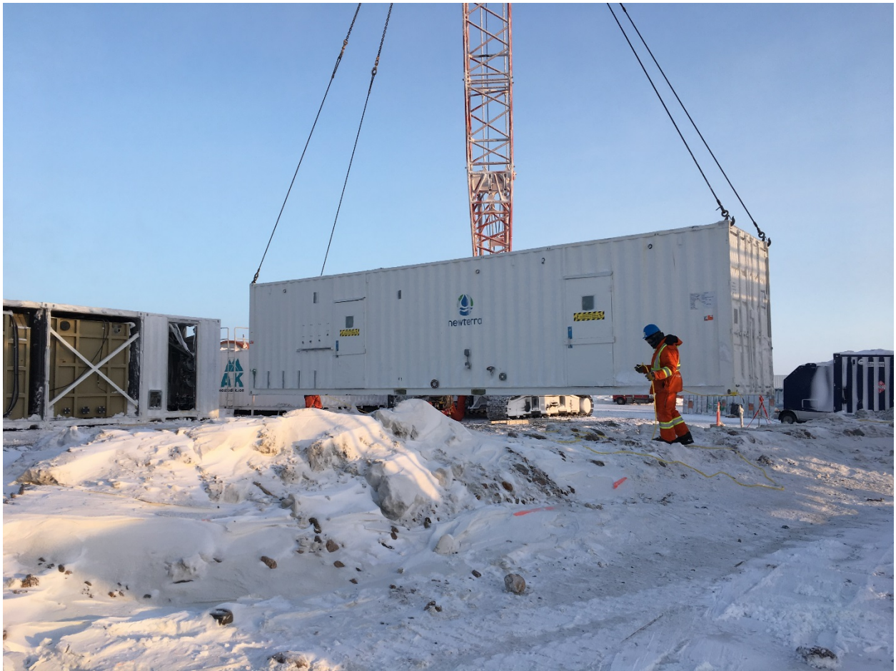
STP – Modules installation 2 of 2
