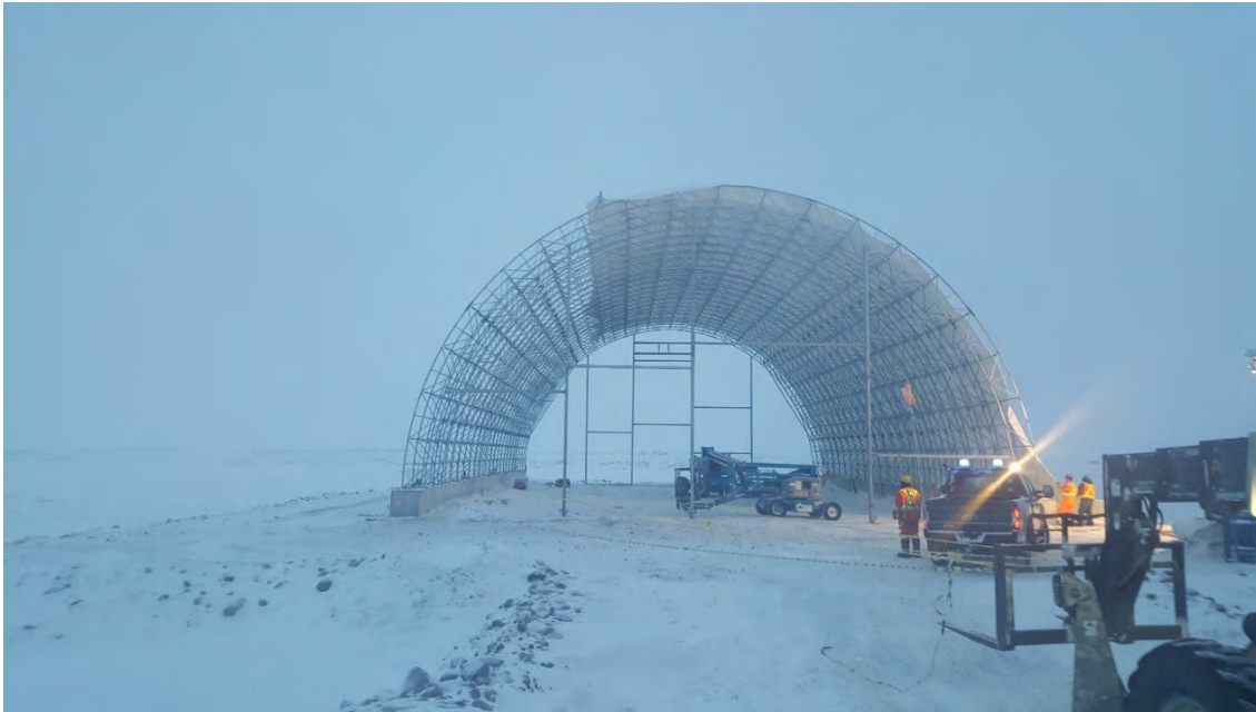
WTP Dome tarp installation
