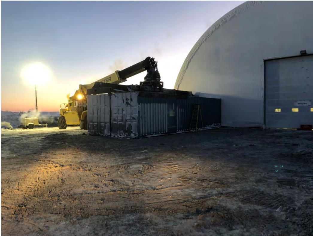
AsWTP container section installation
