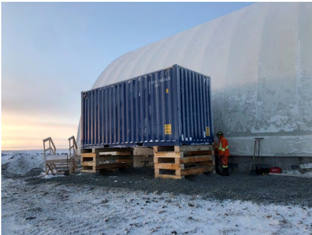
AsWTP electrical room installation
