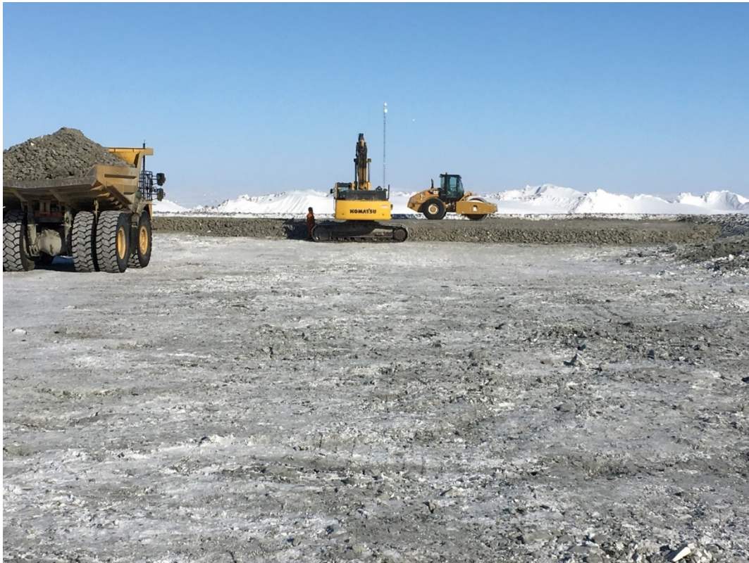
Pad and Berm construction
