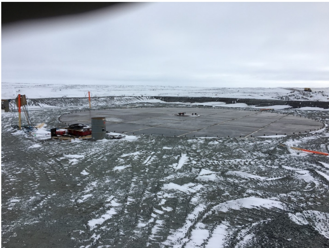
Tank floor construction
