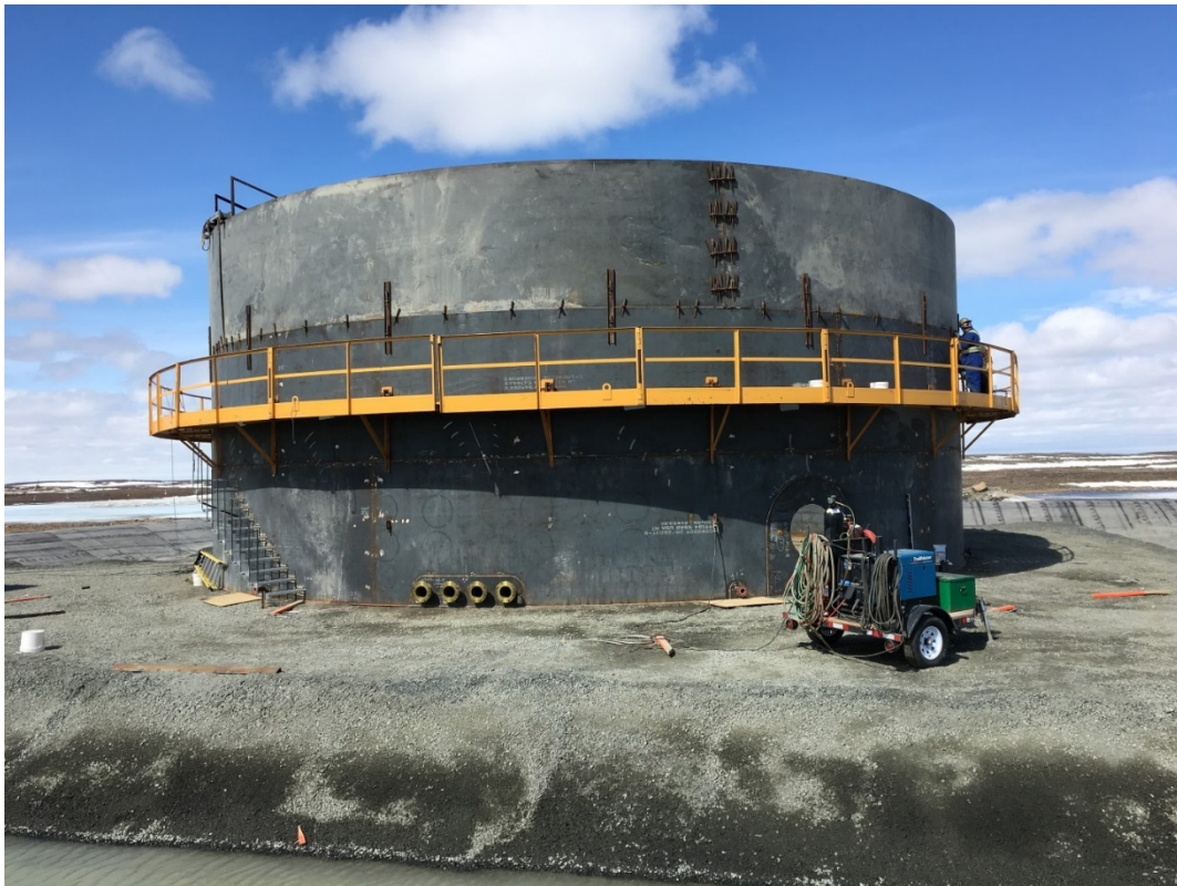
Tank wall welding
