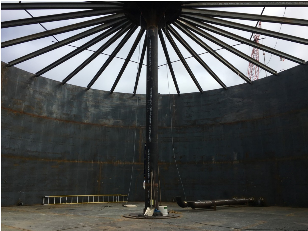
Tank roof structure
