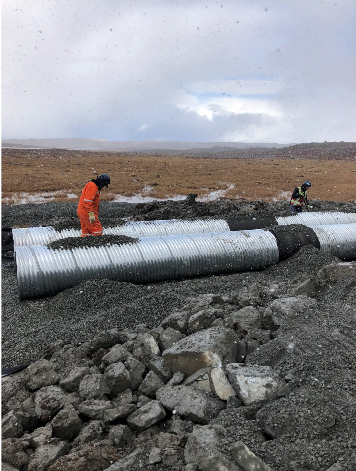
Culvert 11-4 installation
