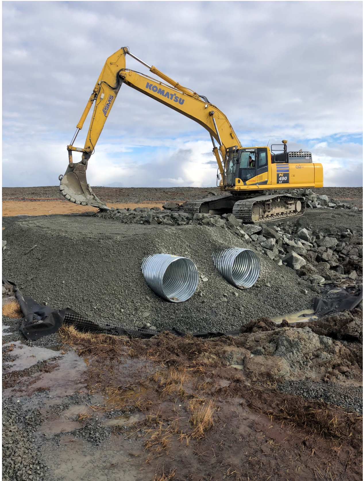
Culvert 11-4 installation
