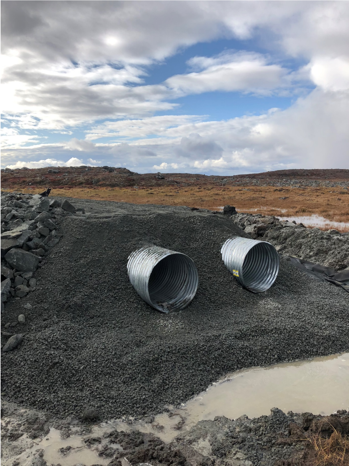
Culvert 11-4 installation
