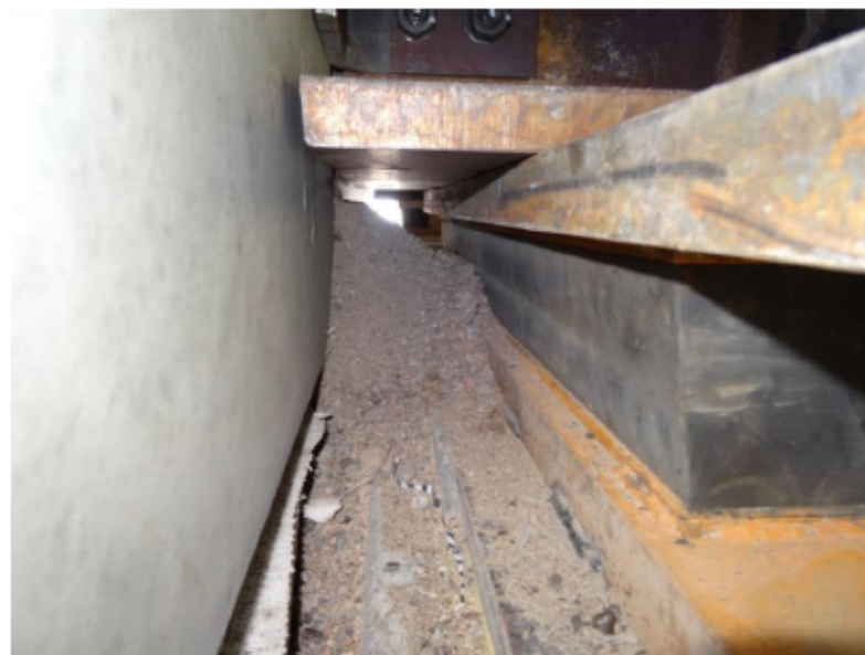
Figure 4-4 Bridge at km 44.5 – north centre bearing – debris spill through ballast wall Evazote joint
