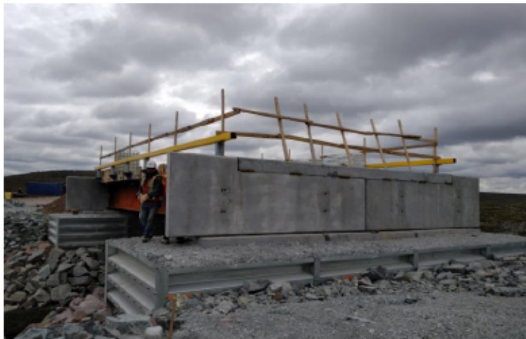
Figure 3-8 Bridge at km 43.5 – Approach Fills Complete Only on South End
