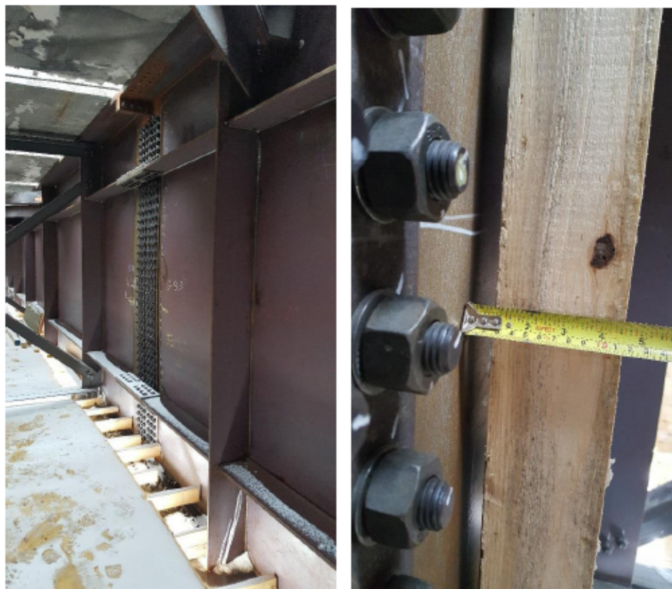
Figure 3-1 Web Panel Out-of-Straightness at Splice Locations (Bridge at km 23.9)
