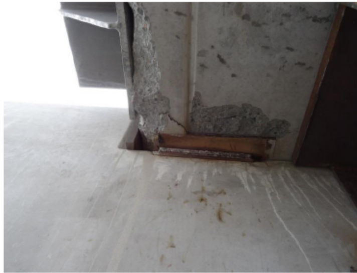
Figure 3-2 Spall in Deck Soffit at km 44.8 Bridge, Southeast Corner
