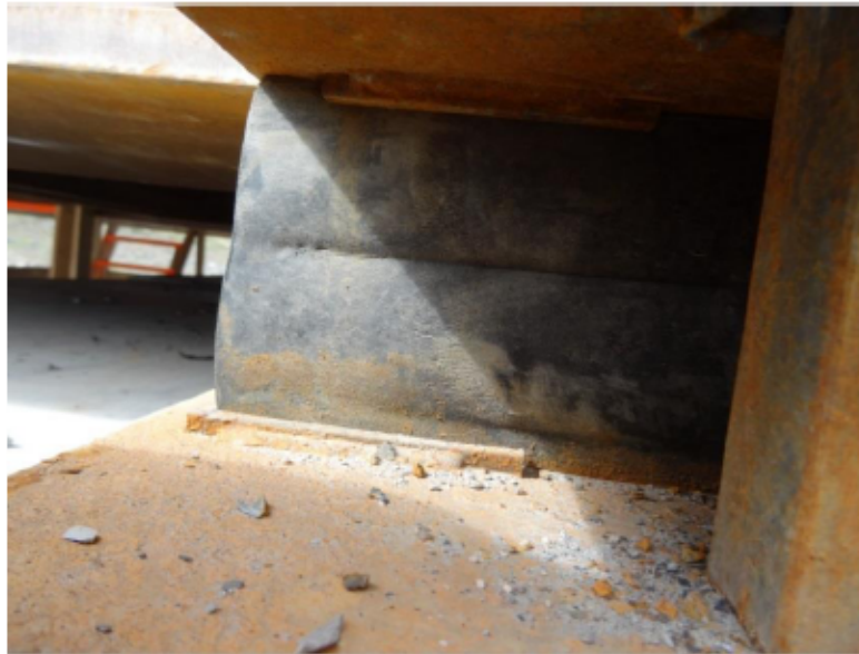
Figure 3-6 Bridge at km 32.3 Southwest bearing – front top keepers have been removed
