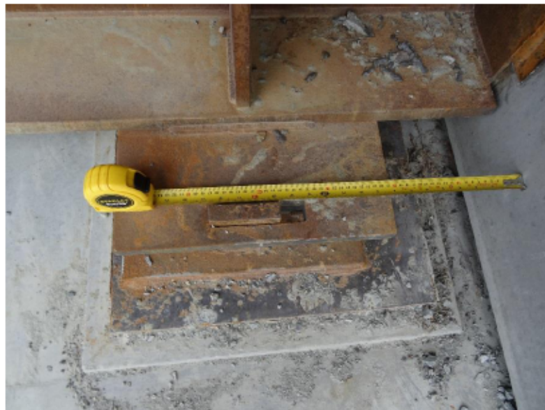
Figure 3-5 Bearing guide plate engaging shear key – bridge at km 3.5, northeast bearing
