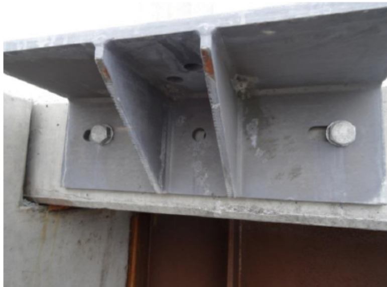
Figure 4-5 Bridge at km 10.5 railing bracket (Note: This bracket could be shifted to capture the centre bolt)
