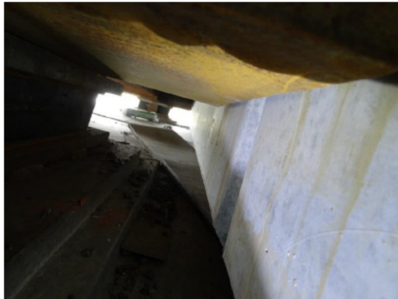
Figure 4-3 Bridge at km 43.5 Evazote loose in front of ballast wall
