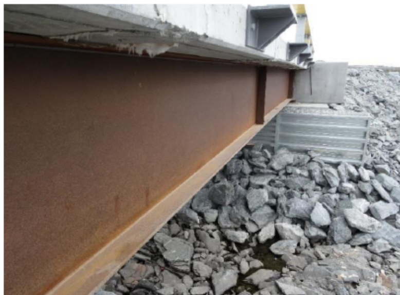
Figure 4-6 Bridge at km 3.6 – Underside of deck joint (southeast)
