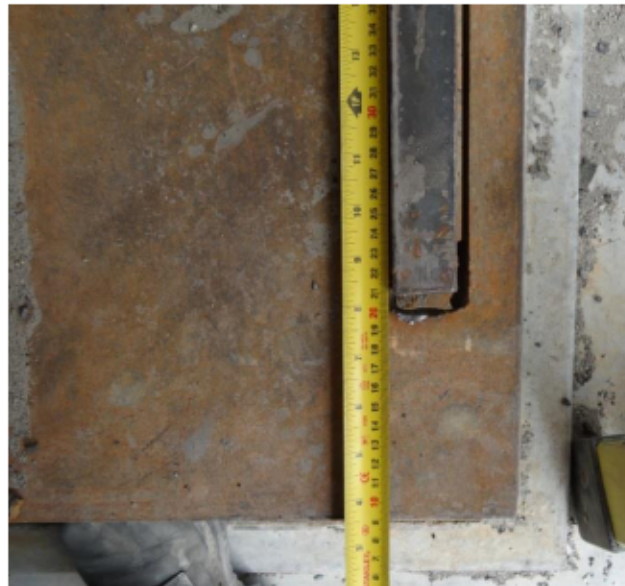
Figure 3-7 Bridge at km 32.3 Southwest bearing – Enlarged bearing guide plate slot by the Contractor during installation
