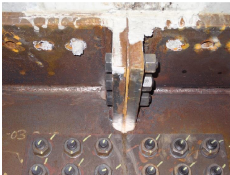
Figure 4-1 Bridge at km 32.3 – compression splice with shim
