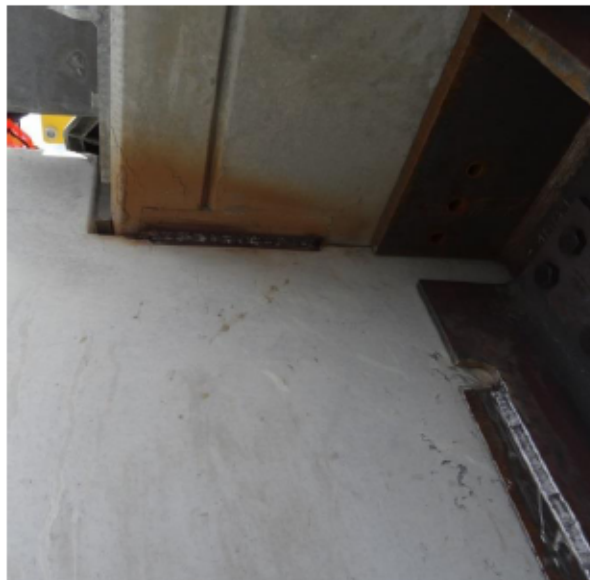
Figure 3-3 Minor Spalling in Ballast Wall Next to Embedded Plate (km 32.3 Bridge, Southeast Corner)
