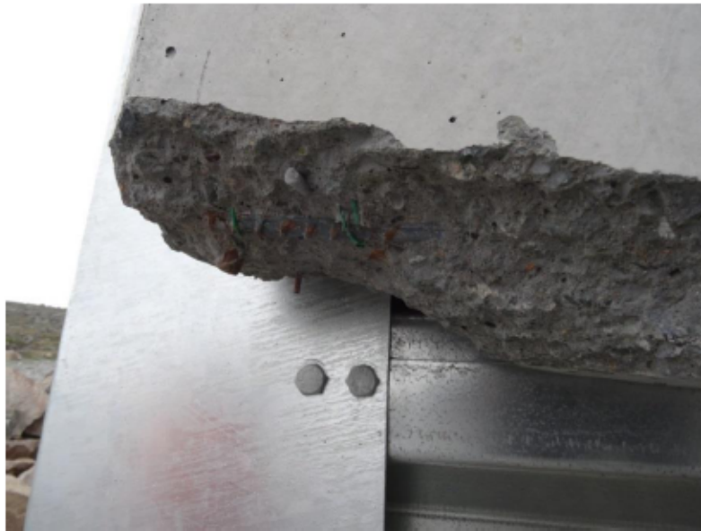
Figure 3-4 Bridge at km 23.9 – Northwest ballast wall bottom corner – exposed rebar in spall
