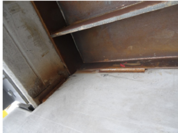
Figure 4: Minor spalling and scorching at ballast wall and deck soffit (SE)
