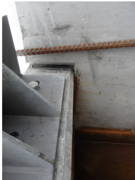
Figure 3: Deck to ballast wall joint (NE)
