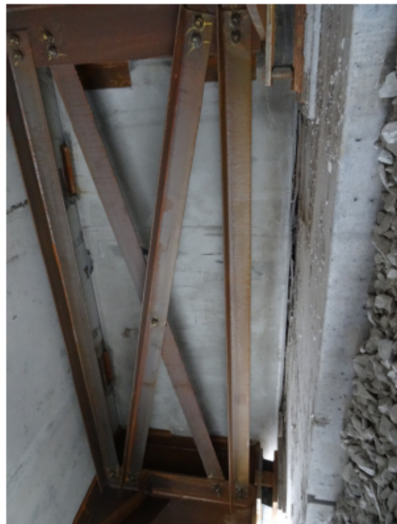
Figure 11: Southeast abutment diaphragm and ballast wall
