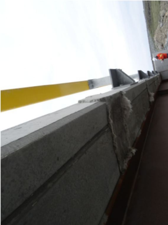
Figure 2: Deck joint (at northwest)
