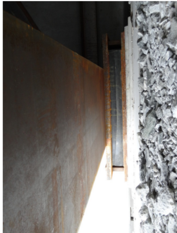
Figure 8: NW bearing front (fabrication imperfection)
