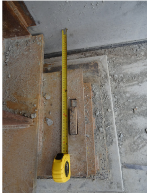
Figure 16: Typical bearing guide plate at the end of its slot
