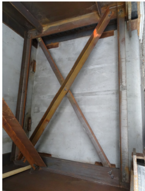
Figure 7: NW abutment diaphragm bracing
