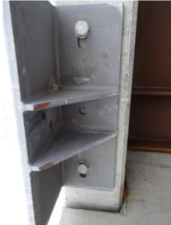
Figure 4: Typical railing connection (SE)
