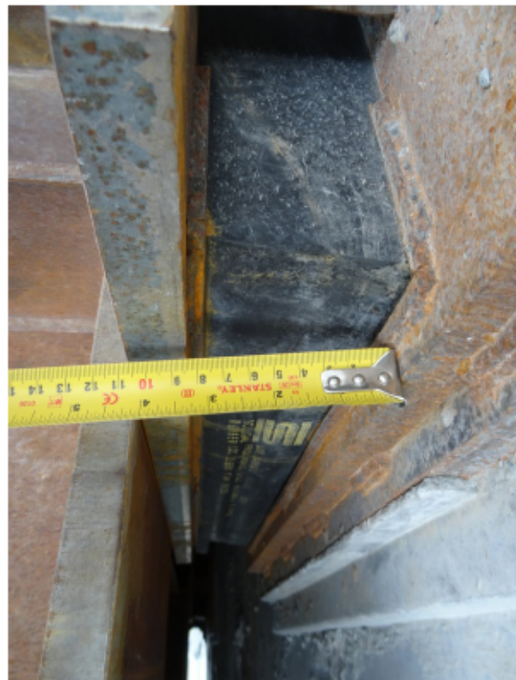
Figure 15: Typical bearing with keepers (southwest)
