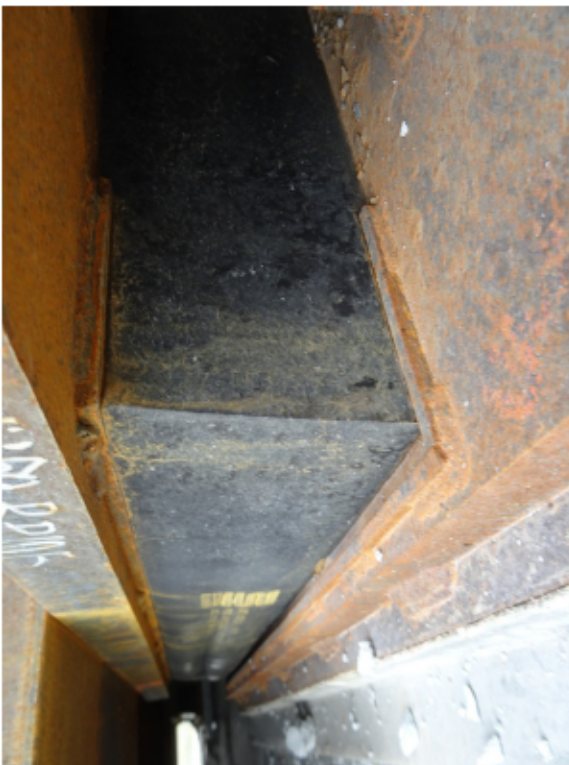
Figure 5: NE bearing front (some protrusion of neoprene over top keeper)
