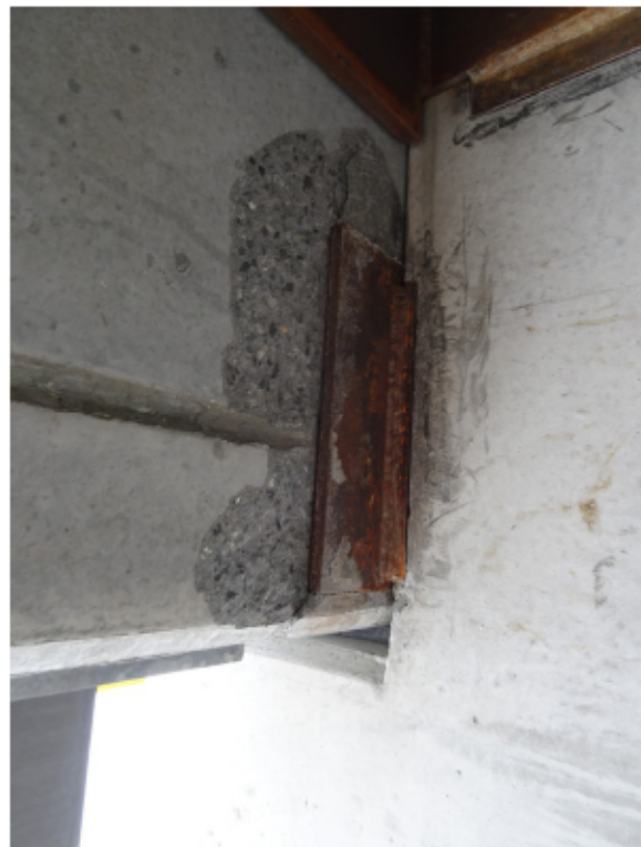
Figure 11: Minor spall at NW deck soffit
