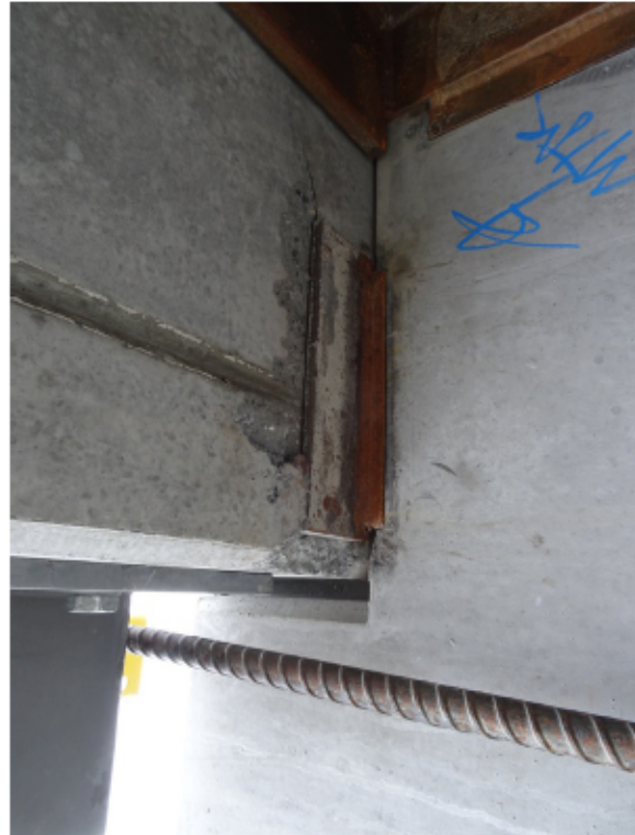
Figure 12: Minor concrete spall, underside of deck (NW corner)
