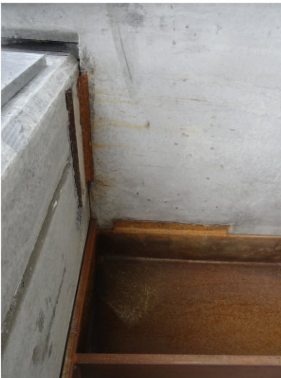
Figure 9: Minor concrete spall at NE abutment
