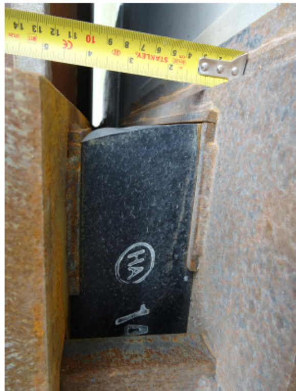
Figure 3: Typical bearing (SE)
