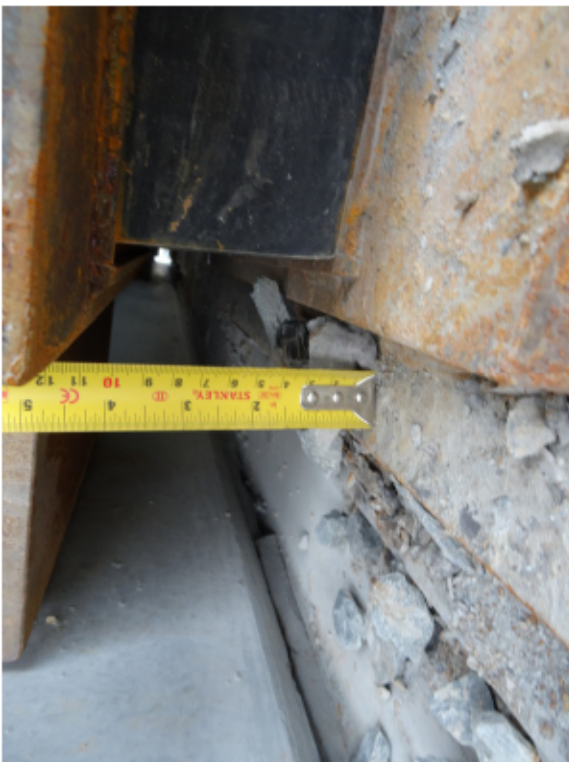
Figure 13: Typical back of bearing (NW)
