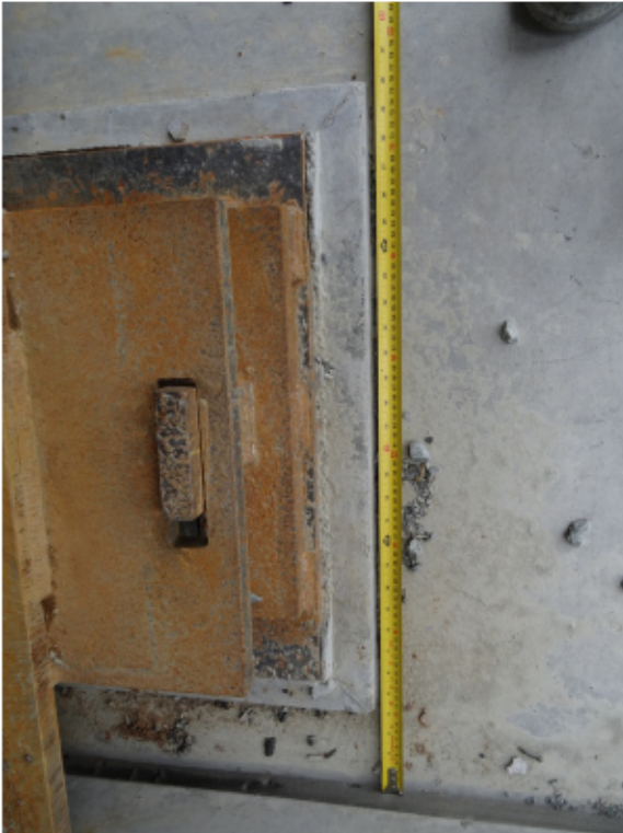
Figure 10: NW bearing - some slot length remaining
