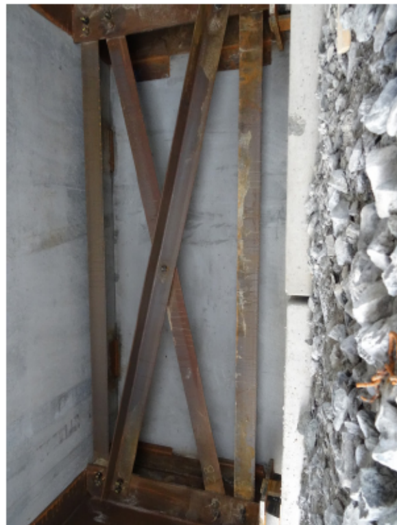
Figure 7: Northeast abutment diaphragm and footings
