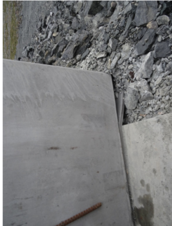
Figure 8: Northeast ballast wall and evazote
