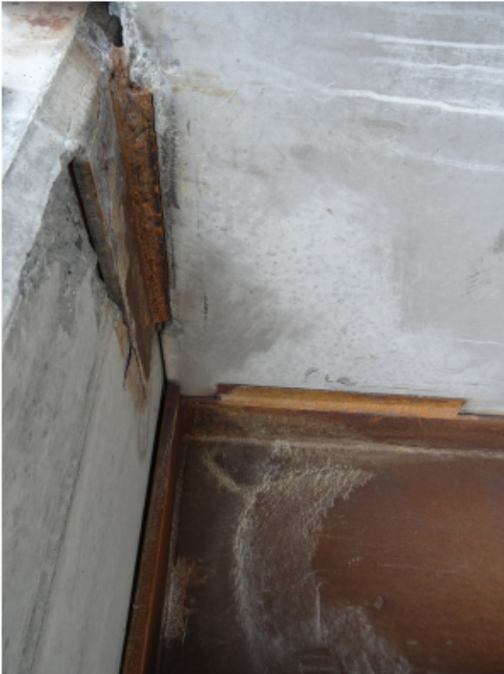
Figure 2: Minor deck soffit spill (SW corner)
