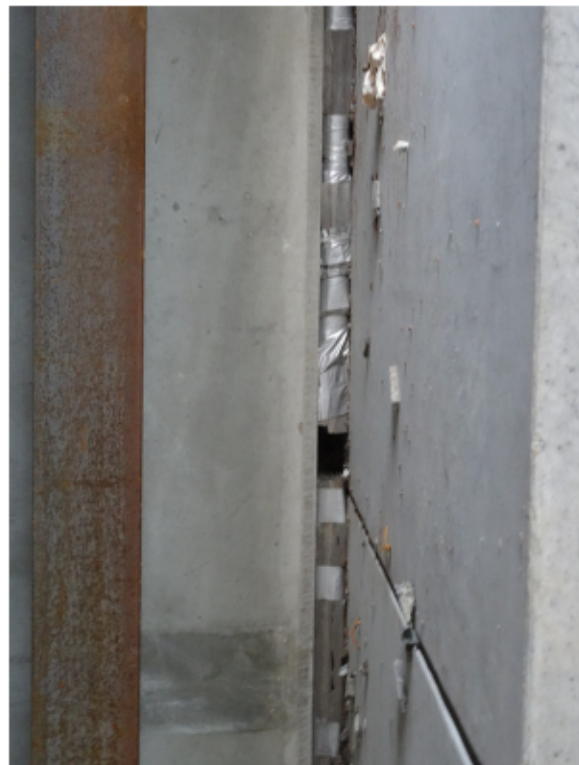
Figure 7: Evazote under NE ballast wall
