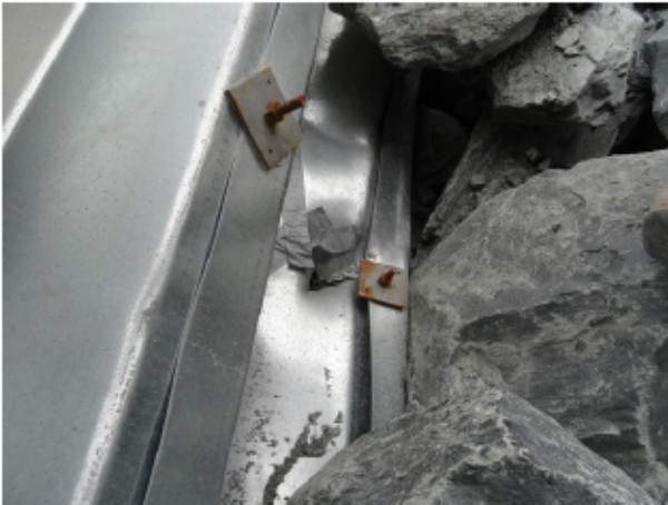
Figure 6: Damaged NE bin wall
