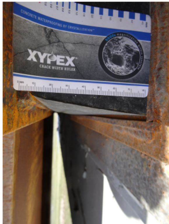
Figure 15: Typical front of bearing (SW)
