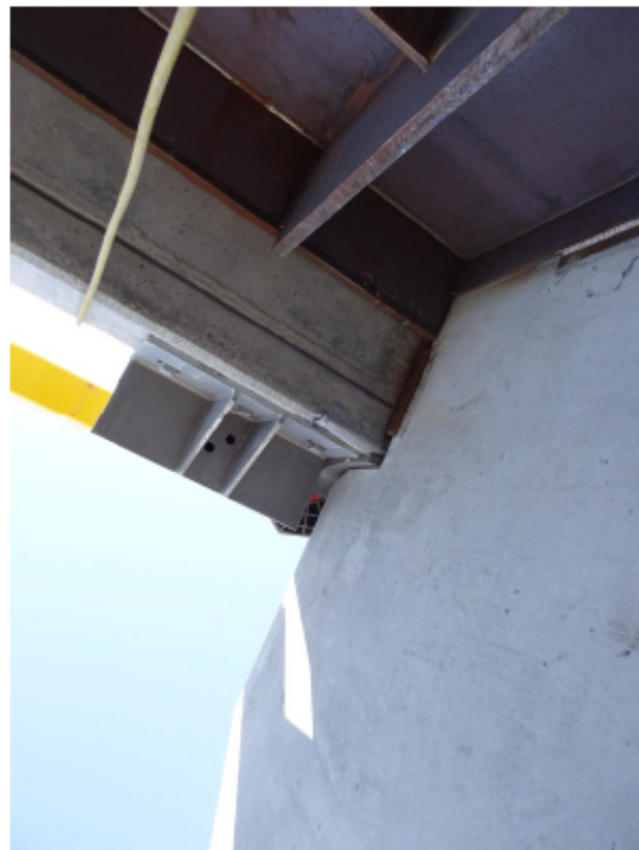
Figure 3: Railing connection and deck soffit (SE corner)
