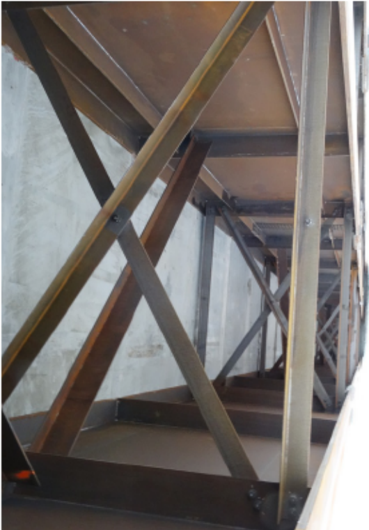
Figure 14: Typical bracing (looking NW)
