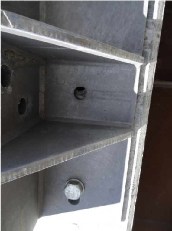
Figure 2: Bridge railing connection into deck (SW)
