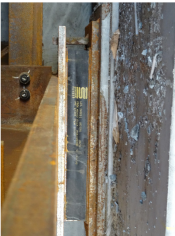
Figure 9: North centre bearing (front)
