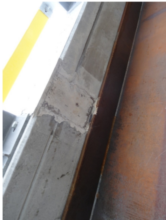
Figure 15: Typical cast-in-place deck joint (SE)
