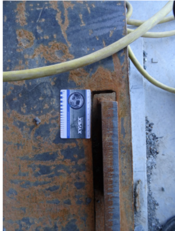
Figure 4: Remaining slot length (SE bearing outside)
