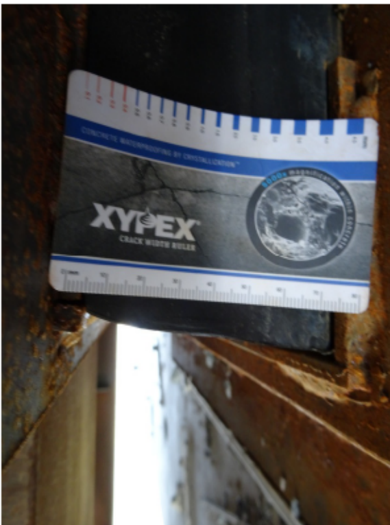
Figure 5: Front of south centre bearing (west side)
