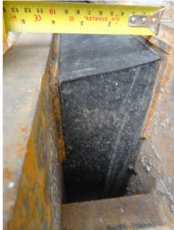
Figure 12: Typical bearing front (SE exterior)
