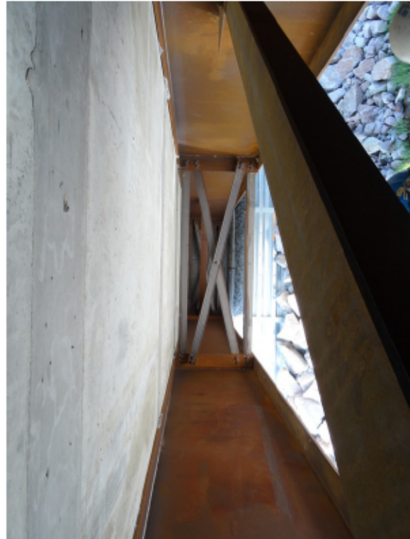
Figure 16: West bracing bay (looking north)
