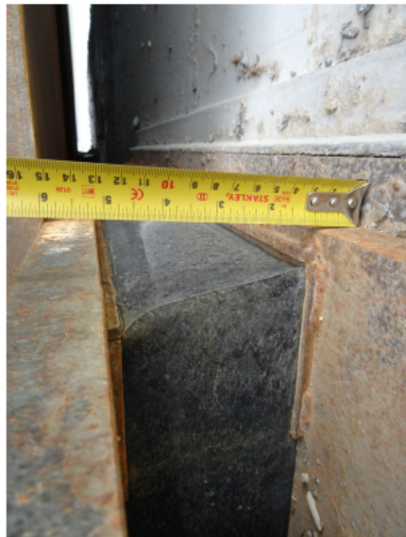
Figure 11: Typical bearing front (NW exterior)
