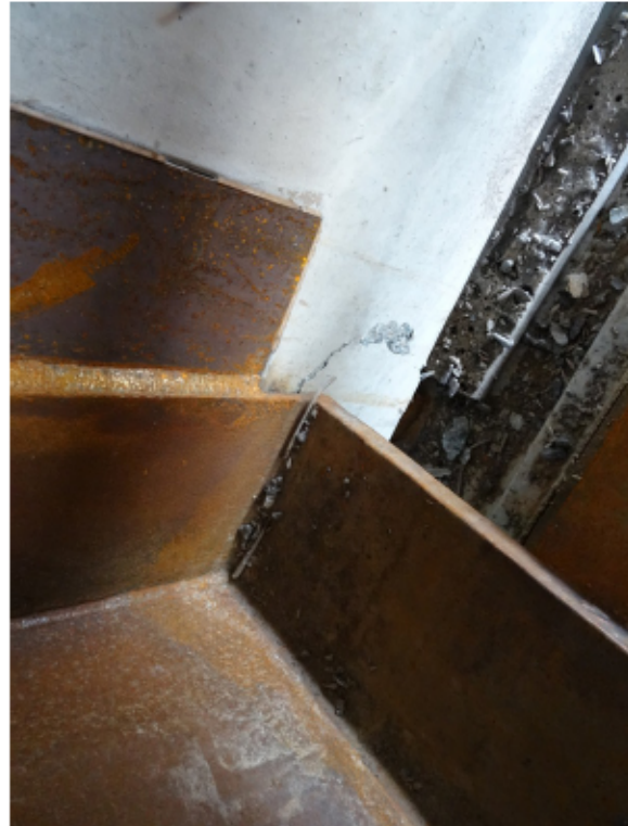
Figure 4: Evazote under south centre girder and ballast wall
