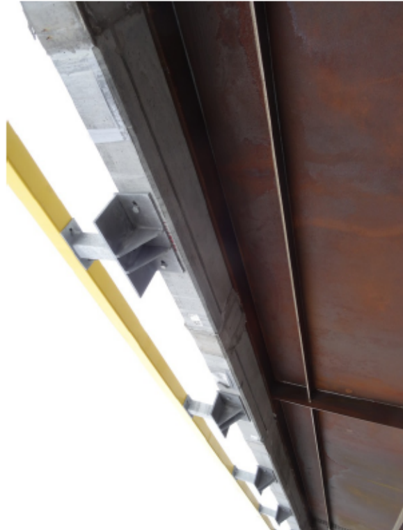
Figure 16: Typical deck edge and railing (SW)
