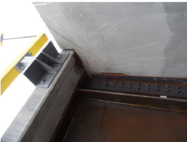
Figure 9: Railing installation (NE)
