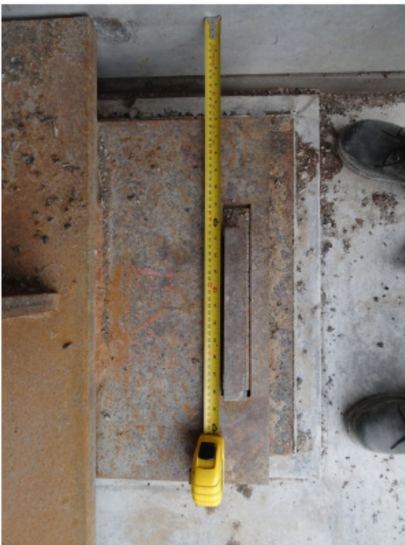
Figure 13: Typical bearing guide plate in slot (SW)
