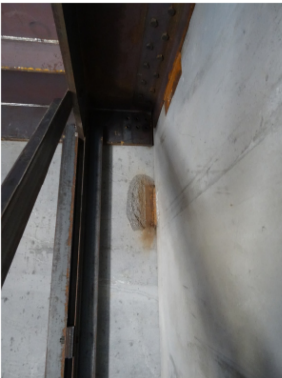
Figure 9: Spall in deck soffit, north centre girder (west side)
