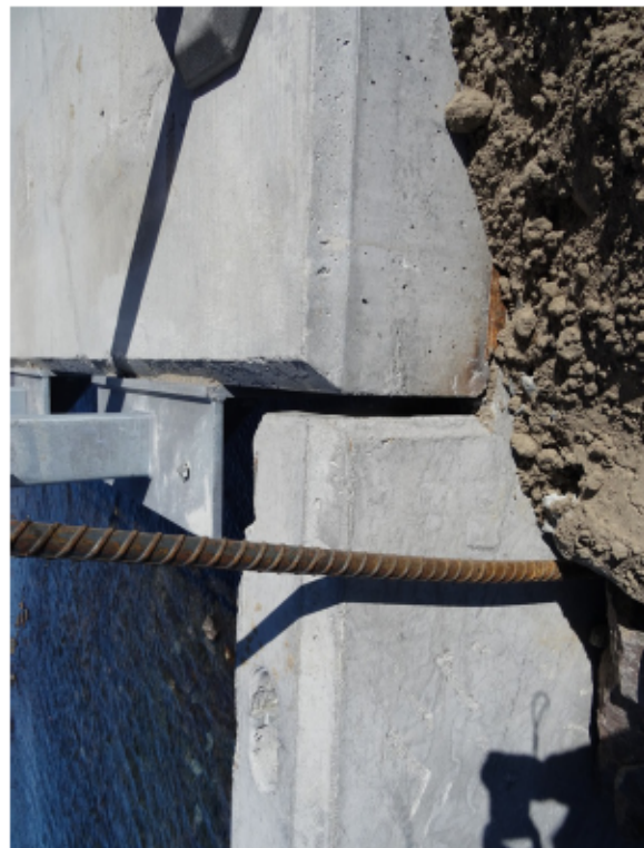
Figure 23: NE ballast wall and deck edge (note evazote missing in joint)
