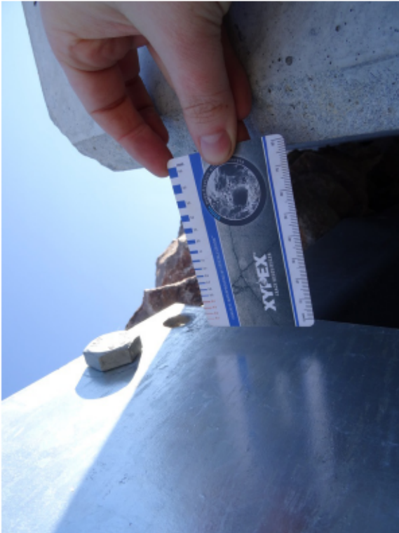
Figure 6: SE binwall and ballast wall gap (top)
