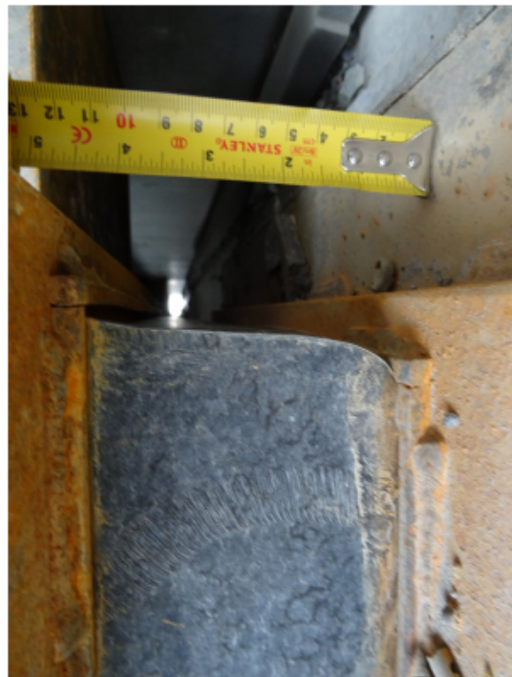
Figure 11: SW bearing back face
