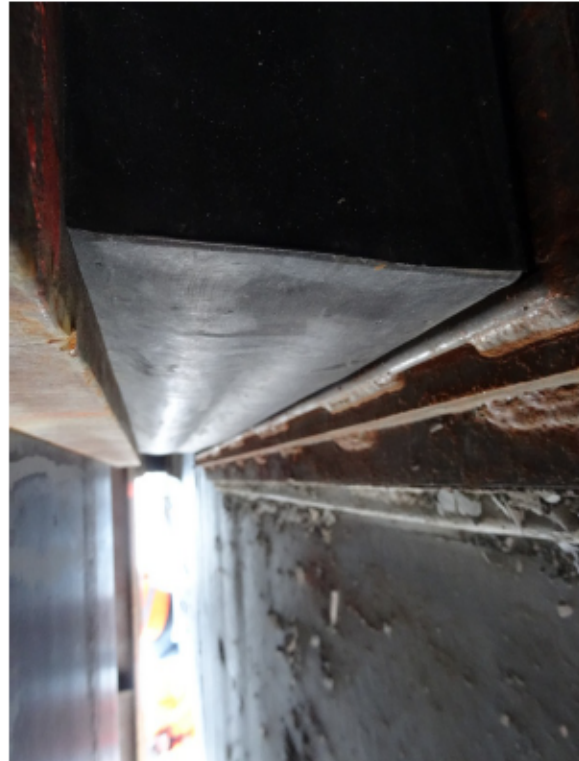
Figure 8: South centre bearing, front face
