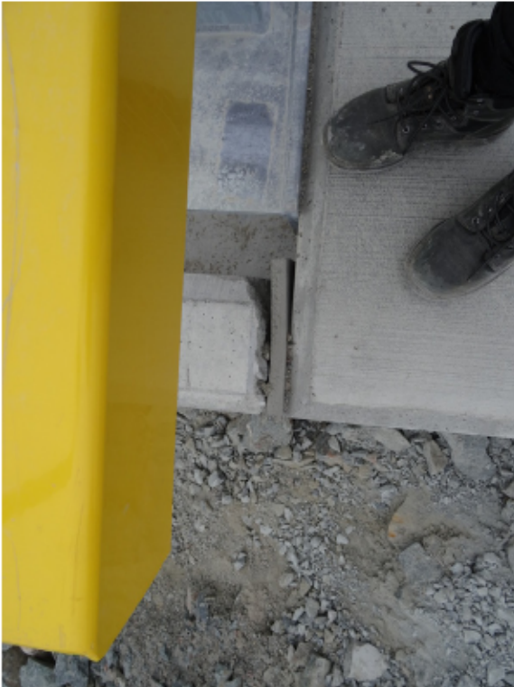
Figure 10: SW ballast wall and deck joint from above
