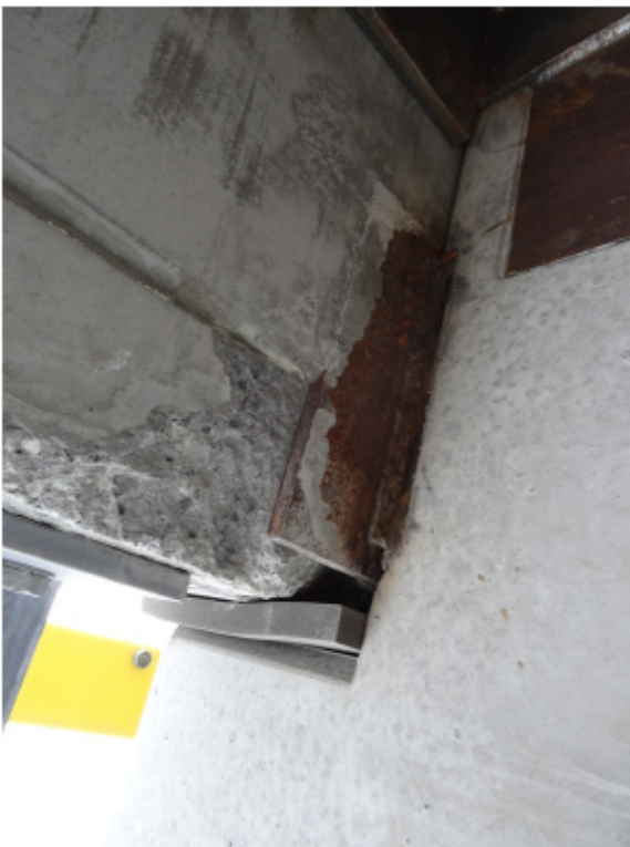
Figure 9: Spall in dek panel corner (SE)
