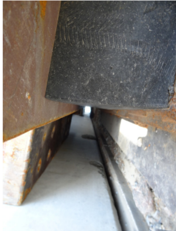
Figure 12: Typical back of bearing (NW top)
