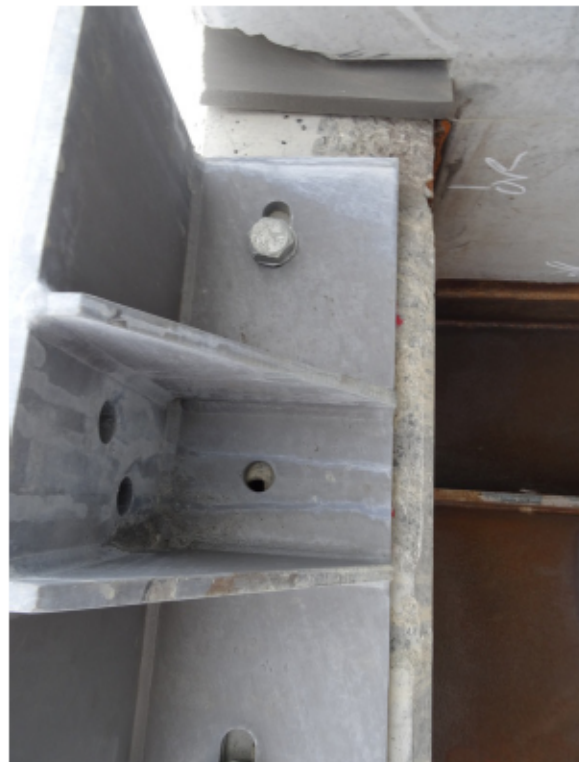
Figure 7: Railing bracket installation (SW end)
