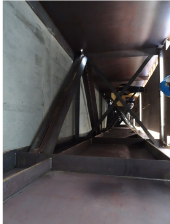
Figure 16: West internal bracing and temporary access platforms (looking south)
