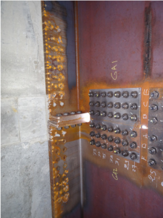
Figure 14: Typical girder splice top (NW first splice, west girder)
