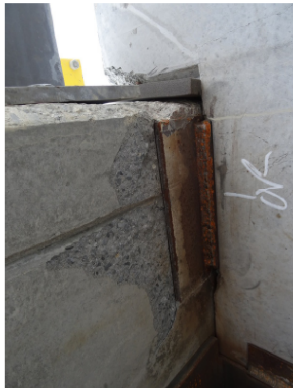
Figure 3: Minor spall in deck soffit (SW corner)
