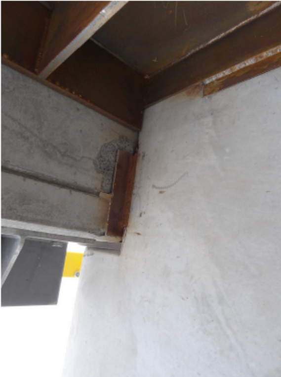
Figure 6: Minor spall in deck soffit (NW corner)
