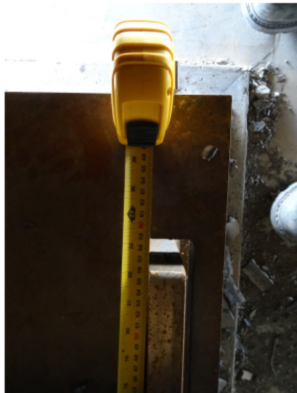
Figure 7: NE bearing remaining slot length
