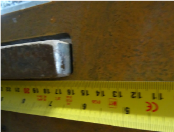
Figure 2: North centre bearing - remaining slot length
