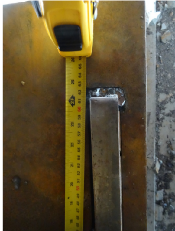
Figure 16: SW bearing front of slot cut by contractor (interior)
