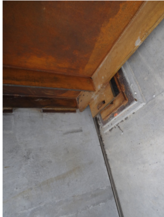
Figure 4: SE bearing slotted hole
