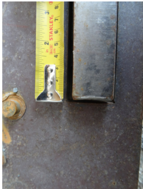
Figure 11: NW bearing remaining slot length
