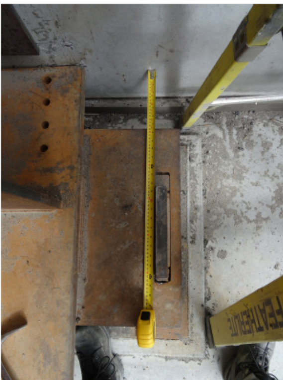
Figure 17: SW exterior bearing slot
