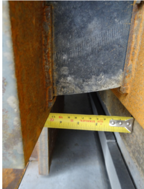
Figure 16: Typical rear of bearing (SE)
