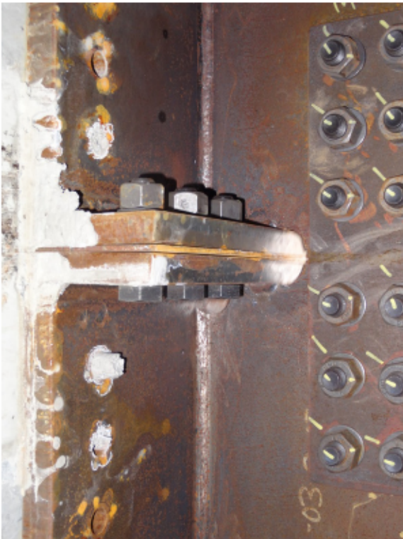
Figure 18: Top compression splice
