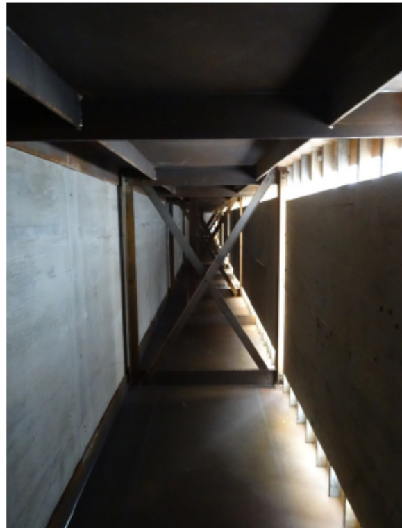
Figure 20: West bracing and temporary access platform (looking north)
