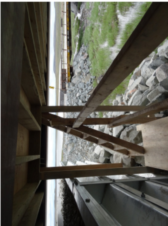
Figure 25: Temporary access to abutment
