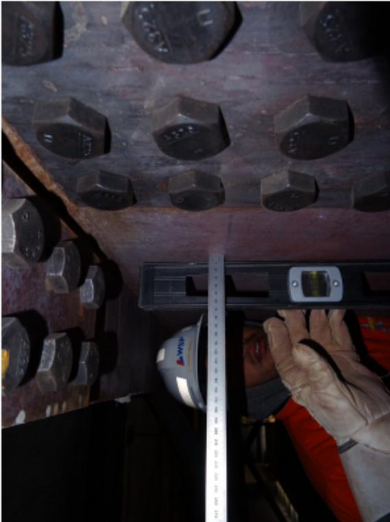
Figure 30: Typical girder web bowing effect
