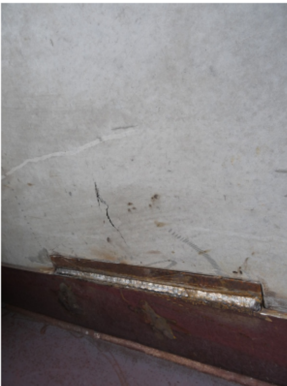
Figure 21: SW ballast wall weld to end of girder
