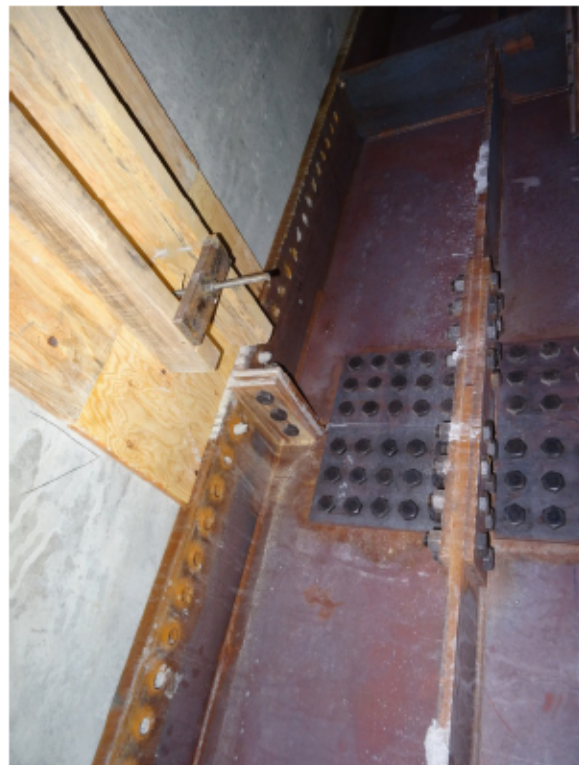
Figure 31: Typical splice and deck joint formwork
