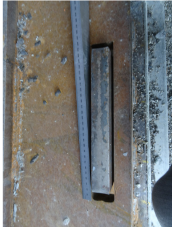
Figure 24: SW bearing slotted hole
