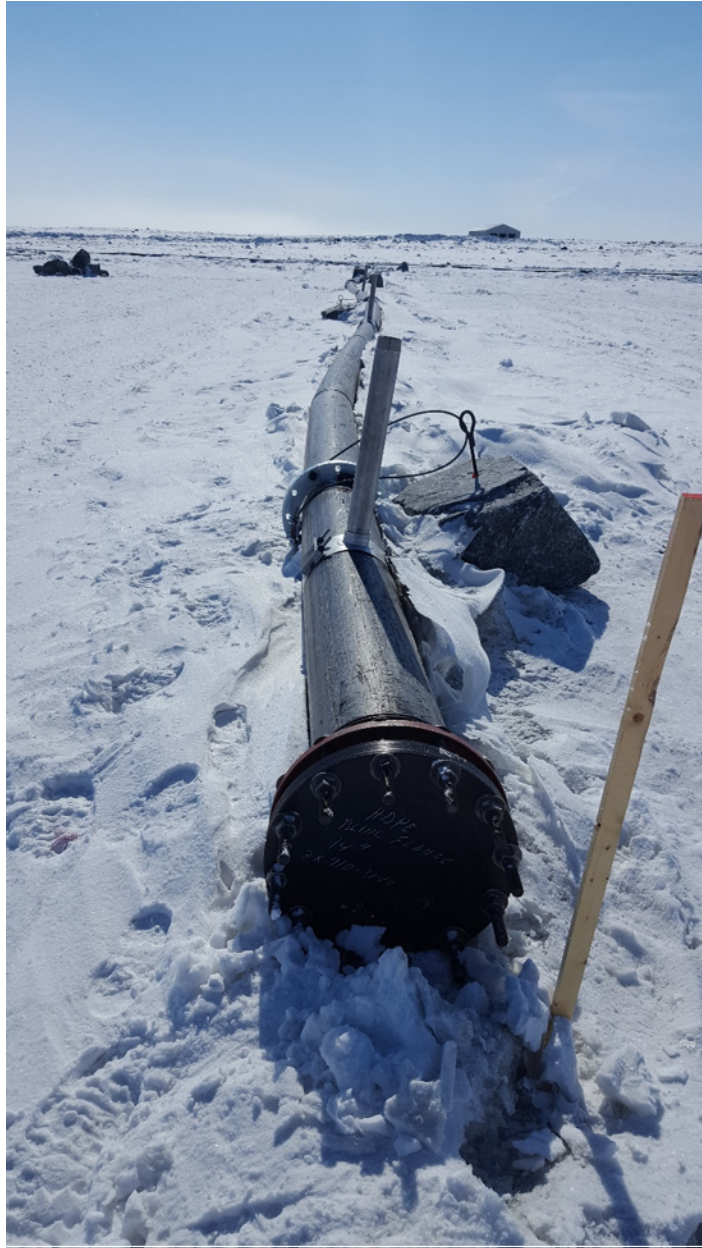
Photograph 1 – View of the West summer diffuser installed on the icesheet (looking SE). The blind flange, discharge port and ballasting can be observed
