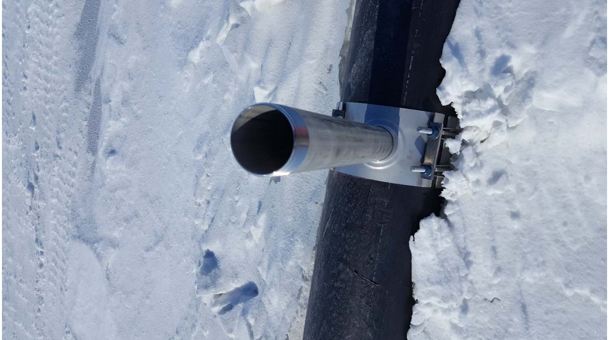
Photograph 4 – View of one of the discharge port
