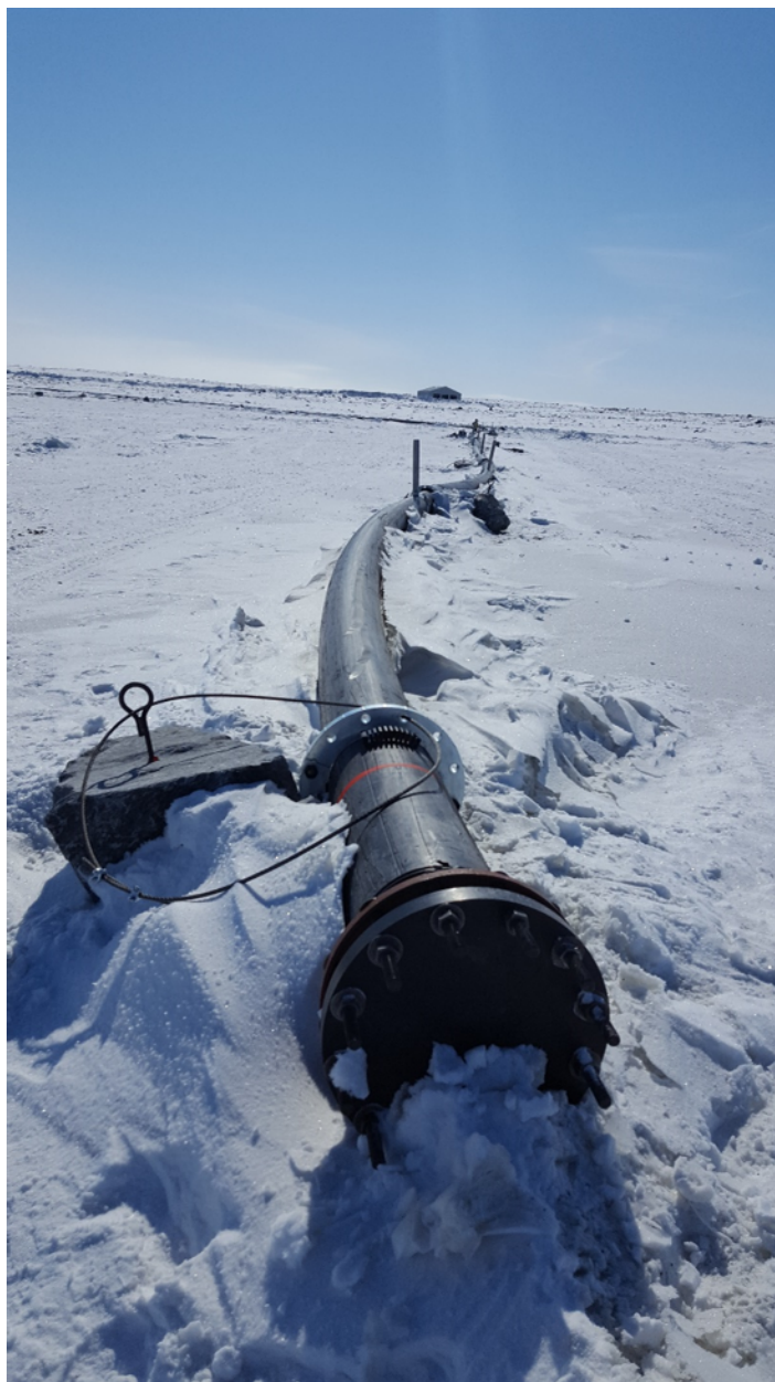
Photograph 2 – View of the East summer diffuser installed on the icesheet(looking SE). The blind flange, discharge port and ballasting can be observed
