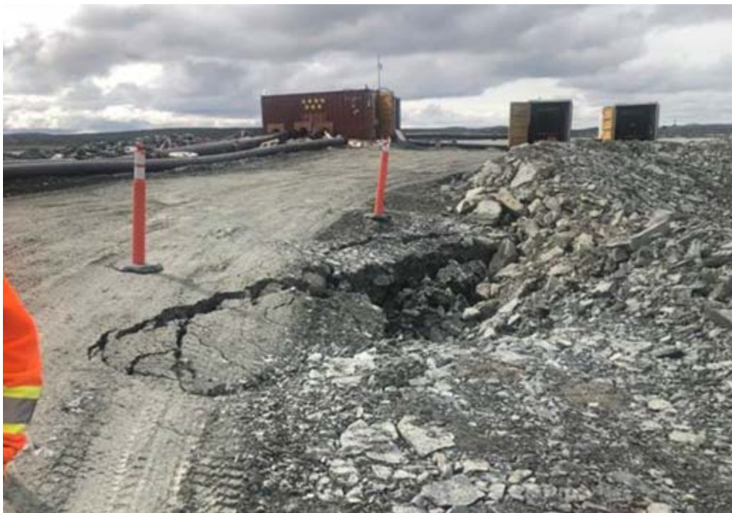
Picture 18 – Observation of instability in the widened portion of the Phase 1 Dewatering Ramp (July 10 2019)
