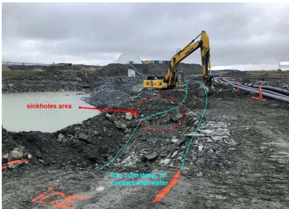
Picture 20 – Removal of snow and ice in the widened access road to the Phase 1 Dewatering Ramp (July 11 2019)
