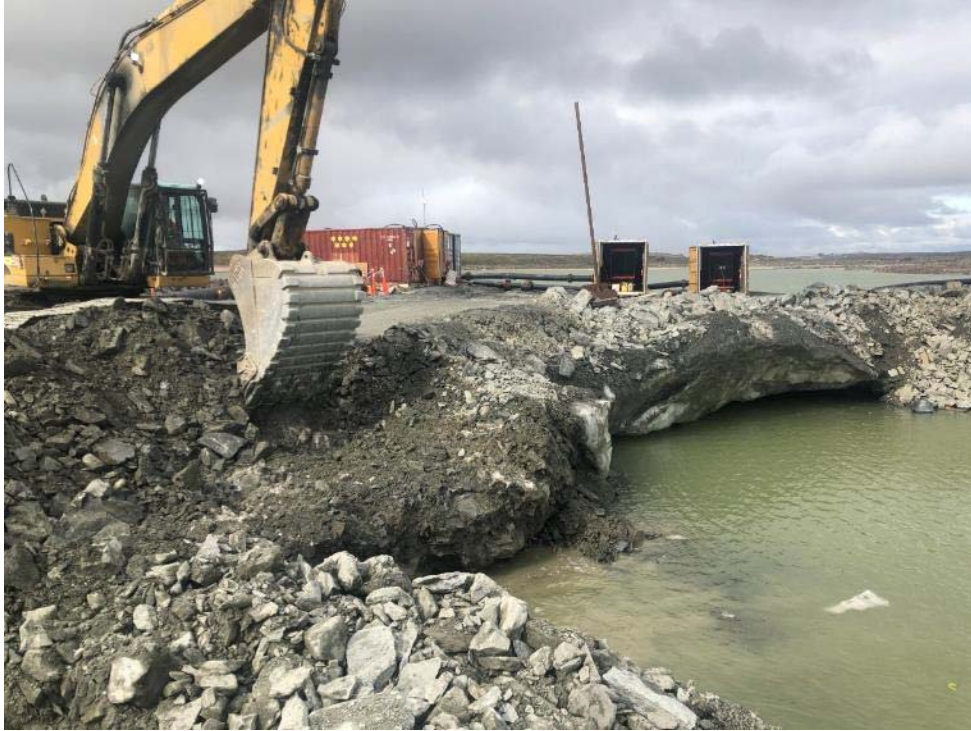
Picture 19 – Removal of snow to mitigate instability in the widened access road to the Phase 1 Dewatering Ramp (July 11 2019)
