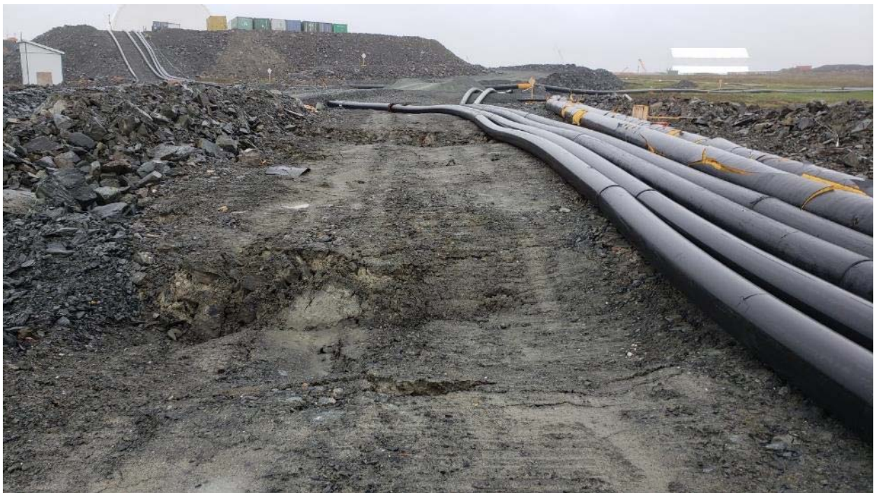
Picture 15 – Construction of the Phase 2 of the Ramp. Placement of rockfill material to construct the access road perpendicular to the Phase 1 Ramp. Picture taken from Phase 1 dewatering pad (April 20, 2019)
