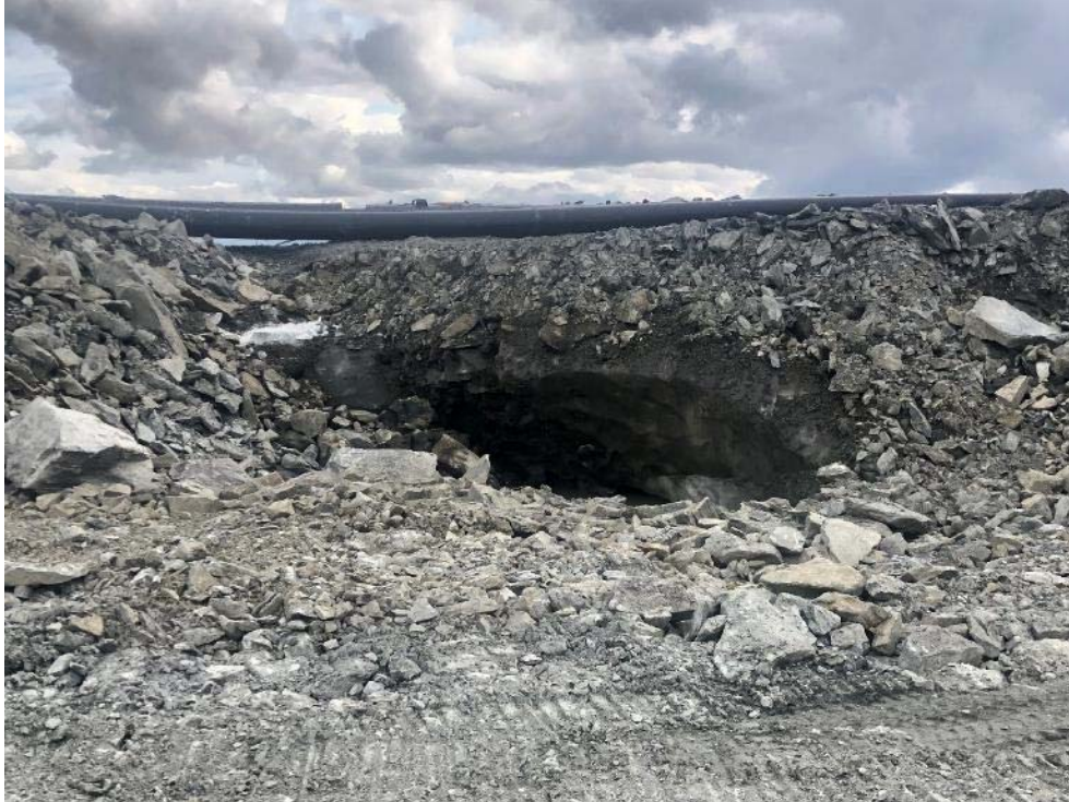
Picture 17 – Observation of ice and snow in the foundation of the old access to the Phase 1 Dewatering Ramp (July 8 2019)
