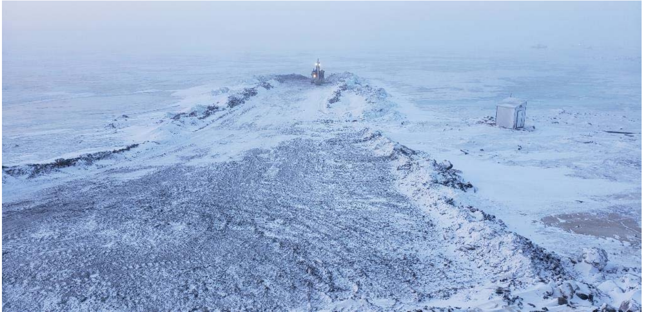
Picture 3 – Construction of the Dewatering Ramp access. Ice blocks are excavated and placed on the side of the ramp (January 14, 2019)
