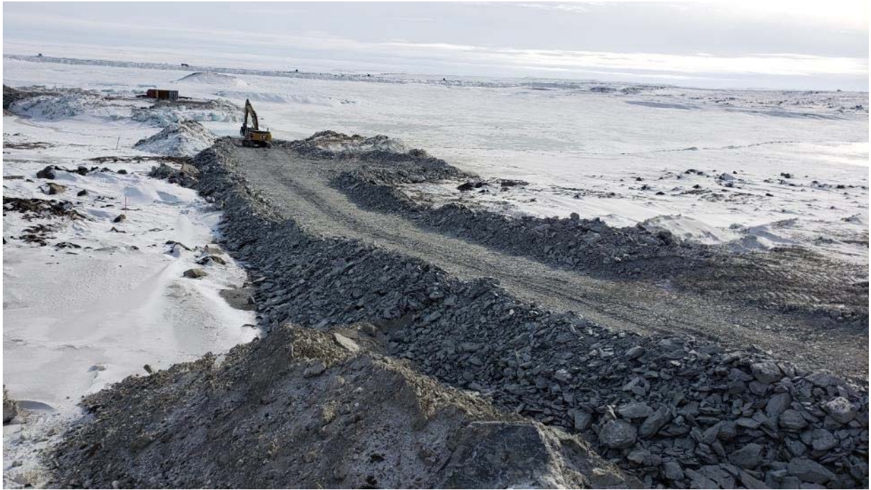
Picture 13 – Construction of new access to lower the dewatering ramp pump pad (Phase 2) (April 14, 2019)
