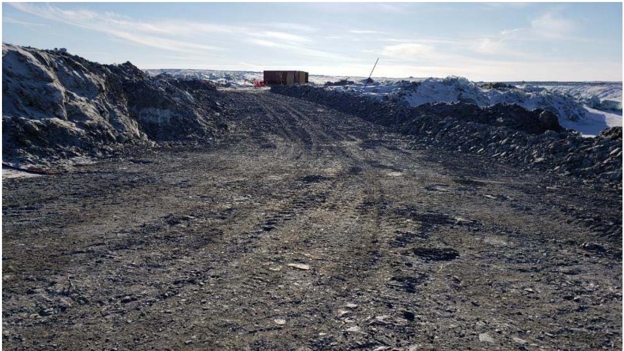
Picture 12 – View of the new Dewatering Ramp access built to mitigate instability (April 12, 2019)
