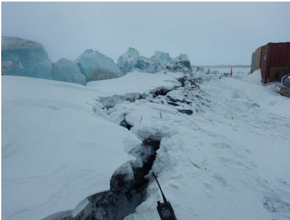
Picture 8 – Observation of tension crack in the bumper area of the pump pad of the Dewatering Ramp (March 25, 2019)
