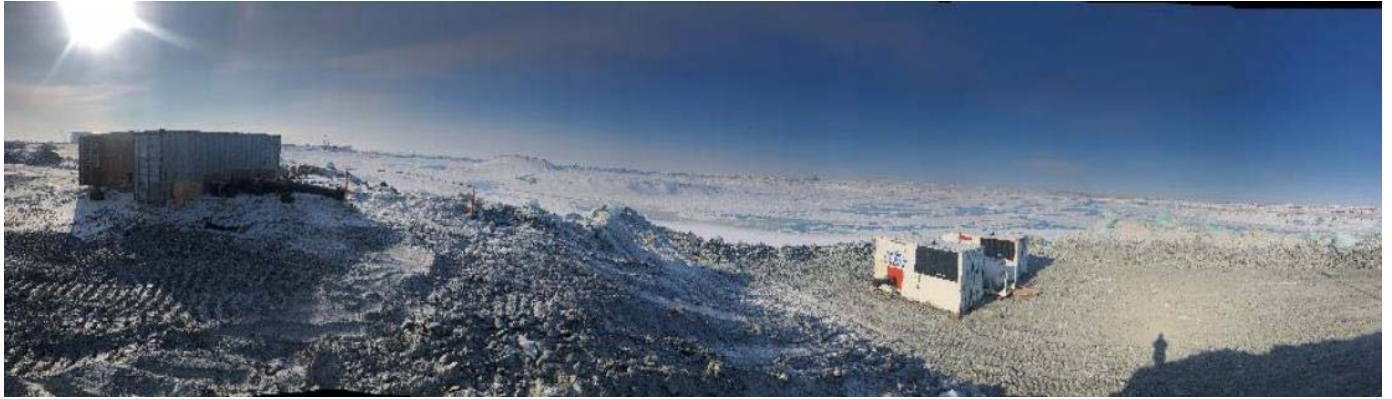
Picture 15 – Construction of the Phase 2 of the Ramp. Placement of rockfill material to construct the access road perpendicular to the Phase 1 Ramp. Picture taken from Phase 1 dewatering pad (April 20, 2019)
