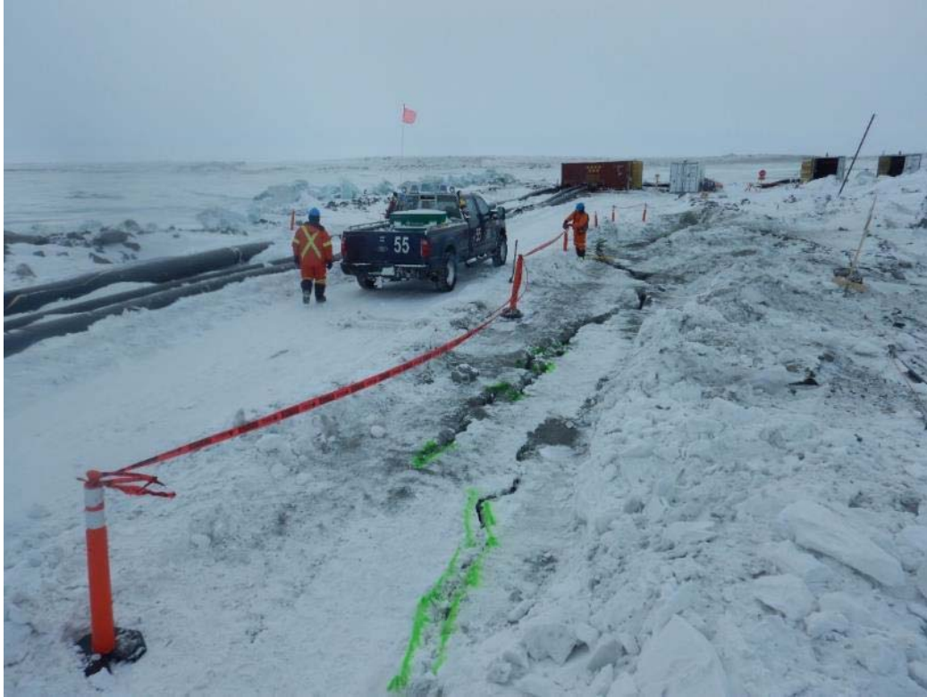
Picture 7 – Observation of tension crack in the bumper area of the access to the Dewatering Ramp (March 25, 2019)
