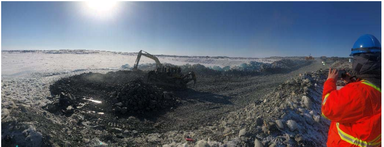
Picture 14 – Construction of the Phase 2 of the Ramp. Placement of rockfill material to construct the access road perpendicular to the Phase 1 Ramp. Picture taken from Phase 1 dewatering pad (April 16, 2019)
