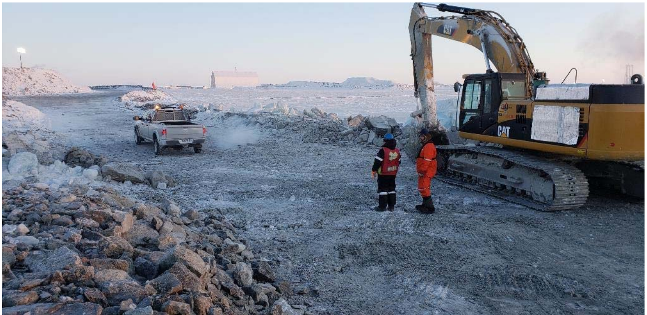
Picture 4 – Construction of the Dewatering Ramp access. Ice blocks are excavated and placed on the side of the ramp (January 17, 2019)
