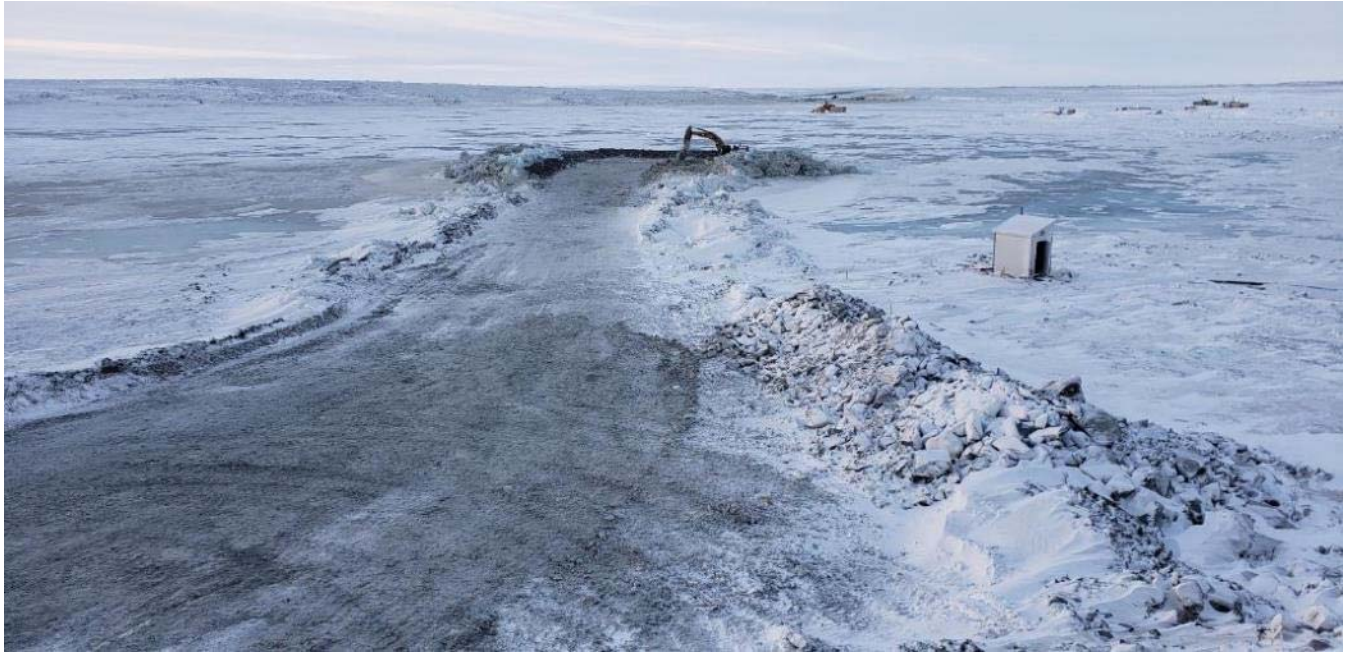
Picture 5 – Construction of the Dewatering Ramp pump pad. Placement of rockfill material in water with an excavator (January 20, 2019)
