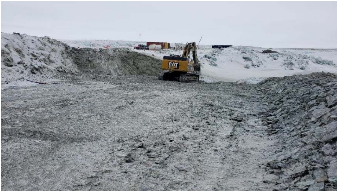
Picture 10 – Widening of the Dewatering Ramp access (construction of a parallel access) to mitigate instability (April 10, 2019)
