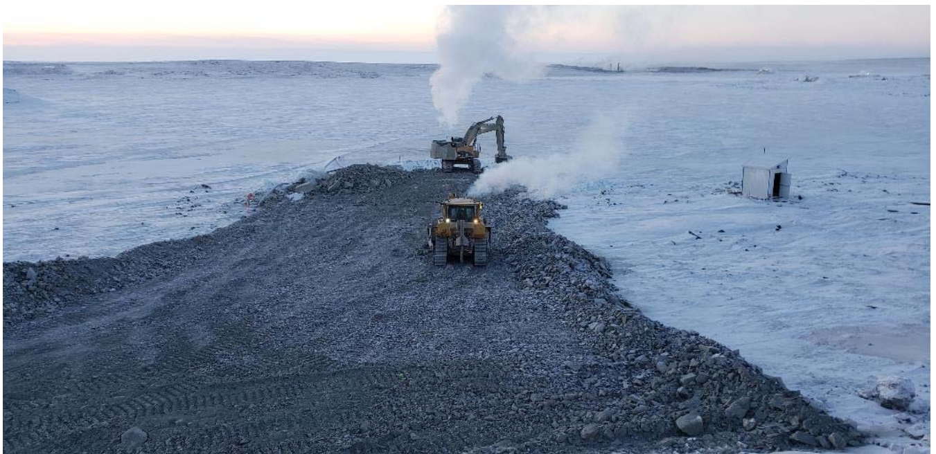
Picture 2 – Removal of ice and snow and placement of rockfill material over land for the Dewatering Ramp construction (January 11, 2019)
