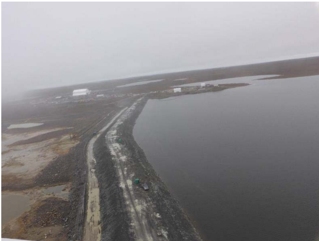
Photo 14. Aerial view of WTD downstream area. View of the dewatering line going toward Mammoth Lake while the seepage discharge line is being installed (September, 2019)
