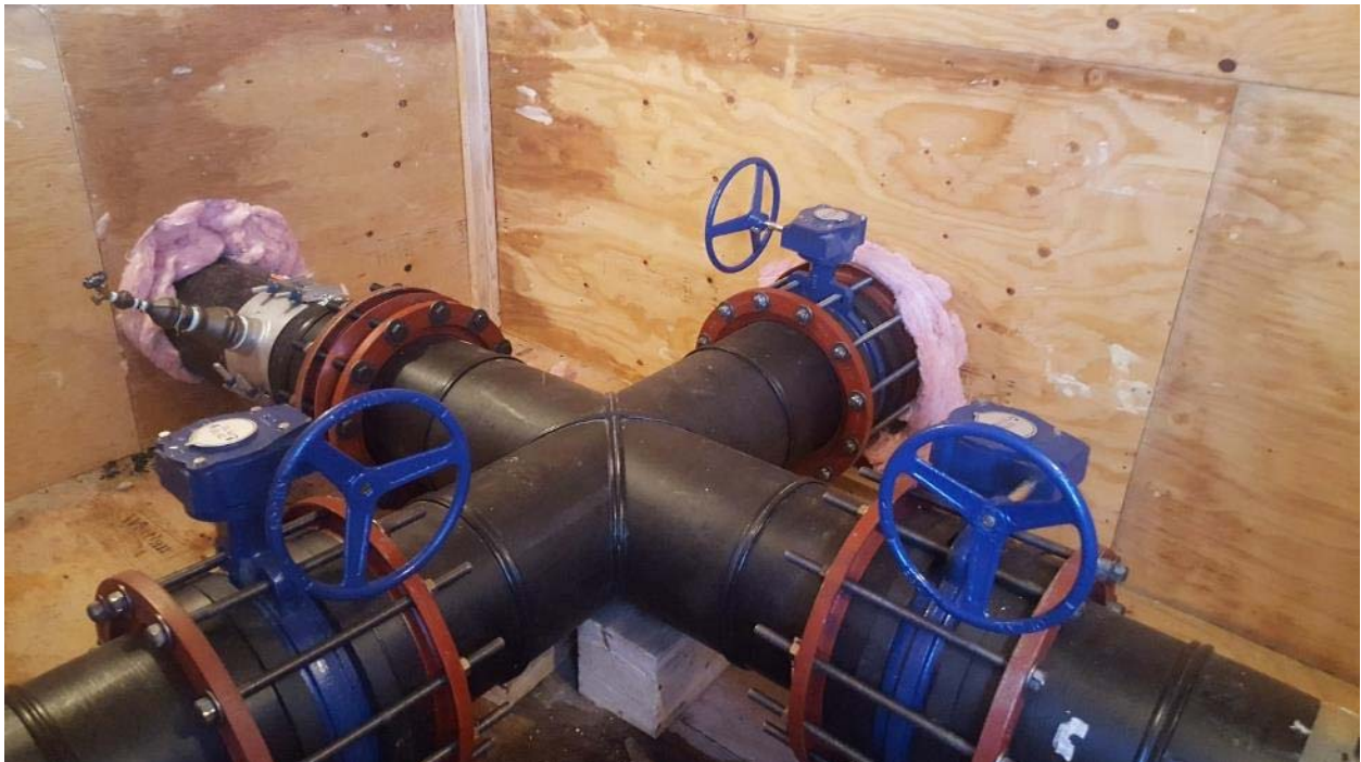
Photo 10. Interior view of the 3:1 reducer and sampling port (March, 2019)
