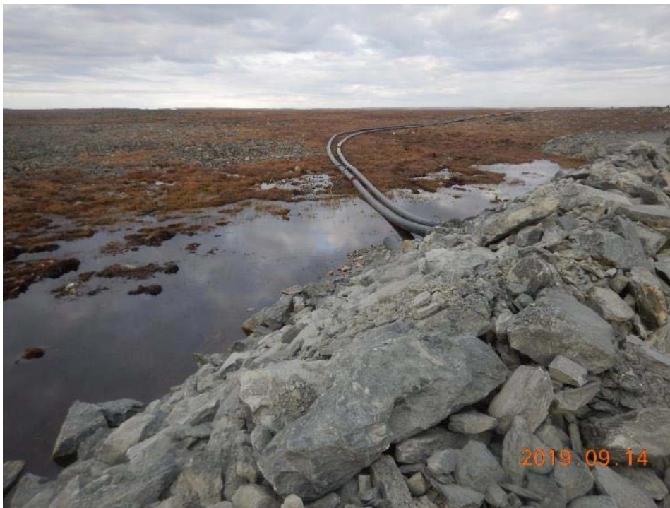
Photo 16 : Dewatering line going toward Mammoth Lake dewatering diffuser (September 2019)
