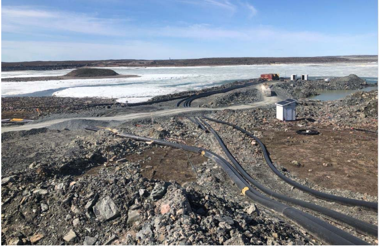
Photo 13. Piping from Dewatering ramp to WTP and then to WTS or Mammoth (May, 2019)
