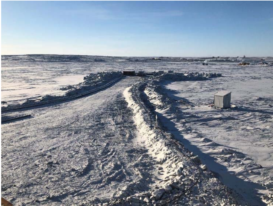
Photo 2. View of the header seacan, 3 HL 250 on the Phase 1 Dewatering ramp and the discharge pipe to WTS (March, 2019)
