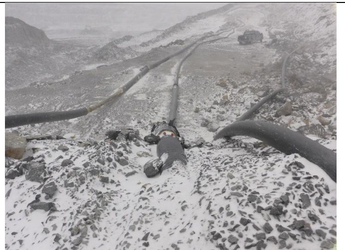
3.2 Old insulated section of line 114 crossing Road 7 straight in the rock, near Quarry 1.
