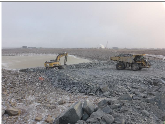
4.1 Backhoe preparing the ground for the bulldozer and loader bringing a load of muck
