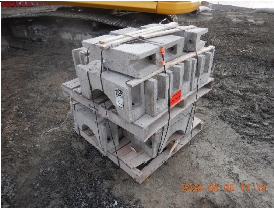
3.3 Concrete ballasts ready to be installed
