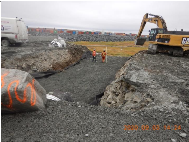
2.1 Dike D1 overflow culvert near camp
