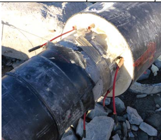
2.5 Six channel heat traced
