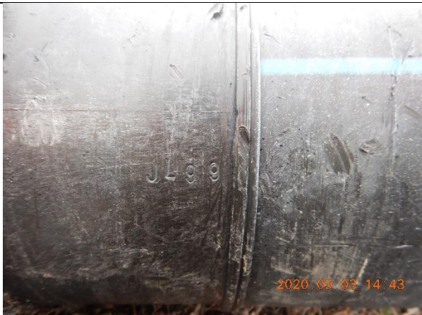
1.1 Fused pipe with punch on line 113, for tracking fusion parameters
