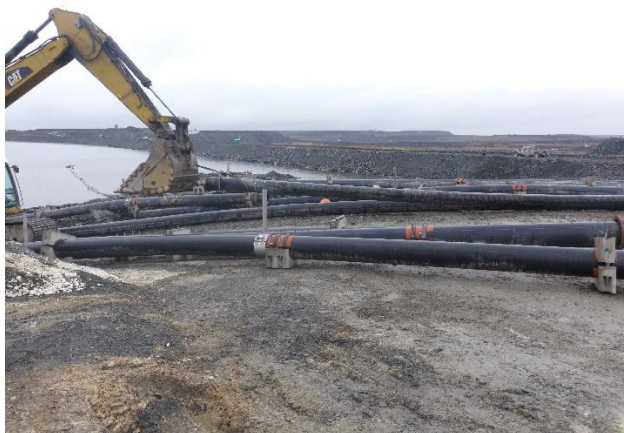
1.5 Last portion of piping being brought on site.
