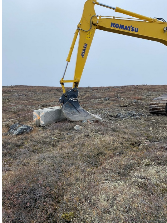
1. Area where the pipeline to the WTS will be installed
