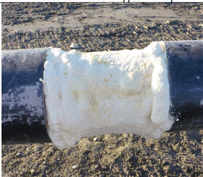
2.3 Urethane over the tape to insulate the pipe
