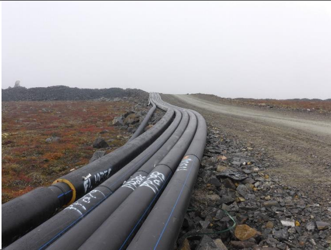
2.1 Fused pipe stockpile near the road leading to the fusion pad.
