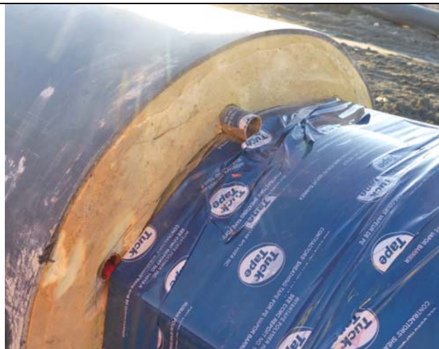
2.2 An empty channel for the temperature probe
