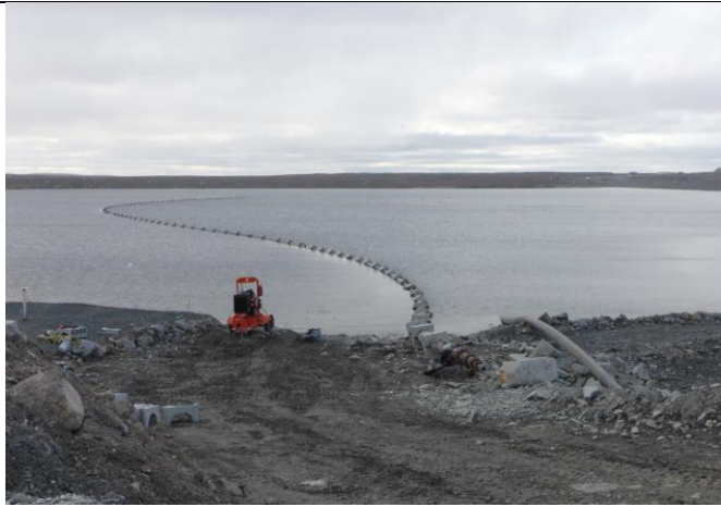
1.1 Winter diffuser before being pulled.
