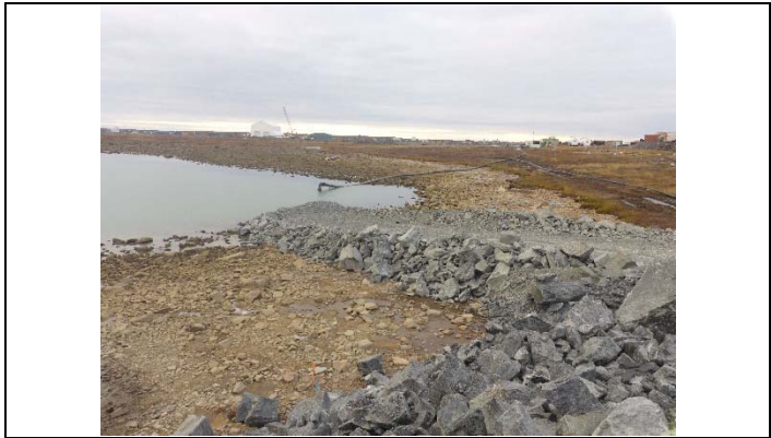
2.1 The pad of lake A-53 has been extended.
