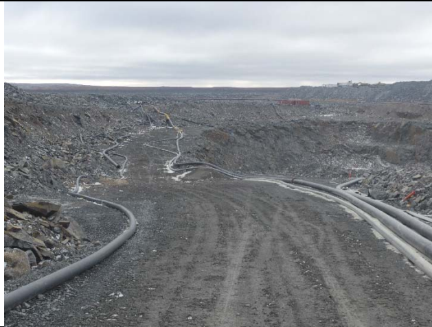
3.1 Line 114 passing on the inner right hand side of the road to Quarry 1.
