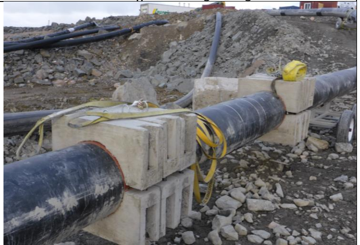
1.4 Installation of ballasts on the insulated part of the winter diffuser.
