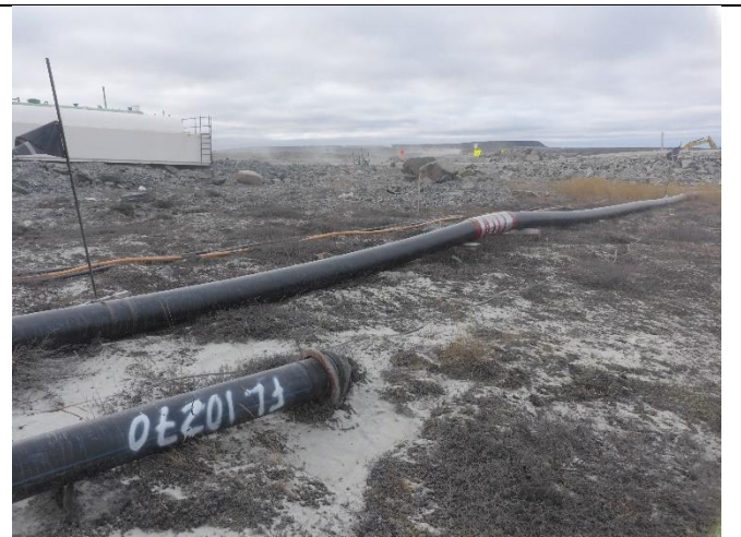
2.2 West end of the section of line 113 & 115 leading to IVR attenuation pond. Regarding West, with the Road 7-Nemo Road intersection in the background
