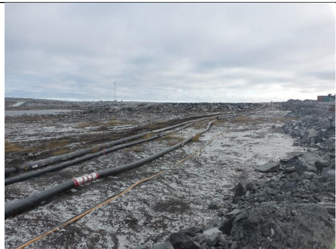
2.1 Line 113 & 115 laid on the ground North of the Orbit pad, regarding East.
