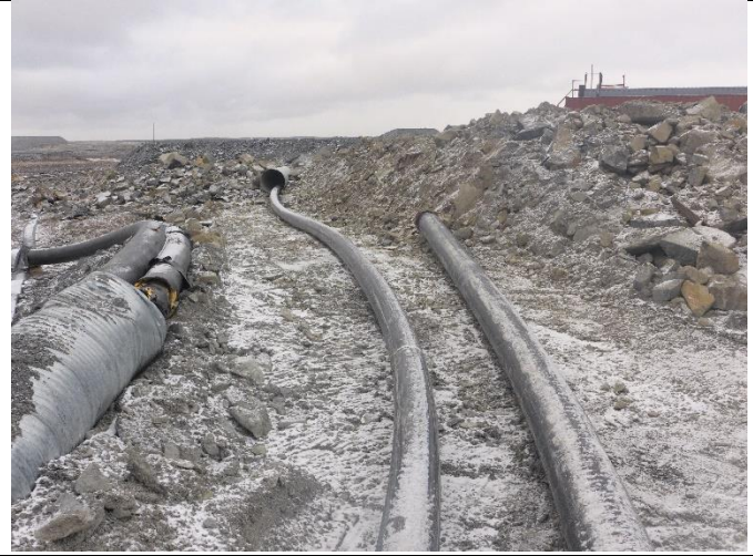
1.1 Whale Tail South diffusers extensions towards the WTP.
