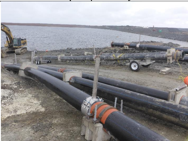
1.4 Pipe placed on trailers and diffuser outlets installed.
