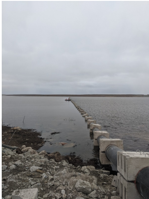
7. Final alignment of the diffuser in the WTS basin
