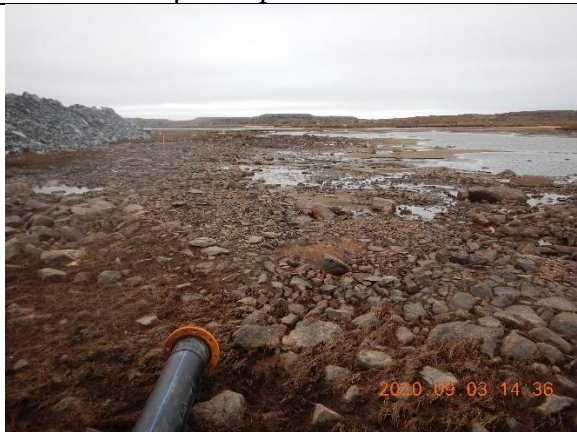
1.3 Line 113 pipe near A-47 and stakes for pad construction
