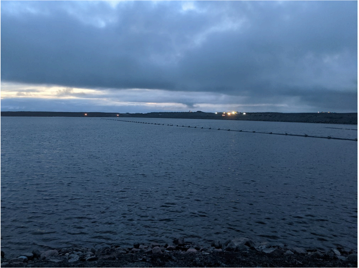
8. Final result before sinking
