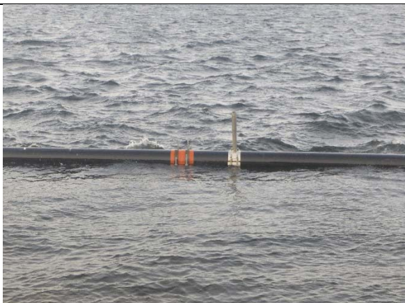
1.2 Ballast placement that was corrected compared to the outlet
