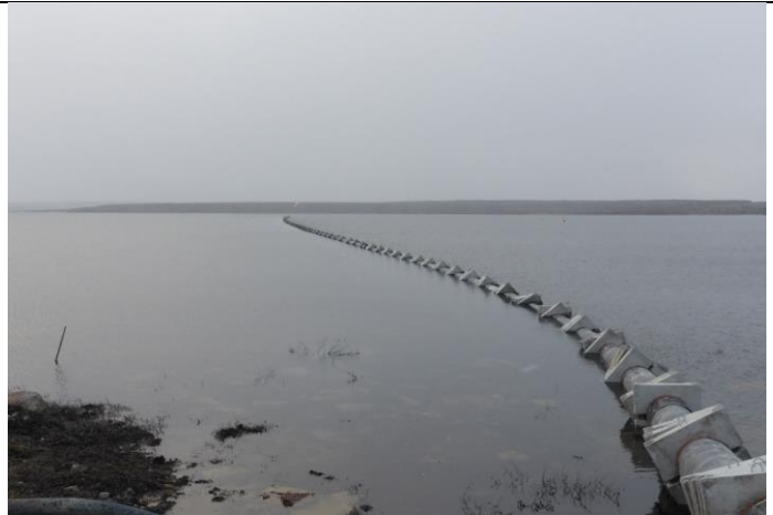
1.2 Winter diffuser being straightened.
