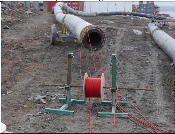
1.4 Insertion of the heat trace
