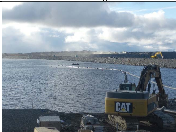
1.3 Summer diffuser being placed in the Whale Tail South Lake
