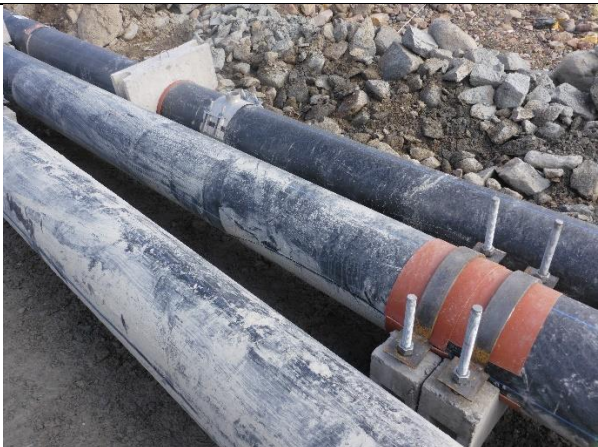
1.2 Changed ballast configuration to ensure adequate floatability.
