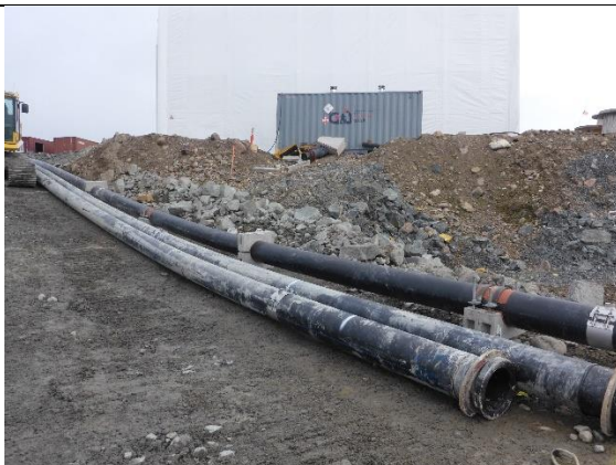
4.3 Concrete ballasts installation at the WTS diffuser
