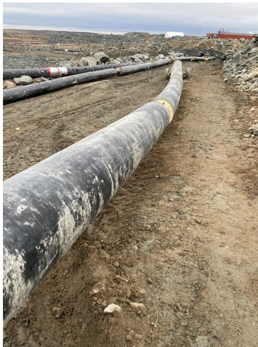
2. View of the installed pipeline
