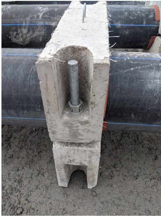
4. Illustration of a 90kg concrete ballast installed along the diffuser
