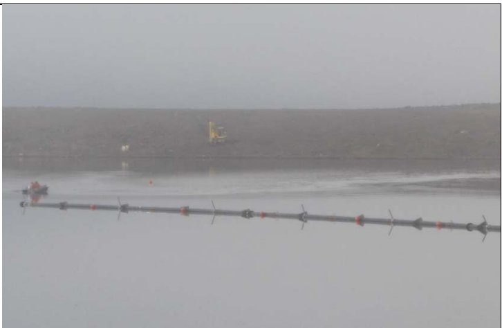
1.2 Excavator on the West shore of WTS and a boat to place the diffuser
