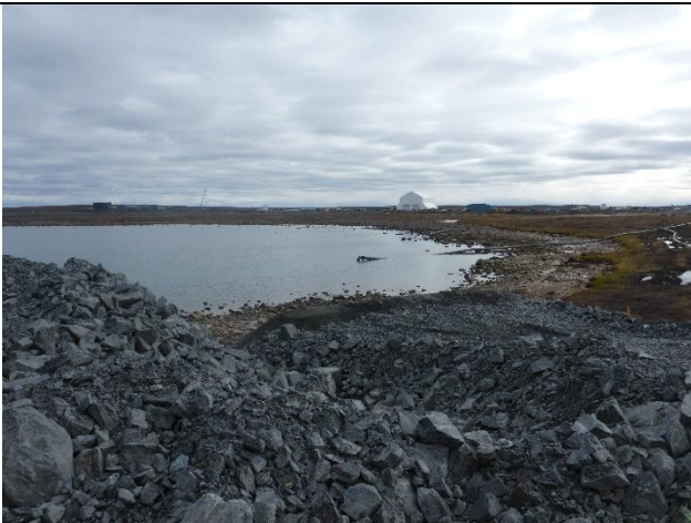
3.1 Pad of lake the A-53 that needs to be extended
