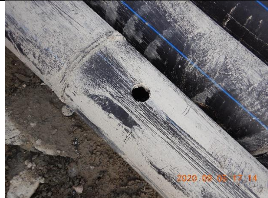
3.2 Hole drilled prior to installing branch saddle
