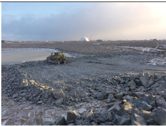
4.2 Bulldozer extending the pad
