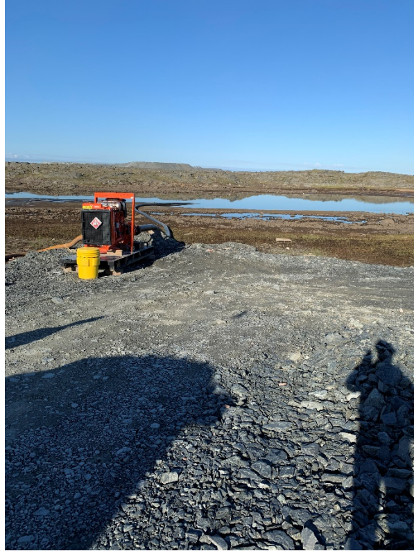
A47 pump and pad
