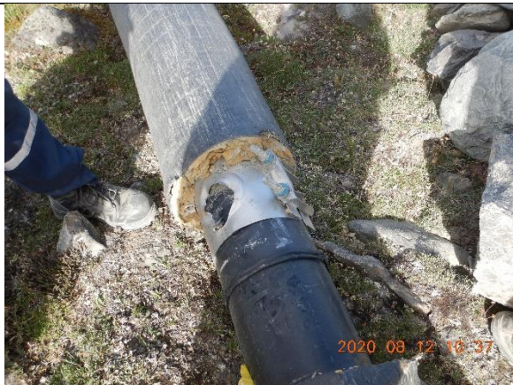
1.1 Holes underneath saddle for former paddlewheel
