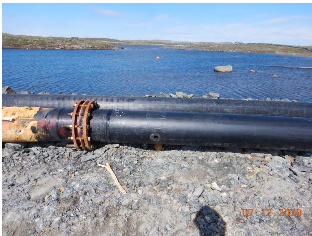
Photo 1. Instrument hole in the line 648-200-WFR-PC11-0214, NE Dike
