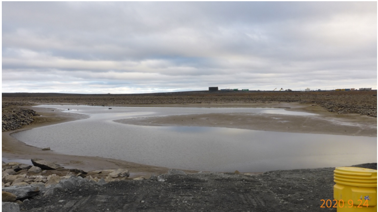
A53 pond after dewatering
