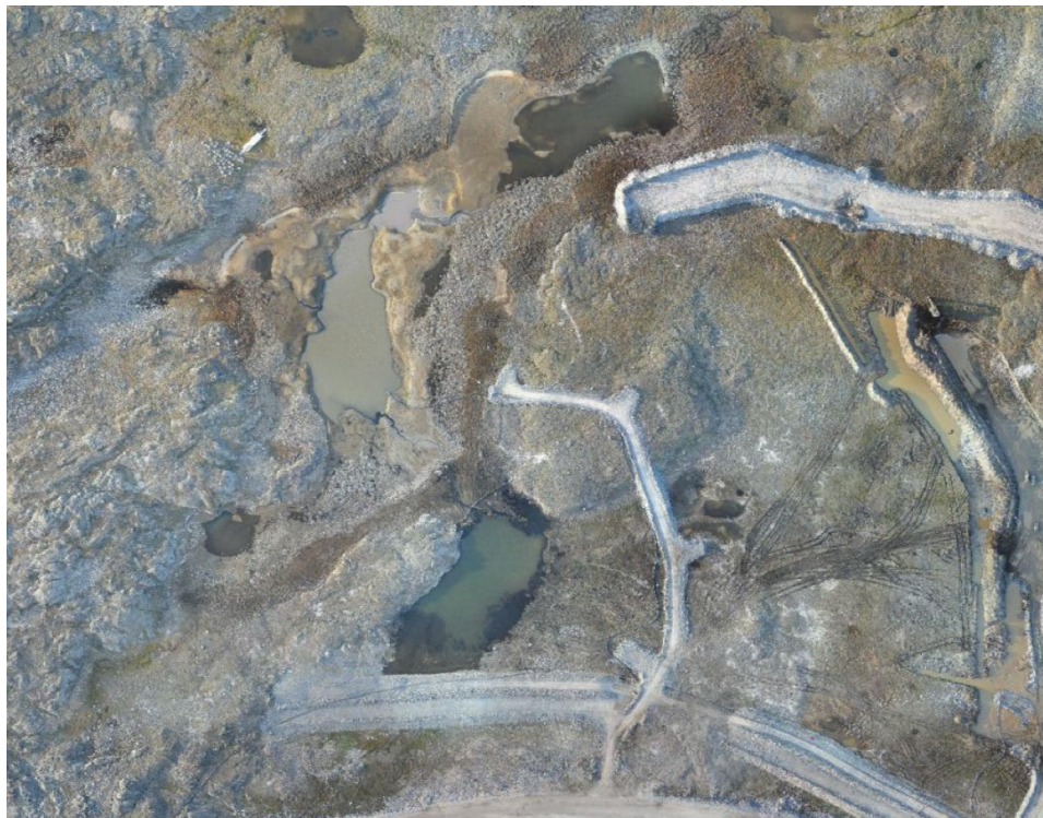
A47 during pumping
