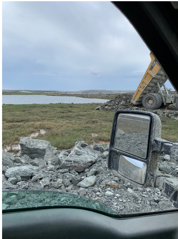
A50 access road construction
