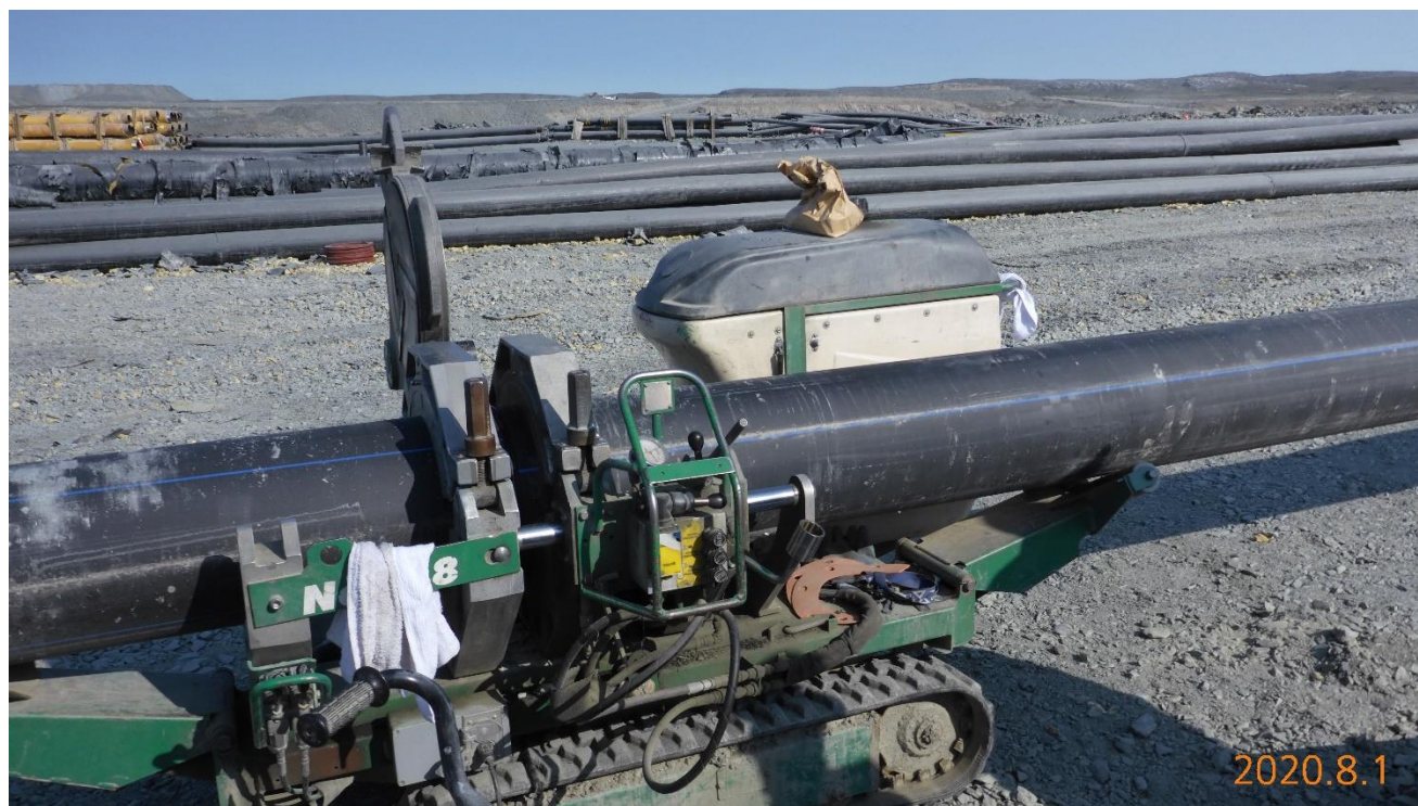
Photo 1. Pipe fusion on 14" DR17 (Blue line)
