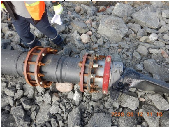
1.5 Reducer 14"x12" at mineflex connection
