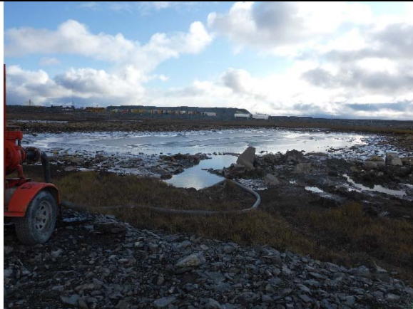
1.3 Lake A-50 being dewatered.
