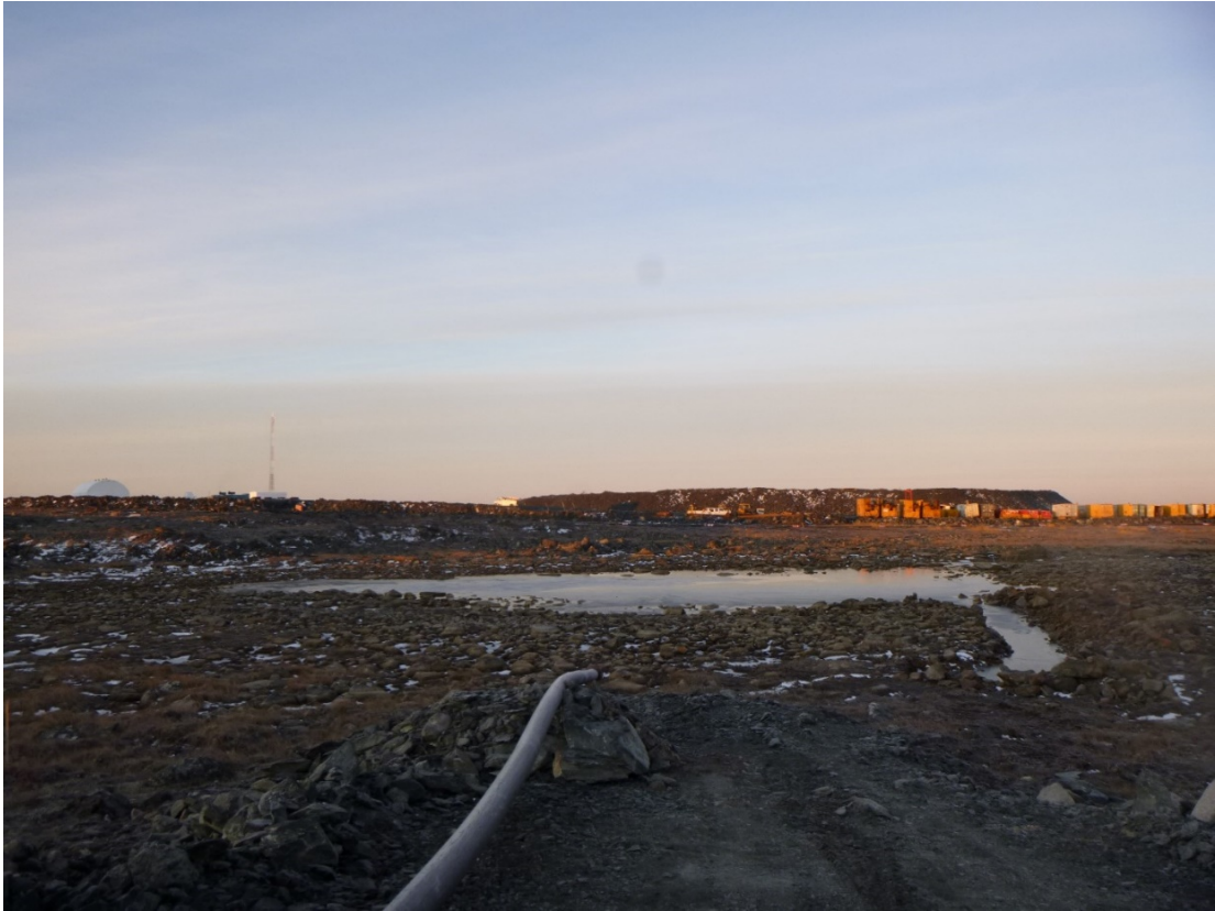
A51 pond after dewatering
