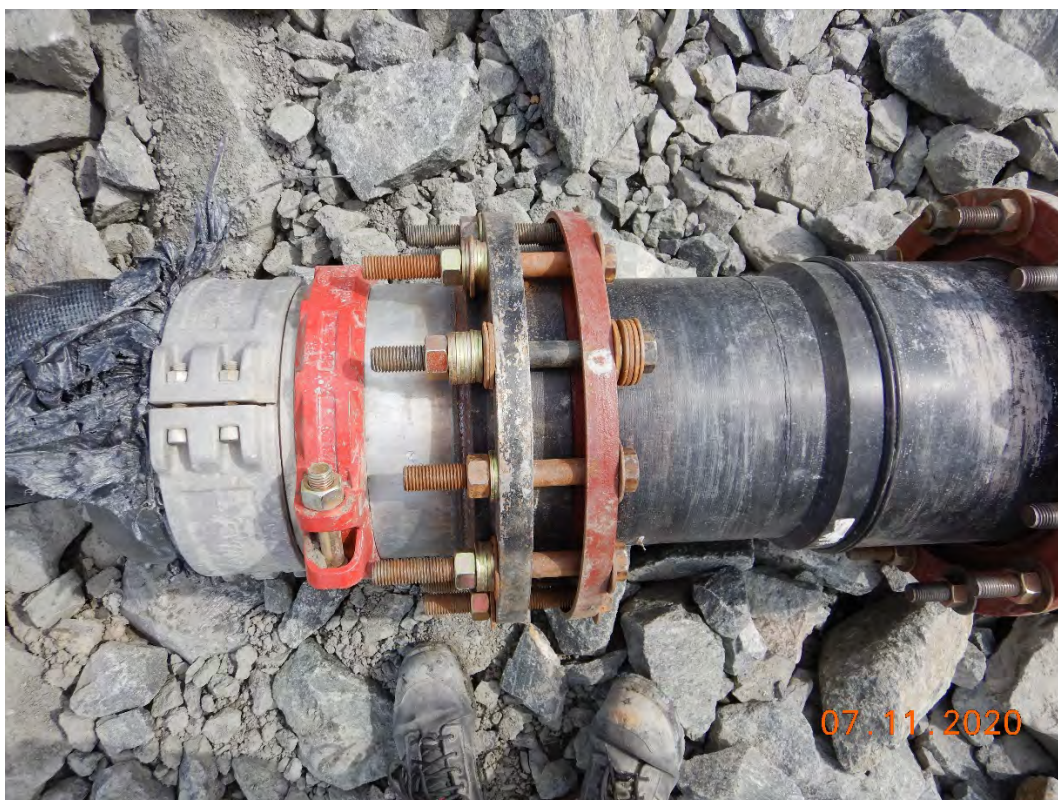
Photo 1. Mineflex hose connection with multiple washer, North of the culvert of AP-5
