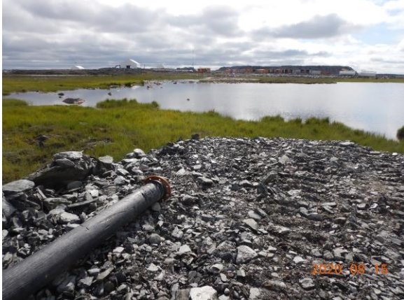
3.1 A50 pumping station, pump and suction to be installed
