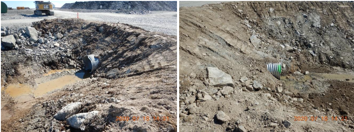
Photo 1. Culvert crossing ring road by AP5
