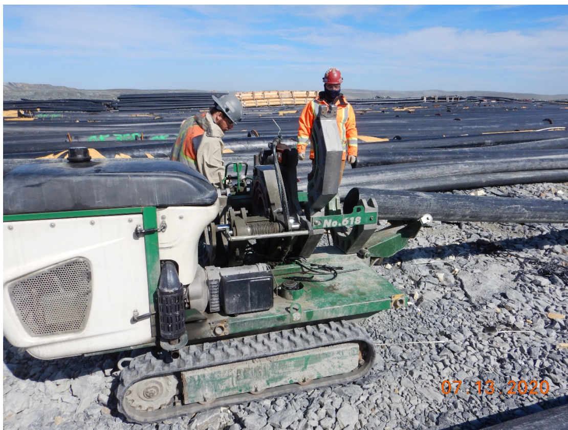
Photo 1. Ongoing fusion on old 8" DR11 Pipe, Fusion Pad
