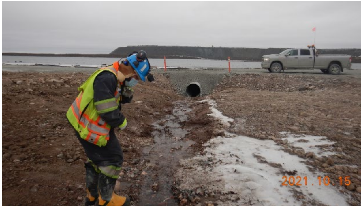
Photo 5. Installed culvert 22-2 with overlaying protective layer with excavated inlet, looking North.
