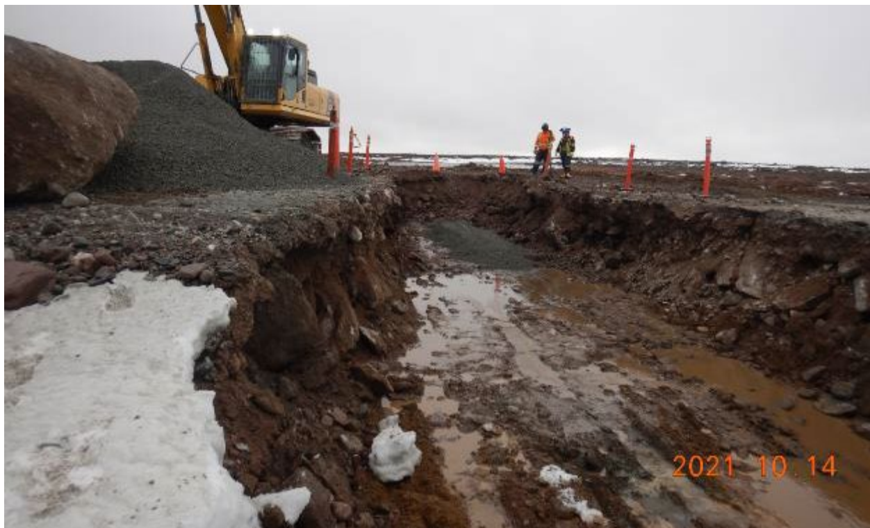
Photo 4. Placement of fine filter layer (0-3/4\"), culvert 22-2, looking South.
