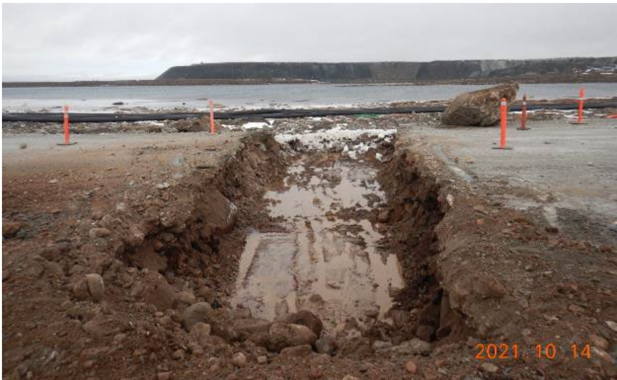
Photo 2: Excavation of the road material to install the culvert 22-2, looking North.
