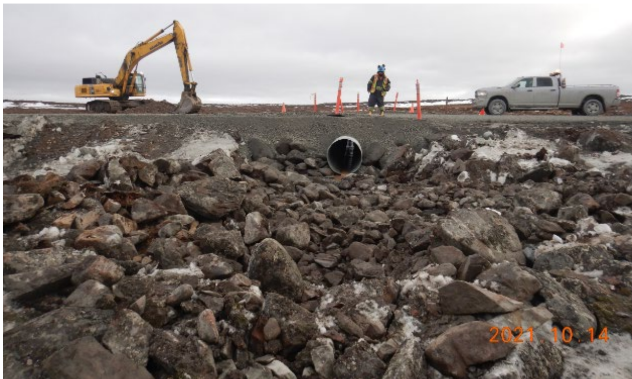
Photo 6. Installed culvert 22-2 with overlaying protective layer, looking South.
