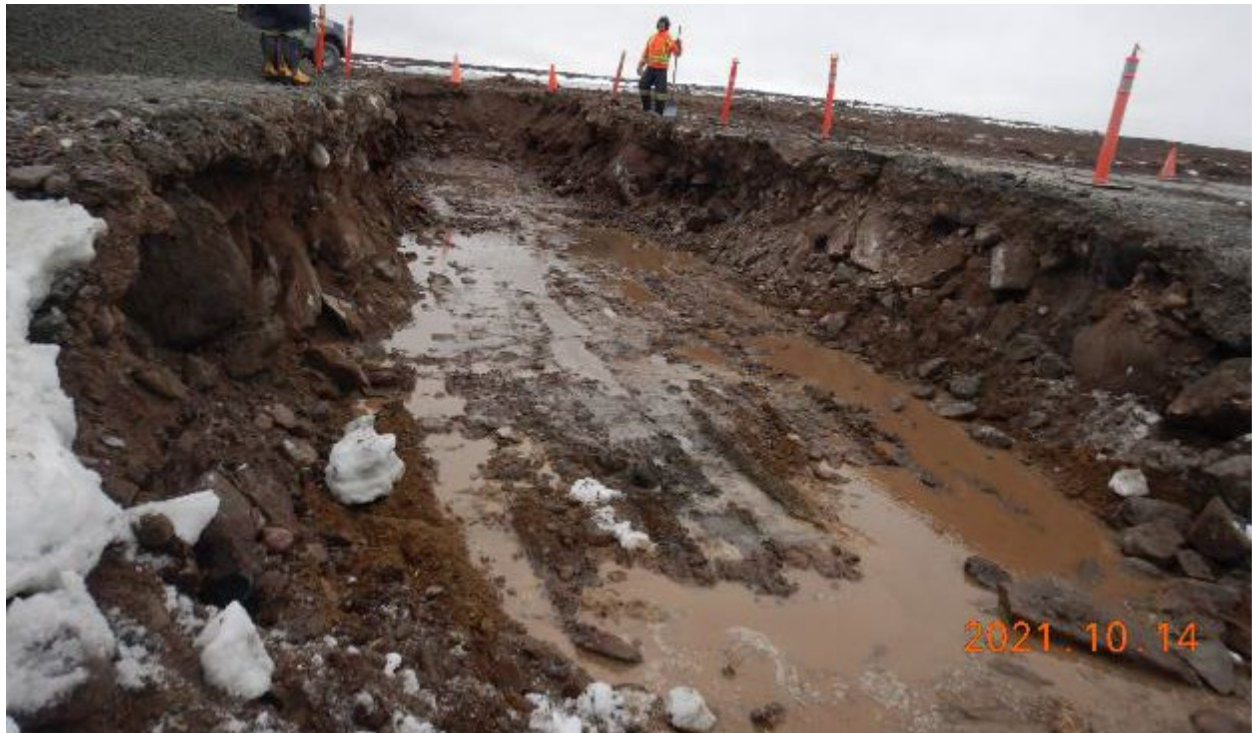
Photo 3. Excavation of the road material to install the culvert 22-2, looking South.
