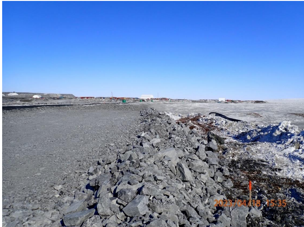
Looking east at completion of Lift #3 at West abutment and upstream slope of thermal capping
