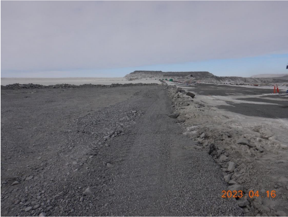
Minor resurfacing and profiling of Phase 2 remediation at East abutment
