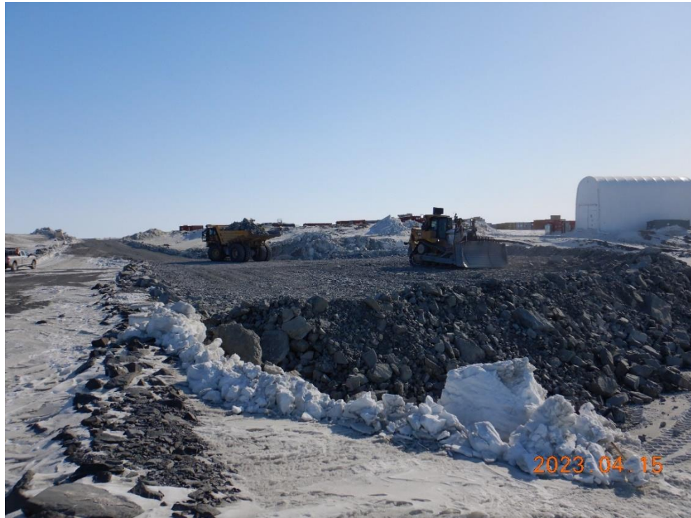
Looking east at completion of East abutment Lift #2 to El. 159 m
