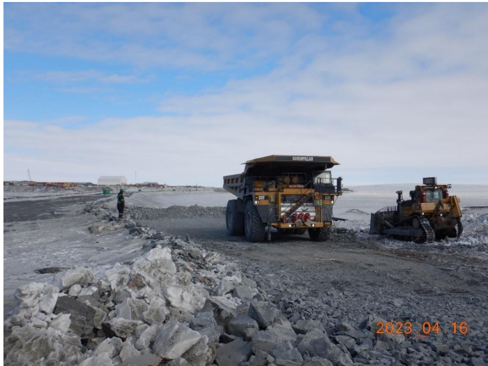
Compaction of completed Lift #2 at West abutment
