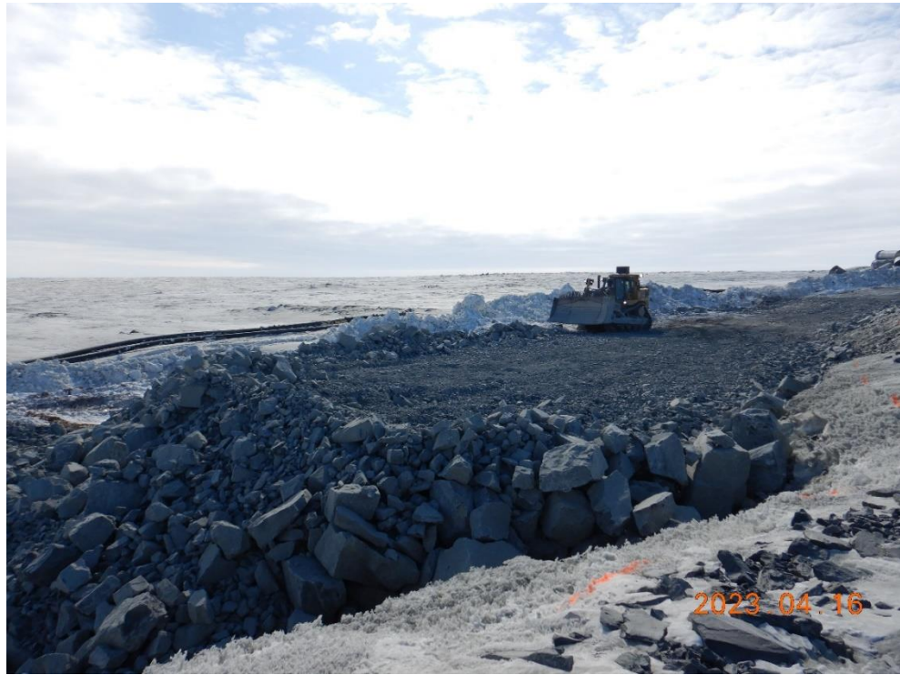
Completion of material placement for Lift #2 at West abutment
