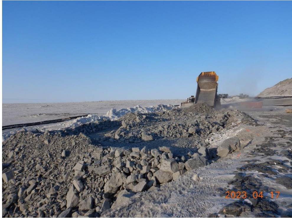
Placement of Lift #3 at West abutment
