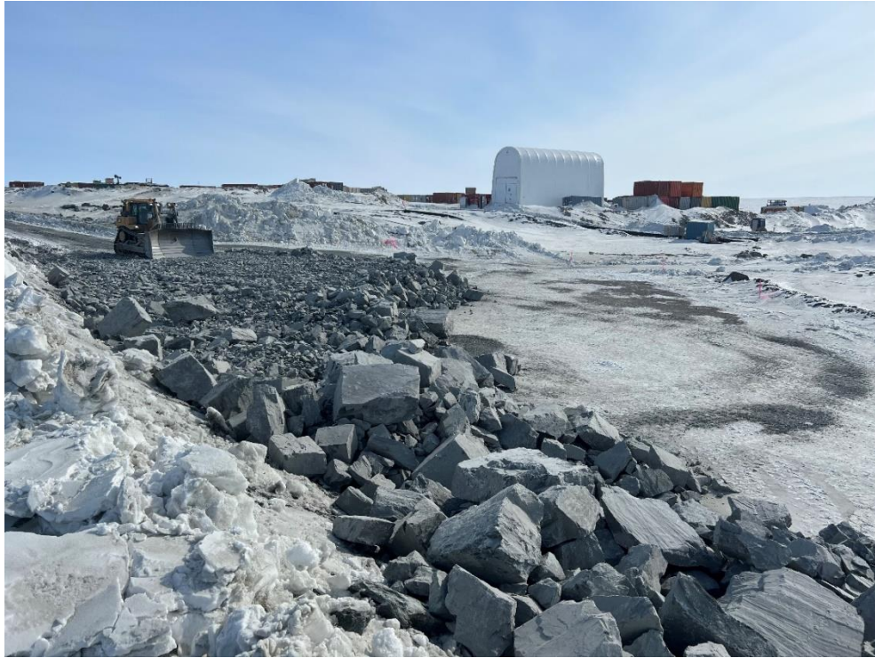
Beginning of East abutment Lift #1
