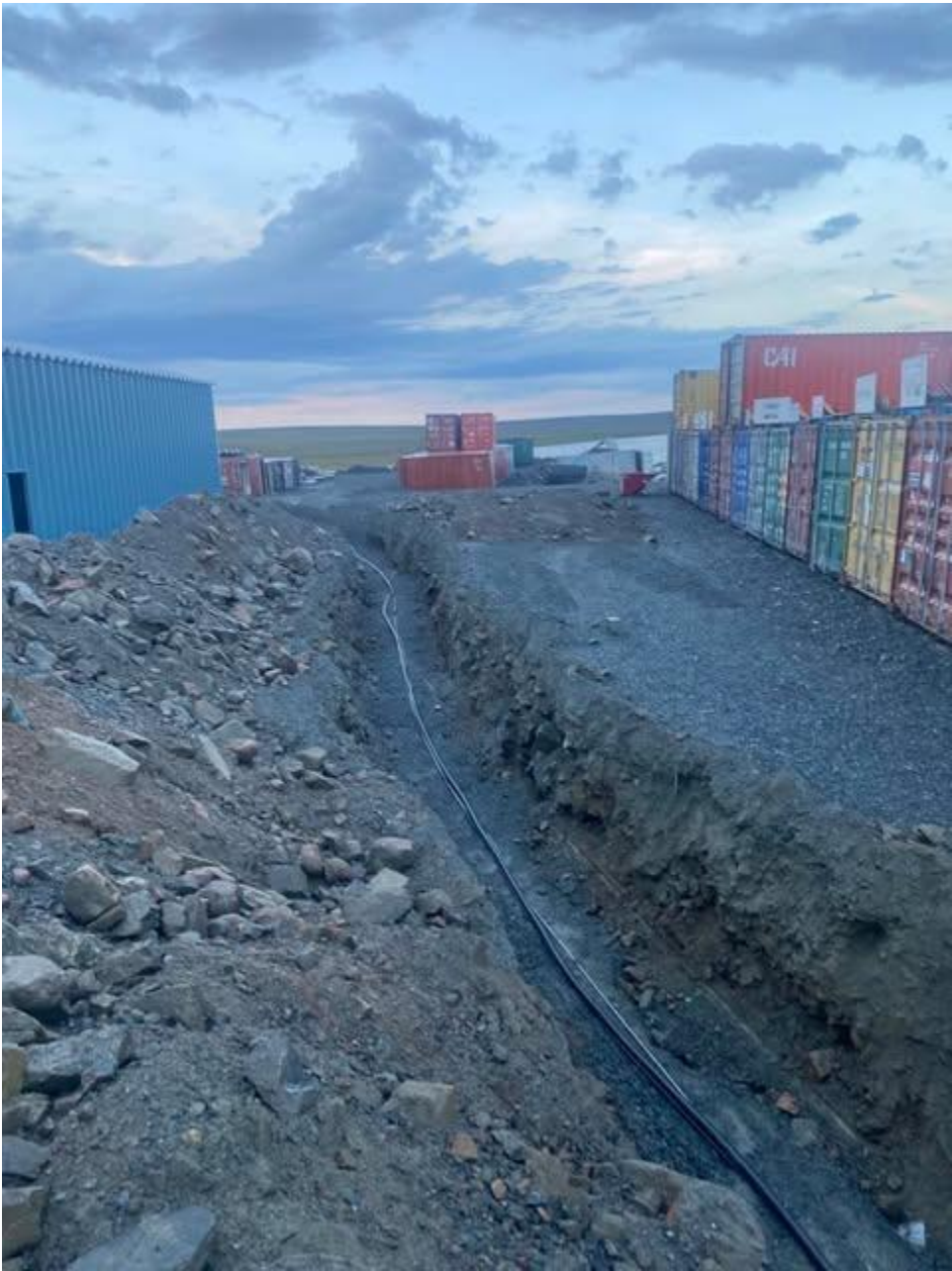
Trench for Main Electrical Cable:
