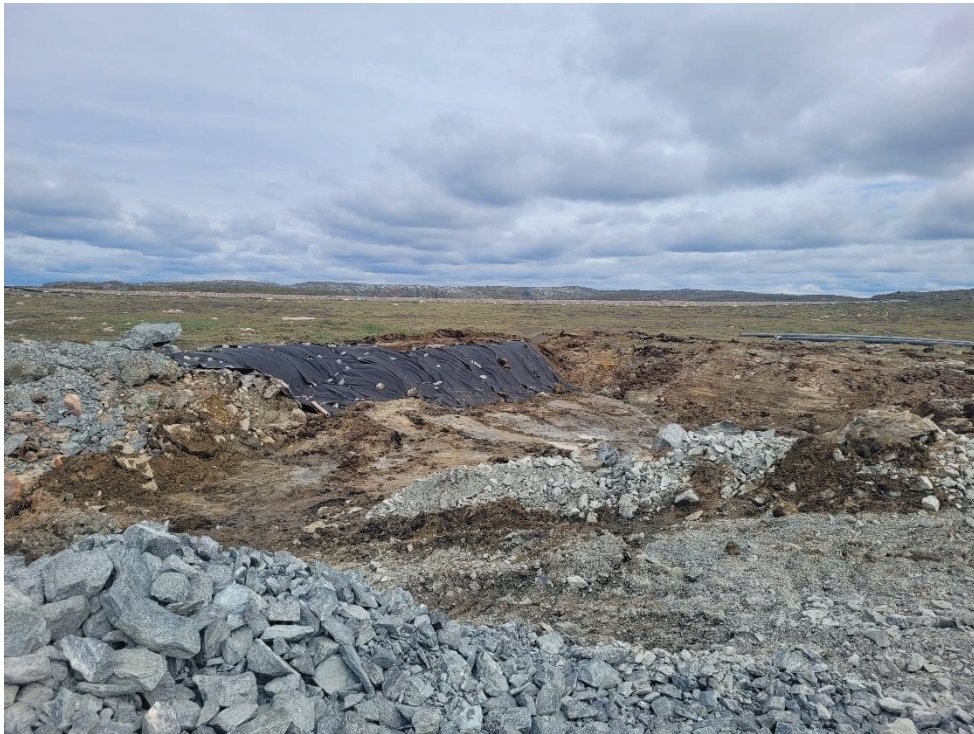
Photo 2. Excavated lakebed sediments and geotextile placed on slope, looking North.
