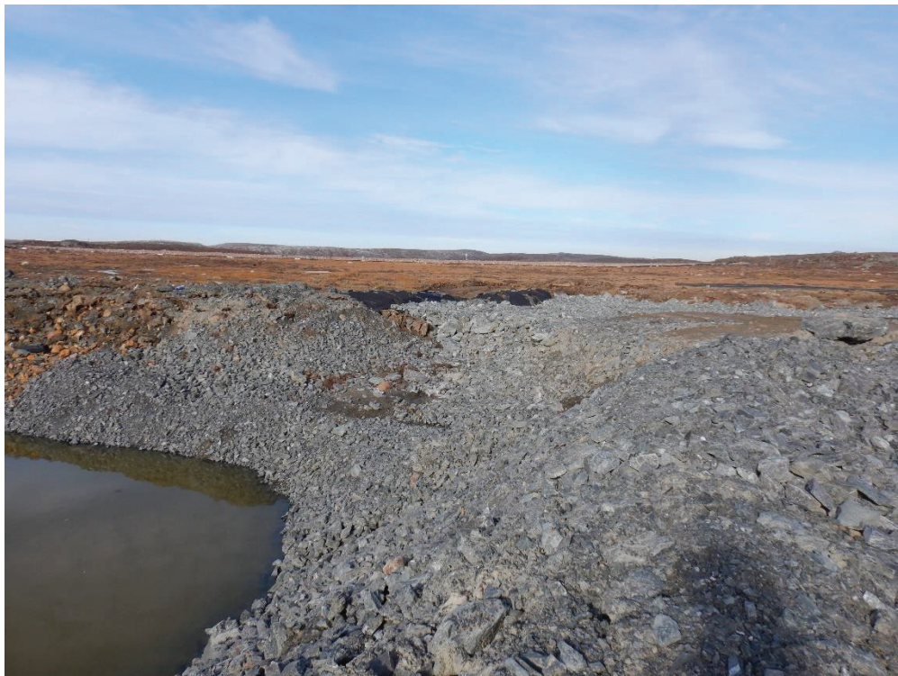
Photo 4. A47-N sump with improved northeast slope for stabilization after construction completion.
