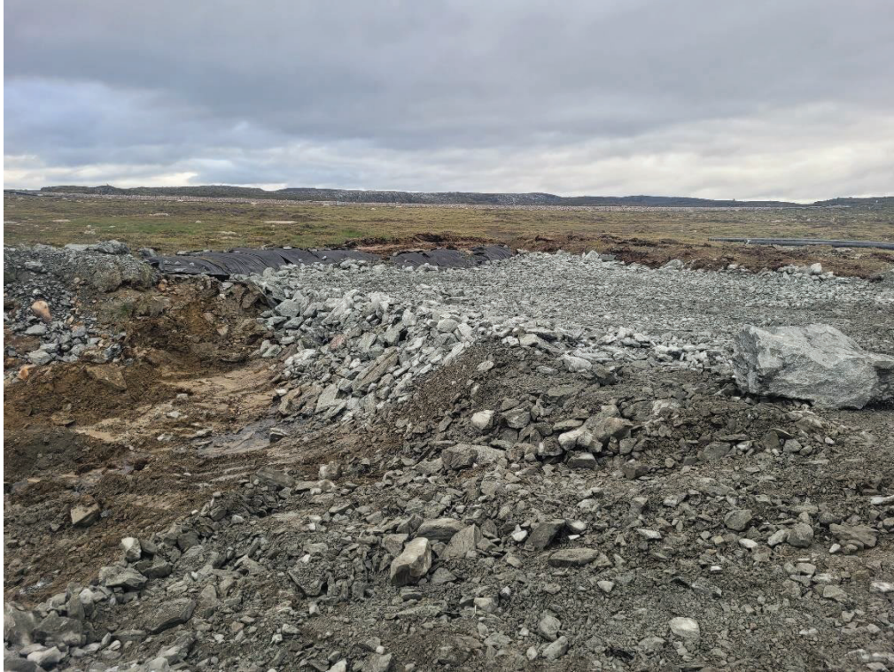
Photo 3. Placement of rockfill material around sump to access sedimented area, looking North.
