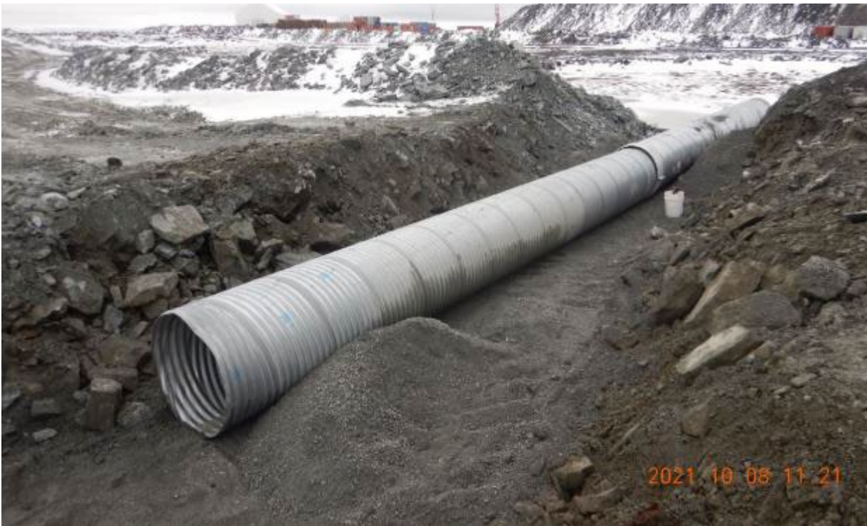
Photo 2. Installed culvert 35-1 on top of a layer of compacted fine filter, looking South-West.
