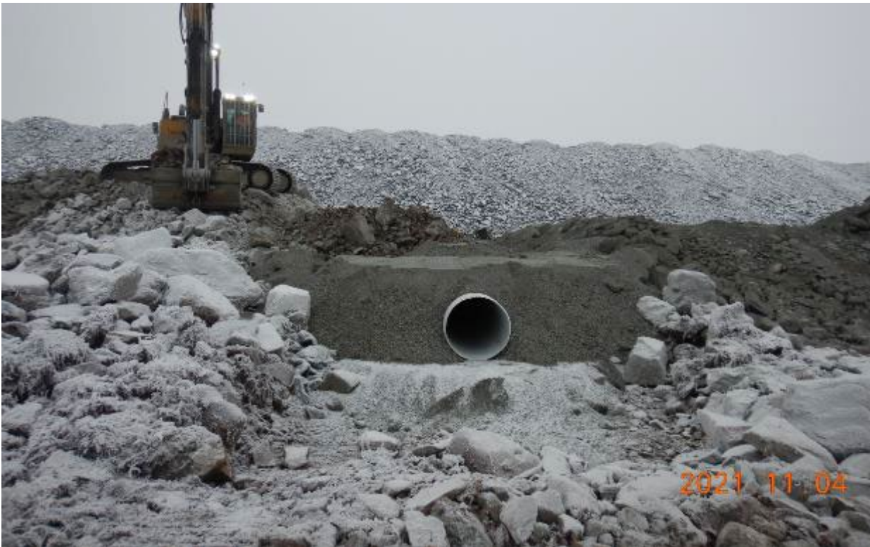
Photo 20. Installed culvert 35-3 with compacted overlying protective layer, looking North-East.
