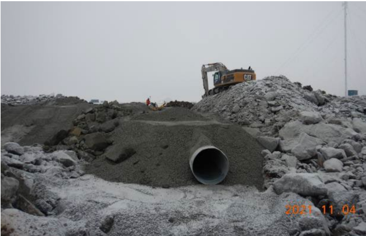
Photo 19. Installed culvert 35-3 with overlaying compacted protective layer, looking South-West.
