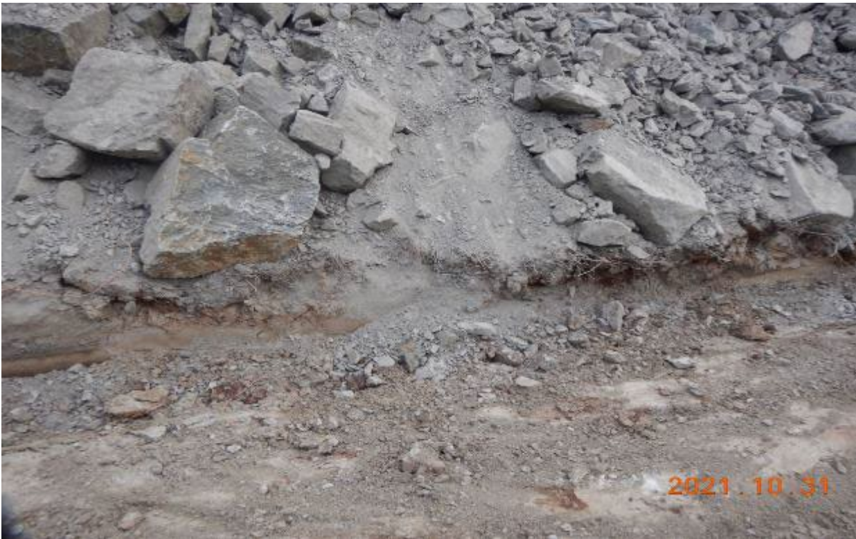
Photo 13. Exposed trench wall of culvert 35-3 showing till foundation underlying tundra.
