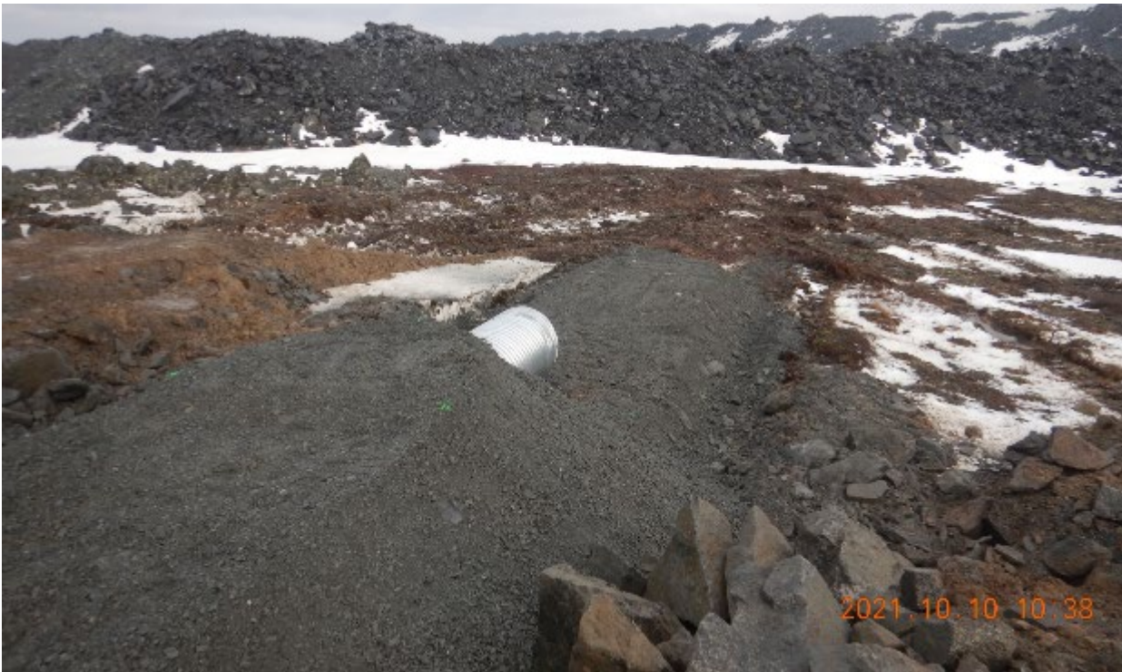
Photo 9. Installed culvert 35-2 with overlying compacted layer, looking North-East at inlet.
