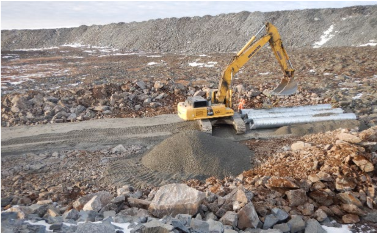
Photo 24. Culvert 35-4 (A, B, C) installation on top of compacted fine filter, looking North at inlet.
