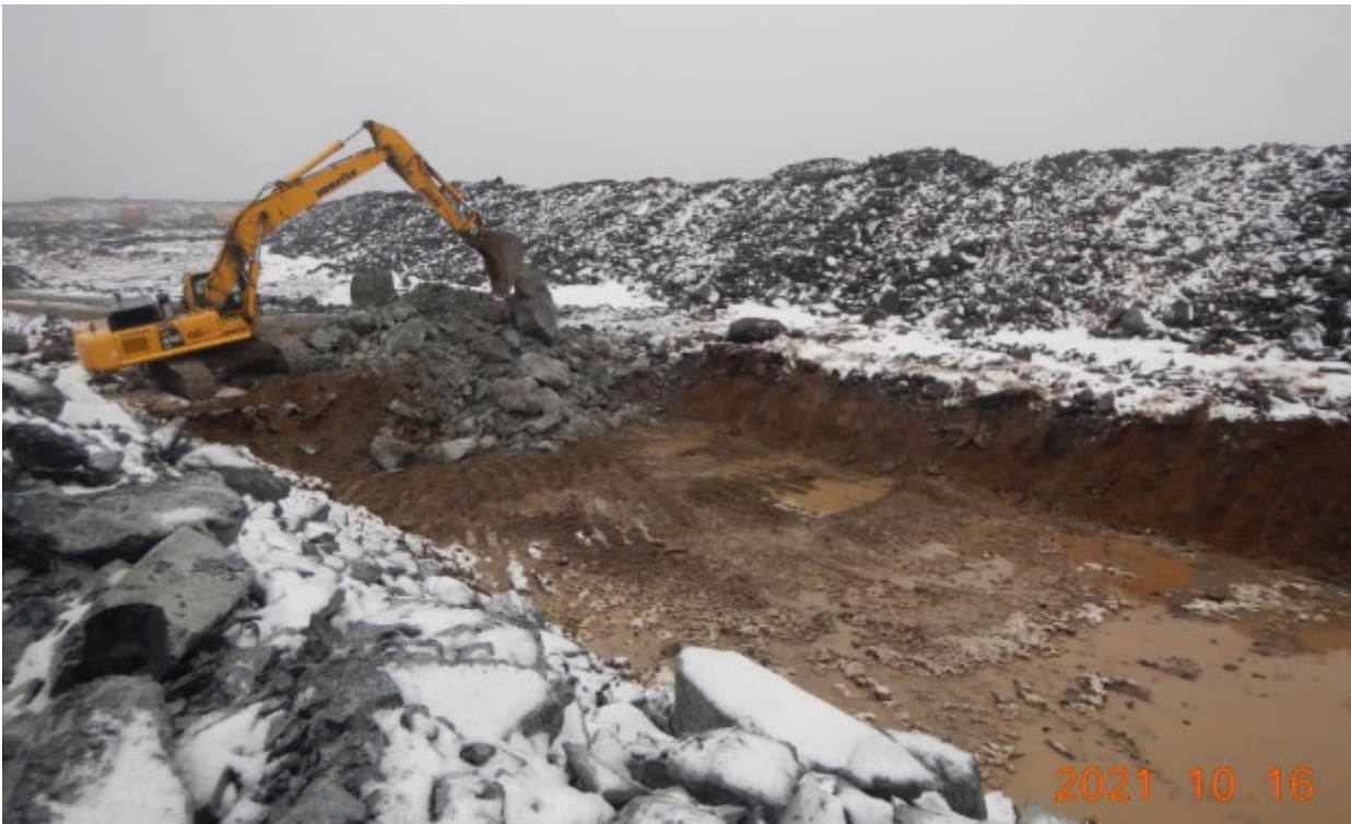
Photo 29: IWD sump being excavated with Komatsu P450, looking North.
