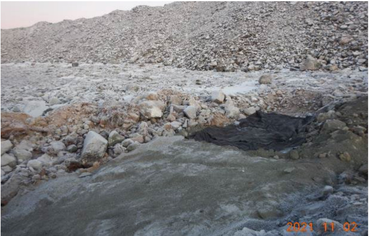
Photo 15. Installed geotextile strips at the North-East end of the trench, culvert 35-3.
