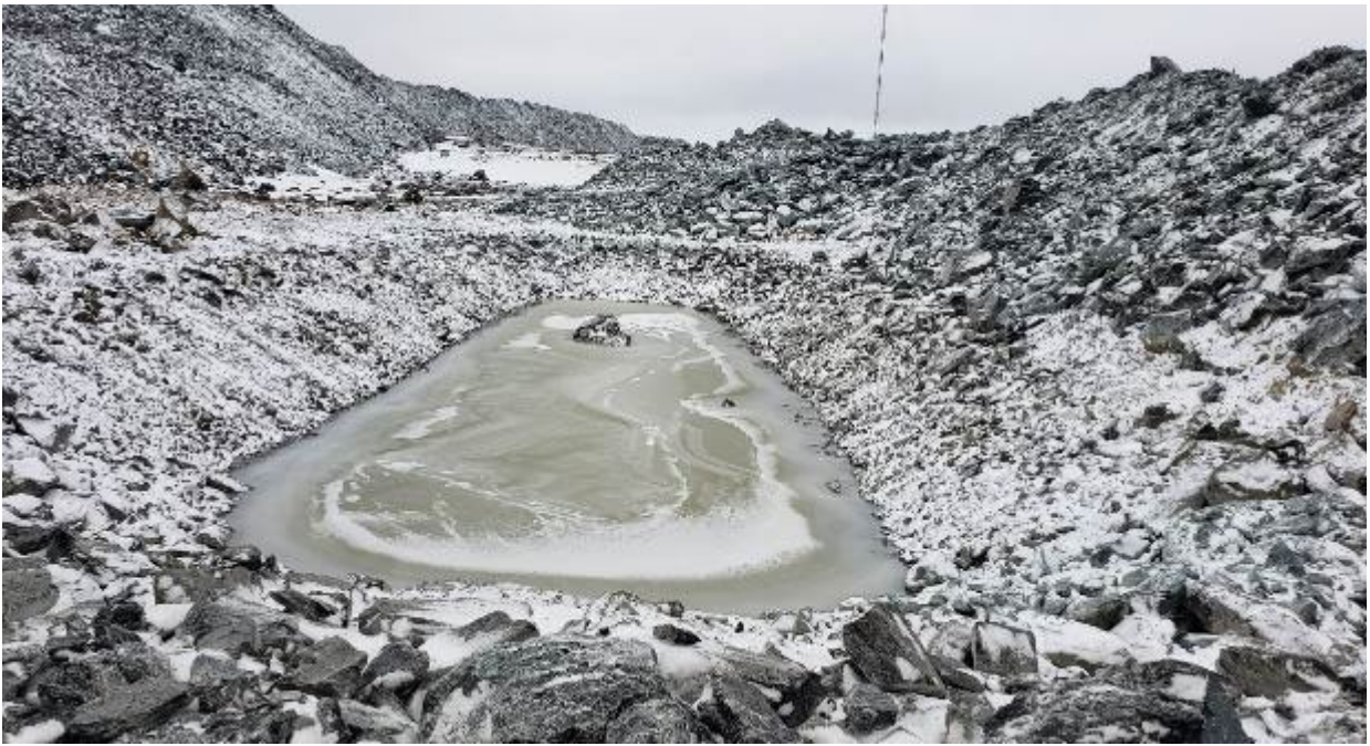
Photo 31. IWD sump once completed with rockfill and slopes in place looking East.
