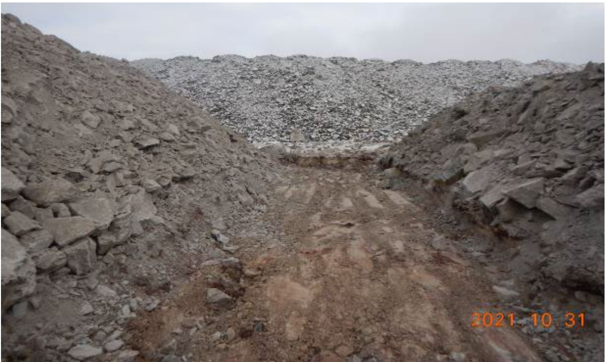
Photo 12. Excavation of road material for installation of culvert 35-3, looking South-West.
