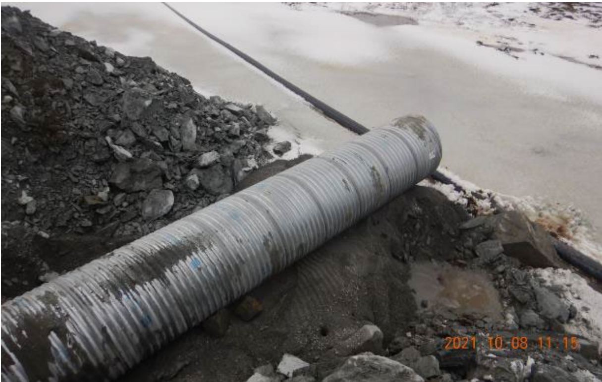
Photo 1. Installed culvert 35-1 on top of an underlying layer of compacted fine filter, looking at outlet (South-West).
