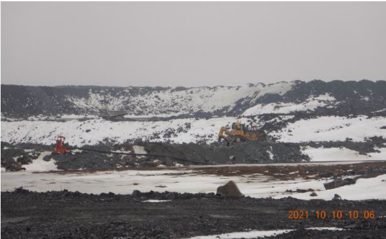
Photo 5. View of the pipe crossing culvert 35-1 backfilled with fine filter material, and in the process of being backfilled with NAG by a bulldozer, looking North-East.
