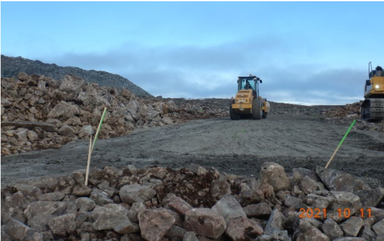
Photo 23. Fine filter subgrade material covering geotextile strips and being compacted by roller-compactor, looking East, towards culvert 35-4 (A, B, C) inlet.
