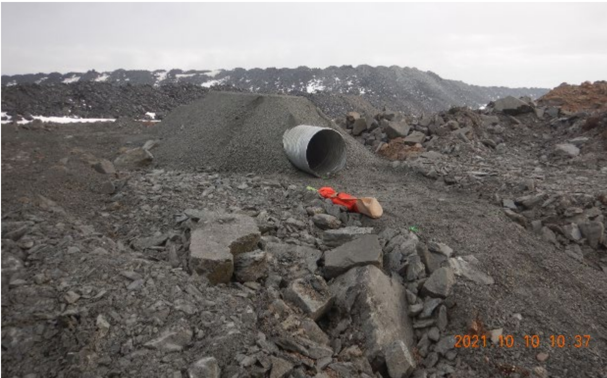
Photo 7. Installed culvert 35-2 with overlying protective layer compacted using a Wacker-Packer, looking North-East at outlet.
