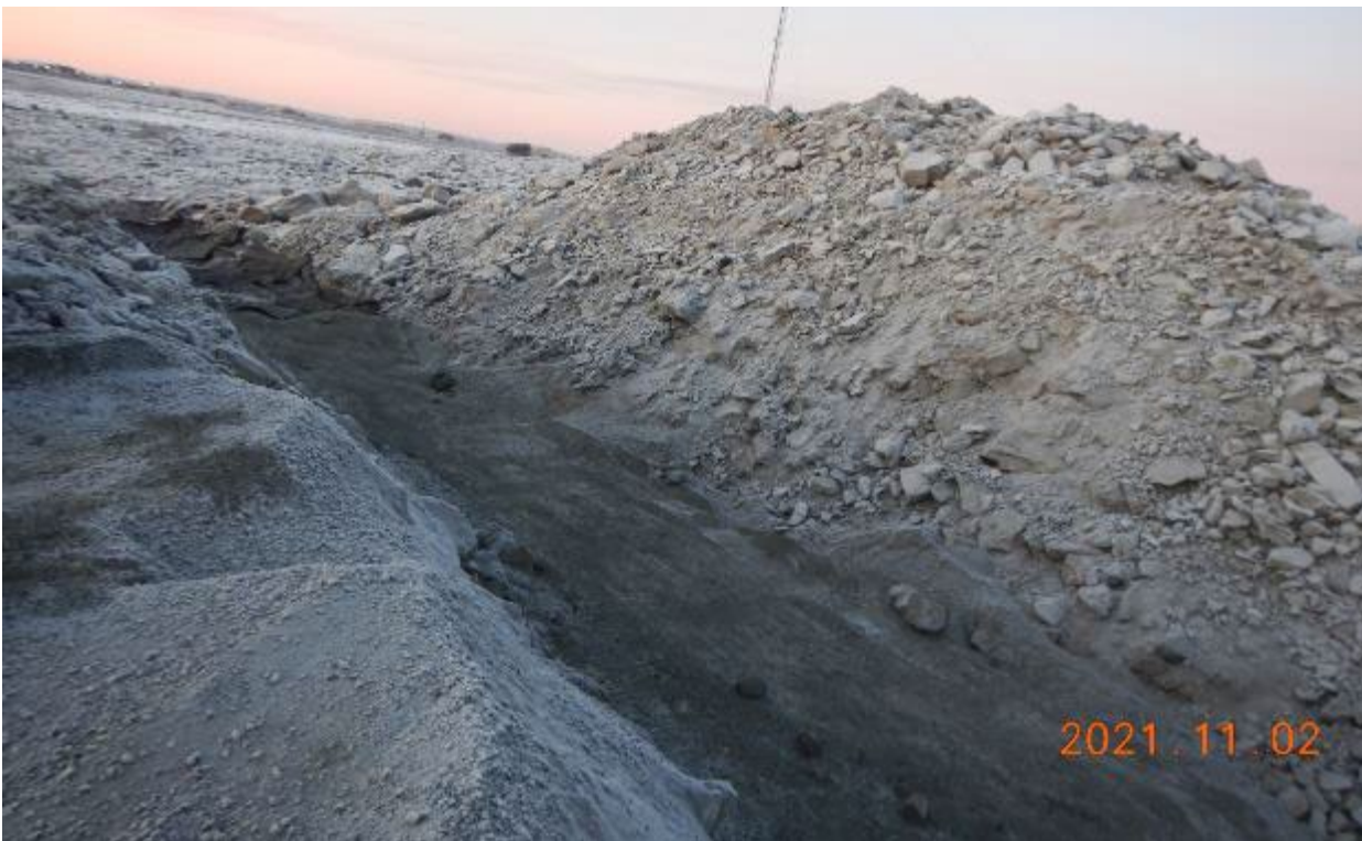
Photo 14. Fine filter layer for culvert 35-3 the width of the road and installed geotextile strips at the South-West end of the trench.
