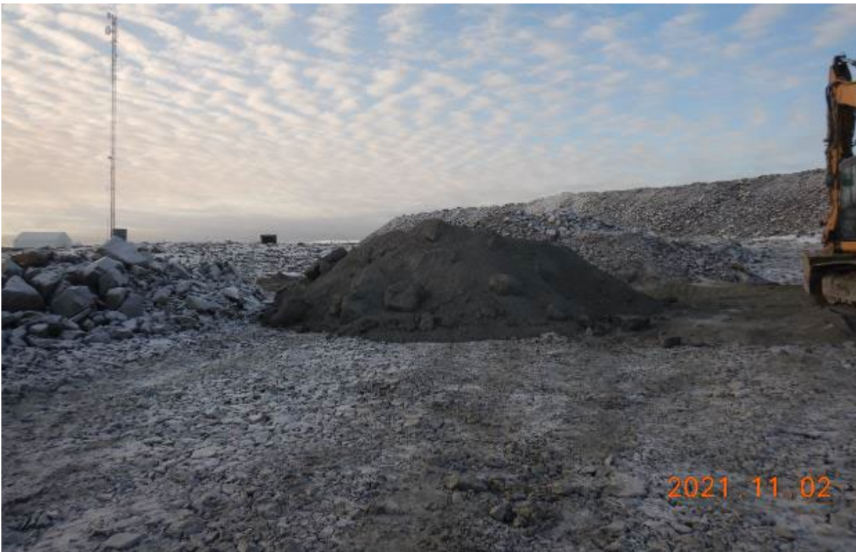
Photo 16. Fine filter subgrade material used as backfill, culvert 35-3.
