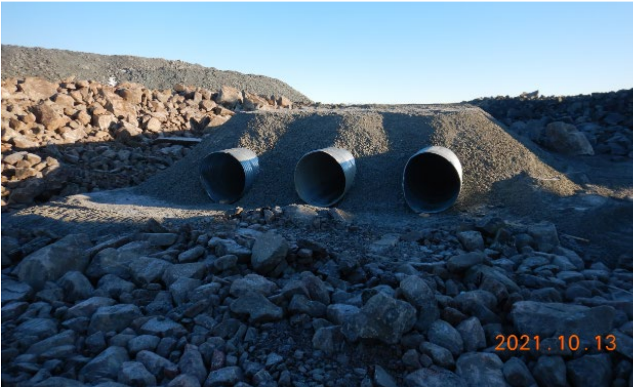
Photo 26. Installed culvert 35-4 (A, B, C), covered with a compacted fine filter layer, looking East at outlet.
