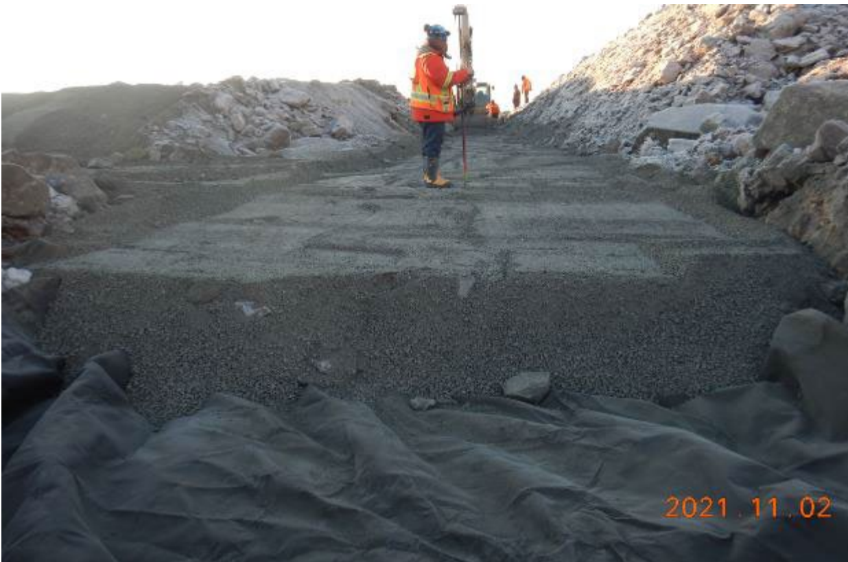
Photo 18. Fine filter subgrade material final thickness, looking South-West, culvert 35-3.
