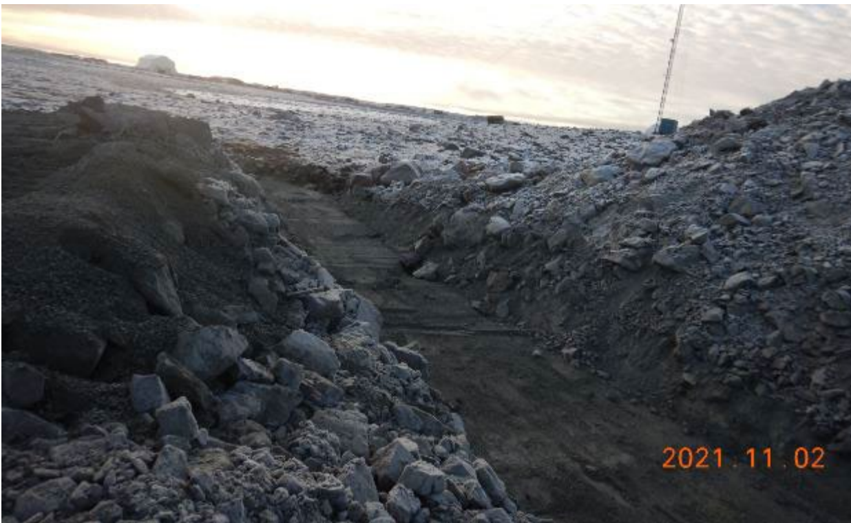
Photo 17. Fine filter subgrade material covering geotextile strips at the South end of the trench for culvert 35-3.
