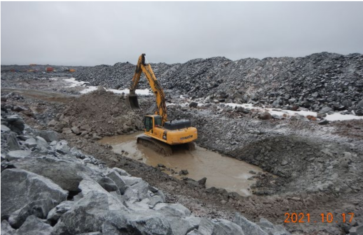
Photo 30. IWD sump being layered with rockfill, looking North.
