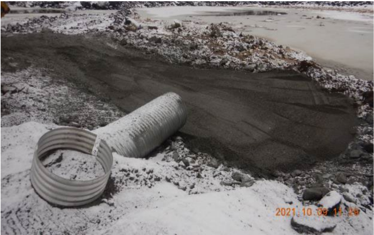
Photo 3. Compacted pad of fine filter material extended to IWB sump for culvert 35-1, looking North-East.
