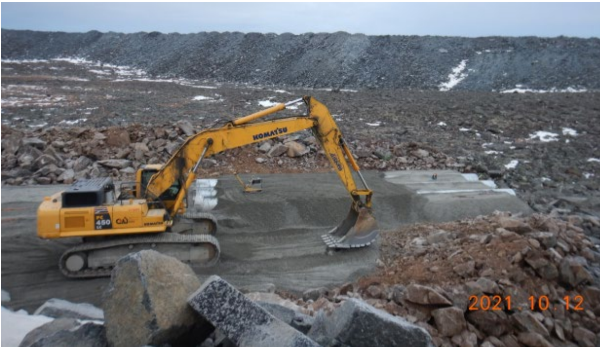
Photo 25. Installed portion of culvert 35-4 (A, B, C) being covered with compacted fine filter protection layer, looking North at inlet.
