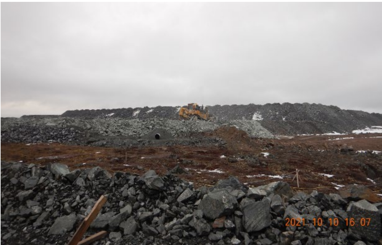
Photo 10. View of the pipe crossing 35-2 backfilled with fine filter material, and in the process of being backfilled with NAG by bulldozer, looking North-East.
