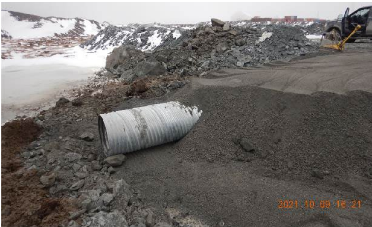
Photo 4. Installed culvert 35-1 with compacted overlying protective layer, looking South at inlet.
