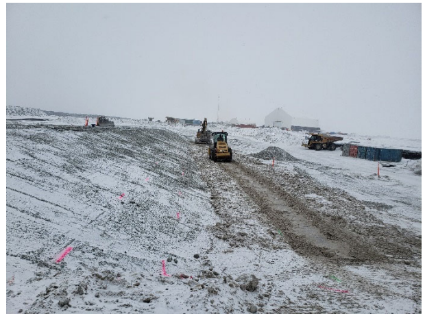
2227: (2021-04-21), looking W from Sta. 0+100. KCG utilizing smooth drum roller to compact placed Zone 4 material.
