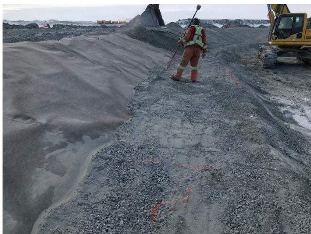
2216: (2021-04-18), looking W from Sta. 0+310. Zone 2B on top of LLDPE liner hinge and Zone 2A placement on slope.
