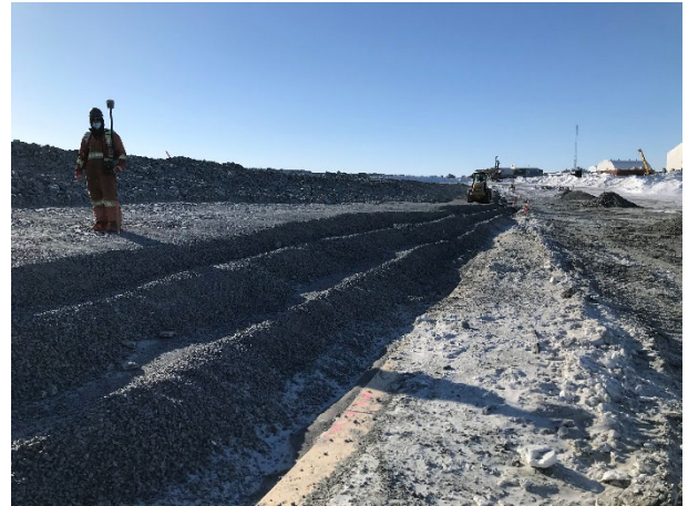
2186: (2021-04-07), looking W from Sta. 0+200. Placement of Zone 3 material on upstream side of liner.
