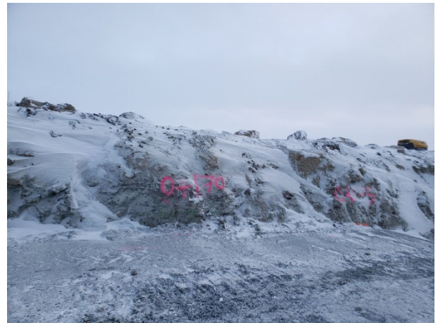
2048: (2021-03-08), looking NE from Sta. 0+170. Additional snow to be removed along upstream excavation wall in advance of Zone 2A (fine filter) material placement.
