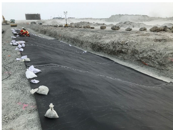
2202: (2021-04-13), looking E from Sta. 0+403. Installed LLDPE liner, between Sta. 0+403 to Sta. 0+437.
