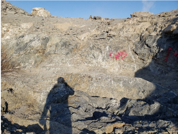
2157: (2021-03-31), looking W from Sta. 0+050. Approved section of key trench foundation.
