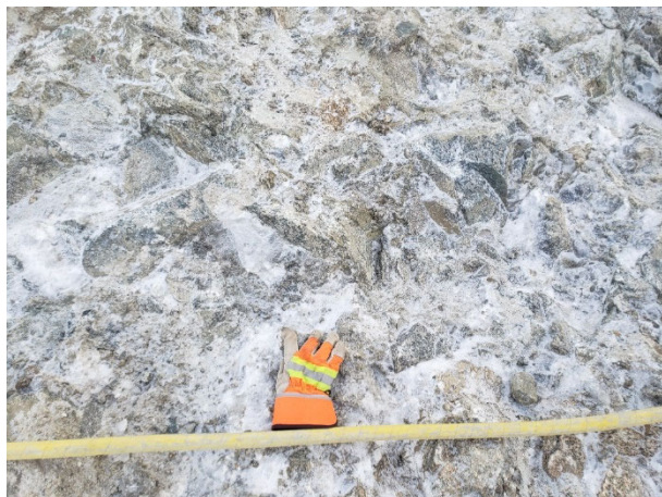
2051: (2021-03-08), looking E from Sta. 0+206. Additional ice and loose bedrock to be removed during key trench foundation preparation.
