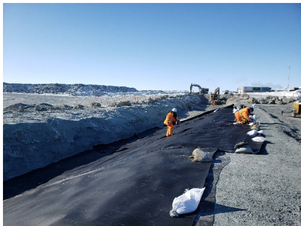
2143: (2021-03-28), looking W from Sta. 0+135. FC liner installing LLDPE liner.
