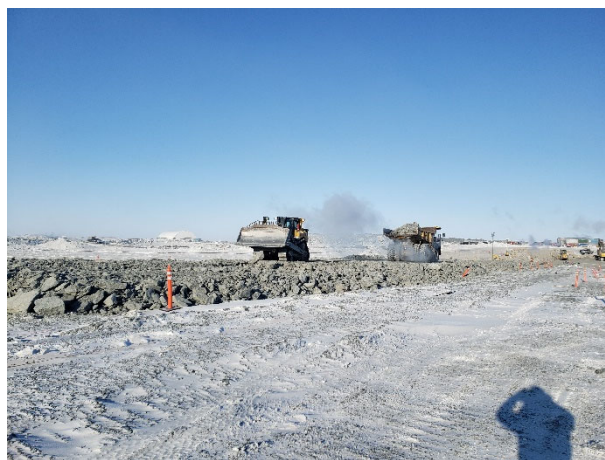
2140: (2021-03-28), looking SW from Sta. 0+260. KCG placing Zone 1 for construction of downstream shell.
