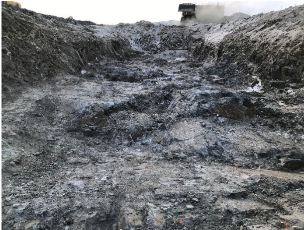
2191: (2021-04-10), looking E from Sta. 0+482. Approved key trench bedrock foundation surface, Sta. 0+482 to Sta. 0+515.
