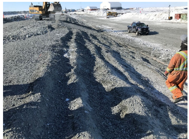
2190: (2021-04-09), looking W from Sta. 0+200. Sloping of Zone 2A upstream under liner.
