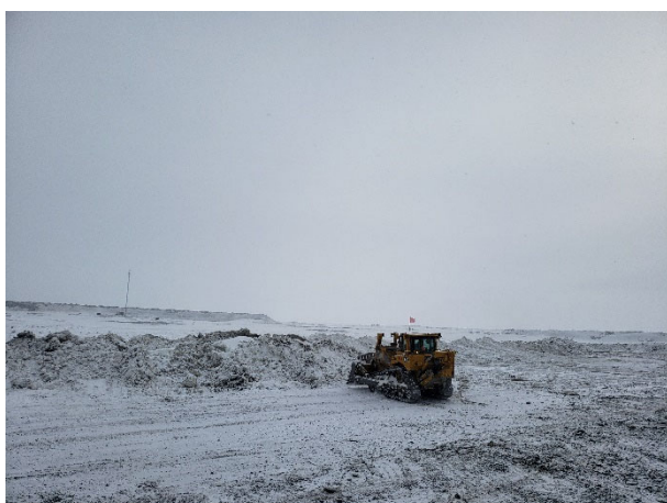
2270: (2021-05-03), looking NE from Sta. 0+490. Komatsu dozer flattening snow stockpiles upstream of the IVR Dyke.
