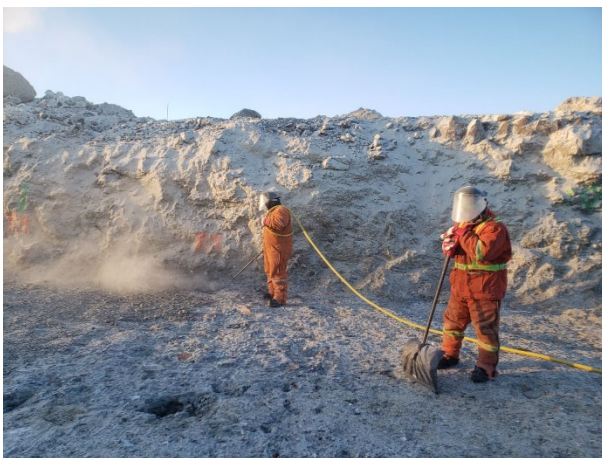
2037: (2021-03-05), looking S from Sta. 0+190. KCG labourers preparing foundation of key trench.
