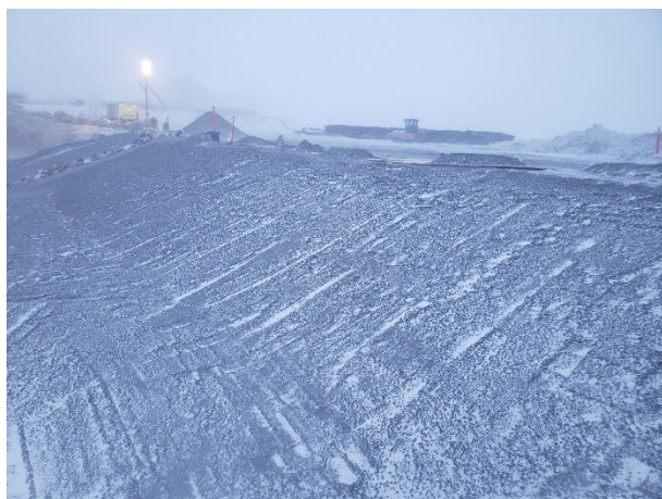
2131: (2021-03-26), looking W from Sta. 0+180. Approved placement of Zone 2A material over LLDPE liner.
