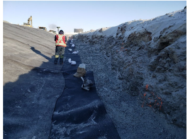
2120: (2021-03-24), looking E from Sta. 0+315. Snow removed along lower portion of downstream trench excavation sidewall and base of Zone 2B in preparation for Zone 2B placement over installed LLDPE.
