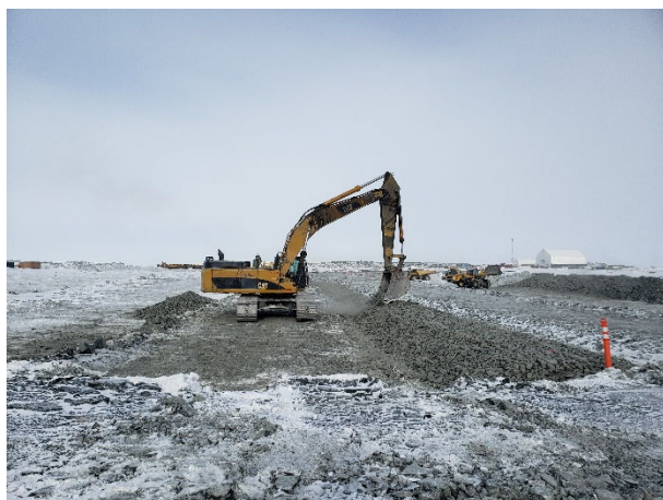
2256: (2021-04-29), looking W from Sta. 0+515. CAT excavator placing Zone 3 over previously placed Zone 2A.
