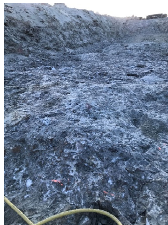
2058: (2021-03-11), looking E from Sta. 0+227. Final foundation approved for placement of Zone 2B material.
