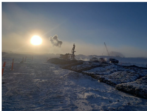
2024: (2021-03-02), looking E from Sta. 0+160. KCG continuing to drill holes for fourth key trench blast.
