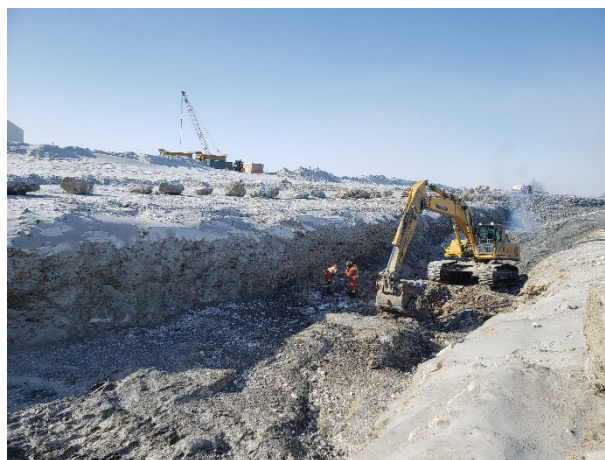
2152: (2021-03-30), looking SW from Sta. 0+435. KCG labourers removing ice and snow within footprint of key trench.
