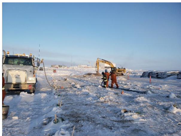
2022: (2021-03-01), looking W from Sta. 0+170. Dyno loading drill pattern for third key trench blast.
