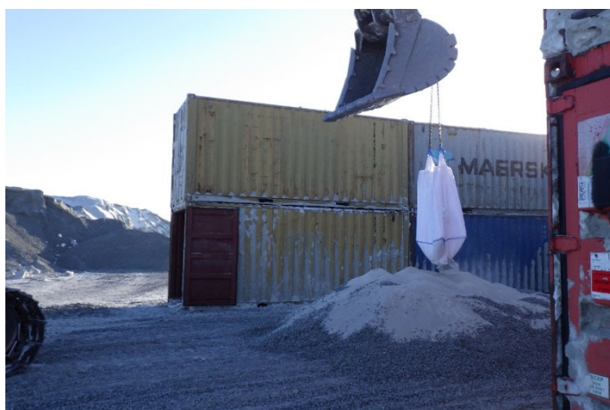
2031: (2021-03-04), looking N at mixing station. KCG producing Zone 2 B FFAB material at the mixing pad.
