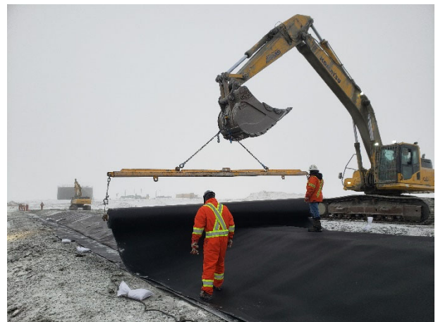
2223: (2021-04-21), looking SE from Sta. 0+460. FC Liner installing LLDPE for upper slope.
