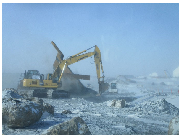
2104: (2021-03-21), looking W from Sta. 0+300. Placement of Zone 2B in key trench.
