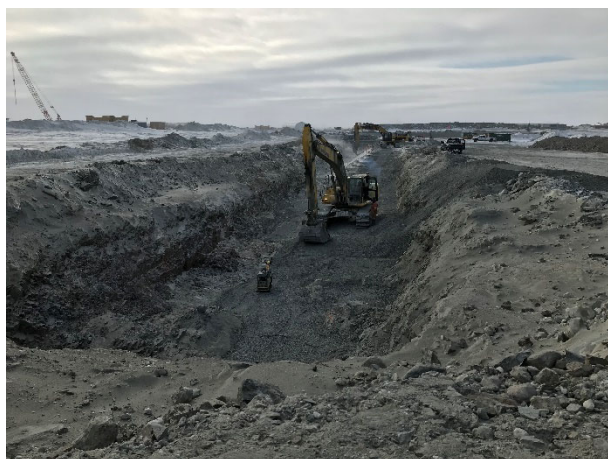
2197: (2021-04-11), looking W from Sta. 0+526. Placement of Zone 2A (FF) in key trench, Sta. 0+482 to Sta. 0+526.
