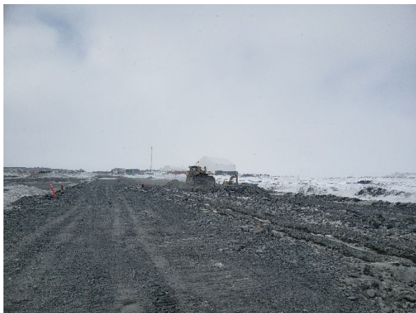
2258: (2021-04-29), looking W from Sta. 0+200. Dozer spreading lift of Zone 1 (rockfill).
