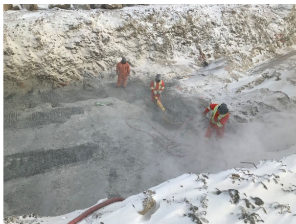
2084: (2021-03-16), looking E from Sta. 0+0+315. Cleaning, placement & compaction of Zone 2B (FFAB) material over bedrock section of key trench
