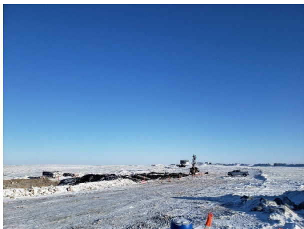
2023: (2021-03-01), looking E from Sta. 0+125. Blast mats installed over drill pattern in preparation for third key trench blast.
