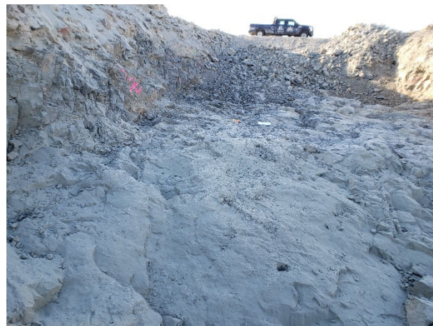
2148: (2021-03-29), looking E from Sta. 0+080. Prepared section of key trench foundation.
