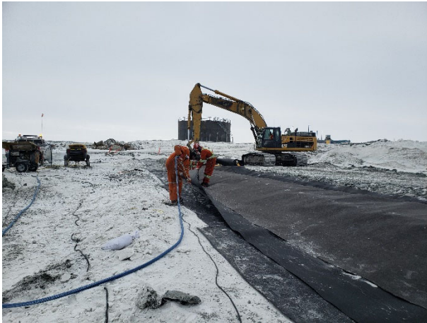
2230: (2021-04-22), looking E from Sta. 0+500. KCG removing snow and ice over LLDPE liner in advance of extrusion weld.
