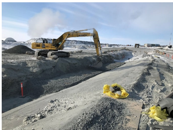
2089: (2021-03-17), looking W from Sta. 0+200. Placement of Zone 2B (FFAB) over LLDPE liner.
