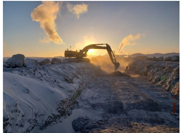
2036: (2021-03-05), looking E from Sta. 0+130. CAT excavator placing Zone 2B FFAB material within footprint of key trench.
