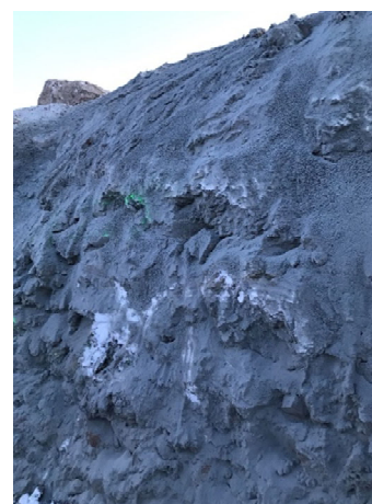
2056: (2021-03-11), looking E from Sta. 0+200. Wind deposited snow on trench walls to be cleaned prior to fill.
