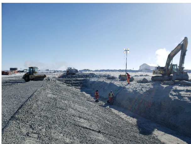
2141: (2021-03-28), looking E from Sta. 0+135. KCG labourers removing snow along toe of Zone 2A in advance of LLDPE installation.
