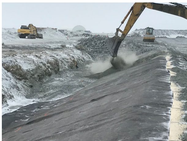
2206: (2021-04-14), looking W from Sta. 0+437. Placement of Zone 2B and Zone 2A on top of LLDPE liner.
