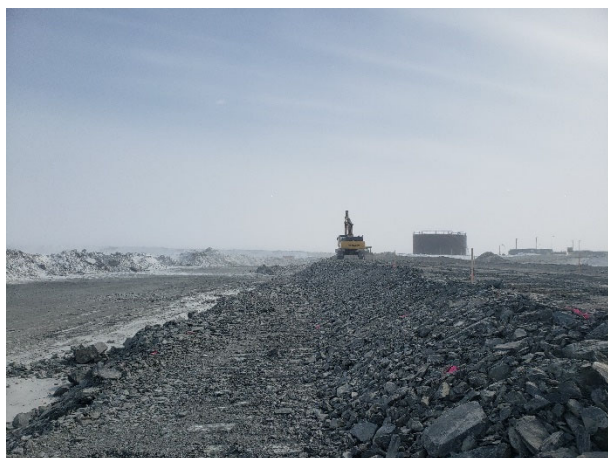
2262: (2021-05-01), looking E from Sta. 0+450. Komatsu excavator shaping upstream Zone 1 slope to design lines.
