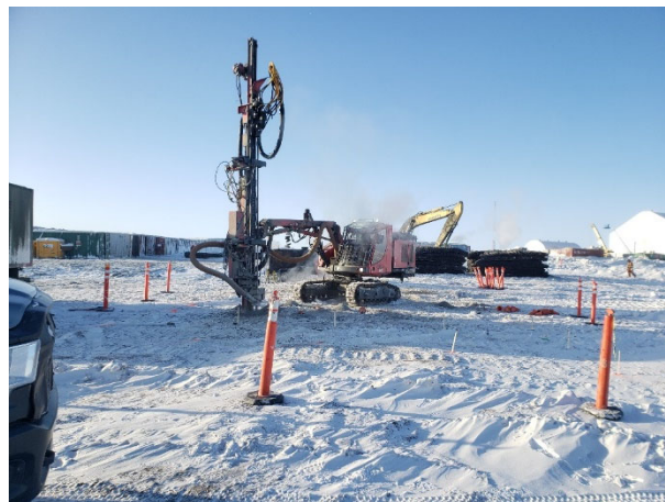
2008: (2021-02-23), looking W from Sta. 0+120. KCG drilling holes through overburden in advance of blasting for key trench at the IVR Dyke.
