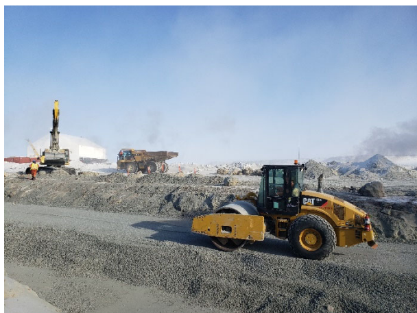
2149: (2021-03-29), looking N from Sta. 0+100. KCG utilizing smooth drum roller to compact placed Zone 2A material.
