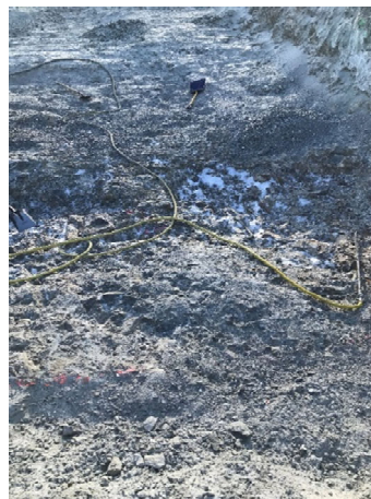
2052: (2021-03-10), looking E from Sta. 0+207. Ice after excavating down 0.3 m.
