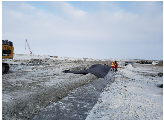
2229: (2021-04-22), looking W from Sta. 0+490. FC liner installing geotextile over Zone 2A material.
