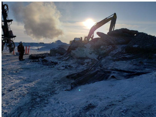
2012: (2021-02-24), looking S from Sta. 0+135. KCG continuing to drill holes for second blast.
