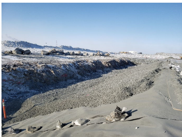
2135: (2021-03-27), looking W from Sta. 0+400. Approved placement of Zone 2A material over LLDPE liner.
