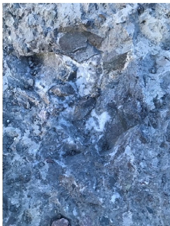
2057: (2021-03-11), looking E from Sta. 0+230. Small pocket of ice (<0.5 square meters) observed in trench floor, typical of this section.
