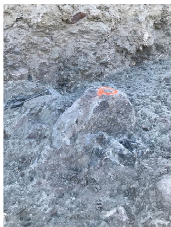
2065: (2021-03-12), looking SW from Sta. 0+254. Boulder sticking out of trench floor.
