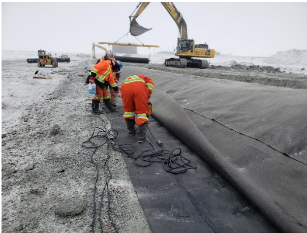
2226: (2021-04-21), looking E from Sta. 0+400. FC liner conducting extrusion weld between installed LLDPE liner panels.
