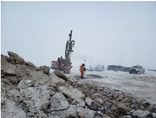
2017: (2021-02-27), looking NE from Sta. 0+150. KCG drilling remaining for third key trench blast.
