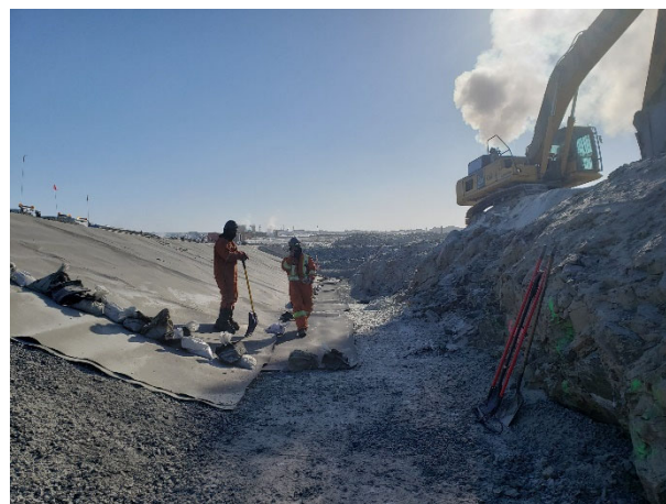
2164: (2021-04-01), looking E from Sta. 0+080. KCG removing snow along downstream key trench excavation wall.
