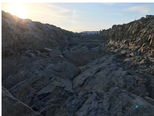
2091: (2021-03-17), looking W from Sta. 0+377. Bedrock in key trench foundation approved for placement of Zone 2B material.
