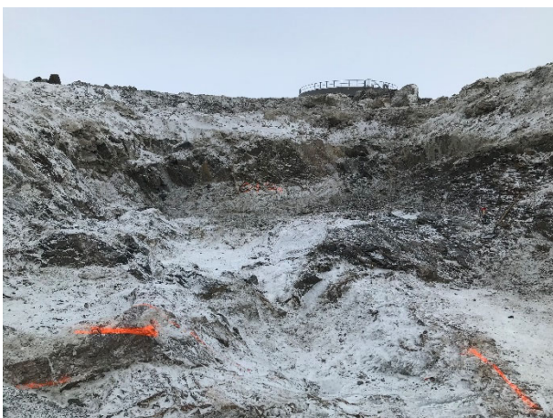
2195: (2021-04-10), looking E from Sta. 0+515. Termination of dam alignment (Eastern abutment) in key trench.
