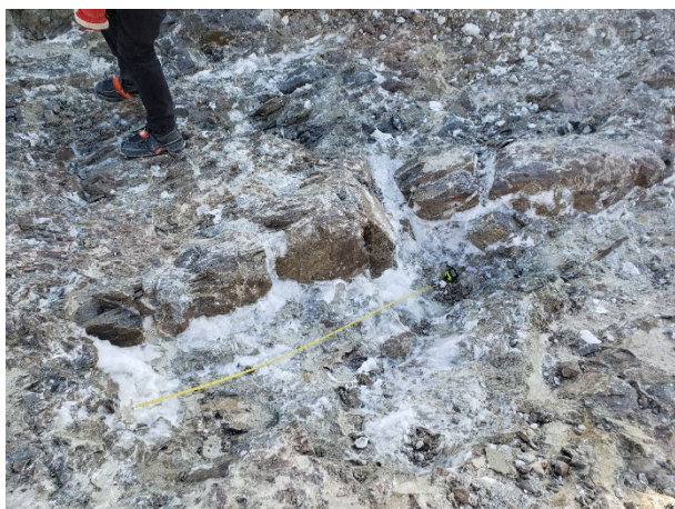
2153: (2021-03-30), looking S from Sta. 0+438. Ice pocket observed in bedrock along base of key trench.
