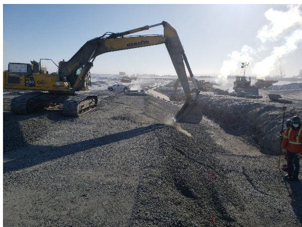
2163: (2021-04-01), looking E from Sta. 0+050. Excavator sloping Zone 2B under liner slope to design lines.
