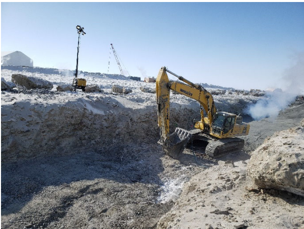
2159: (2021-03-31), looking SW from Sta. 0+450. Excavator utilizing blow pipe to clean key trench foundation.
