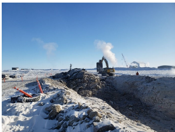
2025: (2021-03-02), looking E from Sta. 0+0+145. CAT excavator removing blast mats at the IVR Dyke.
