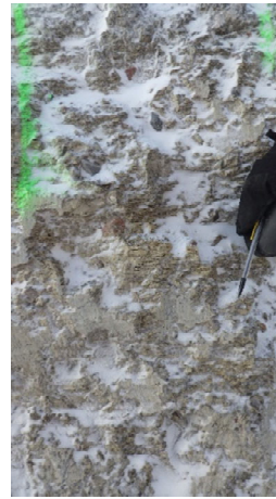
2034: (2021-03-04), looking S from Sta. 0+145. Downstream side wall of key trench excavation: small ice lenses (1-2 mm) observed.
