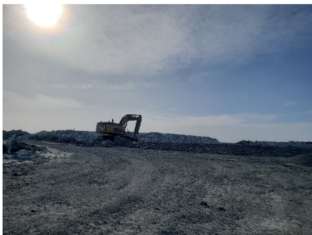
2246: (2021-04-25), looking N from Sta. 0+080. CAT excavator placing Zone 1 rockfill to construct east sidewall of spillway.
