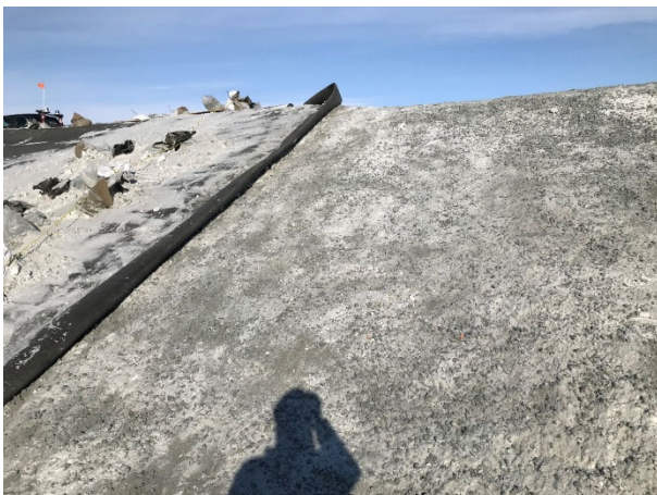
2079: (2021-03-16), looking N from Sta. 0+210. Bedding surface for geotextile/LLDPE liner after cleaning snow
