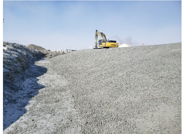
2158: (2021-03-31), looking W from Sta. 0+100. Approved section of Zone 2A/2B under liner.
