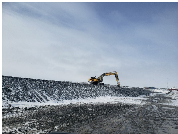
2268: (2021-05-02), looking W from Sta. 0+200. Komatsu excavator finalizing upstream slope at approx. Sta. 0+200, view looking W.
