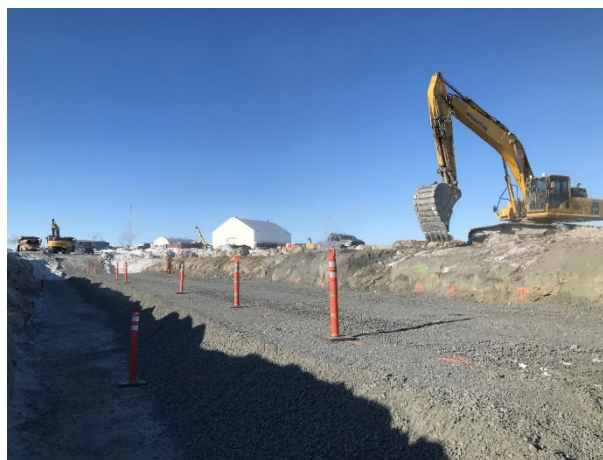
2060: (2021-03-11), looking W from Sta. 0+200. Excavator cleaning loose material, snow and dust from back-break area of trench wall.
