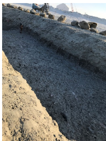
2067: (2021-03-12), looking SE from Sta. 0+250. Approved key trench subgrade foundation from Sta. 0+248 to Sta. 0+280.
