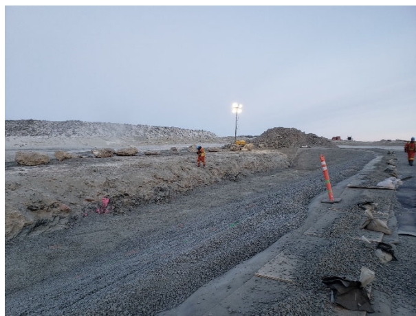
2170: (2021-04-02), looking SW from Sta. 0+065. Approved placement of Zone 2A/2B material.
