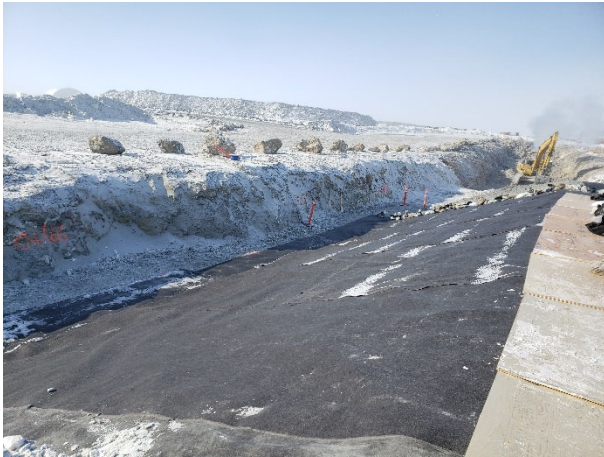
2119: (2021-03-24), looking W from Sta. 0+165. Geotextile installed over LLDPE liner between approx. Sta.0+165 and Sta. 0+135.
