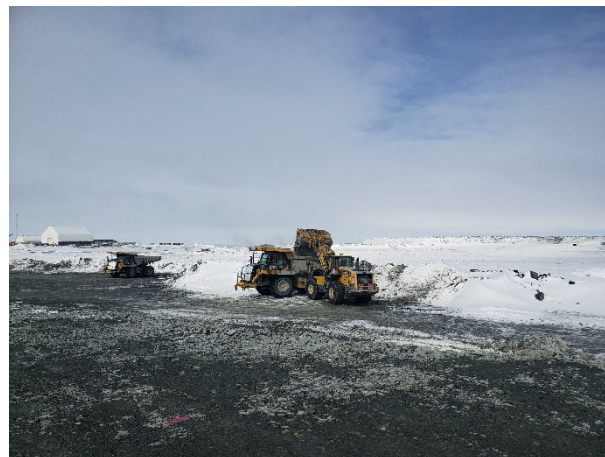
2267: (2021-05-02), looking N from Sta. 0+500. Komatsu loader loading rock truck with overburden/rock upstream of dyke.
