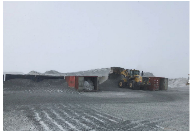
2096: (2021-03-18), looking E at Mixing Station. Additional bentonite mixing station set up to mix 4% and 6% bentonite FFAB separately.
