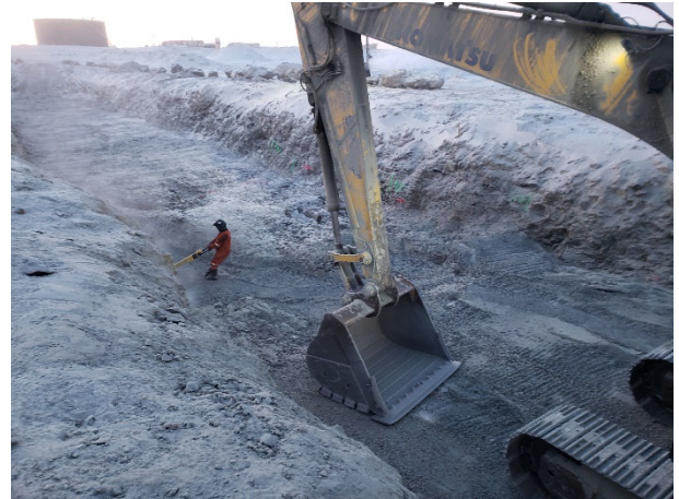
2156: (2021-03-31), looking SE from Sta. 0+430. KCG utilizing plate tamper to compact low spots in key trench.
