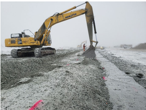
2222: (2021-04-21), looking W from Sta. 0+450. Komatsu excavator trimming Zone 2A slope to design lines.
