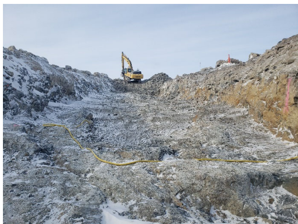
2133: (2021-03-26), looking W from Sta. 0+060. Excavator continuing to prepare key trench foundation.
