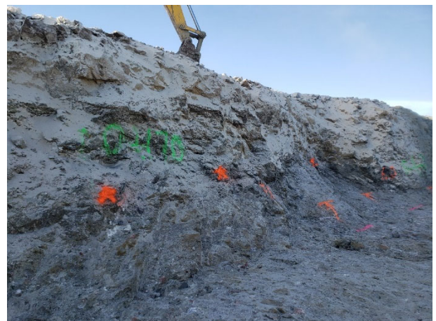
2038: (2021-03-05), looking SW from Sta. 0+170. Orange stars highlight a 100-150 mm thick lens of fine-grained ice rich material along downstream sidewall of excavation.
