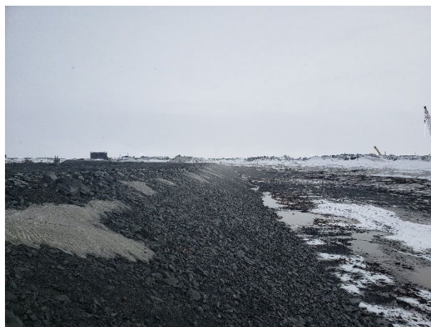
2273: (2021-05-03), looking E from Sta. 0+200. Downstream Zone 1 sloped to design lines.
