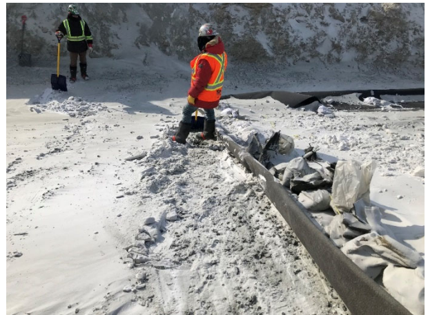
2078: (2021-03-16), looking E from Sta. 0+210. Snow on geotextile/LLDPE liner bedding surface
