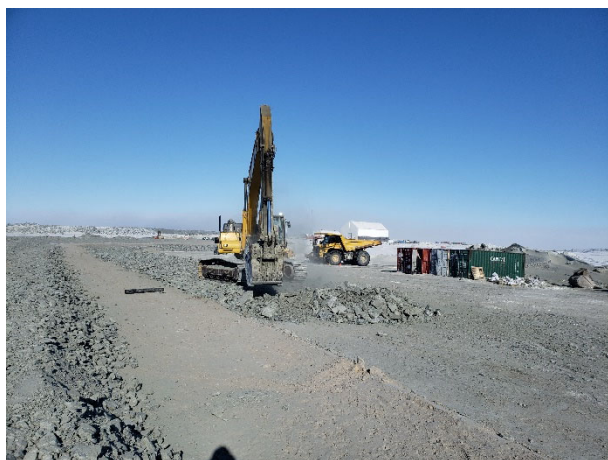
2244: (2021-04-25), looking W from Sta. 0+325. Komatsu excavator placing Zone 1 rockfill.
