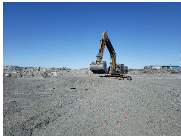
2249: (2021-04-26), looking W from Sta. 0+45. CAT excavator bucket packing placed lift of Zone 2A material.
