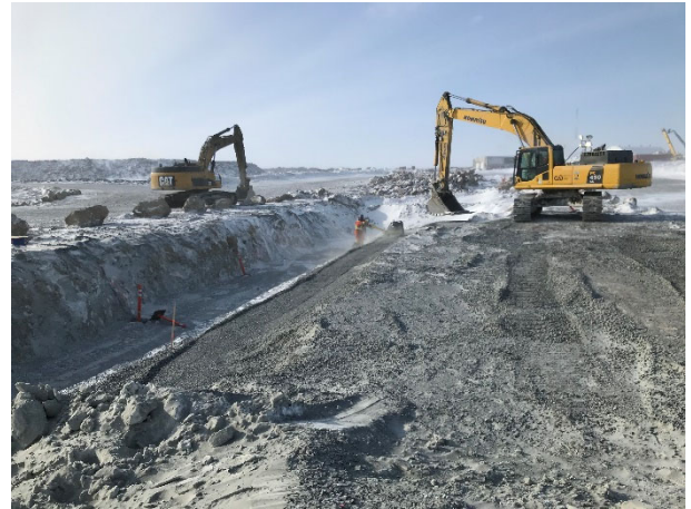
2106: (2021-03-22), looking W from Sta. 0+130. Rebuilding over excavated section between Sta. 0+130 to 0+160.
