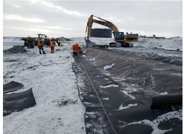
2233: (2021-04-22), looking E from Sta. 0+500. FC liner conducting extrusion weld on LLDPE panels.
