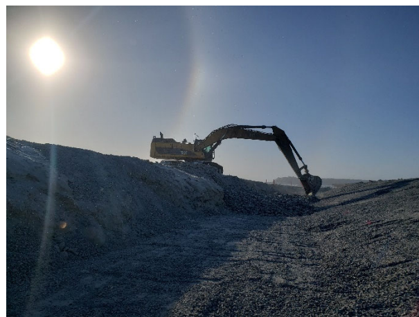
2128: (2021-03-25), looking W from Sta. 0+320. Excavator placing Zone 3 over Zone 2A/2B.
