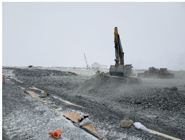
2172: (2021-04-02), looking SE from Sta. 0+090. KCG placing Zone 3 for key trench backfill.
