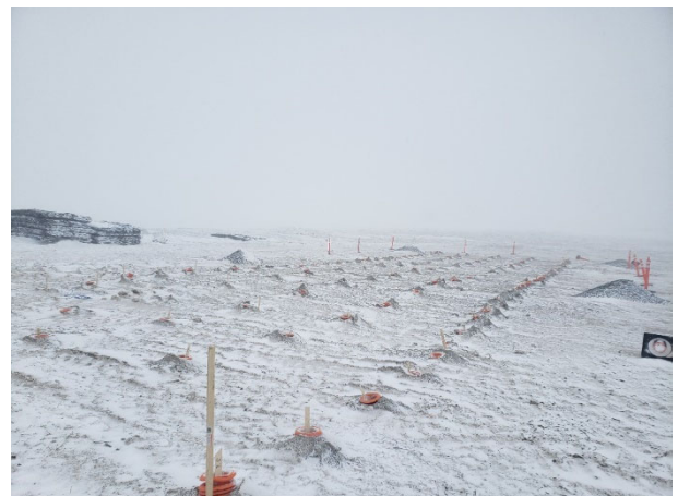
2020: (2021-02-28), looking E from Sta. 0+150. Holes drilled in advance of third blast for key trench construction.
