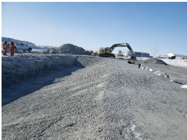
2165: (2021-04-01), looking W from Sta. 0+070. Approved placement of Zone 2A/2B under liner.
