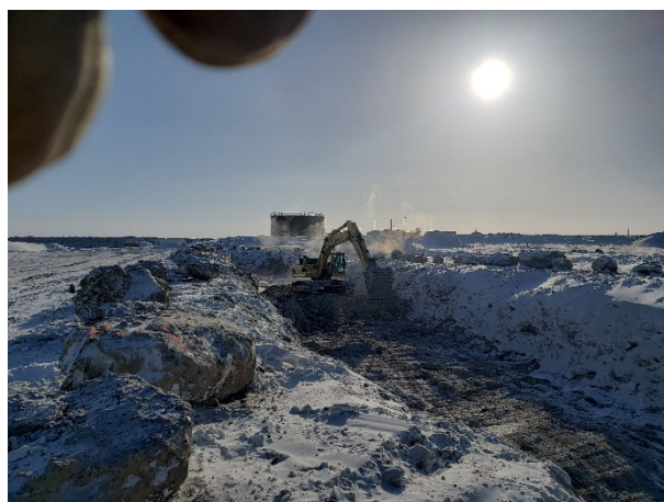
2136: (2021-03-27), looking E from Sta. 0+450. Excavator preparing key trench foundation.
