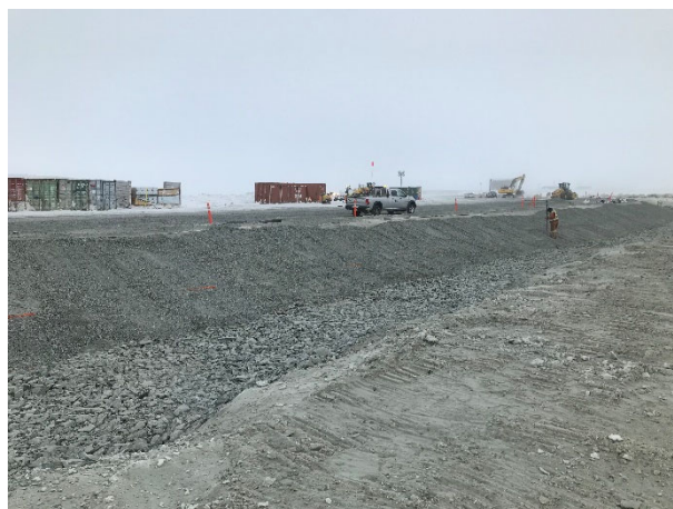
2102: (2021-03-20), looking NE from Sta. 0+165. Zone 2A and Zone 4 on top of LLDPE liner, Sta. 0+165 to Sta. 0+300.
