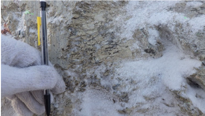
2033: (2021-03-04), looking N from Sta. 0+140. Upstream side wall of key trench excavation: small ice lenses (1-4 mm) observed.
