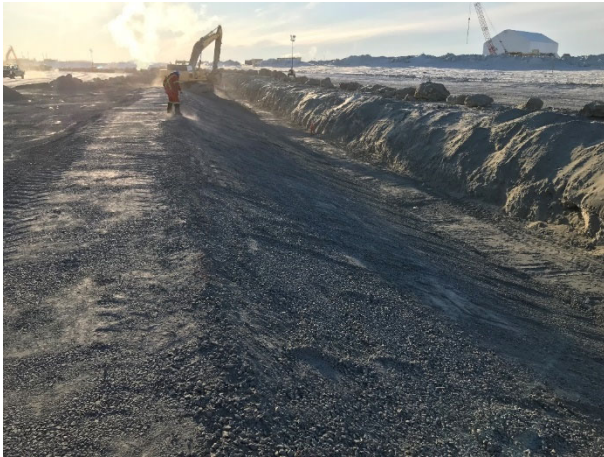
2075: (2021-03-15), looking E from Sta. 0+170. Approved surface for liner placement
