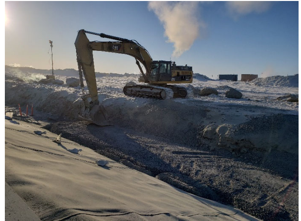
2122: (2021-03-25), looking SE from Sta. 0+330. Approved placement of Zone 2B material over LLDPE liner.
