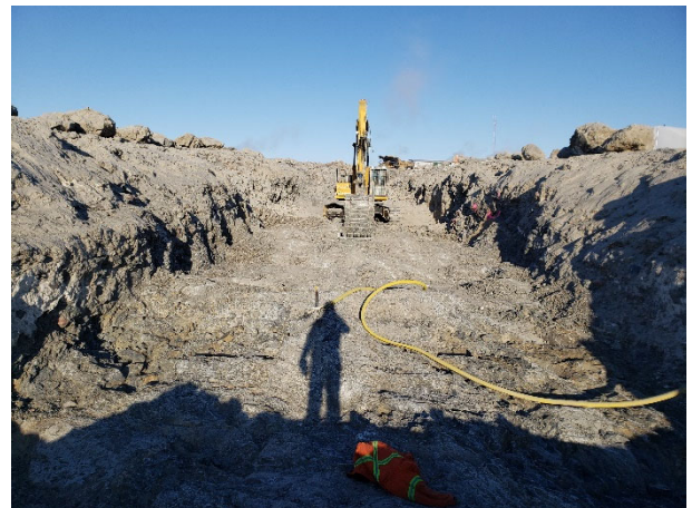
2124: (2021-03-25), looking W from Sta. 0+110. Excavator continuing to prepare key trench foundation.
