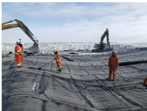
2241: (2021-04-24), looking N from Sta. 0+080. FC Liner heat welding GBM panels P10/P11.
