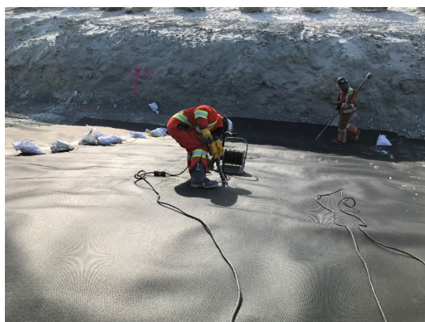
2086: (2021-03-17), looking S from Sta. 0+265. Extrusion weld of R3 on Panel 14.
