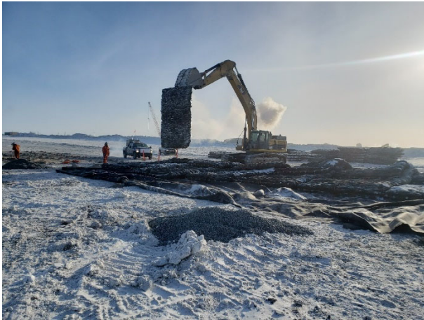
2015: (2021-02-26), looking SE from Sta. 0+130. CAT excavator placing blast mats over geotextile in preparation for second blast schedule for tomorrow.
