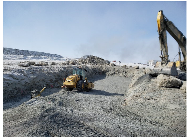
2160: (2021-03-31), looking W from Sta. 0+65. KCG compacting placed lift of Zone 2B material.
