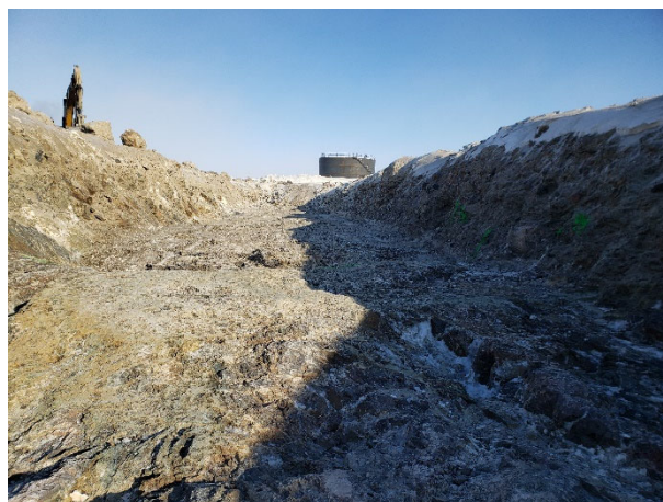
2154: (2021-03-30), looking E from Sta. 0+420. Approved section of key trench.
