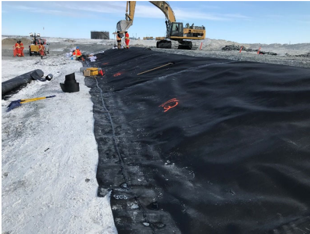
2218: (2021-04-18), looking E from Sta. 0+340. LLDPE liner installation.
