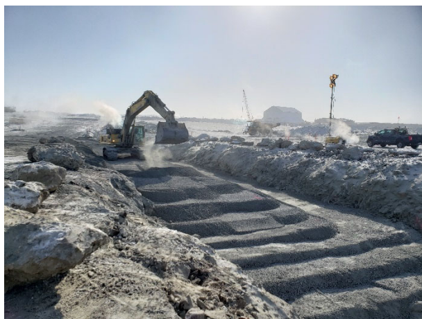
2151: (2021-03-30), looking SE from Sta. 0+090. Excavator placing Zone 2A material.
