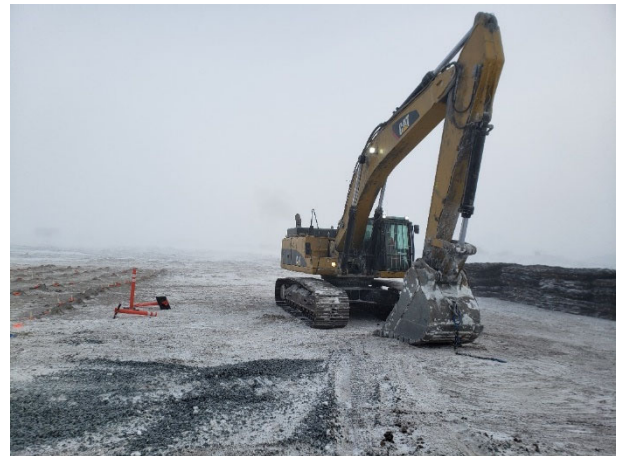
2018: (2021-02-27), looking E from Sta. 0+140. CAT excavator working to remove blast mats over second key trench blast between Sta. 0+129 and Sta. 0+149.
