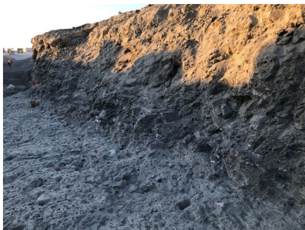
2069: (2021-03-13), looking W from Sta. 0+300. Ice lenses in trench wall from Sta. 0+280 to Sta. 0+300.
