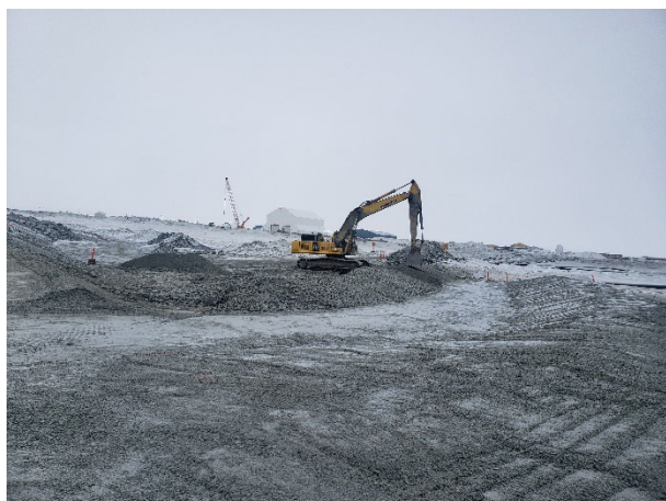
2236: (2021-04-23), looking S from Sta. 0+080. Komatsu excavator placing Zone 2A over spillway slopes.
