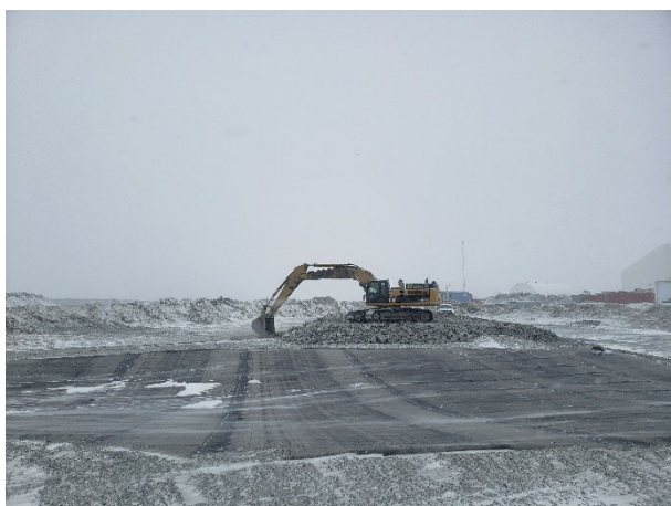
2252: (2021-04-27), looking W from Sta. 0+050. CAT excavator placing Zone 1 along west abutment.
