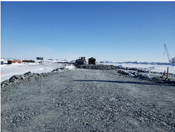
2177: (2021-04-04), looking E from Sta. 0+200. Dozer placing lift of Zone 1 rockfill at approx. Sta. 0+200, view looking E.
