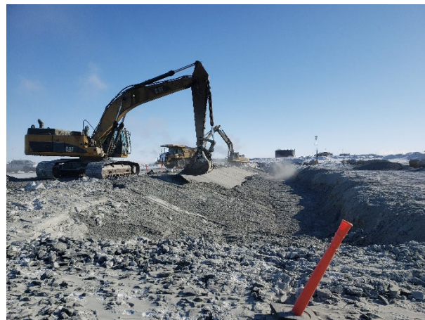
2126: (2021-03-25), looking E from Sta. 0+320. Excavator placing Zone 2A over installed LLDPE.
