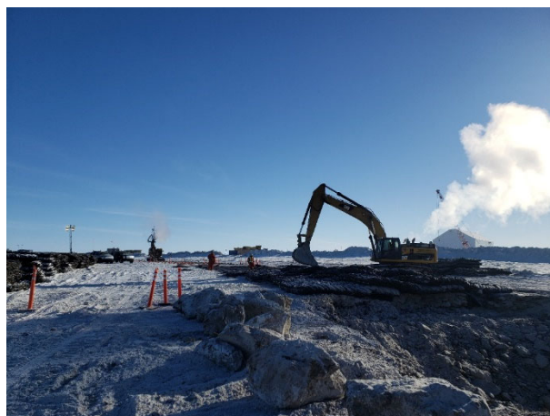
2040: (2021-03-05), looking E from Sta. 0+220. CAT excavator placing blast mats for fifth key trench blast.
