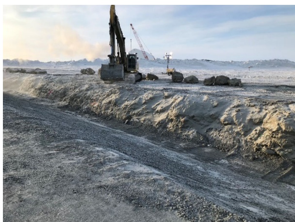
2085: (2021-03-16), looking SE from Sta. 0+240. Excavator cleaning of bedding surface for LLDPE liner at bottom of slope.
