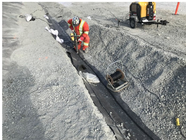
2213: (2021-04-17), looking W from Sta. 0+205. Extrusion weld repair of damaged hinge weld.
