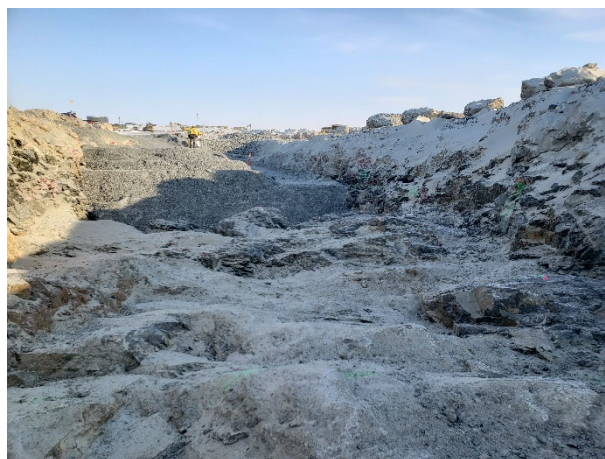
2138: (2021-03-27), looking E from Sta. 0+085. Approved section of key trench foundation.
