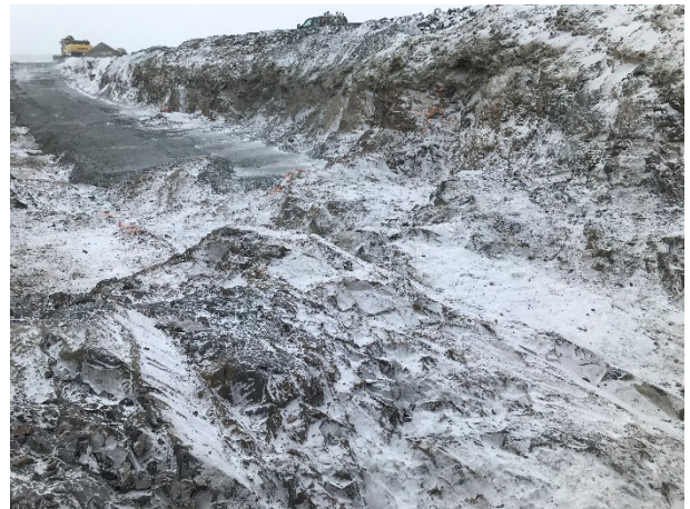
2194: (2021-04-10), looking W from Sta. 0+526. Approved key trench bedrock foundation from Sta. 0+515 to Sta. 0+526. Ice pockets visible on left and right sides of photograph.
