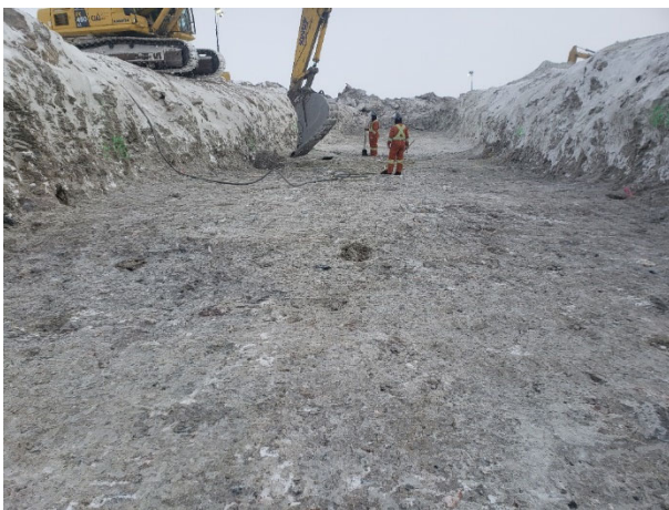
2049: (2021-03-08), looking E from Sta. 0+185. KCG continuing to prepare floor of key trench in advance of Zone 2B FFAB material placement.
