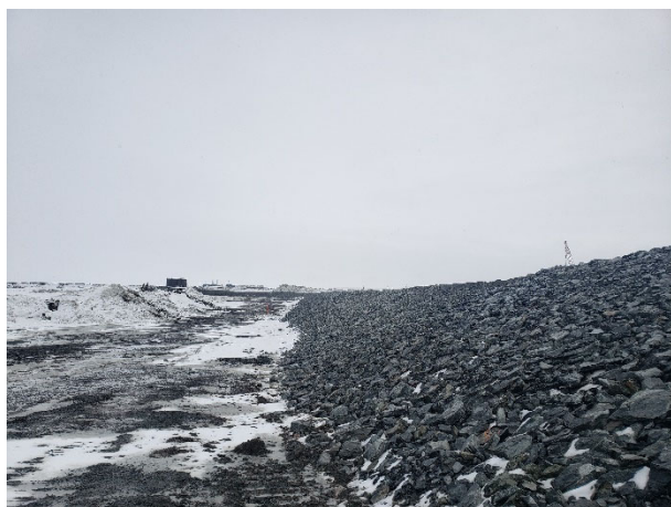
2272: (2021-05-03), looking E from Sta. 0+125. Upstream Zone 1 sloped to design lines.
