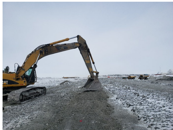
2255: (2021-04-29), looking W from Sta. 0+515. CAT excavator placing Zone 2A over installed LLDPE liner along dyke crest.
