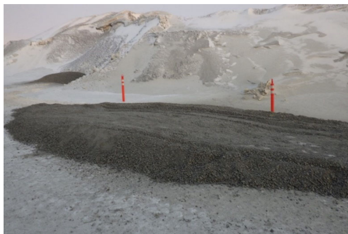
2028: (2021-03-03), looking N at Zone 2A stockpile. Test pad for fine filter Zone 2A material.
