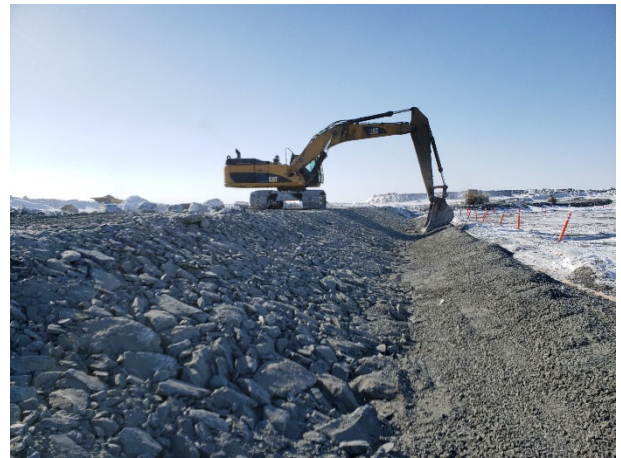
2176: (2021-04-04), looking W from Sta. 0+360. Zone 1 rockfill sloped to design lines at approx. Sta. 0+360, view looking W.
