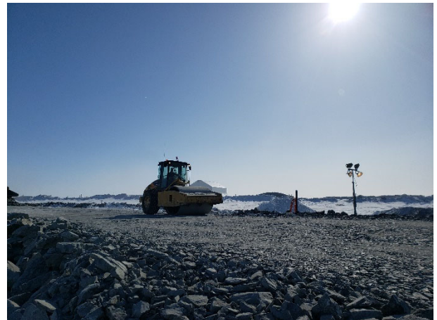
2178: (2021-04-04), looking SE from Sta. 0+185. KCG compacting placed lift of Zone 1 rockfill material at approx. Sta. 0+185, view looking SE.
