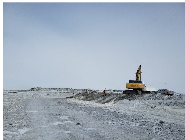
2257: (2021-04-29), looking NW from Sta. 0+400. Komatsu excavator shaping downstream Zone 1 slope to design lines.
