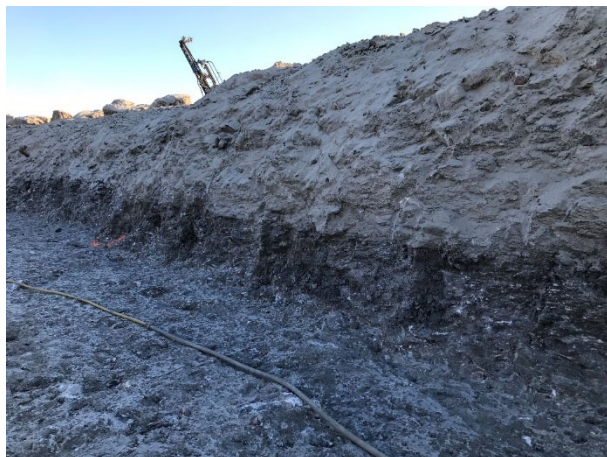
2063: (2021-03-12), looking E from Sta. 0+260. Ice lenses in downstream trench wall from Sta. 0+260 to Sta. 0+270.
