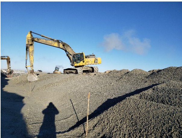
2123: (2021-03-25), looking W from Sta. 0+395. Excavator shaping Zone 2A to design lines.
