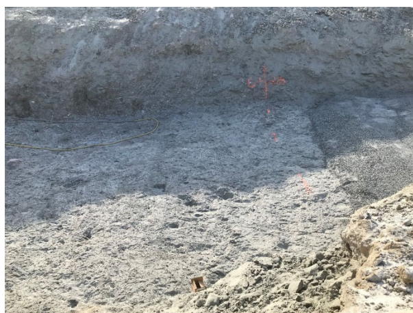
2068: (2021-03-13), looking W from Sta. 0+280. Key trench subgrade foundation approved from Sta. 0+280 to Sta. 0+300.
