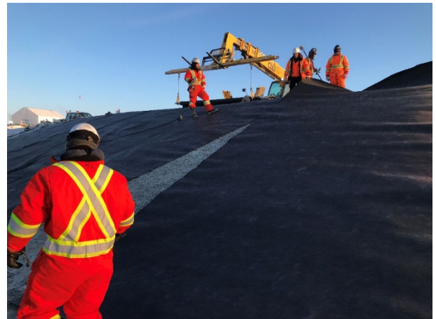
2098: (2021-03-19), looking NW from Sta. 0+310. Installation of geotextile under LLDPE liner.
