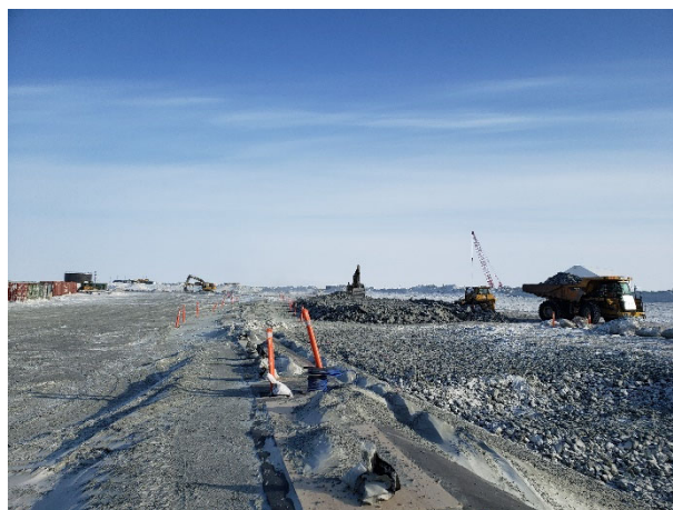
2132: (2021-03-26), looking E from Sta. 0+200. Excavator placing Zone 1 rockfill within footprint of downstream shell.
