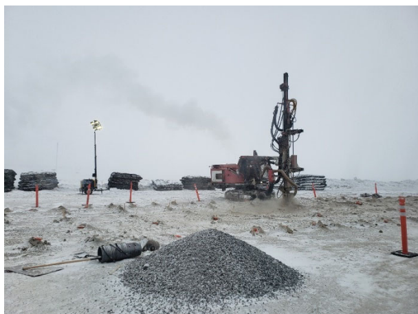
2027: (2021-03-03), looking N from Sta. 0+230. KCG continuing to drill holes for fifth key trench cut.
