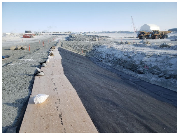
2161: (2021-03-31), looking E from Sta. 0+089. LLDPE liner installed between approx. Sta. 0+120 and Sta. 0+089.
