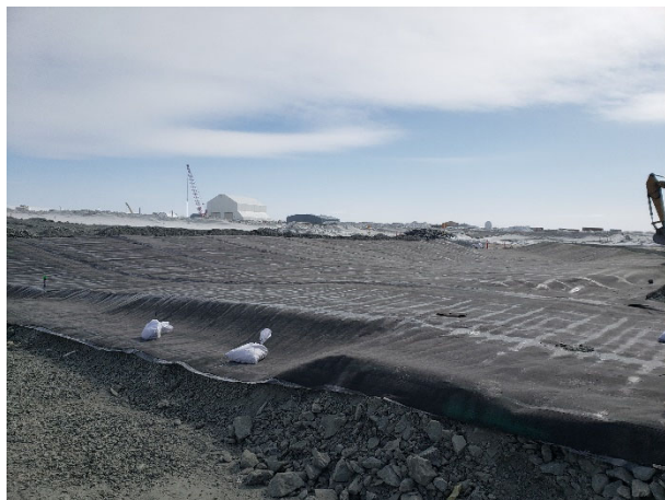
2242: (2021-04-24), looking S from Sta. 0+080. Approved placement of GBM through spillway channel.
