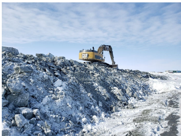
2181: (2021-04-05), looking SW from Sta. 0+200. KCG removing snow over previously placed Zone 2A.
