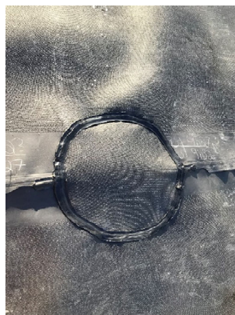
2100: (2021-03-19), looking S from Sta. 0+310. Extrusion welded patch R4 on seam P16/17
