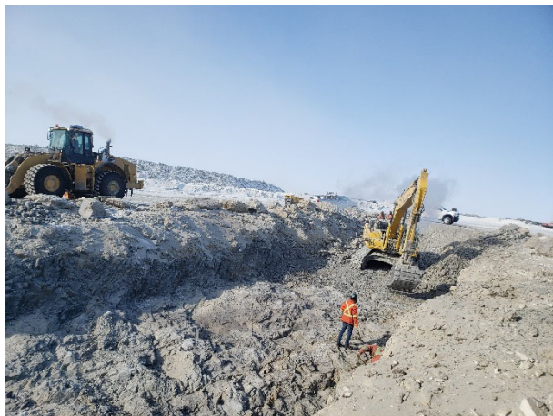
2147: (2021-03-29), looking SW from Sta. 0+065. Excavator preparing key trench foundation.
