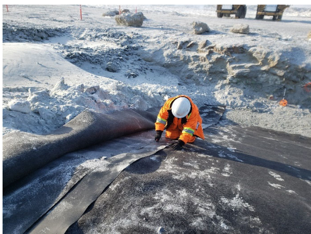
2117: (2021-03-24), looking S from Sta. 0+170. FC liner removing 'smooth' portion of panel P01 at approx. Sta. 0+170 due to damage along seam caused by excavator during snow removal.
