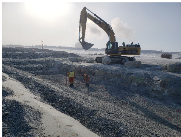
2145: (2021-03-29), looking SE from Sta. 0+140. Excavator removing snow along crest and downstream side walls of trench excavation.
