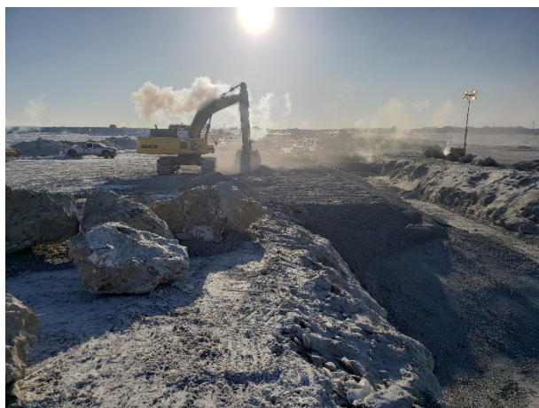
2139: (2021-03-28), looking E from Sta. 0+130. Excavator placing lift of Zone 2A material.
