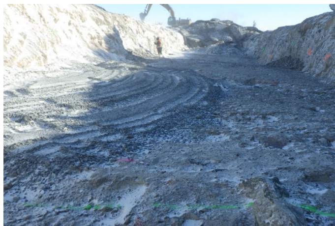
2030: (2021-03-04), looking E from Sta. 0+140. KCG starting to place first 250 mm lift of Zone 2B FFAB material along floor of key trench.
