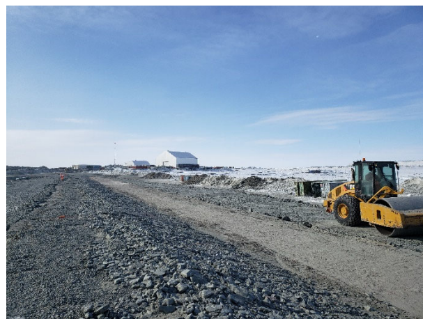
2247: (2021-04-25), looking NW from Sta. 0+280. KCG utilizing smooth drum roller to compact placed Zone 1 rockfill.
