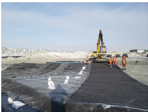
2240: (2021-04-24), looking W from Sta. 0+080. FC liner installing geotextile through spillway channel.
