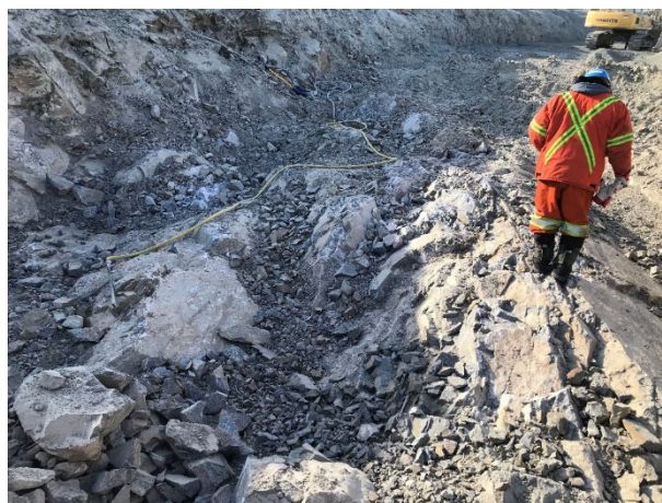
2072: (2021-03-14), looking E from Sta. 0+0+320. Bedrock in key trench foundation.
