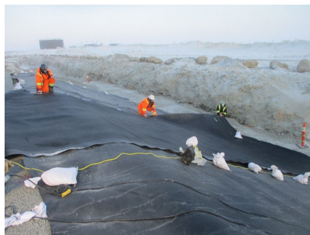
2130: (2021-03-25), looking SW from Sta. 0+150. FC liner installing LLDPE between Sta. 0+150 and Sta. 0+170.
