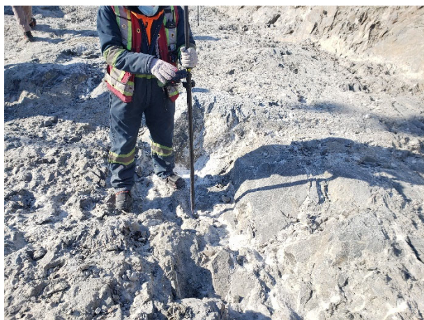
2167: (2021-04-01), looking W from Sta. 0+455. Ice pocket 4.2 meters below ground surface.
