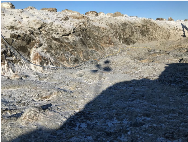
2185: (2021-04-07), looking E from Sta. 0+465. Key trench foundation approved from Sta. 0+465 to Sta. 0+482.
