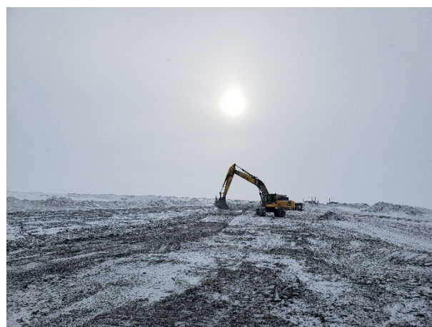
2271: (2021-05-03), looking E from Sta. 0+300. Komatsu excavator leveling dyke crest.
