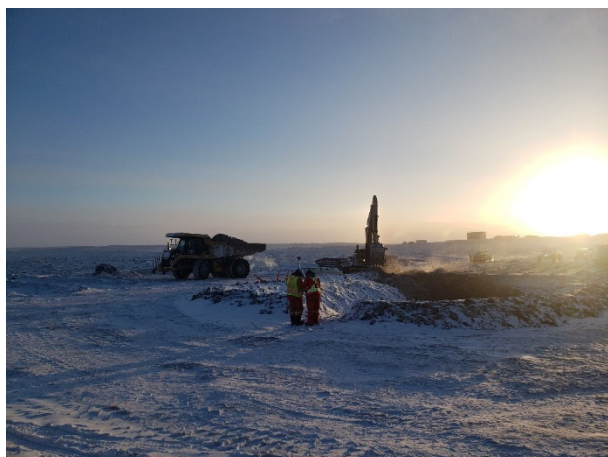
2021: (2021-03-01), looking NE from Sta. 0+120. KCG excavating blasted overburden material from second blast for key trench.
