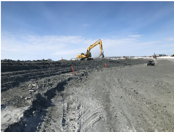
2187: (2021-04-08), looking W from Sta. 0+300. Placement of Zone 2A under liner.
