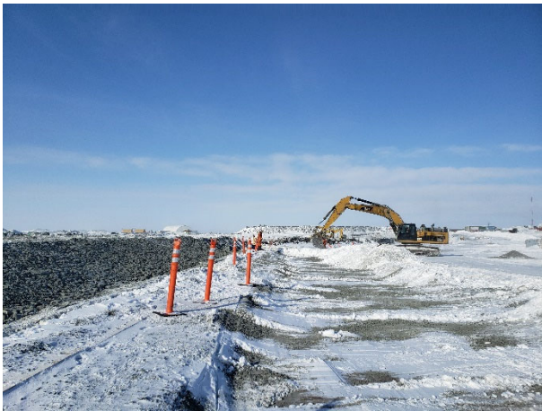
2175: (2021-04-04), looking W from Sta. 0+320. Komatsu excavator removing snow upstream of hinge point.
