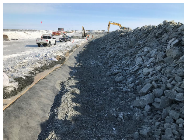
2184: (2021-04-06), looking E from Sta. 0+100. Excavator sloping Zone 1 in advance of Zone 3 placement.
