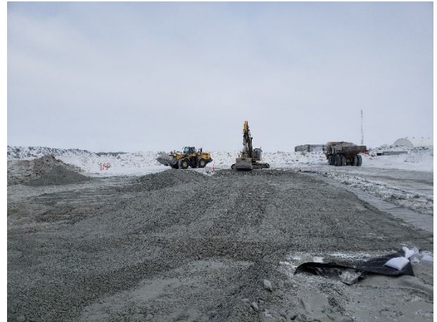
2231: (2021-04-22), looking W from Sta. 0+050. Komatsu excavator placing Zone 2A along west abutment for upper liner slope.
