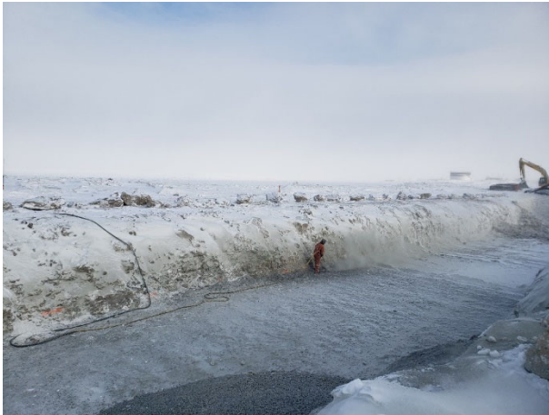
2045: (2021-03-07), looking NE from Sta. 0+130. KCG labourer removing snow along trench excavation side walls in advance of Zone 2B FFAB placement.
