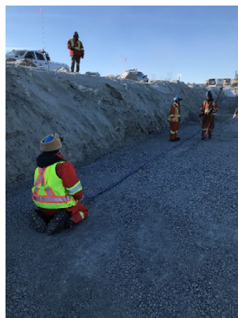
2059: (2021-03-11), looking W from Sta. 0+220. Installation of horizontal thermistor.
