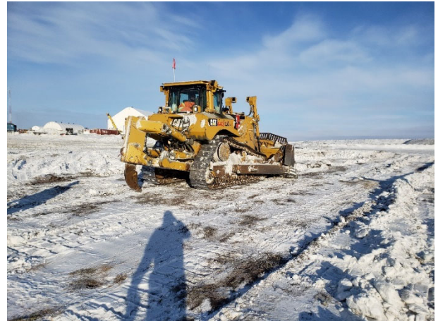
2002: (2021-02-20), looking N from Sta. 0+160. CAT dozer continuing to remove snow and organics within footprint of downstream shell at Dyke D1.
