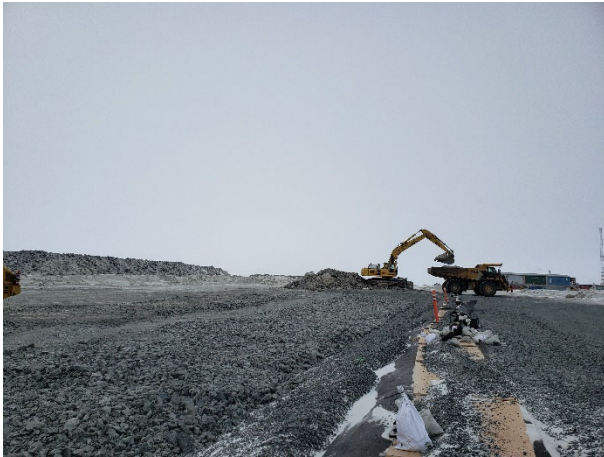
2173: (2021-04-02), looking W from Sta. 0+040. Komatsu excavator loading rock truck with stockpiled overburden material.
