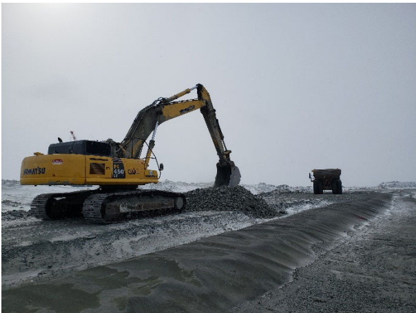
2228: (2021-04-21), looking SW from Sta. 0+380. Komatsu excavator placing Zone 3 along dyke crest over installed LLDPE liner.
