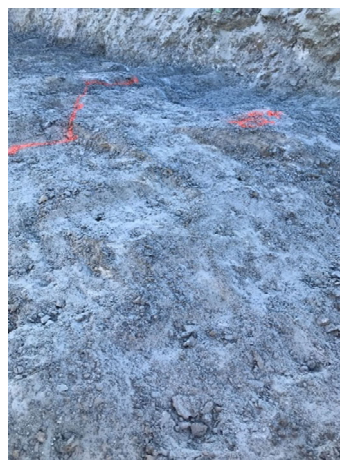
2054: (2021-03-10), looking E from Sta. 0+225. High spot of subgrade foundation (50 mm too high).
