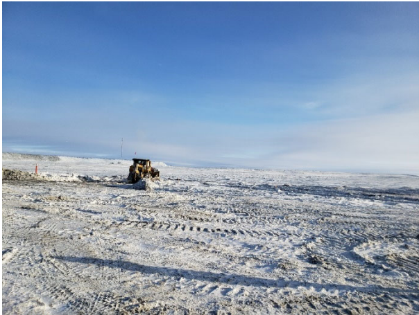
2001: (2021-02-20), looking NE from Sta. 0+100. CAT dozer removing snow within footprint of upstream shell at Dyke D1.
