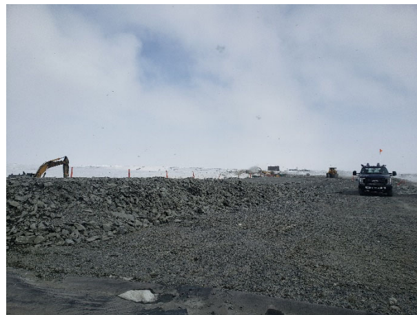
2259: (2021-04-29), looking E from Sta. 0+090. Zone 2A and Zone 3 placed over existing LLDPE liner.
