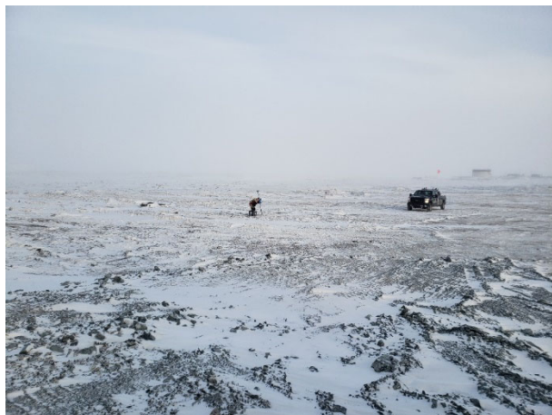
2007: (2021-02-22), looking E from Sta. 0+060. Surveyor laying out drill pattern in preparation for drilling activities scheduled for tomorrow.
