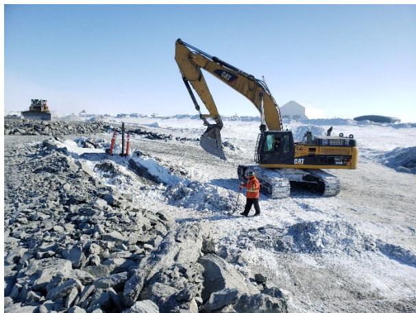
2179: (2021-04-04), looking SE from Sta. 0+185. CAT excavator removing snow within footprint of downstream shell near existing thermistor.
