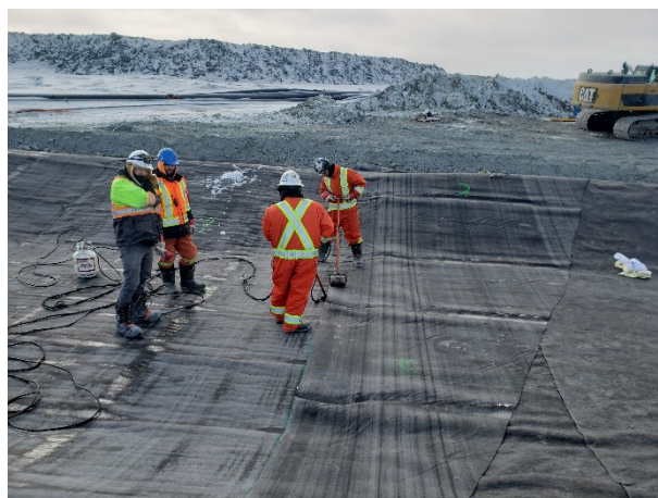
2239: (2021-04-23), looking W from Sta. 0+080. FC Liner heat welding GBM panels P1/P2.
