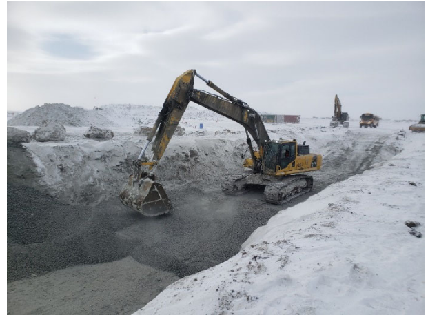
2046: (2021-03-07), looking W from Sta. 0+145. CAT excavator placing 250 mm lift of Zone 2B FFAB material.
