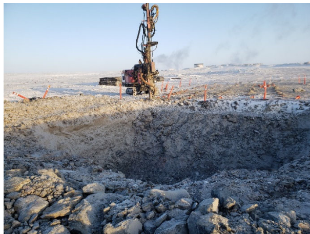
2013: (2021-02-25), looking E from Sta. 0+115. Key trench excavation from first blast between Sta. 0+117 and Sta. 0+129.
