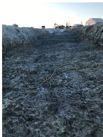
2053: (2021-03-10), looking E from Sta. 0+205. Key trench foundation approved, Sta. 0+205 to 0+227.
