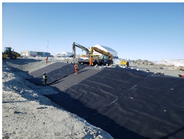
2168: (2021-04-01), looking NW from Sta. 0+070. FC Liner installing LLDPE liner panels.
