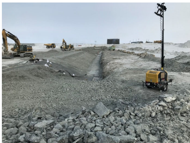
2199: (2021-04-12), looking E from Sta. 0+400. Zone 2A in key trench sloped 3H:1V in preparation for LLDPE liner installation.
