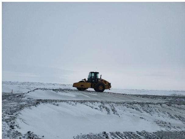
2266: (2021-05-02), looking SE from Sta. 0+090. KCG utilizing smooth drum roller to compact placed Zone 1.
