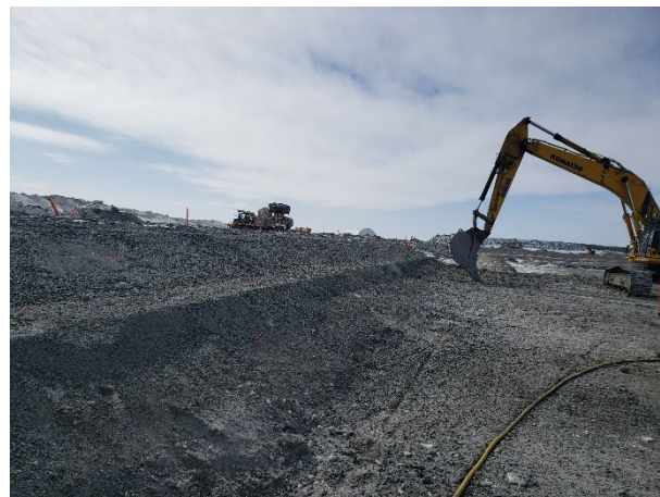
2243: (2021-04-24), looking W from Sta. 0+375. Komatsu excavator removing snow over footprint of upstream shell in advance of Zone 4 placement.
