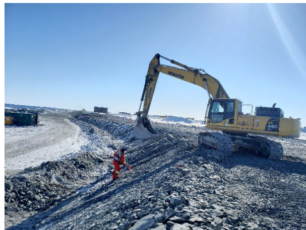
2261: (2021-04-30), looking E from Sta. 0+300. Komatsu excavator shaping upstream Zone 1 (rockfill) to design lines.
