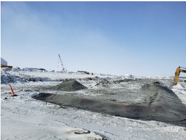
2234: (2021-04-22), looking W from Sta. 0+520. Geotextile installed over LLDPE liner placed along east abutment.
