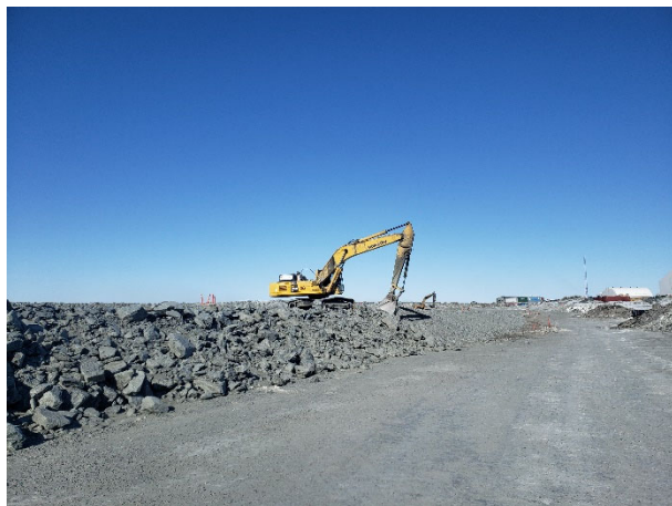
2248: (2021-04-26), looking W from Sta. 0+120. Komatsu excavator shaping Zone 1 to design lines.
