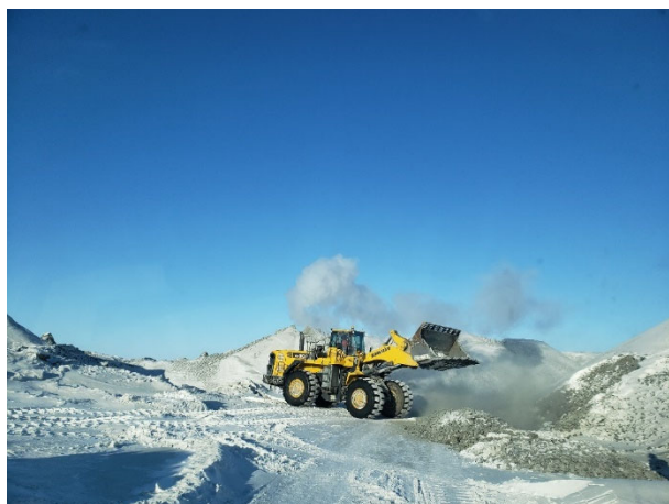
2010: (2021-02-24), looking E from Zone 3 stockpile at WSRF. KCG loader creating test pad for Zone 3 material.
