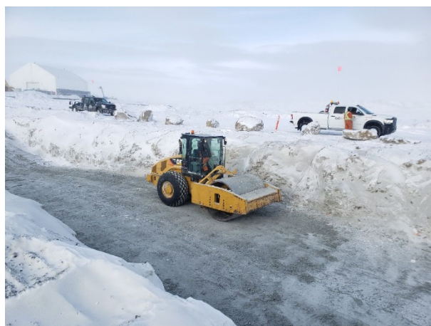
2044: (2021-03-07), looking NW from Sta. 0+140. Smooth drum roller compacting placed lift of Zone 2B FFAB material.
