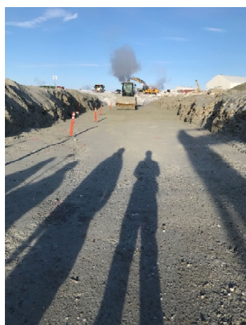
2055: (2021-03-10), looking W from Sta. 0+0+180. Fill placement approved for placement of Zone 2A on top of Zone 2B from Sta. 0+180 to Sta. 0+205.
