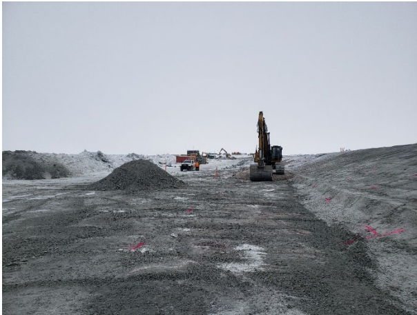
2224: (2021-04-21), looking E from Sta. 0+130. Komatsu excavator placing Zone 4 material upstream of installed LLDPE liner.
