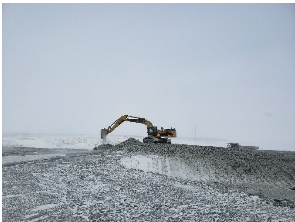
2264: (2021-05-01), looking N from Sta. 0+085. CAT excavator placing Zone 1 (rockfill) for thermal berm.
