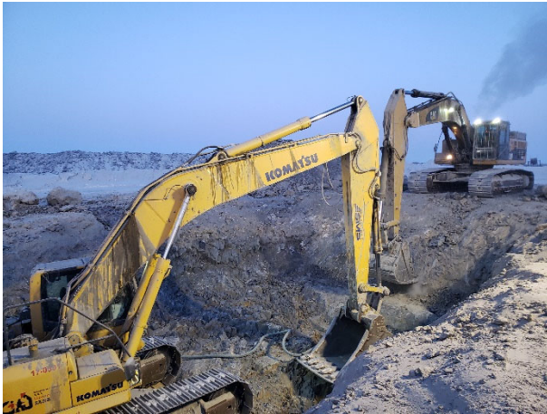
2155: (2021-03-31), looking SW from Sta. 0+055. KCG continuing to clean key trench between Sta. 0+055 and Sta. 0+045.
