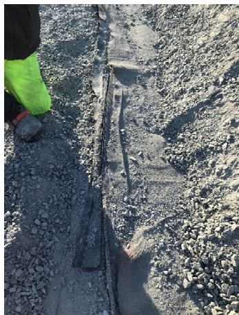
2212: (2021-04-17), looking E from Sta. 0+200. Exposed hinge weld damage.
