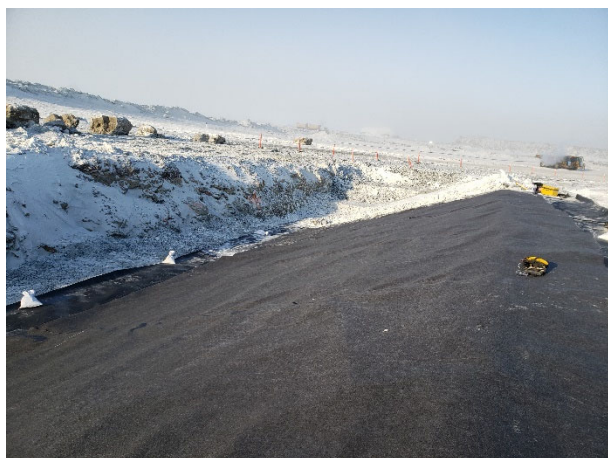
2115: (2021-03-24), looking W from Sta. 0+335. Geotextile installed over LLDPE liner between approx. Sta. 0+335 and Sta. 0+315.
