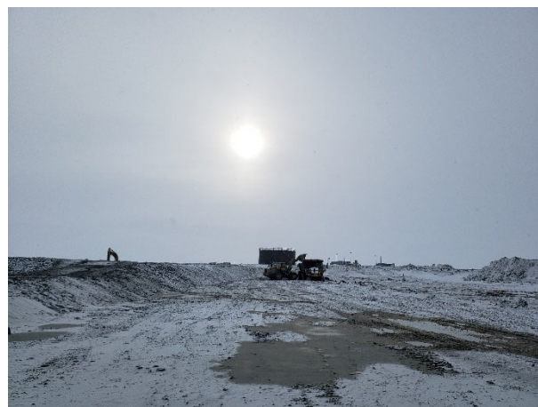
2269: (2021-05-03), looking E from Sta. 0+500. Loader loading rock truck with overburden/waste rock material downstream of IVR dyke.
