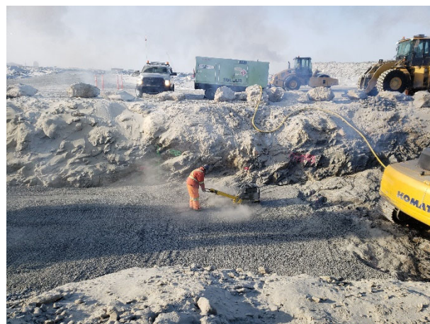
2146: (2021-03-29), looking S from Sta. 0+085. KCG labourer using plate tamper to compact first lift of Zone 2B over bedrock.
