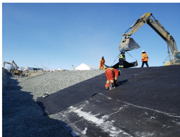
2142: (2021-03-28), looking NW from Sta. 0+140. FC liner installing geotextile.
