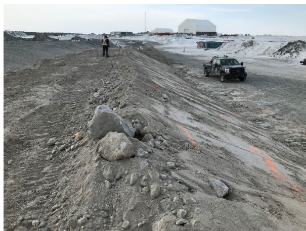
2217: (2021-04-18), looking W from Sta. 0+280. Esker material placed and sloped.
