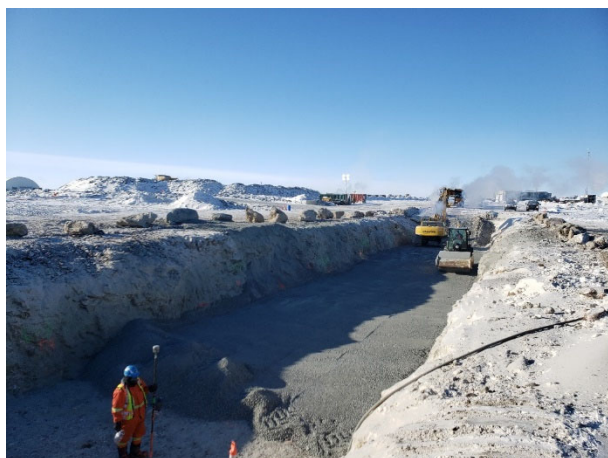
2041: (2021-03-05), looking W from Sta. 0+190. KCG compacting second placed lift of FFAB material.
