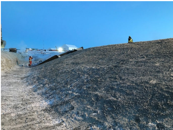
2097: (2021-03-19), looking W from Sta. 0+315. Approved bedding surface for geotextile/geomembrane.
