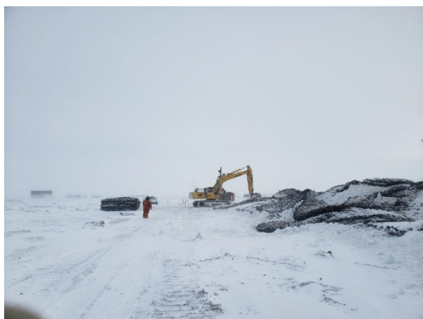
2043: (2021-03-07), looking E from Sta. 0+275. CAT excavator removing snow along tie in between sequence 6 and 7 in advance of drilling.
