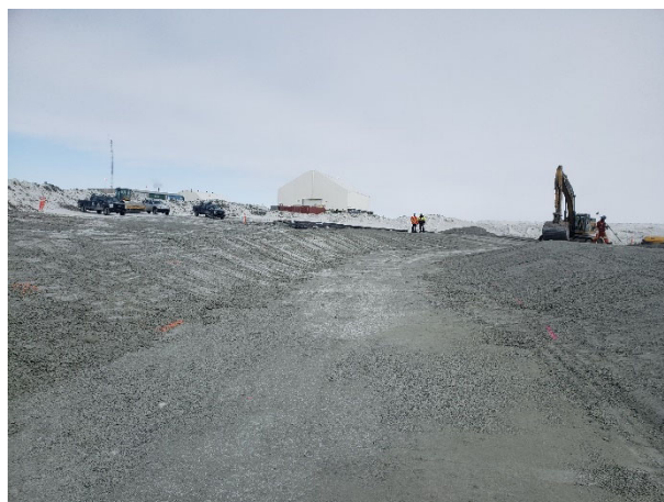
2237: (2021-04-23), looking N from Sta. 0+080. Approved placement of Zone 2A in spillway channel.
