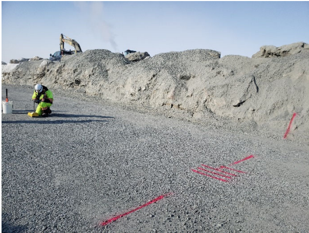
2121: (2021-03-24), looking W from Sta. 0+405. QC conducting compaction testing on placed Zone 2B material.
