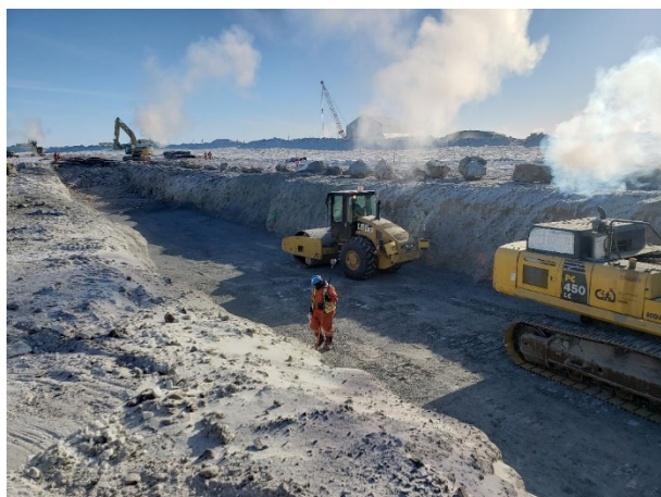
2039: (2021-03-05), looking SE from Sta. 0+150. KCG compacting first placed lift of FFAB material.
