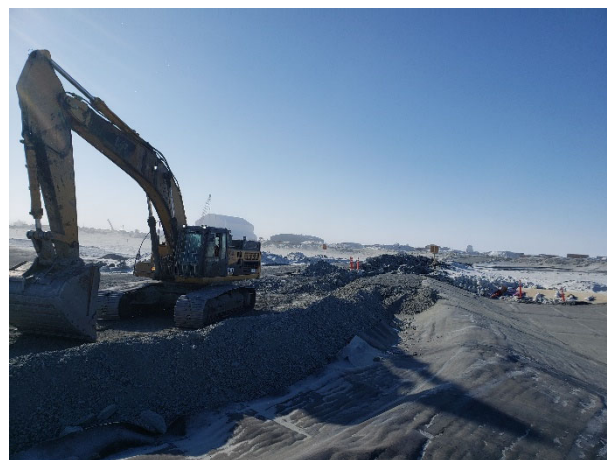
2245: (2021-04-25), looking S from Sta. 0+080. CAT excavator placing Zone 2A (FF) over installed geotextile/GBM.
