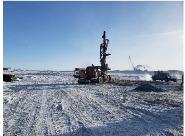
2016: (2021-02-26), looking E from Sta. 0+140. KCG drilling holes for third key trench blast.
