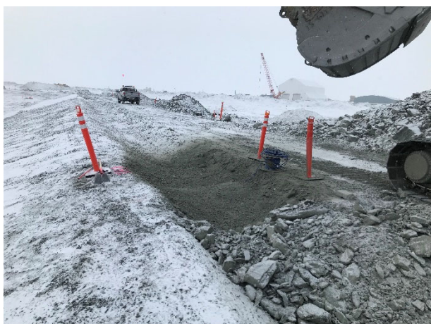
2210: (2021-04-16), looking E from Sta. 0+0+230. Trench for LLDPE liner tie-in.
