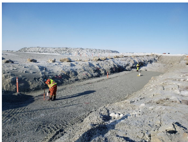
2137: (2021-03-27), looking SW from Sta. 0+110. QC representative conducting PNG testing on placed Zone 2A material.
