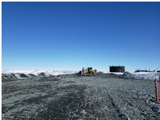
2260: (2021-04-30), looking E from Sta. 0+490. Komatsu dozer placing Zone 1 (rockfill) material for thermal berm along east abutment.
