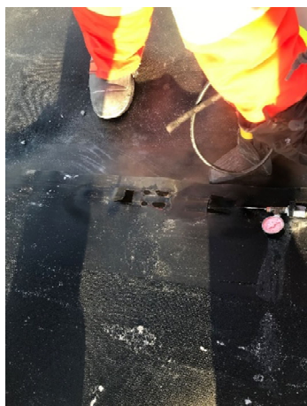
2099: (2021-03-19), looking W from Sta. 0+310. Damage to seam P16/17 due to stuck welder
