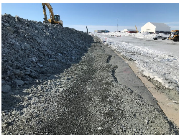
2183: (2021-04-06), looking W from Sta. 0+195. Snow removed over Zone 2A in advance of Zone 3 placement.
