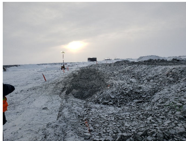
2180: (2021-04-05), looking E from Sta. 0+310. Lift of Zone 3 and Zone 2A placed during KCG nightshift.
