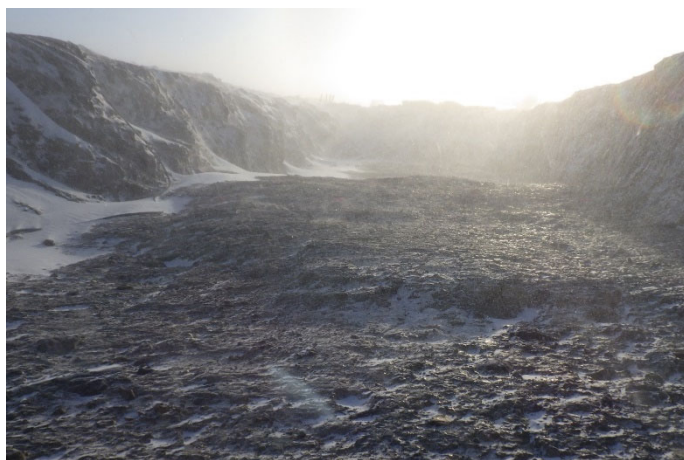
2029: (2021-03-04), looking W from Sta. 0+0+160. Key trench excavation prepared between Sta. 0+130 and Sta. 0+160.
