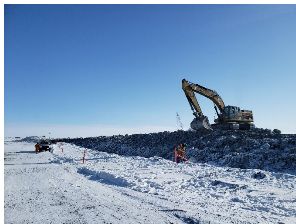
2182: (2021-04-05), looking SE from Sta. 0+165. CAT excavator sloping Zone 1 rockfill to design lines along upstream slope.
