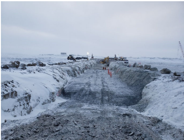
2047: (2021-03-08), looking E from Sta. 0+130. Zone 2B FFAB material placed to approx. elev. 160.0 m (2.5 m below existing ground). Area approved for placement of fine filter.
