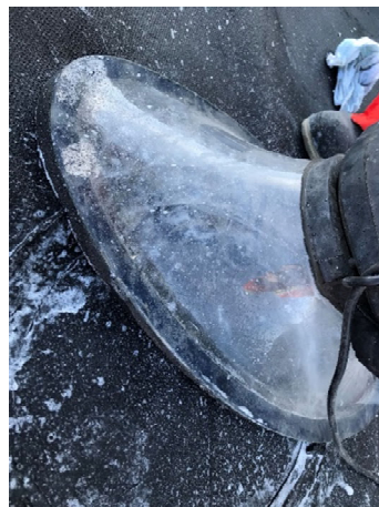
2088: (2021-03-17), looking S from Sta. 0+265. Vacuum box test on patch R3, Panel 14.
