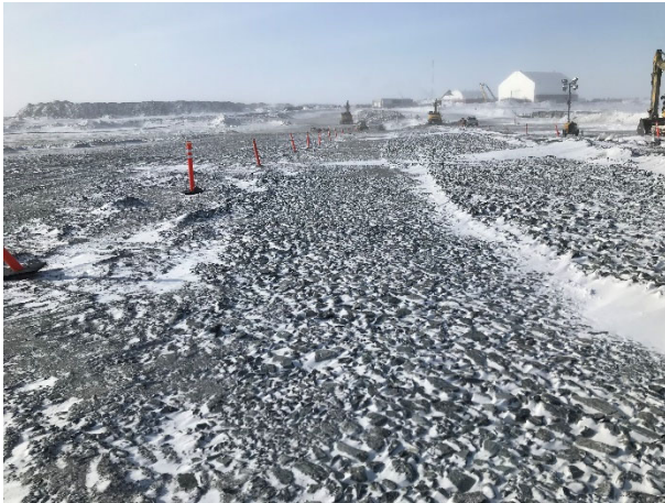
2105: (2021-03-22), looking W from Sta. 0+0+165. Approved downstream dam footprint foundation between Sta. 0+165 and Sta. 0+318.
