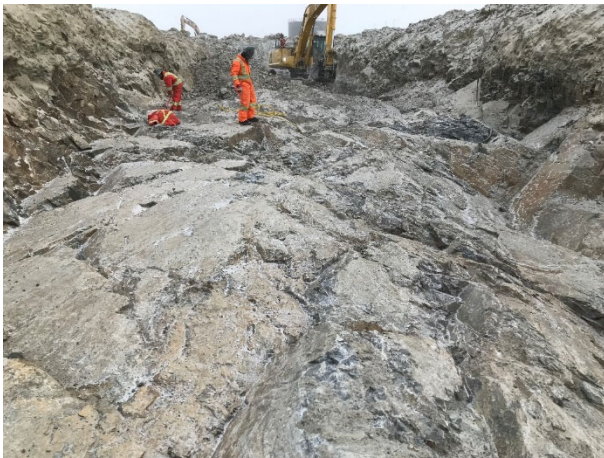
2095: (2021-03-18), looking E from Sta. 0+377. Approved key trench foundation, Sta. 0+377 to 0+388.
