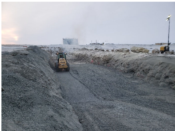
2171: (2021-04-02), looking E from Sta. 0+460. KCG compacting placed Zone 2B material.
