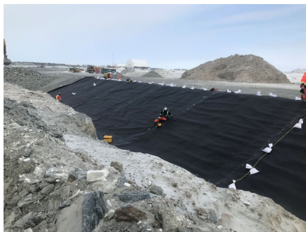
2205: (2021-04-14), looking S from Sta. 0+0+437. Liner installation, between Sta. 0+437 to Sta. 0+519.
