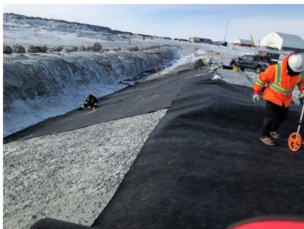
2083: (2021-03-16), looking W from Sta. 0+250. Geotextile installation on lower key trench slope
