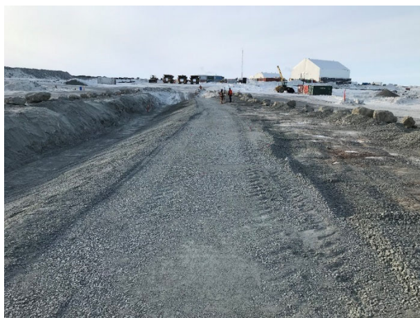
2071: (2021-03-14), looking W from Sta. 0+270. Zone 2A material placed to original ground level.
