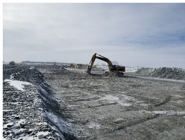
2253: (2021-04-28), looking W from Sta. 0+430. CAT excavator removing snow/ice within footprint of Zone 1 rockfill.
