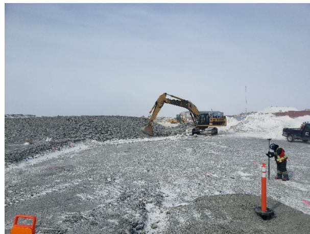
2265: (2021-05-01), looking W from Sta. 0+060. CAT excavator removing snow within footprint of spillway.
