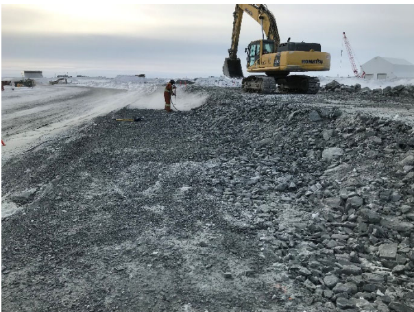
2189: (2021-04-09), looking E from Sta. 0+200. Snow being removed along upstream under liner hinge.
