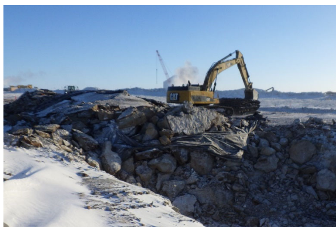
2032: (2021-03-04), looking SE from Sta. 0+0+185. CAT excavator removing blast mats at the IVR Dyke.
