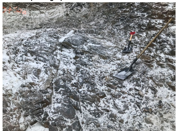
2196: (2021-04-10), looking E from Sta. 0+520. Closely spaced joint set/fracture zone on downstream side of key trench foundation.
