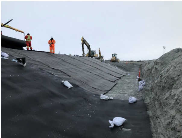
2077: (2021-03-15), looking E from Sta. 0+170. Liner installation.
