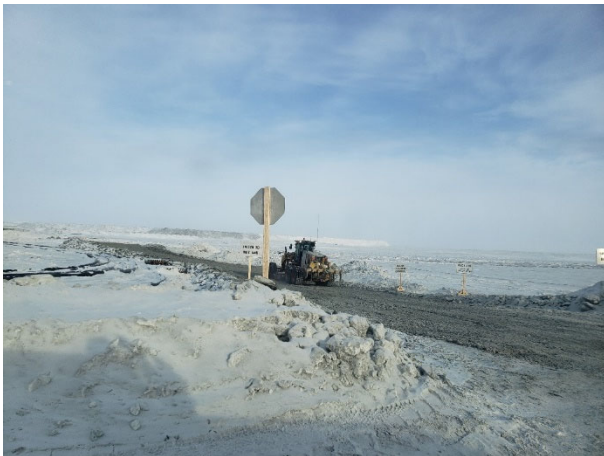
2003: (2021-02-21), looking NE from west dyke access. CAT grader improving road access along west abutment of IVR Dyke.
