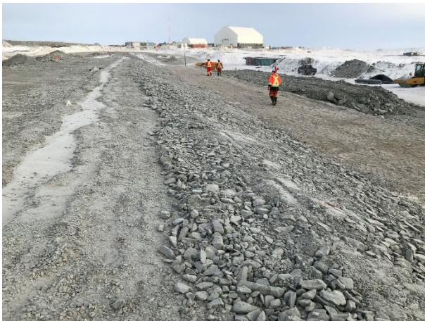
2220: (2021-04-19), looking W from Sta. 0+250. Zone 3 placed on upstream slope.
