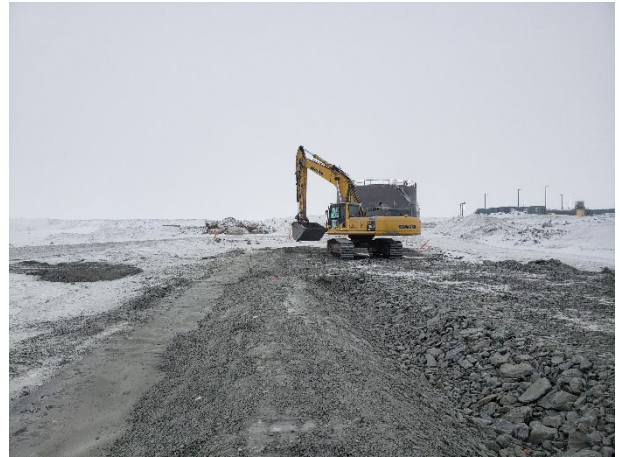
2225: (2021-04-21), looking E from Sta. 0+500. Komatsu excavator placing Zone 2A along east abutment in advance of liner placement.
