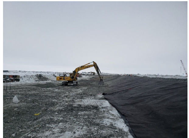
2221: (2021-04-20), looking E from Sta. 0+130. Komatsu excavator placing Zone 2B over liner.
