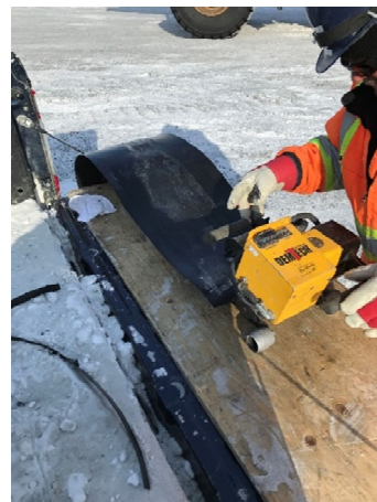
2080: (2021-03-16), Calibration weld of LLDPE liner.
