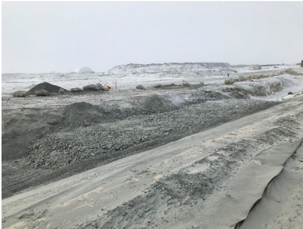
2093: (2021-03-18), looking SW from Sta. 0+320. Placement of Zone 4 on top of Zone 2B overlying liner.
