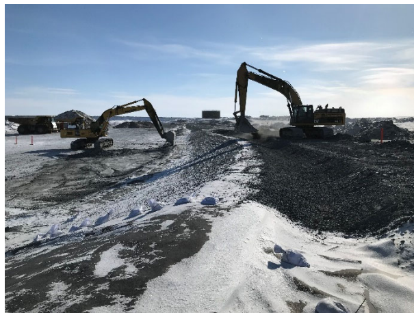
2215: (2021-04-17), looking E from Sta. 0+220. Snow removal and tie-in trench preparation for LLDPE liner installation.
