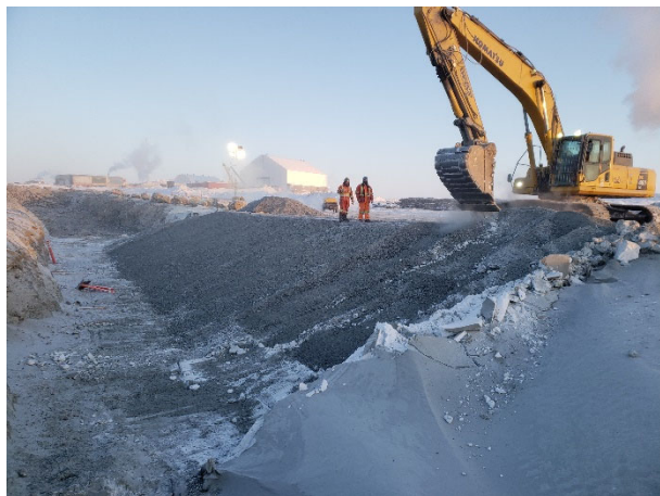
2113: (2021-03-24), looking NW from Sta. 0+175. Excavator shaping Zone 2A to design lines at approx. Sta. 0+175.
