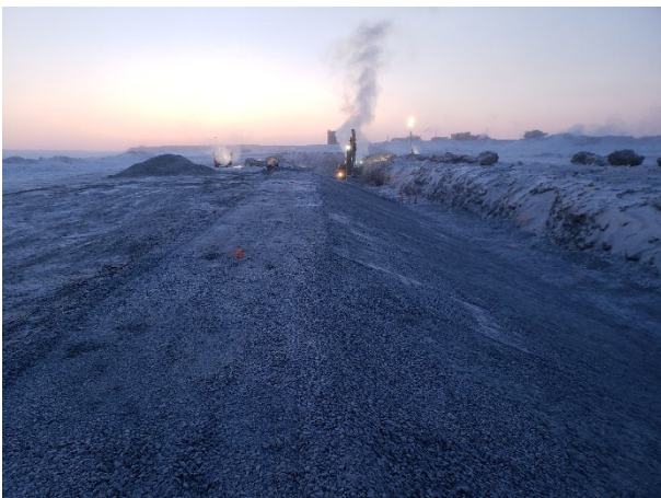
2111: (2021-03-24), looking E from Sta. 0+315. Fill placement of Zone 2B material under liner.
