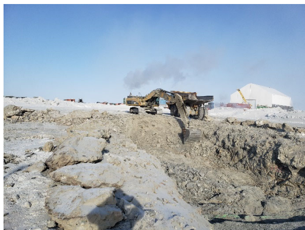
2150: (2021-03-30), looking NW from Sta. 0+060. Excavator removing blasted material to prepare key trench foundation.
