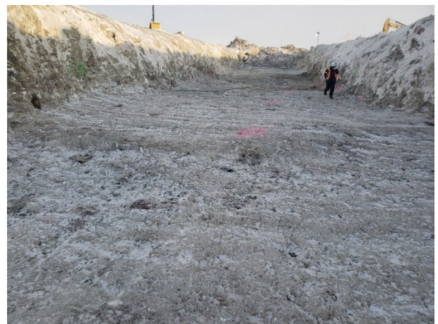
2050: (2021-03-08), looking E from Sta. 0+180. Key trench foundation approved between Sta. 0+180 and Sta. 0+205.
