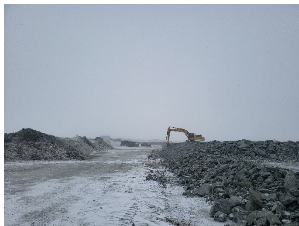
2251: (2021-04-27), looking E from Sta. 0+200. Komatsu excavator sloping upstream Zone 1 to design lines.
