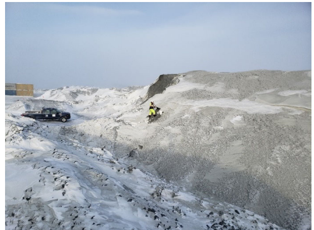
2006: (2021-02-22), Tetra Tech QC sampling Zone 2A filter material from southern face of existing stockpile.
