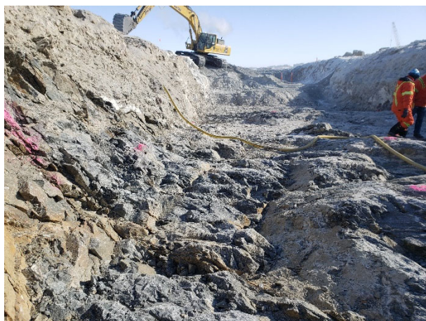
2127: (2021-03-25), looking E from Sta. 0+115. Prepared section of key trench.
