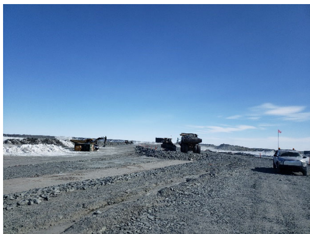
2250: (2021-04-26), looking W from Sta. 0+270. Dozer spreading Zone 1 material.
