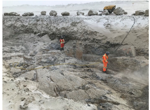
2094: (2021-03-18), looking SE from Sta. 0+372. Cleaning of bedrock surface in key trench.
