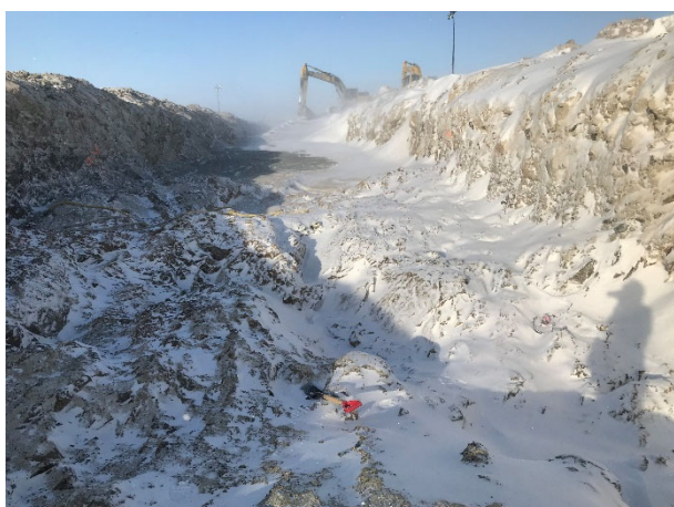
2103: (2021-03-21), looking W from Sta. 0+423. Key trench bedrock foundation from Sta. 0+423 to Sta. 0+445.
