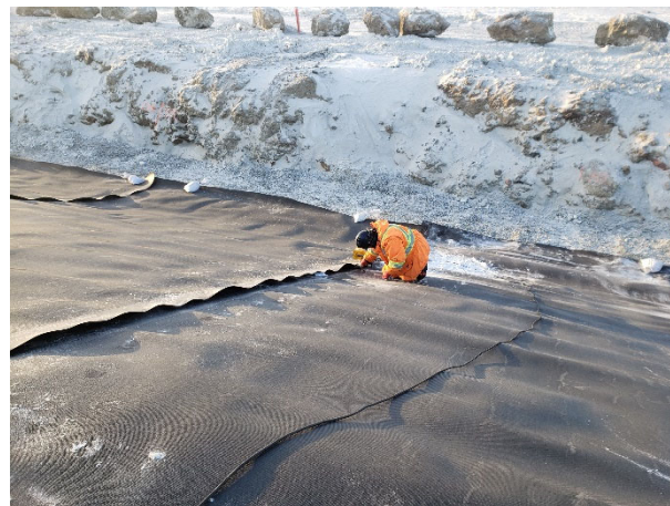
2114: (2021-03-24), looking S from Sta. 0+320. FC liner welding LLDPE liner Sta. 0+321 between panel seams P23/P24.
