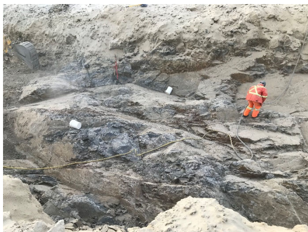
2101: (2021-03-20), looking S from Sta. 0+408. Approved key trench bedrock foundation, Sta. 0+408 to Sta. 0+423.
