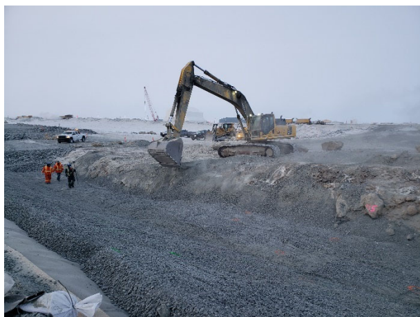
2169: (2021-04-02), looking SE from Sta. 0+070. Komatsu excavator removing snow along downstream crest of key trench.
