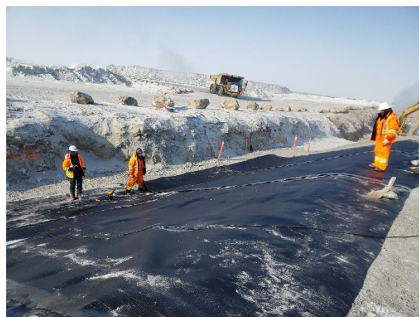
2118: (2021-03-24), looking SW from Sta. 0+165. FC liner installing LLDPE between approx. Sta. 0+165 and Sta. 0+135.
