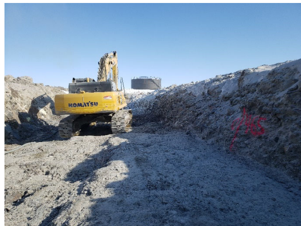
2166: (2021-04-01), looking E from Sta. 0+450. Approved section of key trench.
