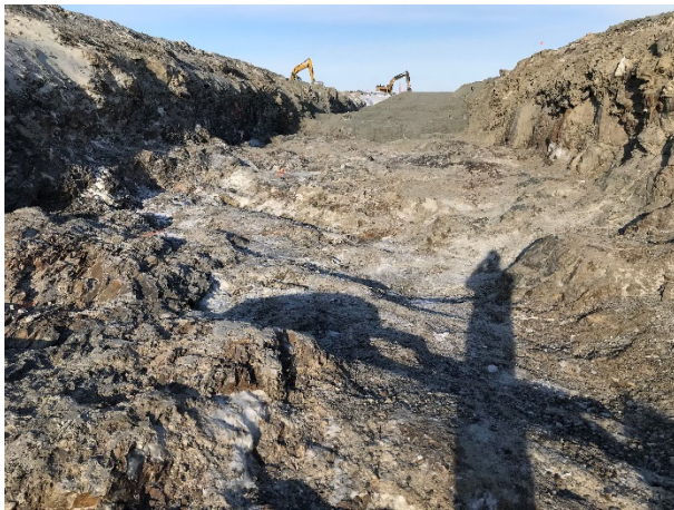
2193: (2021-04-10), looking W from Sta. 0+515. Approved key trench bedrock foundation, Sta. 0+482 to Sta. 0+515.
