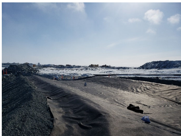
2238: (2021-04-23), looking SW from Sta. 0+080. GBM installed along spillway channel.
