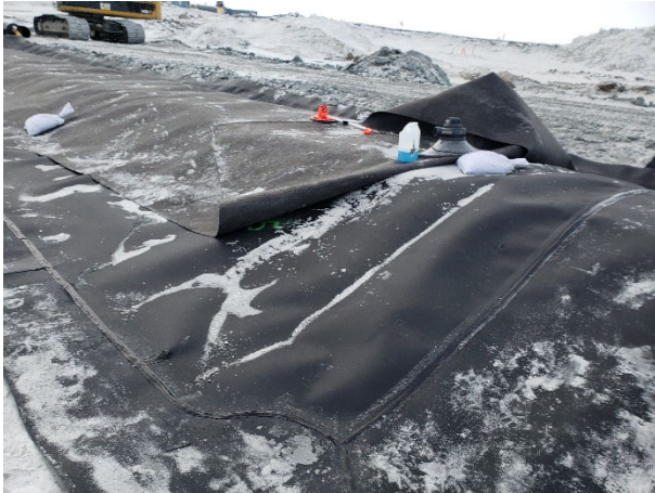
2232: (2021-04-22), looking SE from Sta. 0+483. Extrusion weld between panels P124/P125.
