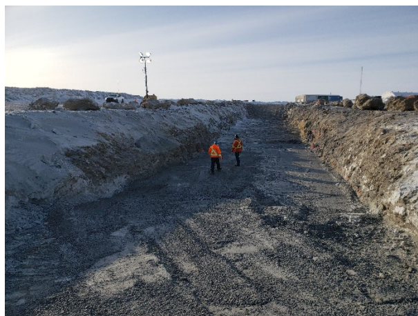
2134: (2021-03-26), looking W from Sta. 0+130. Snow removed over previously placed Zone 2B in preparation for additional placement during nightshift.
