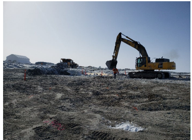
2235: (2021-04-22), looking S from Sta. 0+080. Komatsu excavator removing snow and ice from foundation of key trench.
