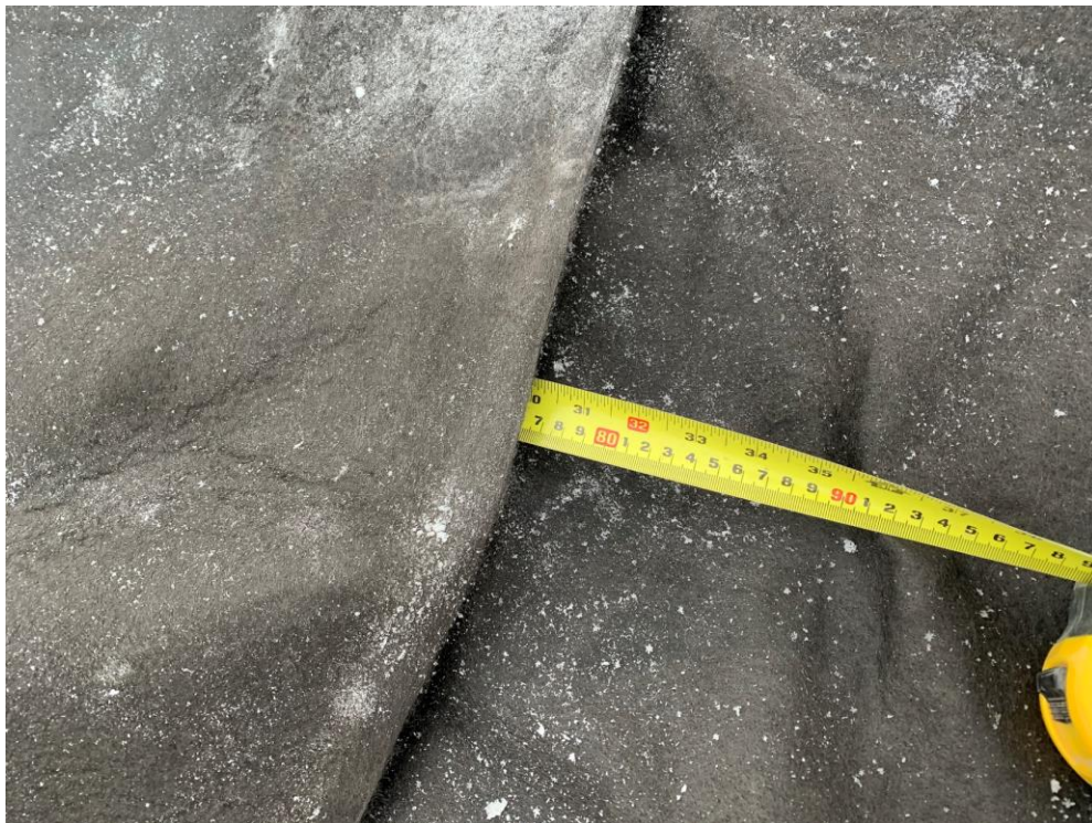
Figure 12: All the overlaps measured are conforming to minimum requirement of 600
