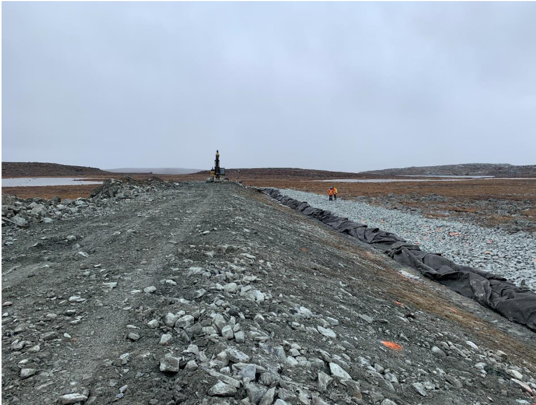
Figure 1: Access road slope completed between 0+188 and 0+284.5
