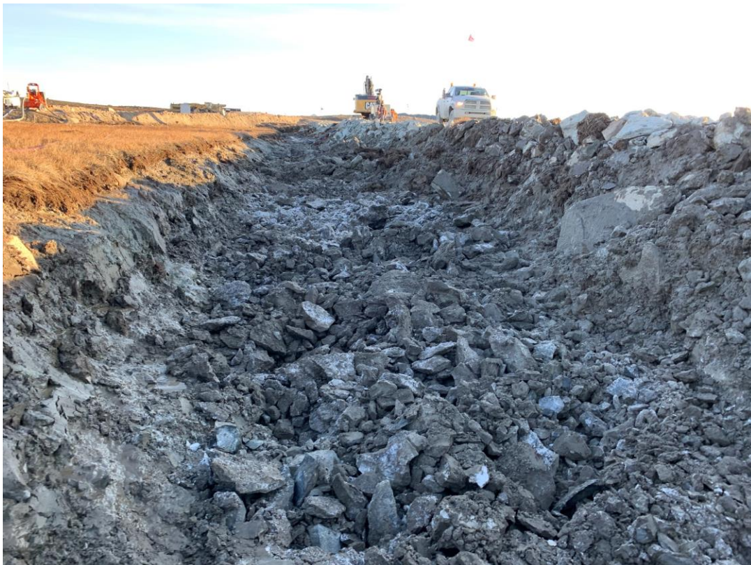
Figure 6: A layer of hammered ice-rich material between 0+029 and 0+070
