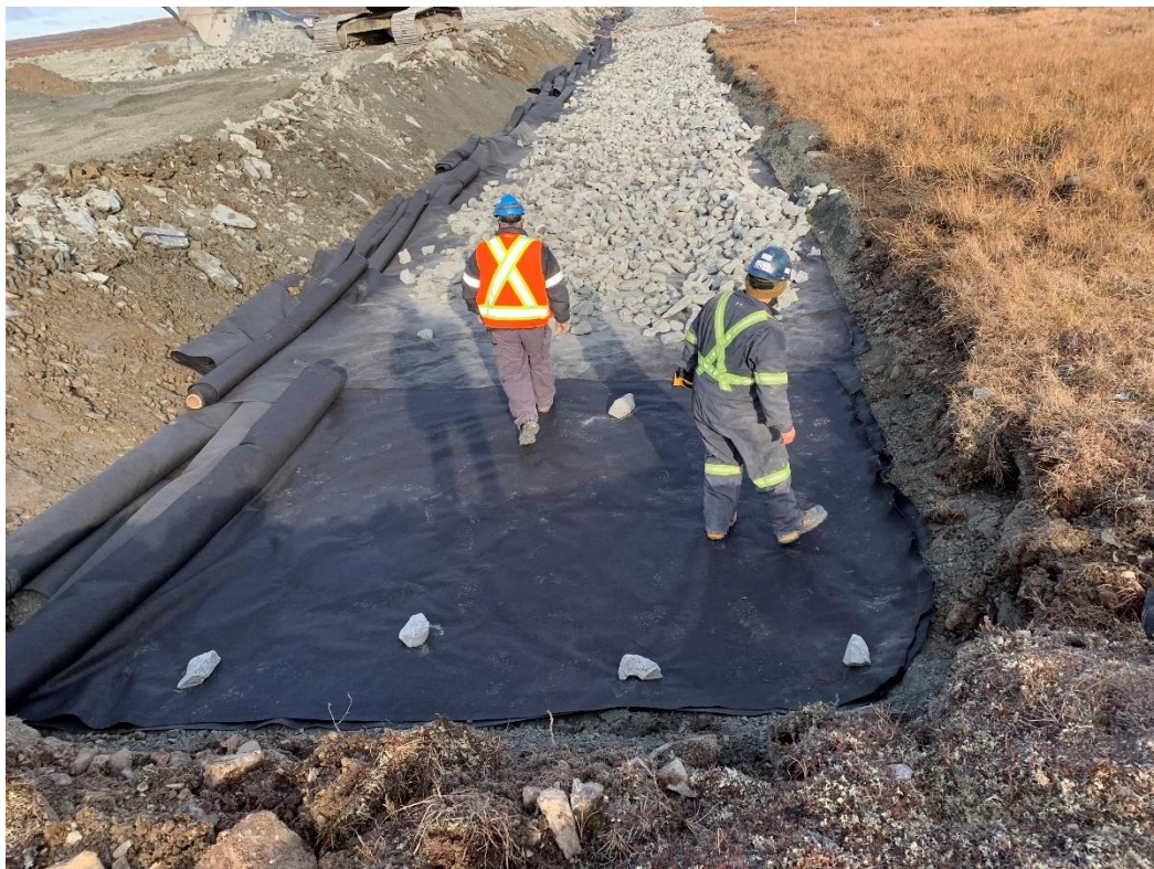
Figure 4: Geotextile placement between 0-015 and 0+032
