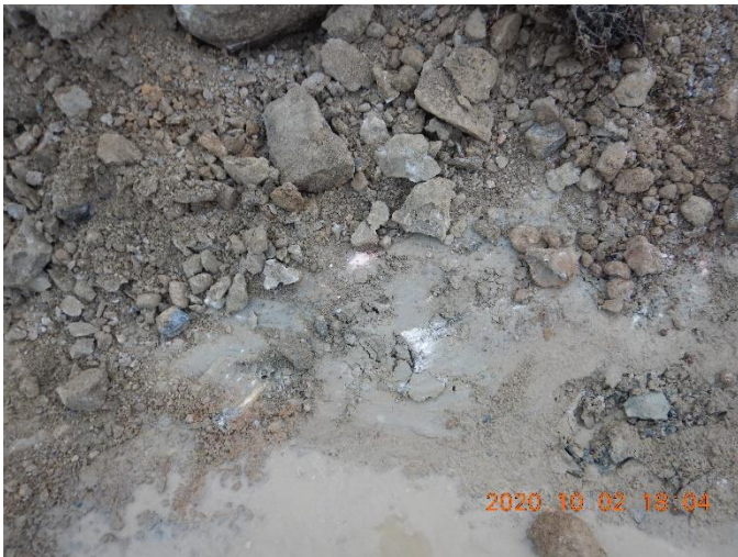
Photo 6. Looking at foundation material once ice-rich material removed (0+230 to 0+240). There was no more ice in the material at the excavated level. White spots on the photos are broken rocks, not ice.
