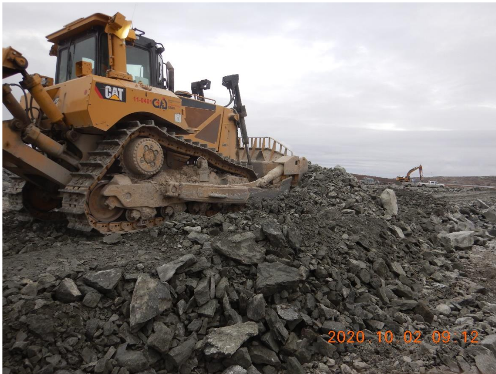
Photo 1. Rockfill placement for final lift of the access road along the west side of the channel looking south from around 0+050
