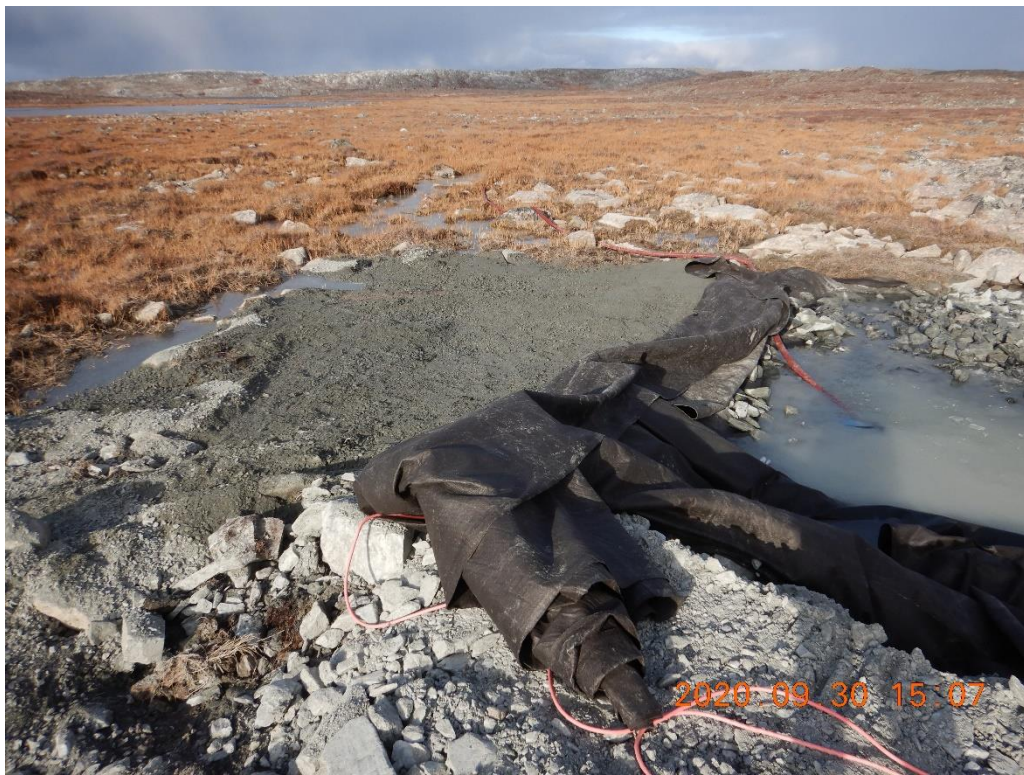
Photo 11. Downstream area of the energy dissipator. Thin layer of fine filter material placed on top of backfilled downstream sump. Top of fine filter material is at natural ground elevation.
