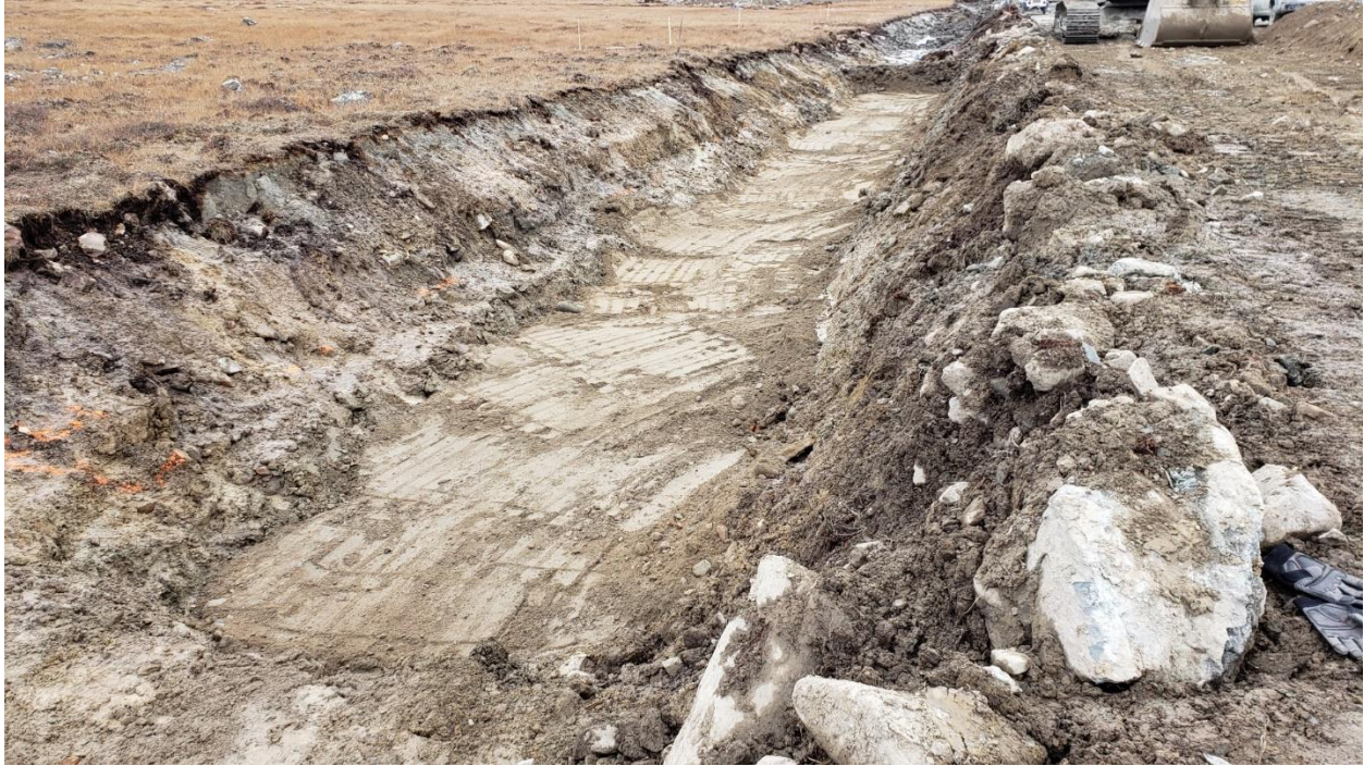
Photo 14: backfilling of the ice-rich till zone with compacted esker material, first 600mm completed. St.0+125 looking South East.
