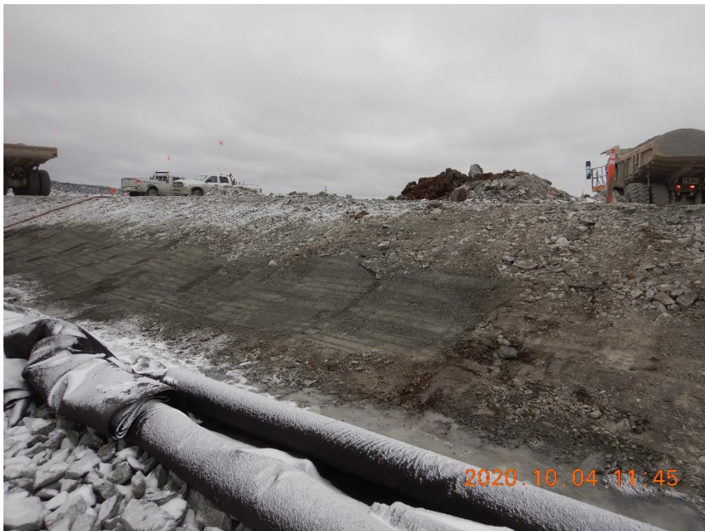
Photo 3. Foundation after corrections (boulder, soft pockets and organic matter removal), Sta 0+050 looking south
