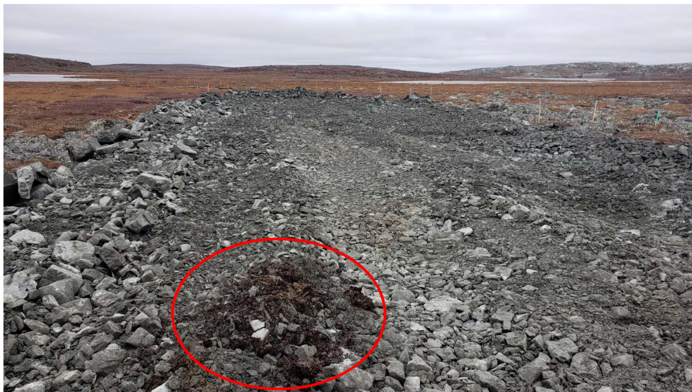
Photo 2: Station 0+200 looking North. Softer material from foundation protruding through the rockfill layer that was too thin. Before it got out of control, QA asked to retreat 50m from there and restarted with another lift 500mm over the existing one. Material shown was on the downstream end of the platform and it was left in place and covered.
