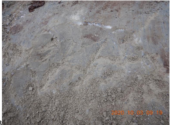
Photo 2. Foundation spot check STA 0+260, about 0.3m below grade. Visible presence of ice. Some ice lenses at mm scale and an isolated 1cm thick one.
