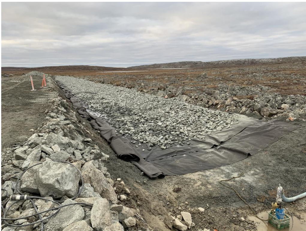
Figure 4: Preliminary riprap placement over the geotextile to hold it in place
