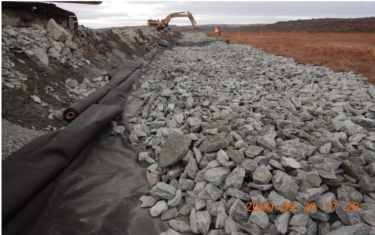
Photo 4: rip rap placement over the geotextile, St.0+035 looking North.
