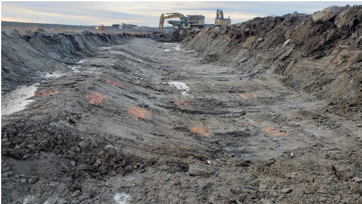
Photo 9: final excavation reached at bottom of the channel with tablet completed on the upstream slope. The downstream slope was not built to preserve excavator reach to place aggregates.
