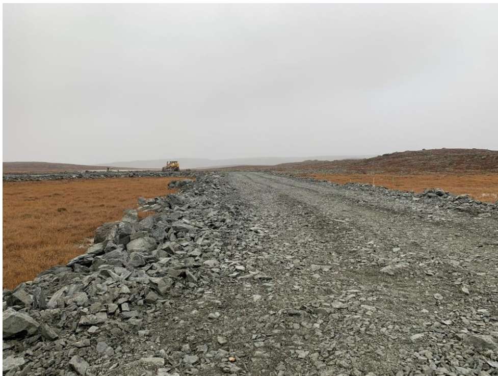
Figure 4: Visual gradation of the second lift
