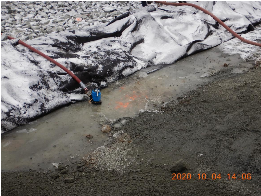
Photo 4. Water being pumped at slope toe prior to FF placement, STA 0+015 to 0+025
