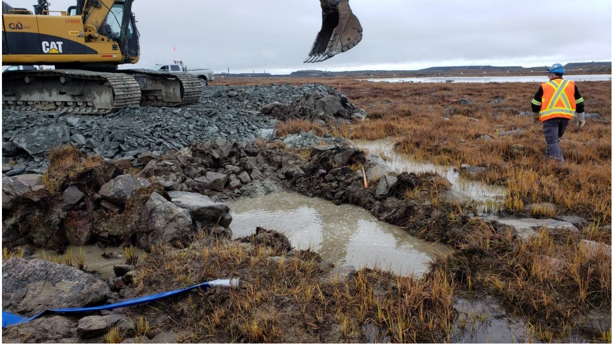
Photo 5: excavation of the temporary sump to manage water 5m North of the outlet, St.0+285 looking South.
