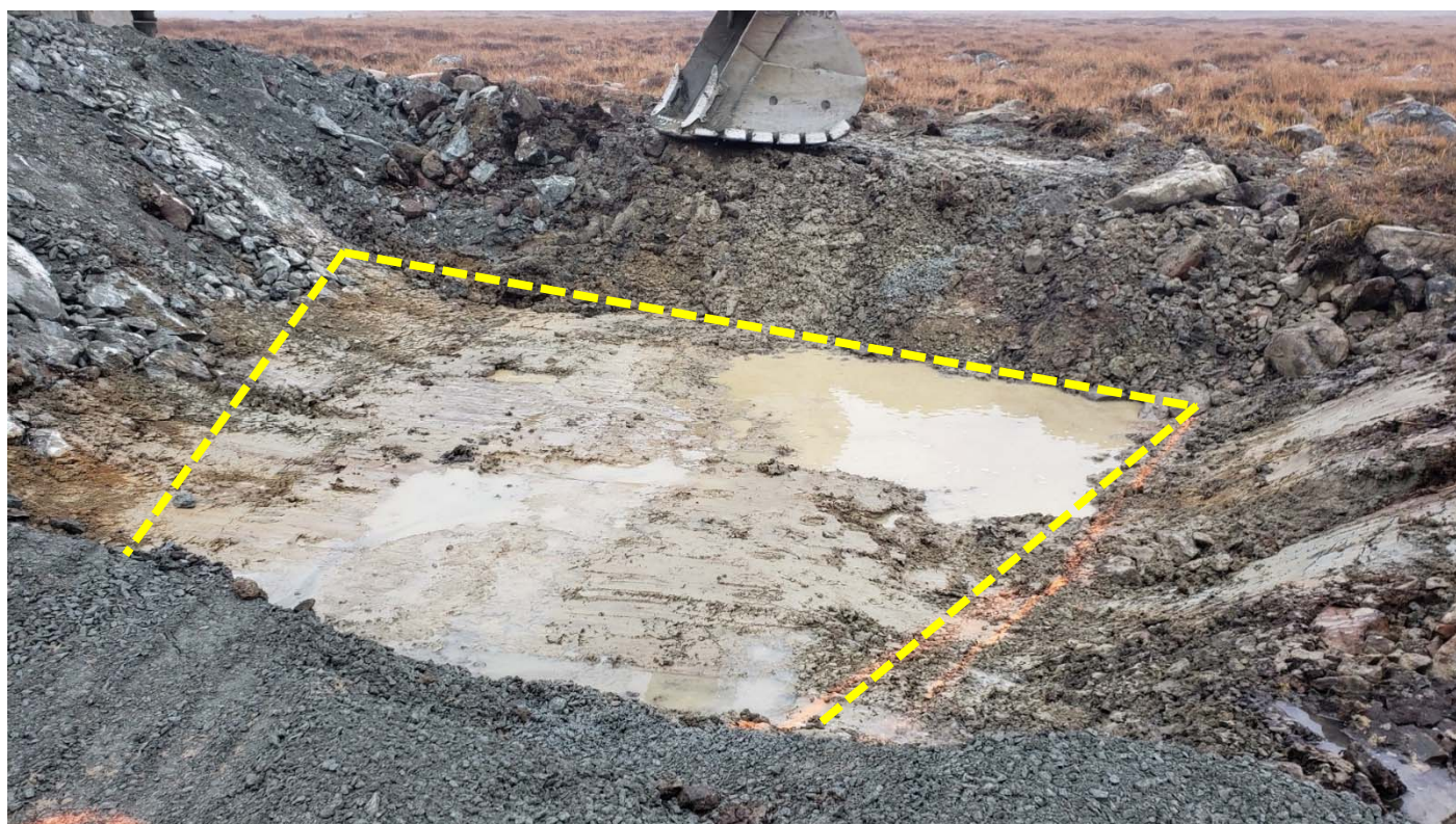
Photo 1:energy dissipator excavation. Line and grades checked by QA. St.0+281 looking North
