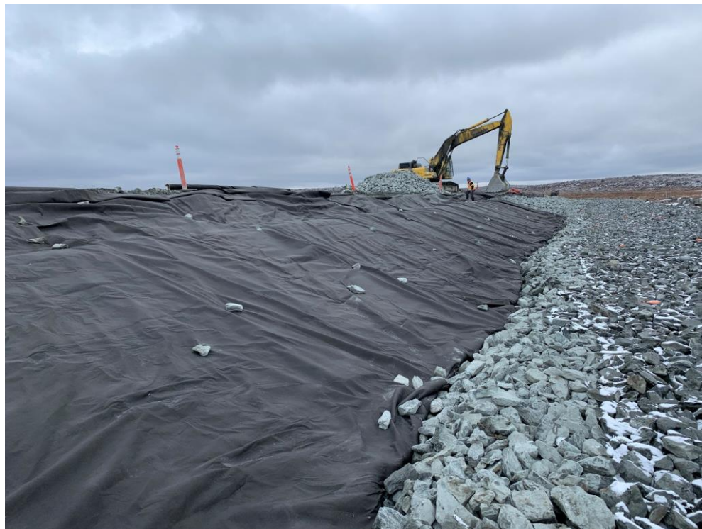
Figure 10: Geotextile placement between 0+160 and 0+284.5
