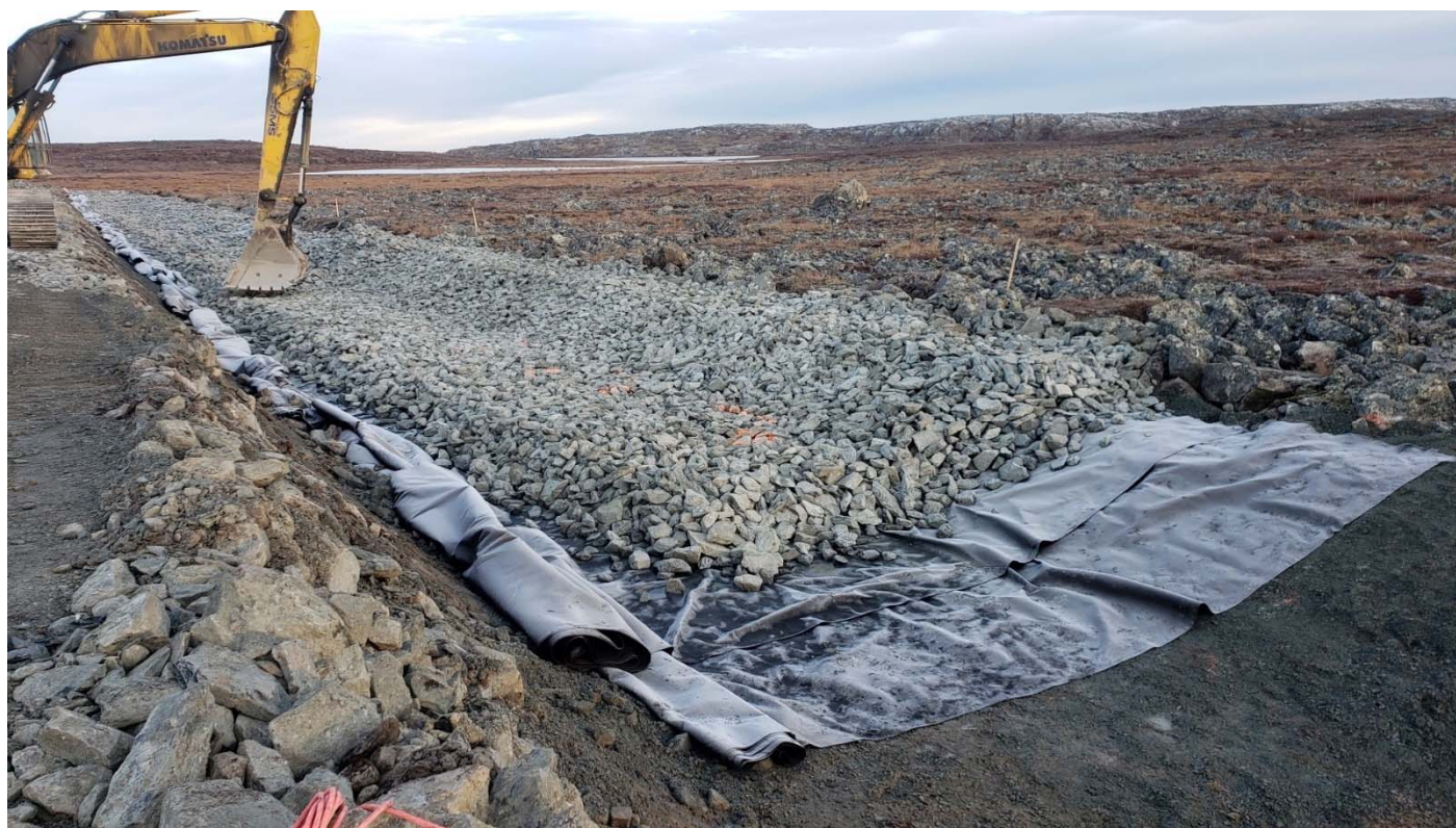
Photo 6: rip rap placement over the geotextile, final thickness adjusted and profiled, St.0+150 looking North.
