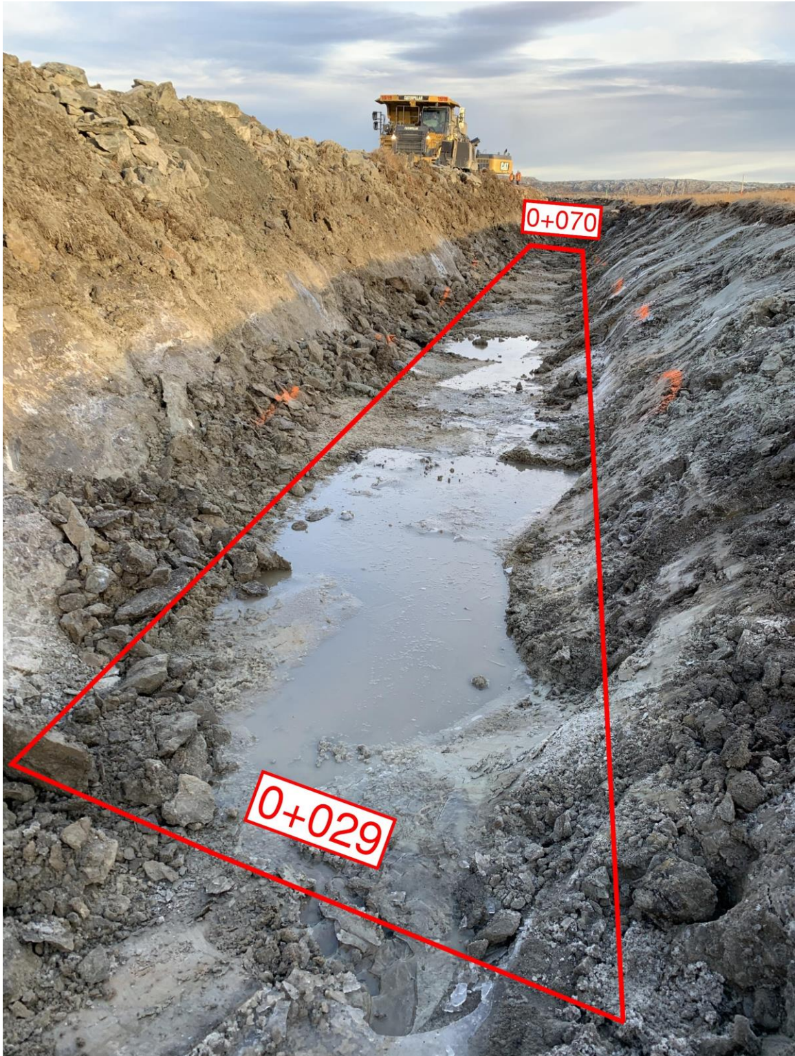
Figure 1: Ice removal approval between 0+029 and 0+070
