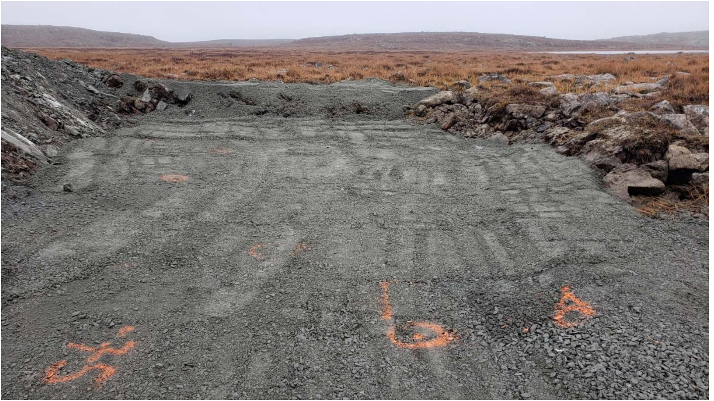
Photo 2: energy dissipator covered with Fine filter adjusted to match actual topography and surrounding boulder fields.
