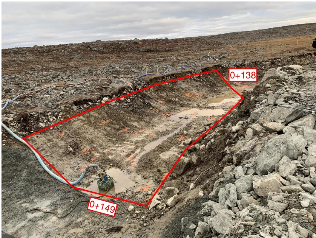
Figure 1: Foundation approval between 0+138 and 0+149
