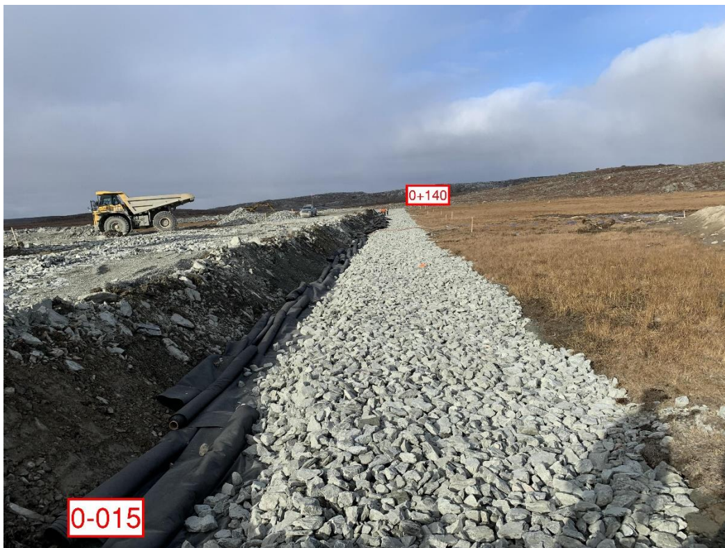
Figure 2: Riprap between 0-015 and 0+140
