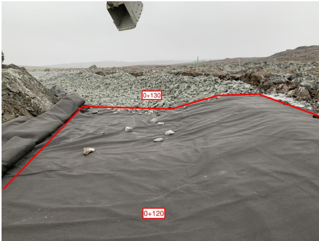
Figure 1: Geotextile between 0+120 and 0+130
