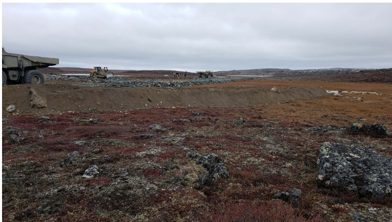
Photo 1: water management road built upstream of channel to control water contained within sector 0+000 to 0+100. Original stream was not blocked by this access.
