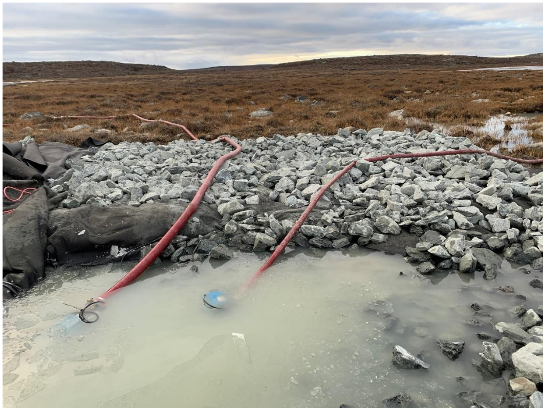
Figure 8: Pumps added at the end of the channel (0+284.5)
