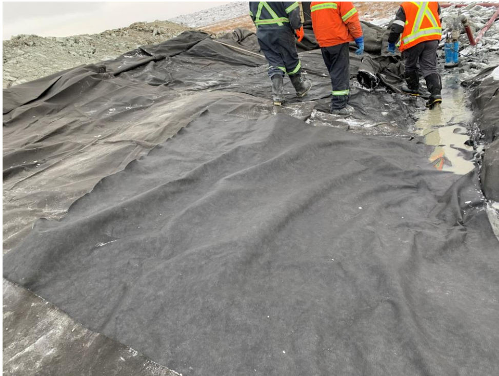
Figure 13: Holes in the geotextile are appropriately patched
