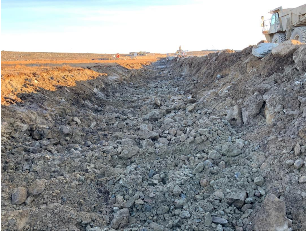
Figure 5: A layer of hammered ice-rich material between 0+090 and 0+125
