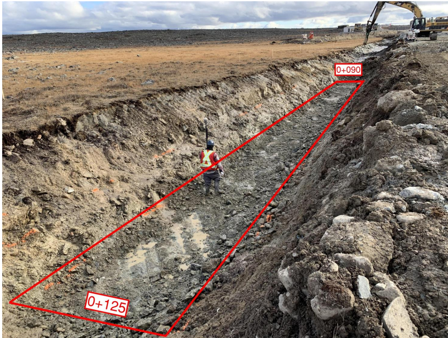
Figure 1: Ice removal approval between 0+090 and 0+125
