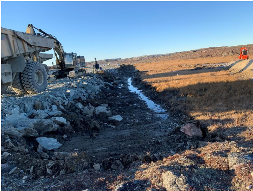
Figure 4: Preliminary excavation between 0+015 and 0+024
