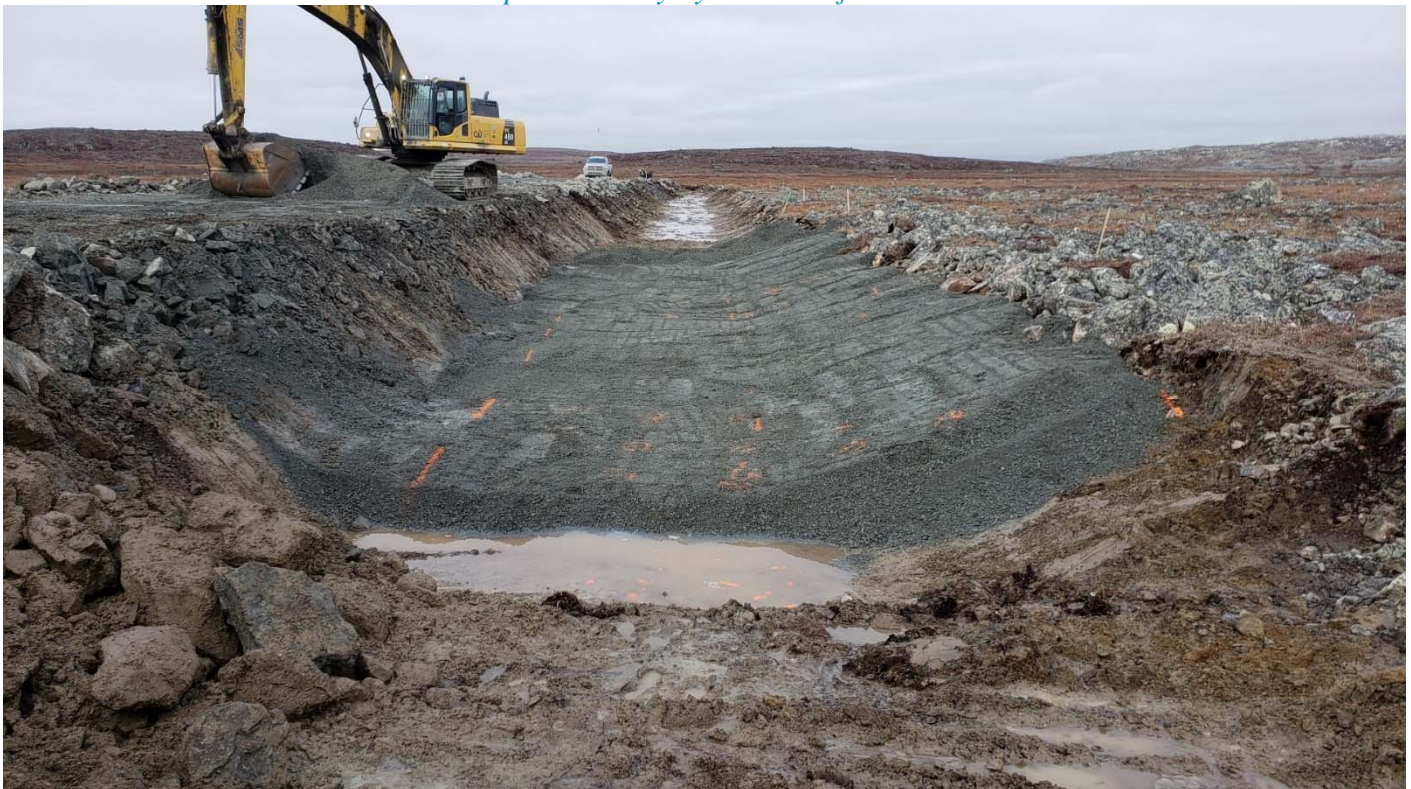
Photo 3: Fine filter almost to final grade between Stations 0+147 and 0+181.
