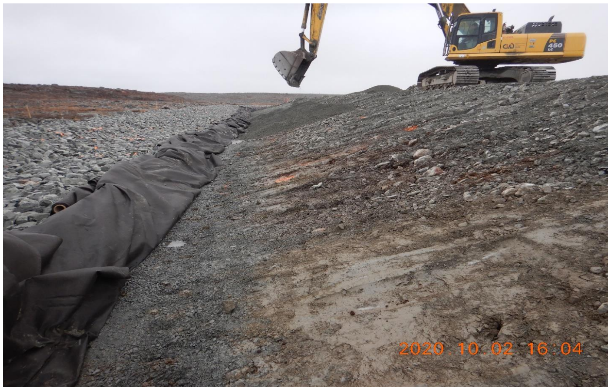
Photo 29: fine filter placement in downstream slope, St. 0+170 looking South-East.
