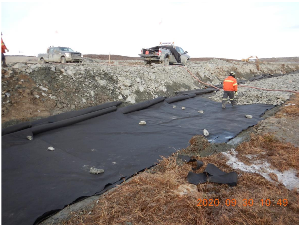
Photo 5. Geotextile installation on top of FF layer. Two layers of Tencate Mirafi 1100N with proper overlaps. Looking north from 0+020.
