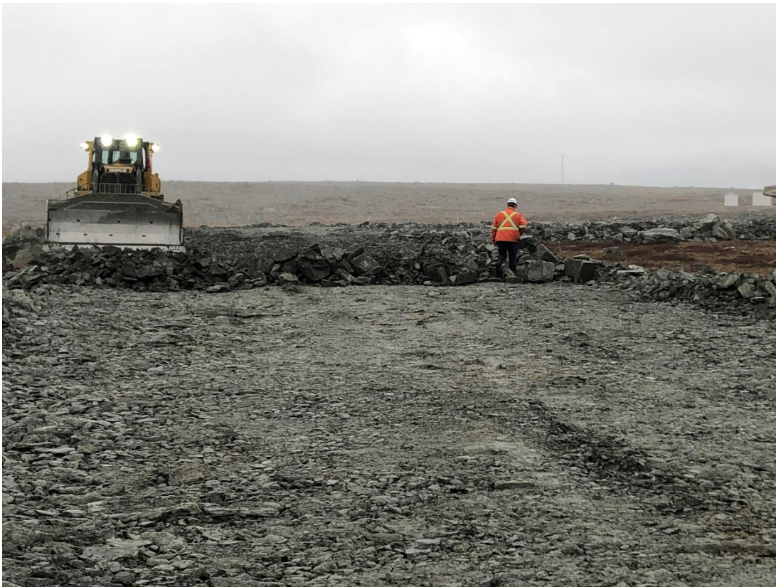
Photo 4: construction of the second lift of the downstream berm construction with ultramafic rockfill, St. 0+180 looking South.
