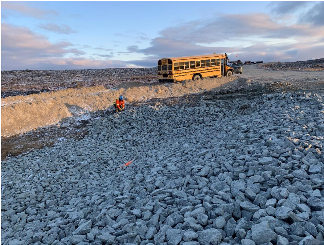
Figure 3: Final riprap placement at the entrance of the channel (0-015)
