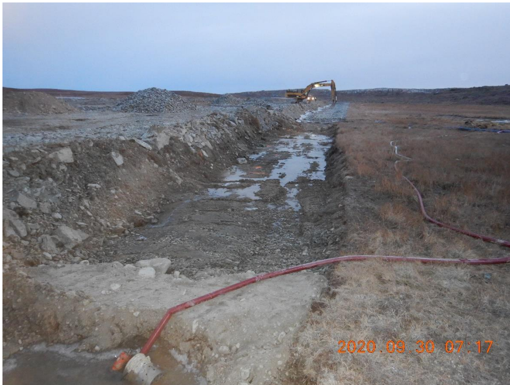
Photo 1. Bottom of the exvaction from -0+015 to 0+029 before final clean up. Looking north. Water in the excavation is coming from tundra runoff and has been removed, along with superficial thawed material, prior to approval.
