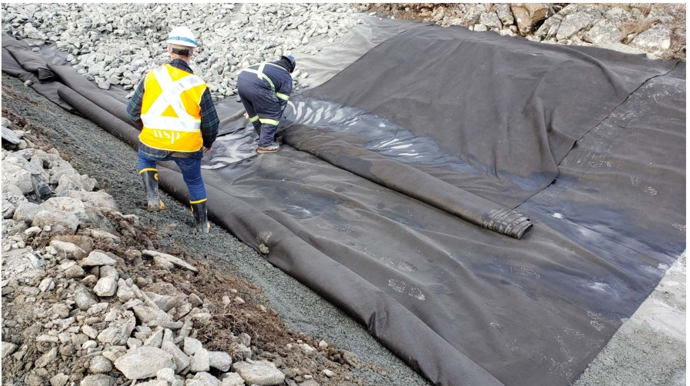
Photo 5: geotextile placement of 2 layers of Novatex V. Bottom layer overlap of 600mm respected, top layer overlapping the first layer by half a roll.
