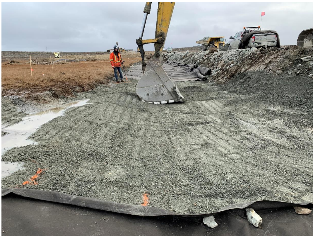
Figure 6: Fine filter approval between 0+070 and 0+090
