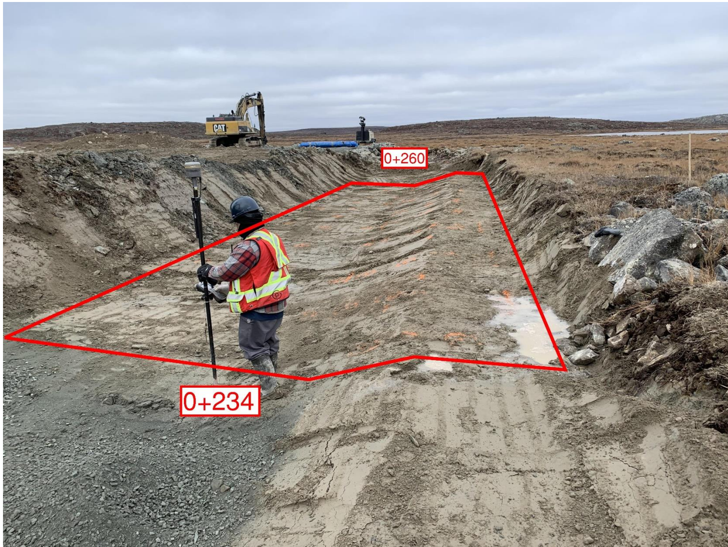
Figure 1: Foundation approval between 0+234 and 0+260
