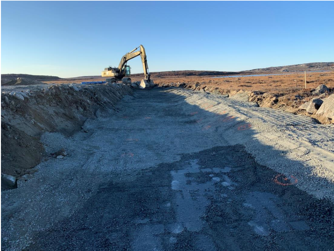
Figure 7: Fine filter fill between 0+234 and 0+281 (ongoing)
