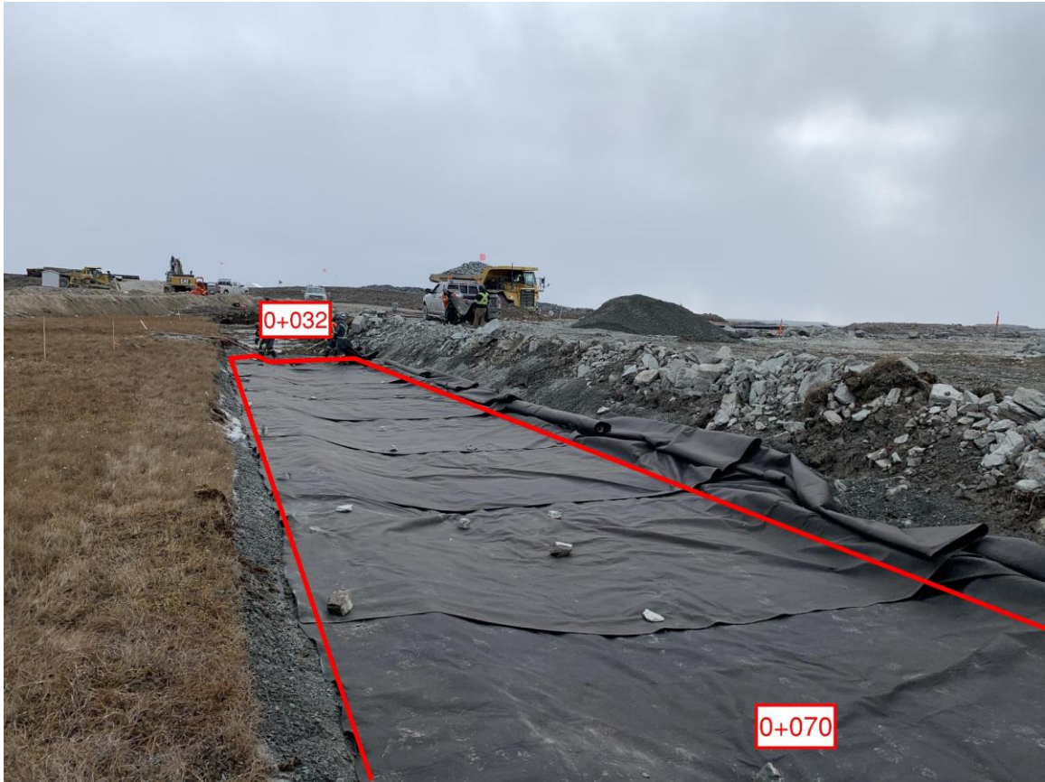
Figure 3: Geotextile between 0+032 and 0+070
