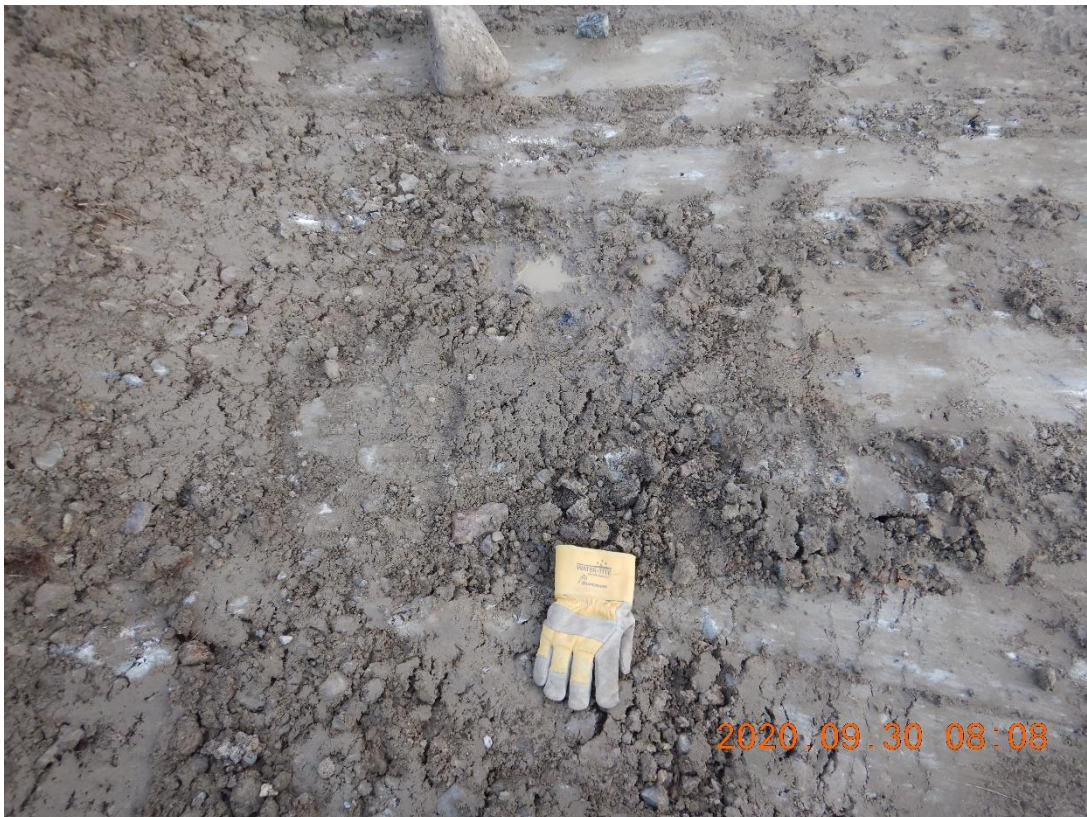
Photo 3. Close up view on foundation material in 0+000 to 0+029 area. Ice poor material, mix of sand, gravel and finer material. Superficial thawed soil and water removed prior to backfilling FF. Sample EX-15 taken in that area.
