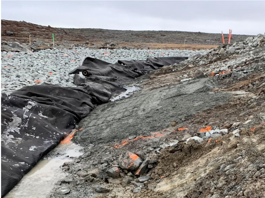
Figure 5: Excavated soft spot filled with well compacted fine filter
