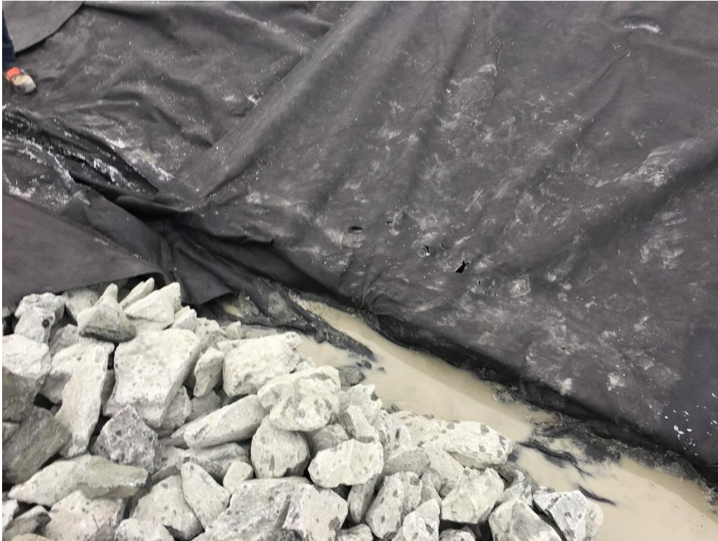
Photo 8. Damaged geotextile. Rip rap material has been manually removed at the toe to allow proper overlap of the patch to be installed
