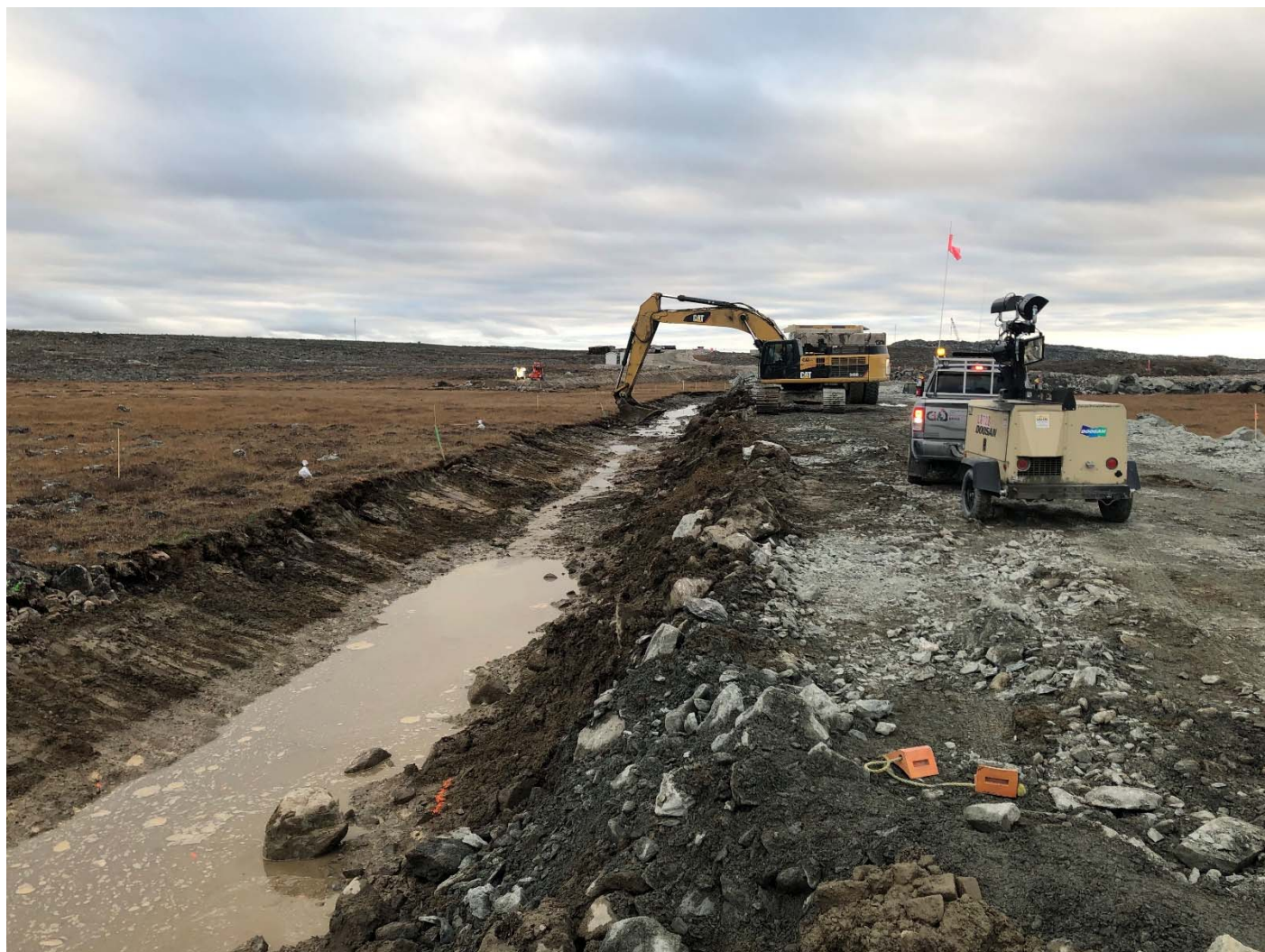
Photo 4: first pass of excavation for the South sector. St.0+139 looking towards 0+035. Lots of water draining from the tundra is managed through series of sumps.
