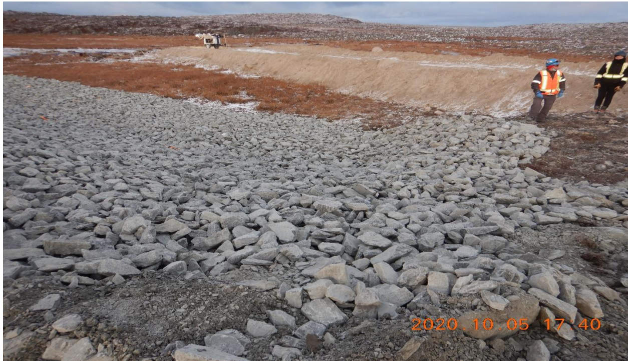
Photo 34: Channel inlet completed with rip rap placement.
