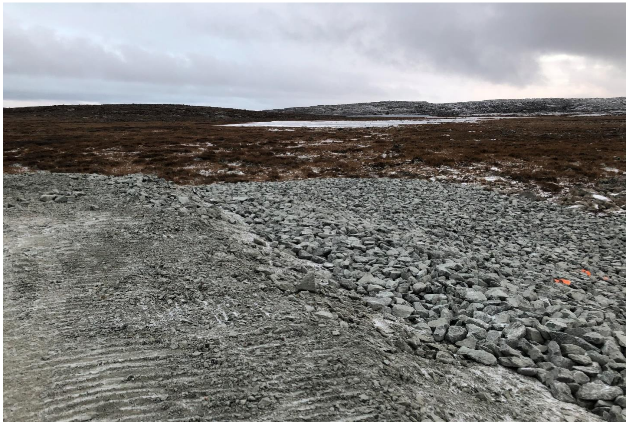
Photo 35: channel outlet completed with geotextile and rip rap.
