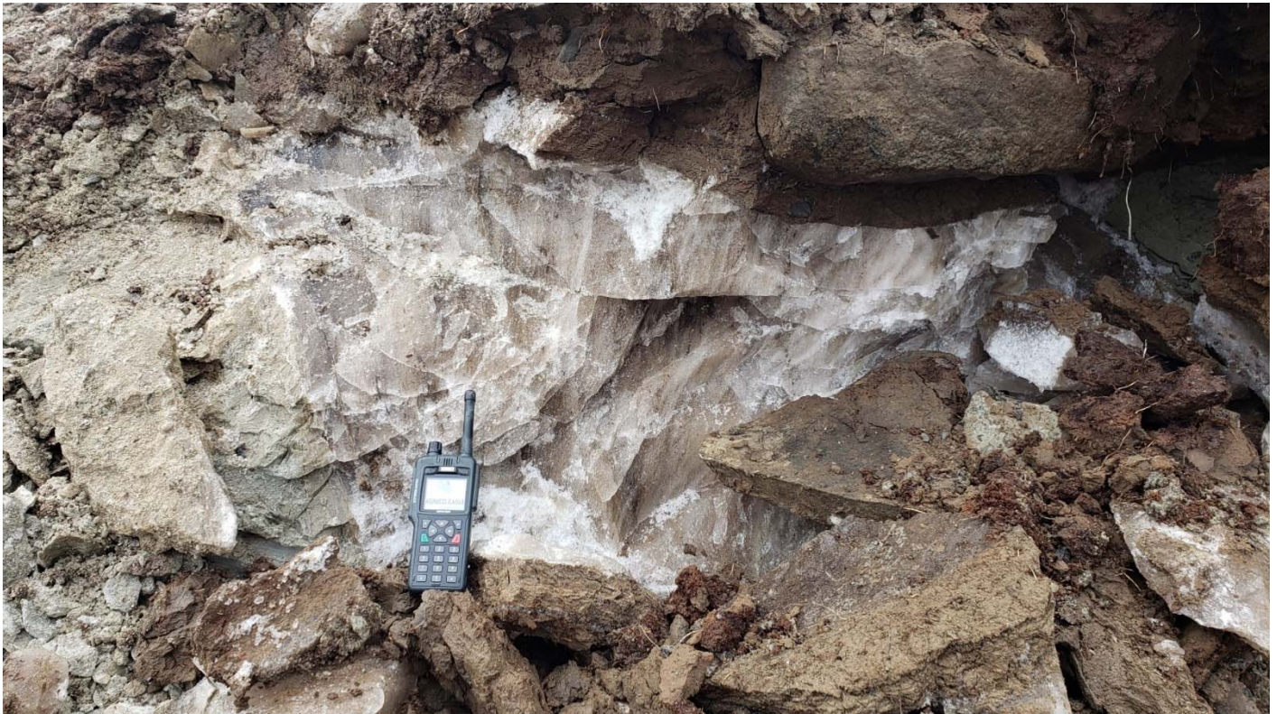
Photo 5: partial view of the ice lens found under the rockfill at the base of the slope St. 0+243, original size 1.2m long x 0.9m deep x 0.6 m wide. Lens was entirely removed and replaced with rockfill.
