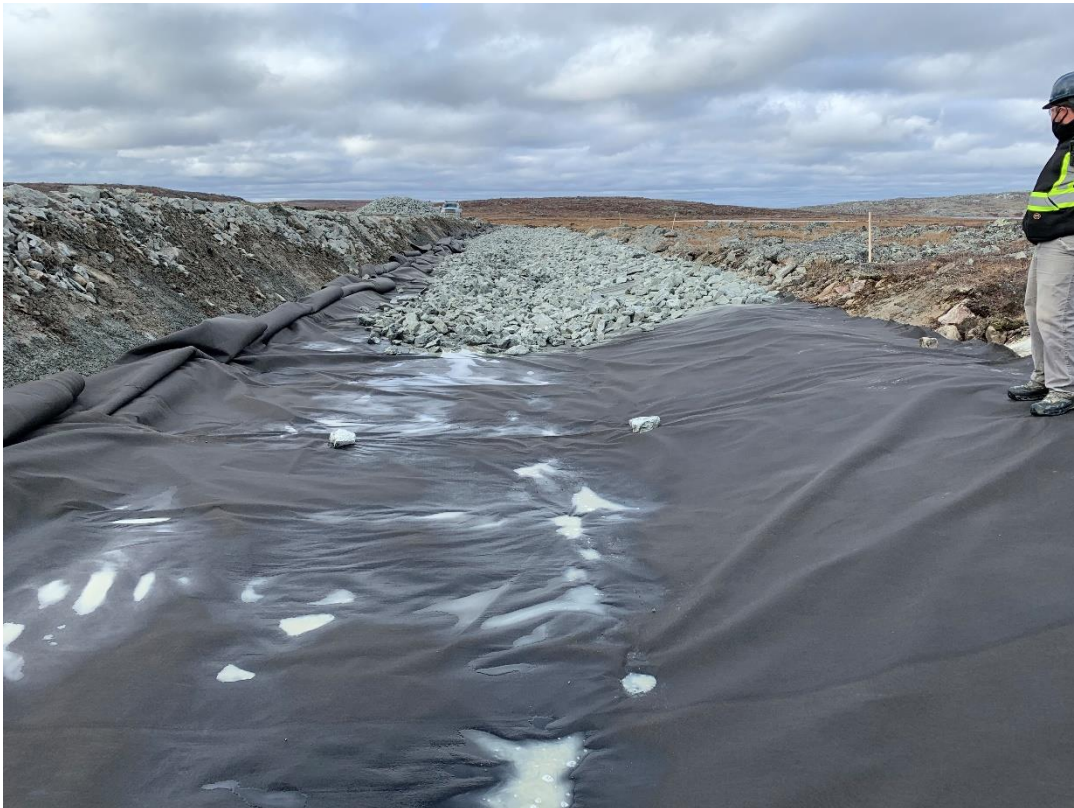
Figure 2: Geotextile placement between 0+284.5 and 0+152
