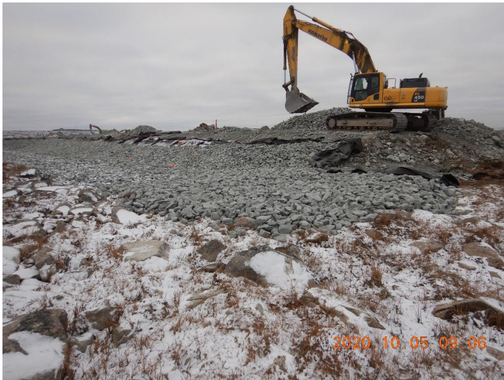
Photo 1. Preparing surface to lay geotextile on. Exceeding mterial removed to remain at natural ground elevation. There is a natural slope from west to east. Photo is looking at west side of the channel downstream end
