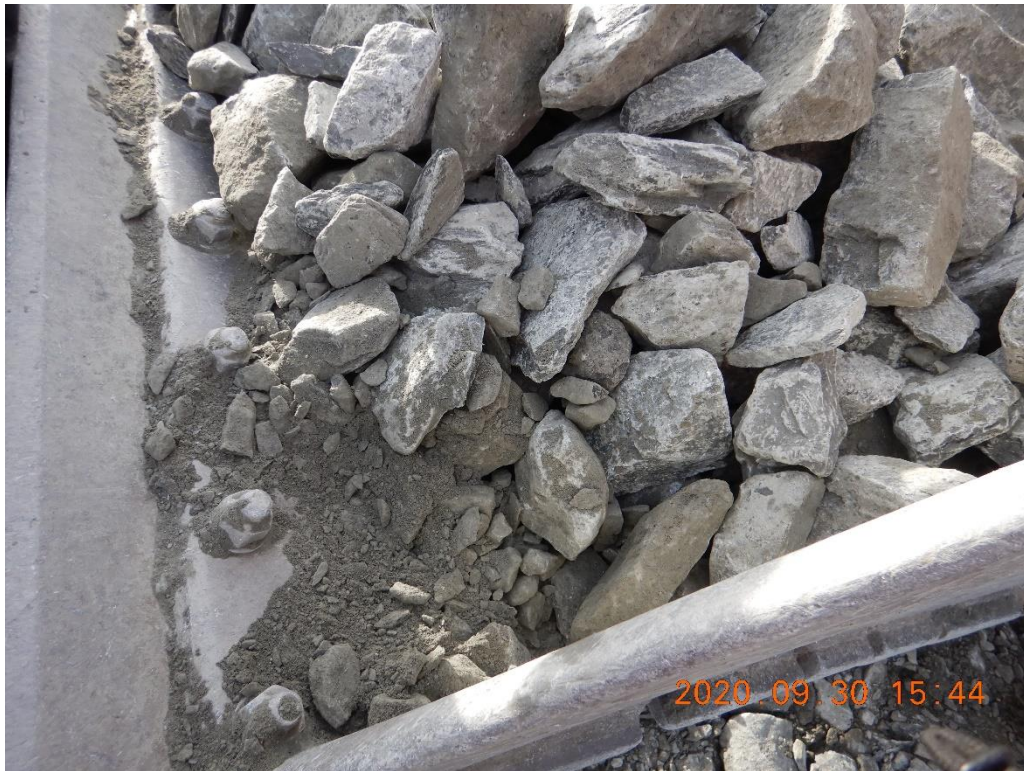
Photo 10. Non-compliant rip rap material containing fines and gravel <100mm. Excavator were told not to place any material of that kind. Manual cleaning will be required at some location along the channel where finer material was observed within the rip rap. Refer to comment section above.
