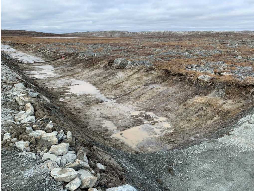
Figure 3: Foundation approval between 0+181 and 0+205
