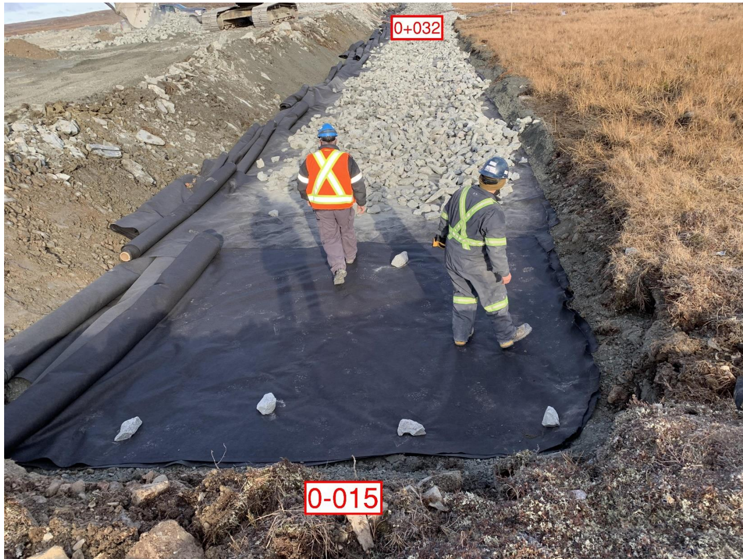
Figure 1: Final geotextile between 0-015 and 0+032
