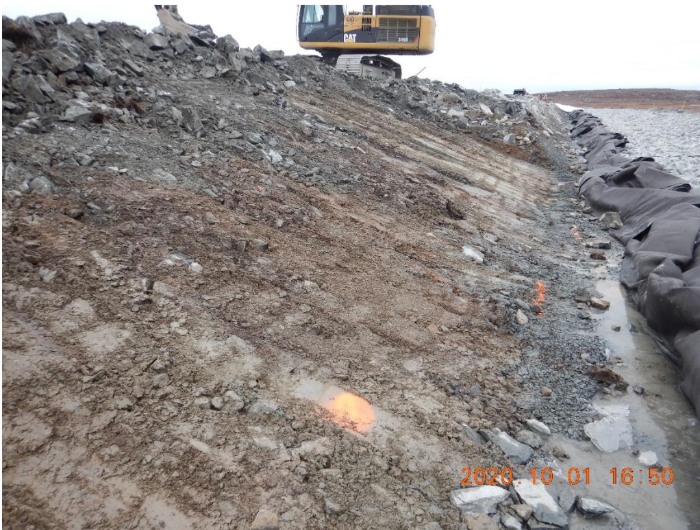
Photo 3. Excavation of the side of the road to prepare west slope of the channel, looking north STA 0+160. Some water ponding on top of the invert fine filter layer. Rolls of remaining geotextile moved on the rip rap to leave as much room as possible for the excavator to work the slope.
