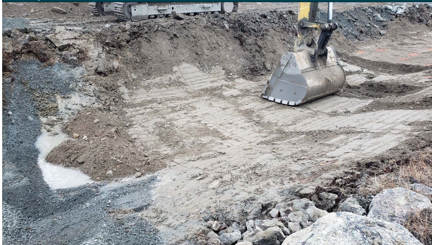
Photo 1: 2 nd lift of esker fine material in replacement of ice-rich till St. 0+235 looking North. Material placed in 600mm lifts compacted with the bucket of the excavator.
