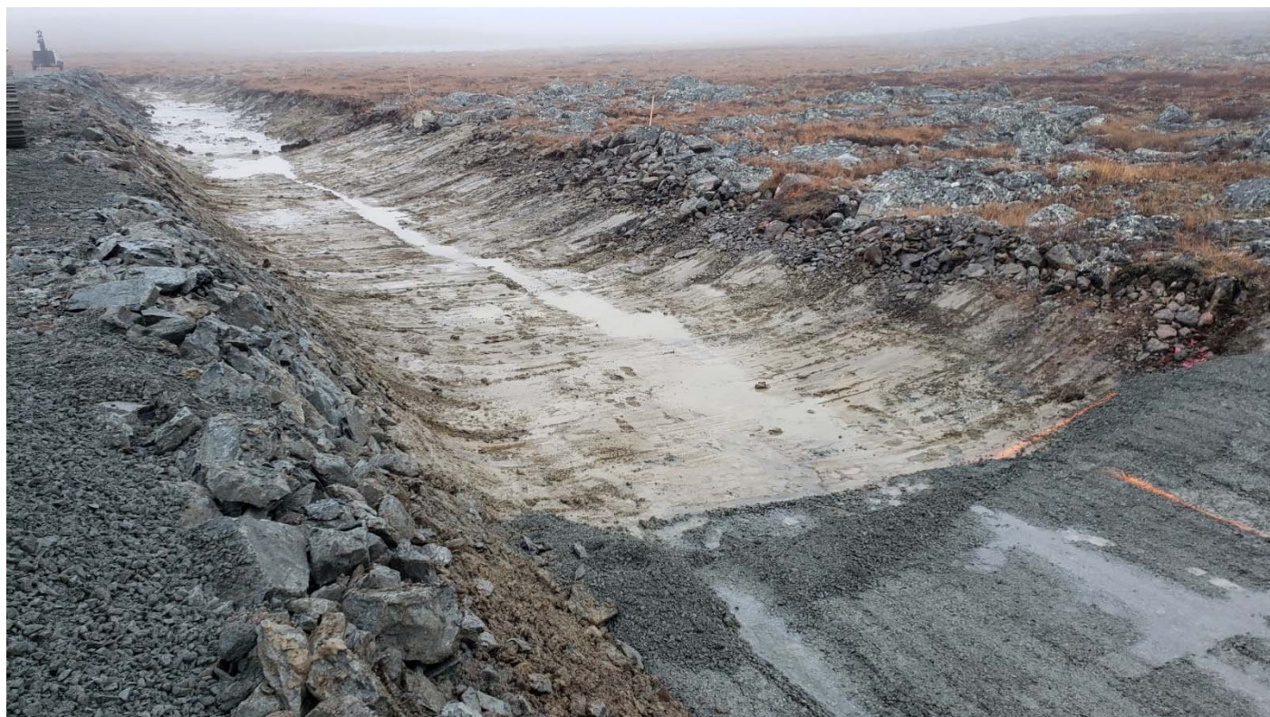
Photo 1: Ice rich till section between 0+235 and 0+260, after clean up and before hammering. Unsuitable foundation material visible ice greater than 10% of the surface, presence of ice lenses.
