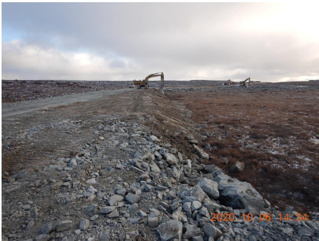
Figure 3. Sloping west side of the access road, reusing leftover material including esker. Sta 0+250 looking South
