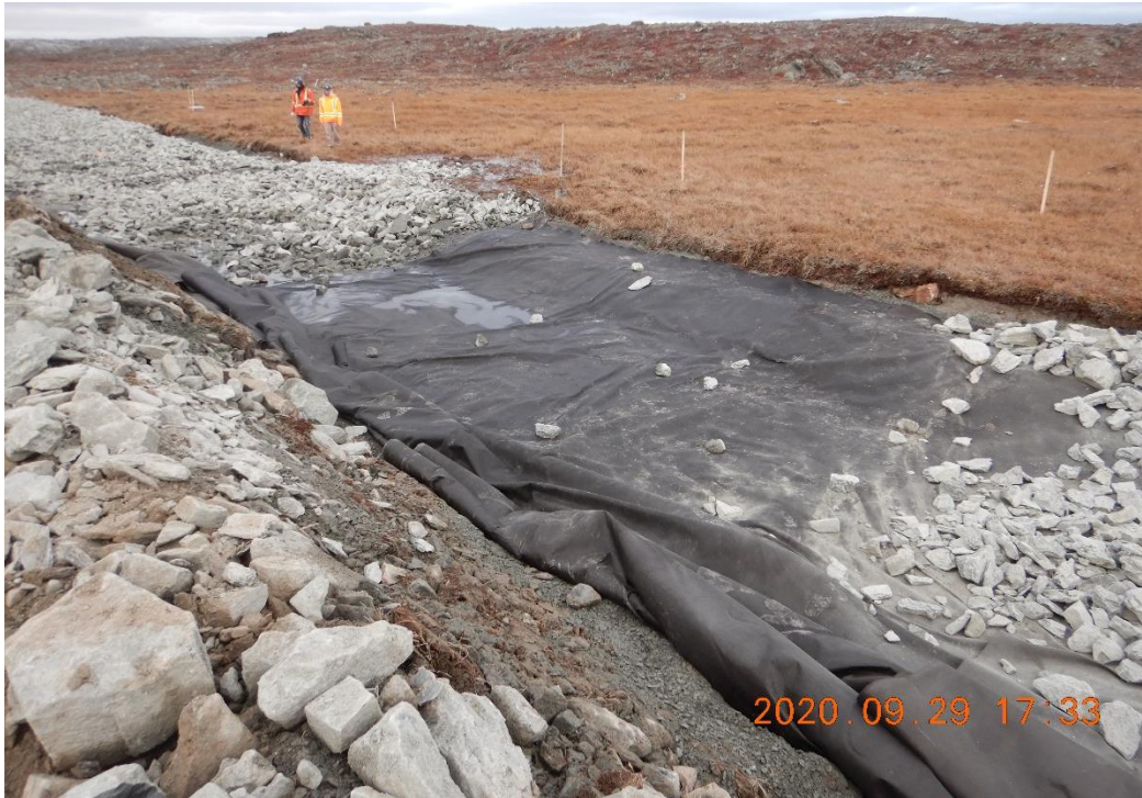
Photo 6: Rip rap placement on geotextile. Sta 0+070 looking north west. Water ingress (tundra runoff) at around 0+100 is visible on the photo. Water is properly flowing within the rip rap material, over the geotextile.
