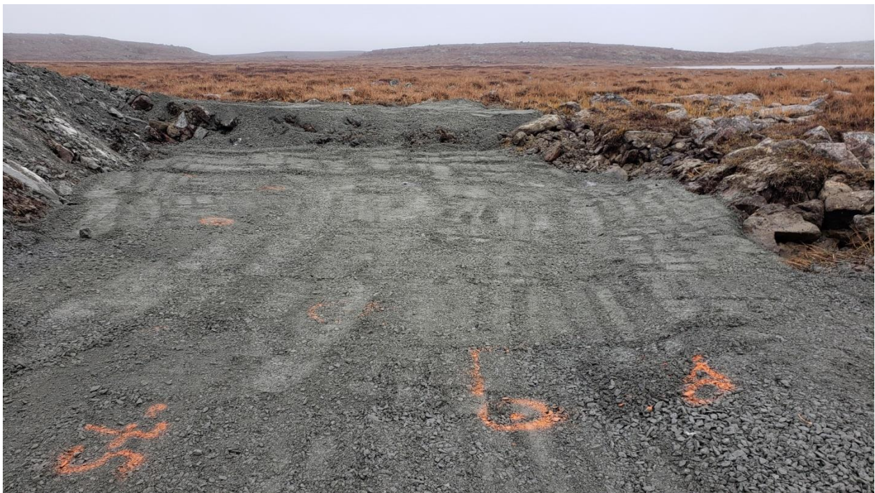
Photo 21: energy dissipator at the channel outlet covered with fine filter, St.0+275 looking North-West.
