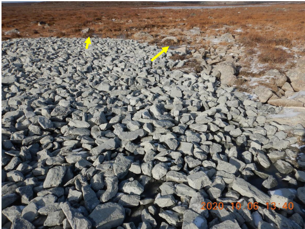
Figure 7. Downstream end of the channel. Water flowing through the rip rap layer and seeping out in the tundra at different locations (yellow arrows). Looking North.
