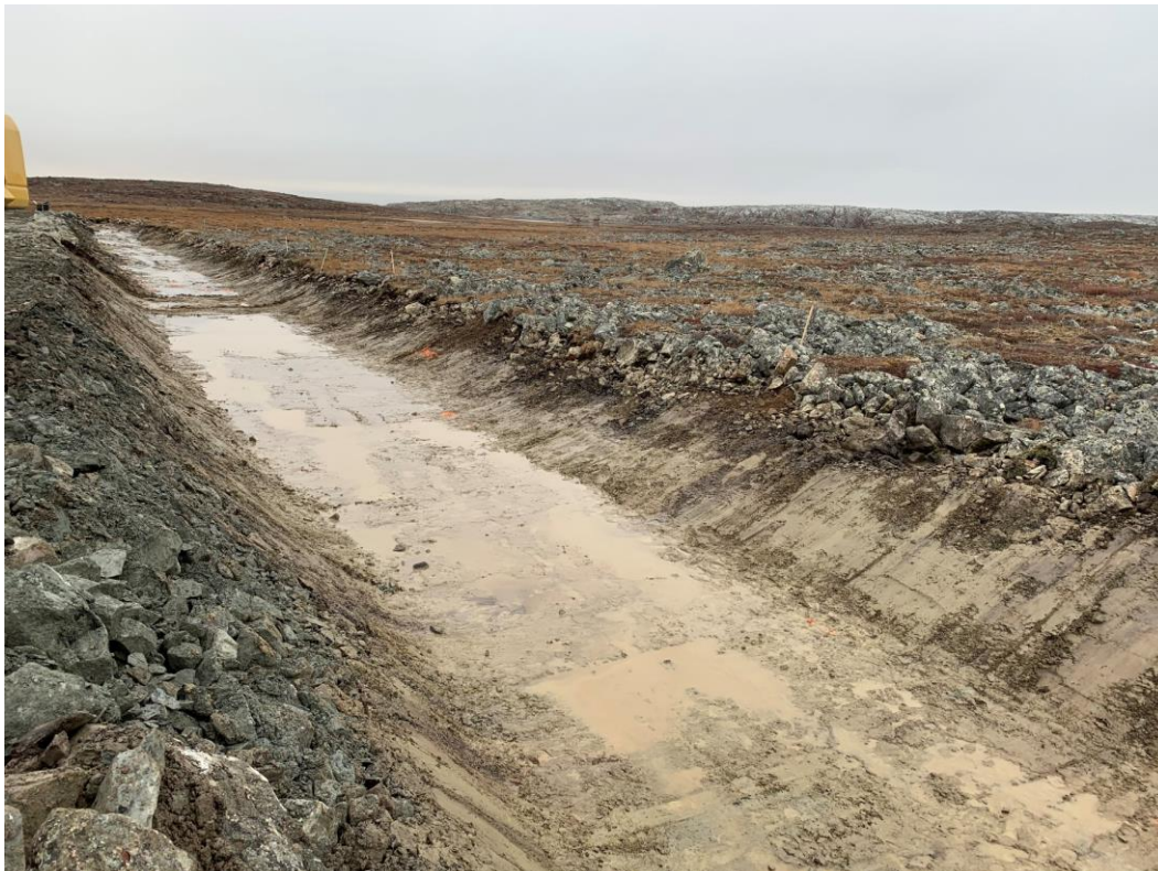
Figure 2: Foundation approval between 0+149 and 0+181
