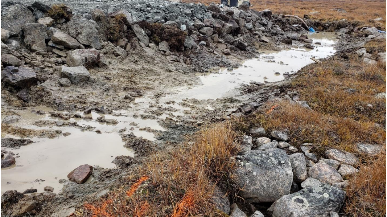
Photo 6: First step of the excavation where 500mm of material is dug to promote drainage of the overburden, St.0+270 looking North-east.
