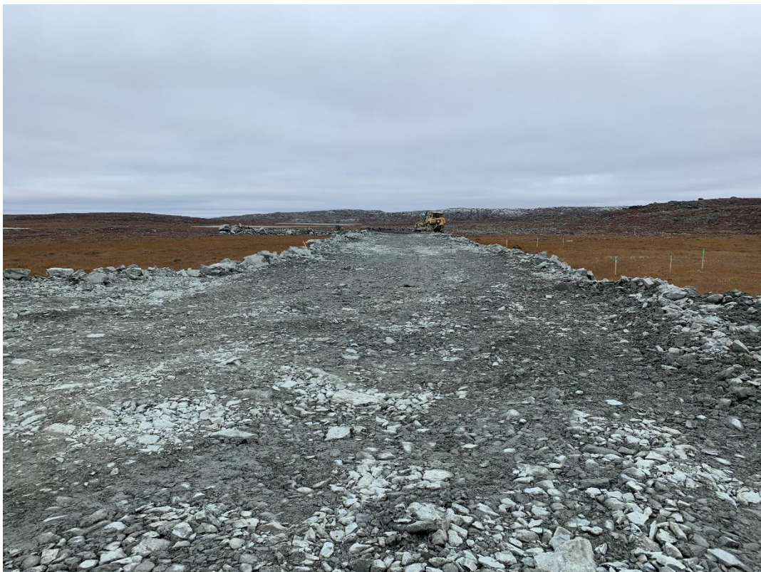
Figure 4: The first part of the access road is well compacted and stable (0+024 to 0+111)
