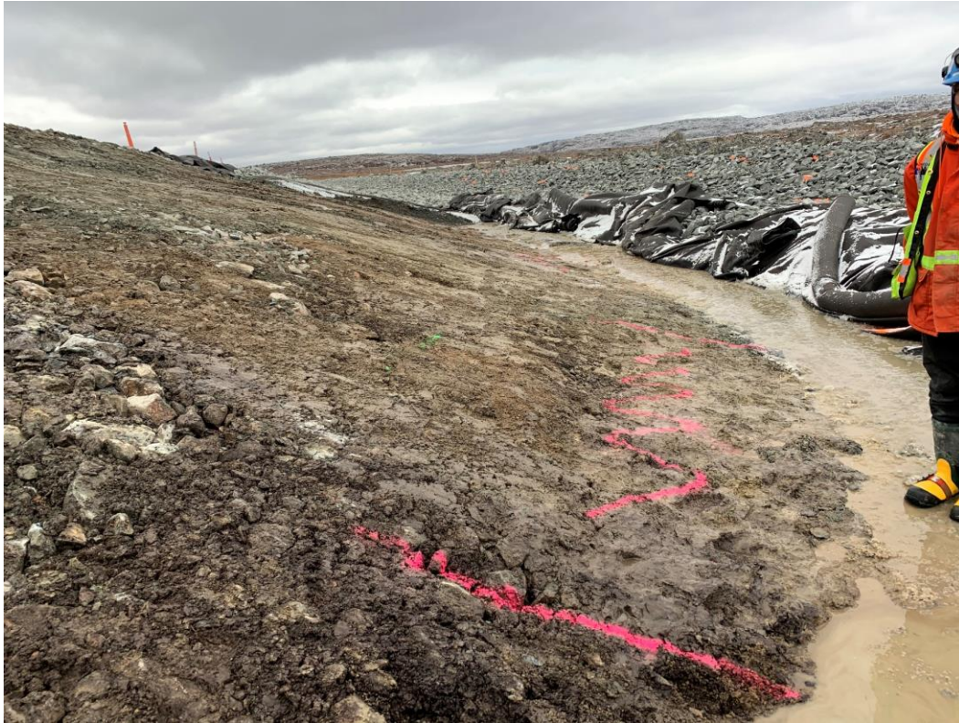
Figure 3: Foundation approval between 0+140 and 0+155
