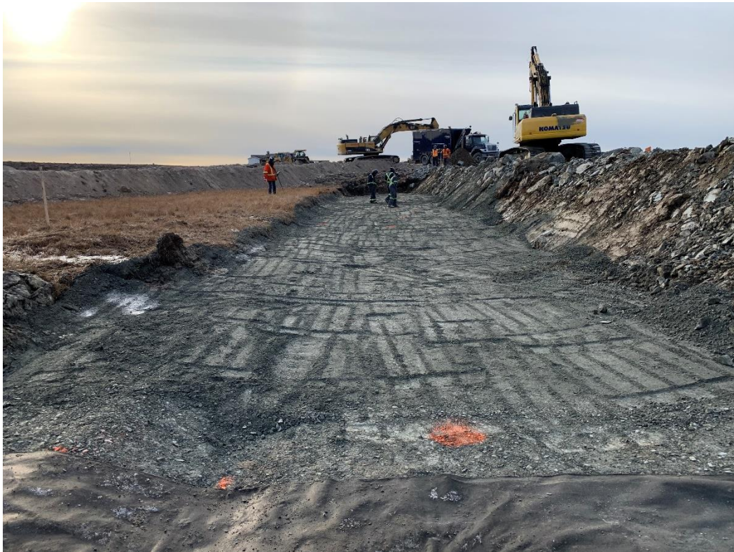
Figure 3: Fine filter fill approval between 0-015 and 0+029
