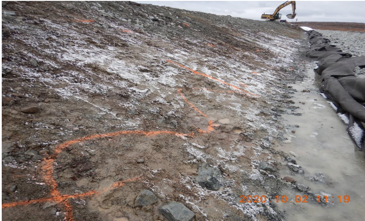
Photo 28: approved surface of the downstream berm sloped ready for fine filter placement, St.0+200 looking North-West.
