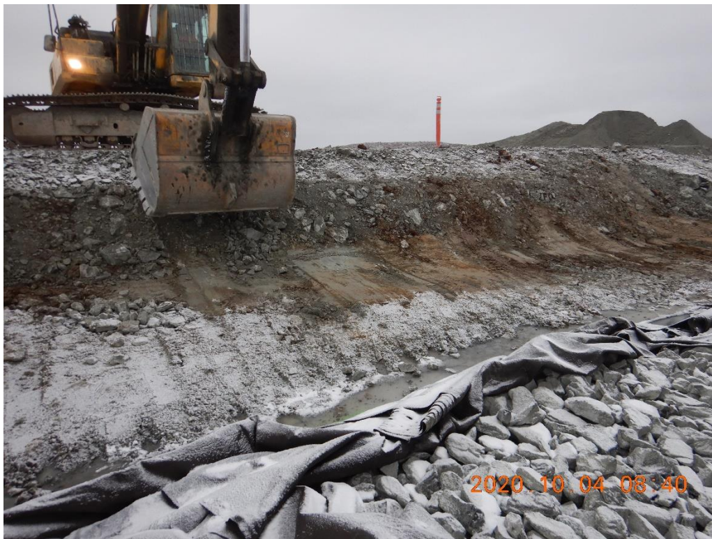
Photo 1. West slope excavation on going. Organic matter and boulders being removed to expose adequate foundation. Looking west between 0+050 to 0+090.
