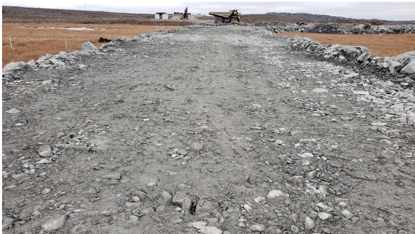
Photo 1: Close view of downstream platform, 0+075 looking South, compaction of the entire width achieved by haul trucks.
