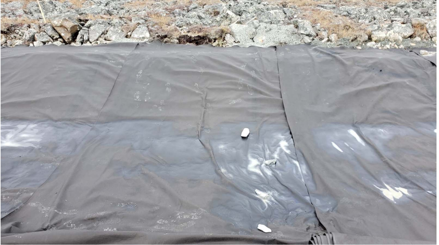
Photo 6: geotextile placement, example of a completed section St.0+150. Flow of the channel towards left of photo.
