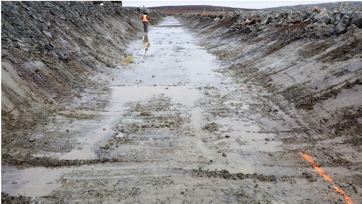
Photo 8: Final excavation at bottom of channel before the upstream tablet was completed, St.0+140 looking North-West.
