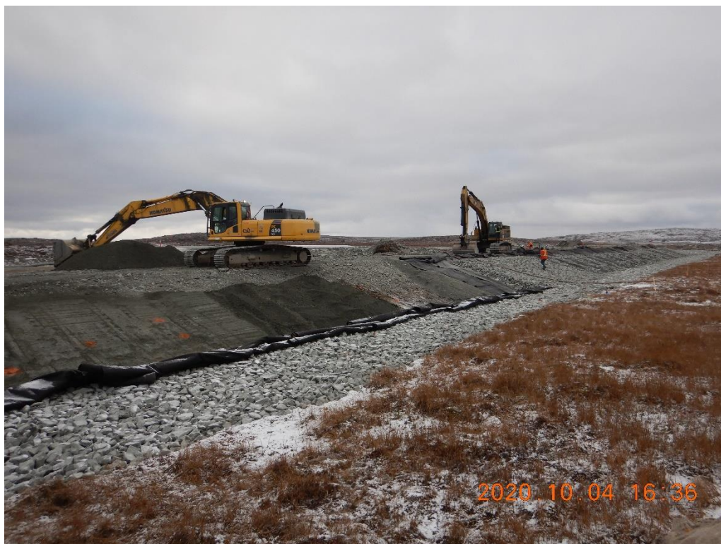
Photo 10. Upstream end of the channel. FF and Rip Rap placement. Sta -0+015 looking north
