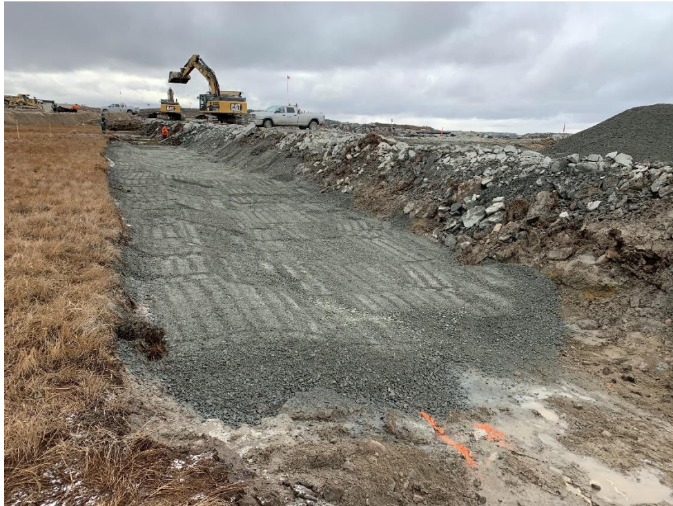
Figure 7: Fine filter approval between 0+029 and 0+070
