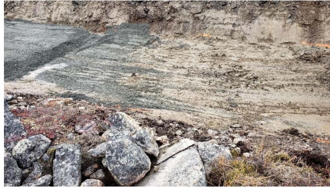
Photo 2: for the section where water keeps coming at the bottom of the excavation, mud and water is mixed with FF then material is pushed away by the side of the excavator bucket.
