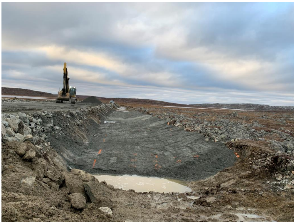
Figure 4: Fine filter fill between 0+149 and 0+205
