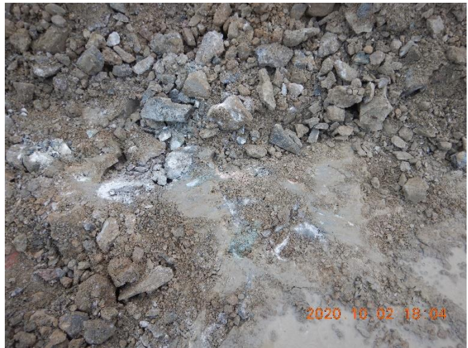
Photo 6. Looking at foundation material once ice-rich material removed (0+230 to 0+240). There was no more ice in the material at the excavated level. White spots on the photos are broken rocks, not ice.
