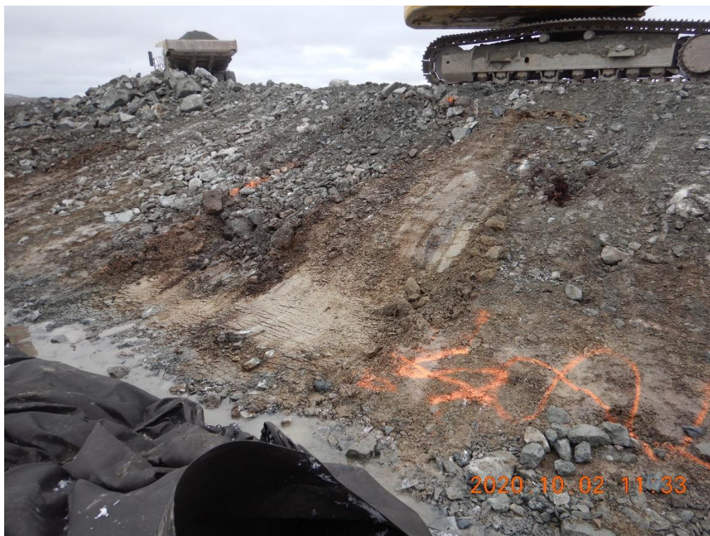
Photo 4. Ongoing process of removal of soft oversaturated material at the toe of the slope. About 0.1 to 0.3m removed in the center of the photo. Exposed material is much dryer and competent. Marked material on the right hand side remains to be excavated.
