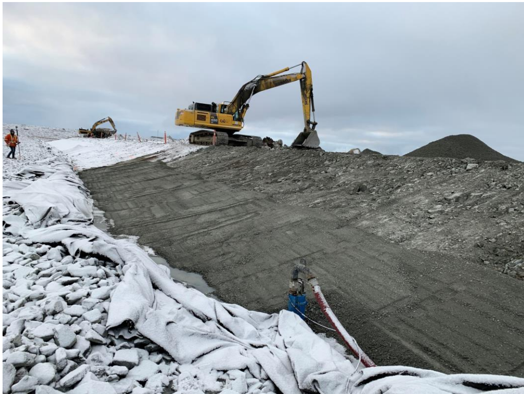
Figure 8: Fine filter approval between 0+260 and 0+284.5
