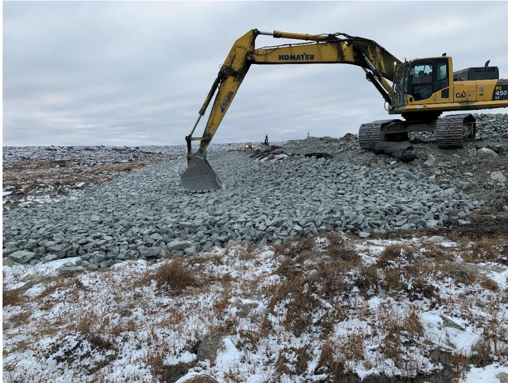
Figure 1: Final riprap placement at the energy dissipator (0+281 to 0+290)
