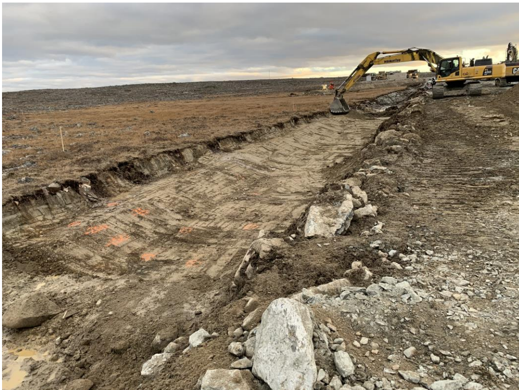
Figure 6: Esker placement between 0+090 and 0+125
