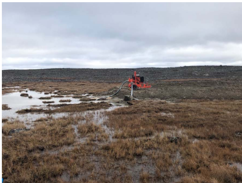
Photo 1: water management upstream of channel to control water contained within sector 0+000 to 0+100.
