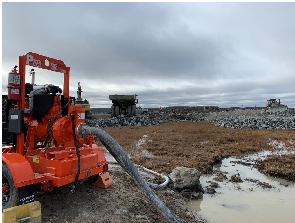
Figure 2: Pumping station for the upstream part of the channel
