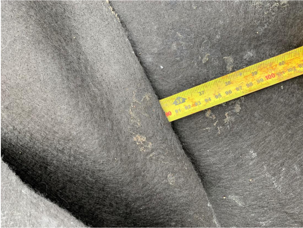
Figure 1: Overlaps are conforming to technical requirements
