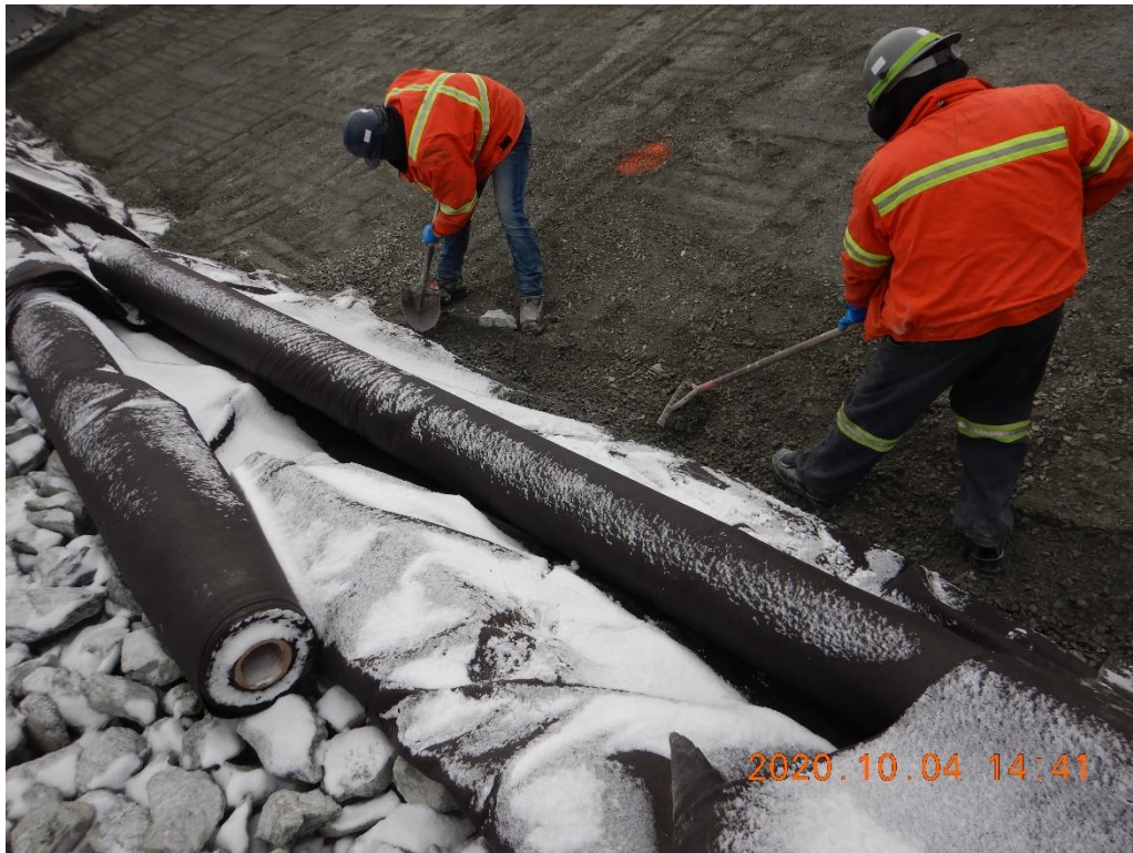
Photo 7. Ongoing finishing of the FF at the toe of the slope to ensure adequate continuity with invert FF layer and to allow easier geotextile unrolling
