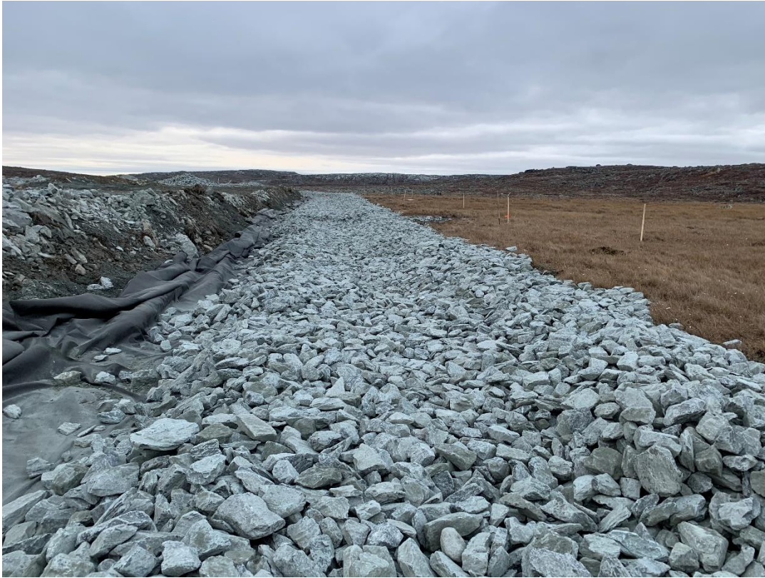
Figure 9: Geotextile and preliminary riprap between 0+034
