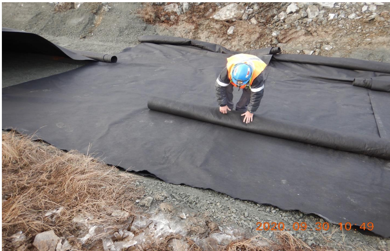
Photo 23: geotextile installation showing overlap of the different layers installed, St. 0+050.
