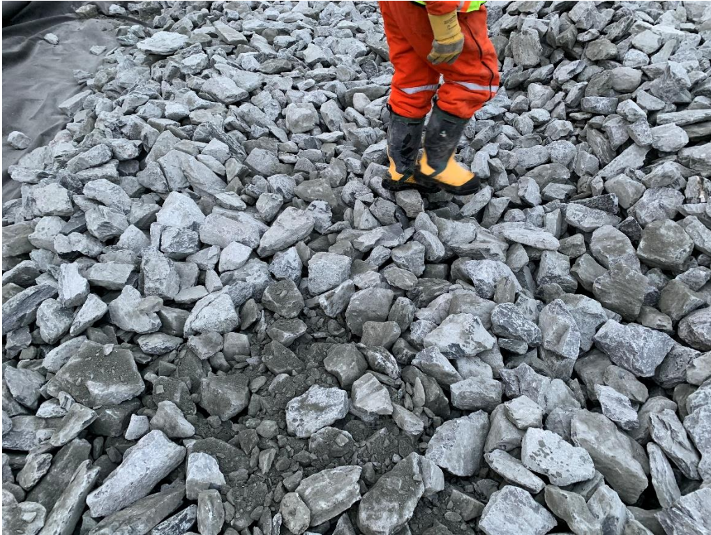
Figure 1: Nonconforming material to be removed before final approval
