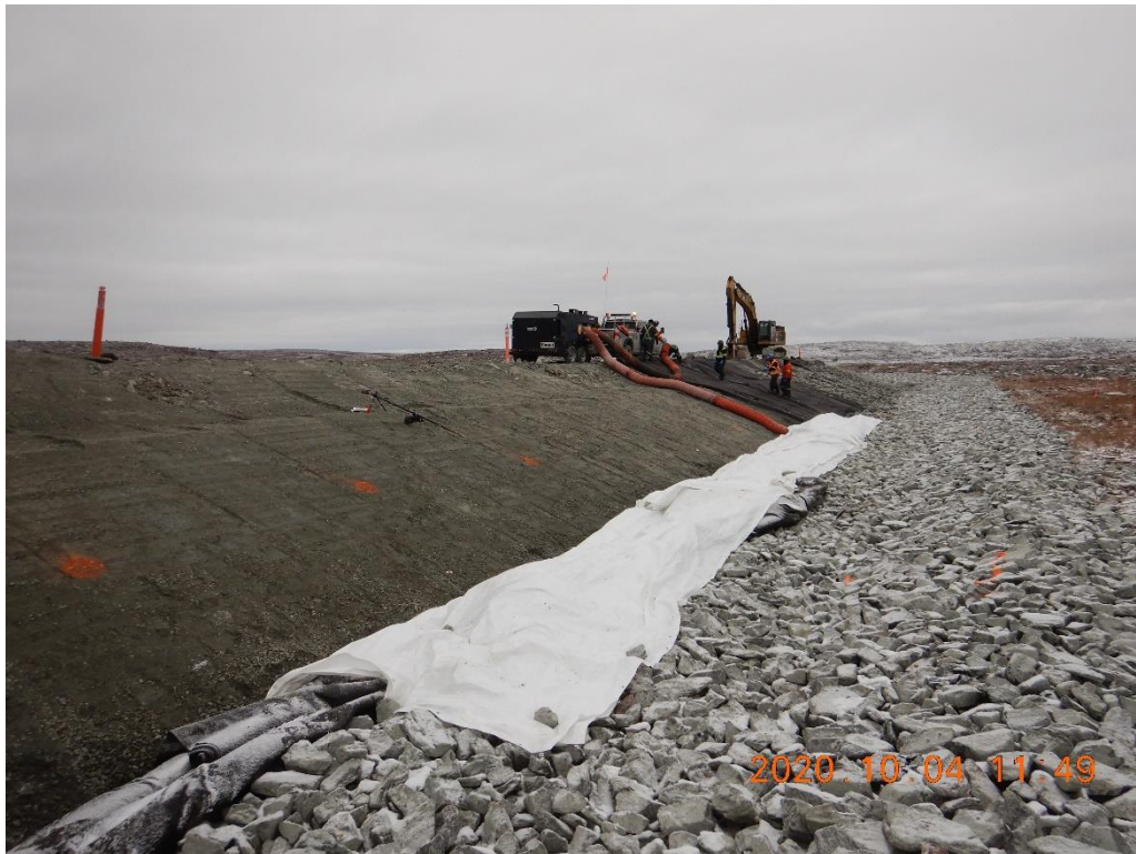
Photo 6. Frost fighter and tarp setup used when needed to unfreeze the geotextile rolls.
