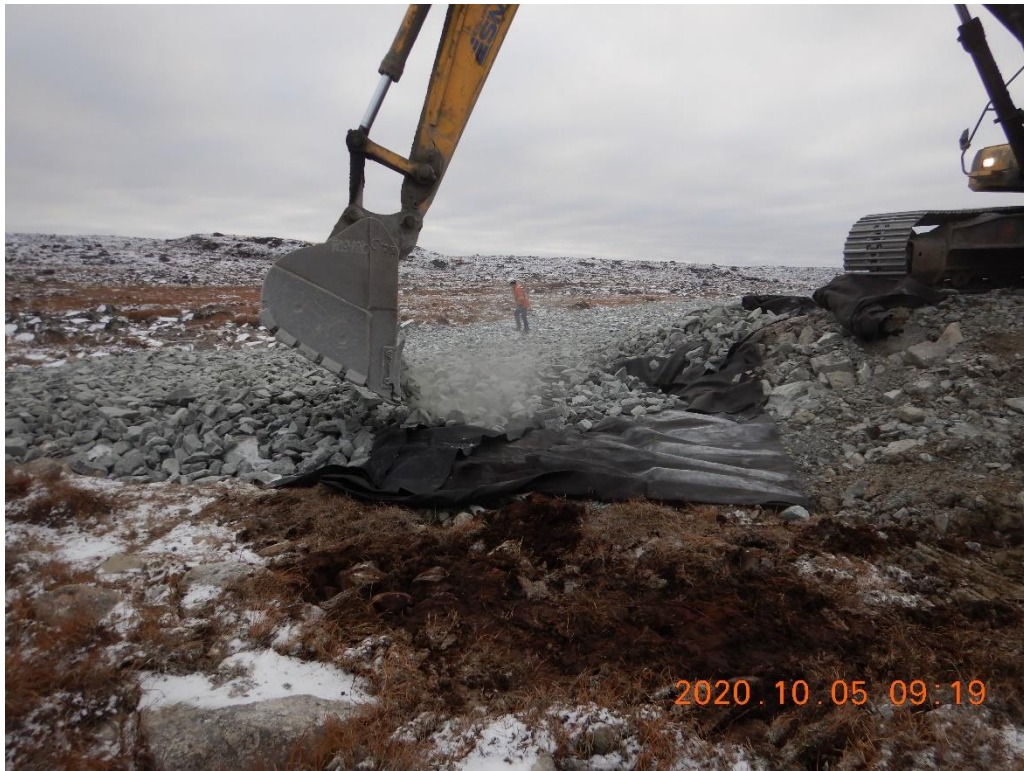
Photo 2. Rip rap placement at downstream end of the channel. Geotextile laying at natural ground elevation. Looking South-East.
