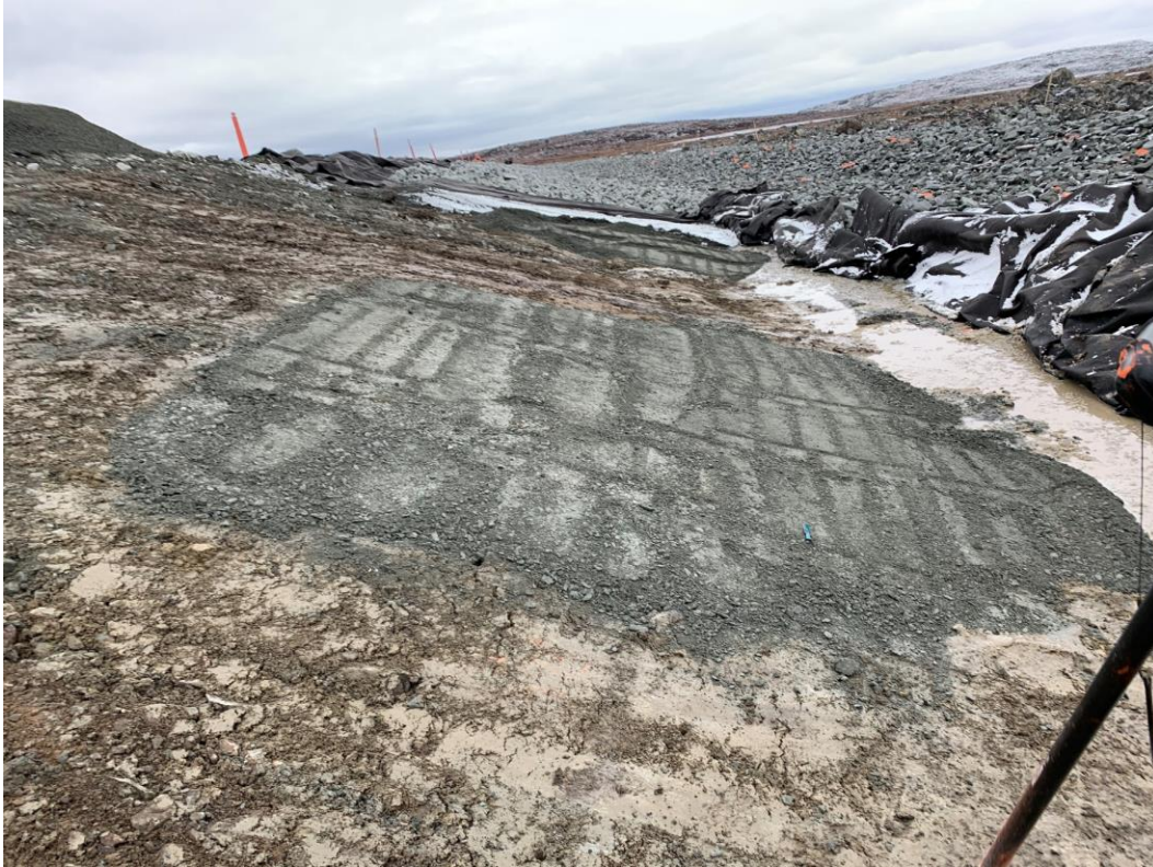
Figure 3: Excavated material replaced by well-compacted fine filter
