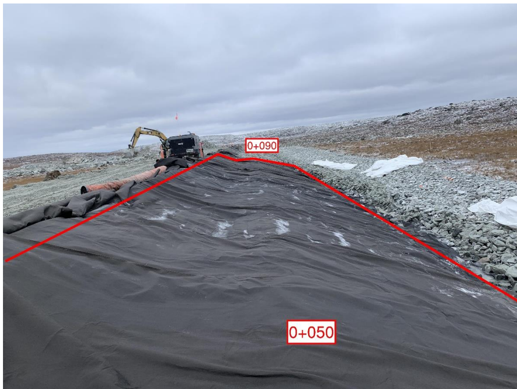
Figure 2: Geotextile between 0+050 and 0+090
