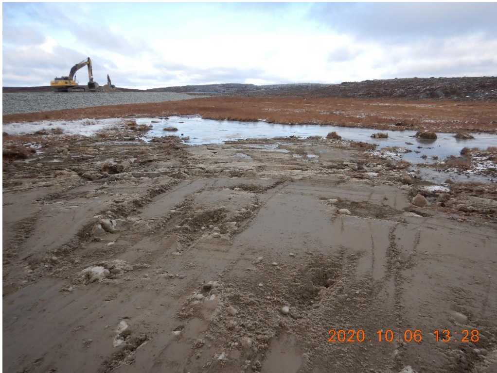
Figure 2. Main dewatering sump used during construction has been backfilled with esker material
