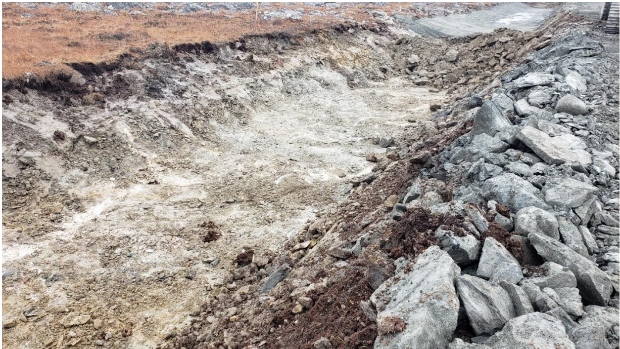
Photo 10: ice-rich till at the bottom of the planned excavation, St.0+250 looking North.
