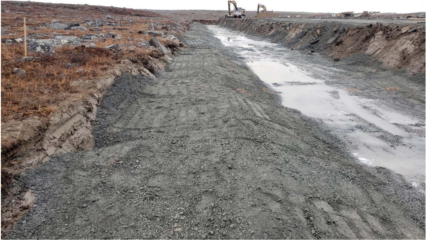
Photo 4: fine filter placement completed on the upstream tablet, St.0+240 looking South. Tablet was built on the entire length between 0+281 to 0+139.
