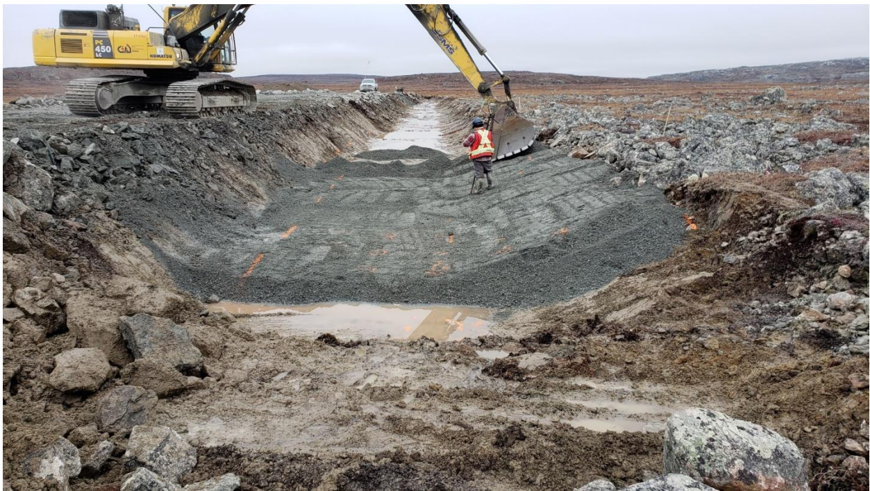
Photo 17: fine filter placement, St.0+145 looking North-West.
