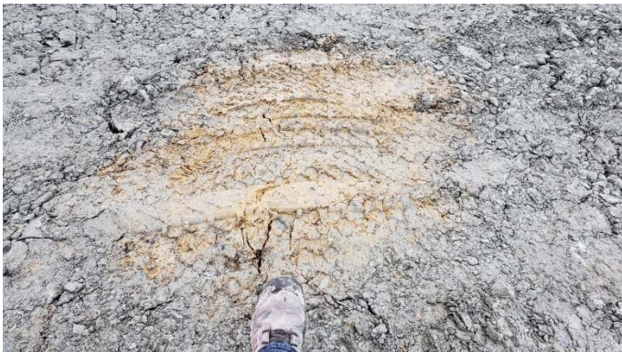
Photo 2: first pass of the excavation of the channel to drain surface water, 0+250 looking north at the sump at the end of the channel. \pm 0.5\text{m} of original tundra was removed on that picture.
