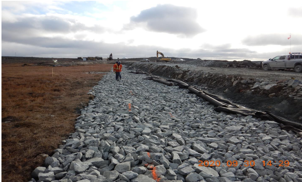
Photo 26: rip rap placement completed on the upstream side for section 0+015 to 0+090, looking South-East. Downstream berm not sloped to final grade.
