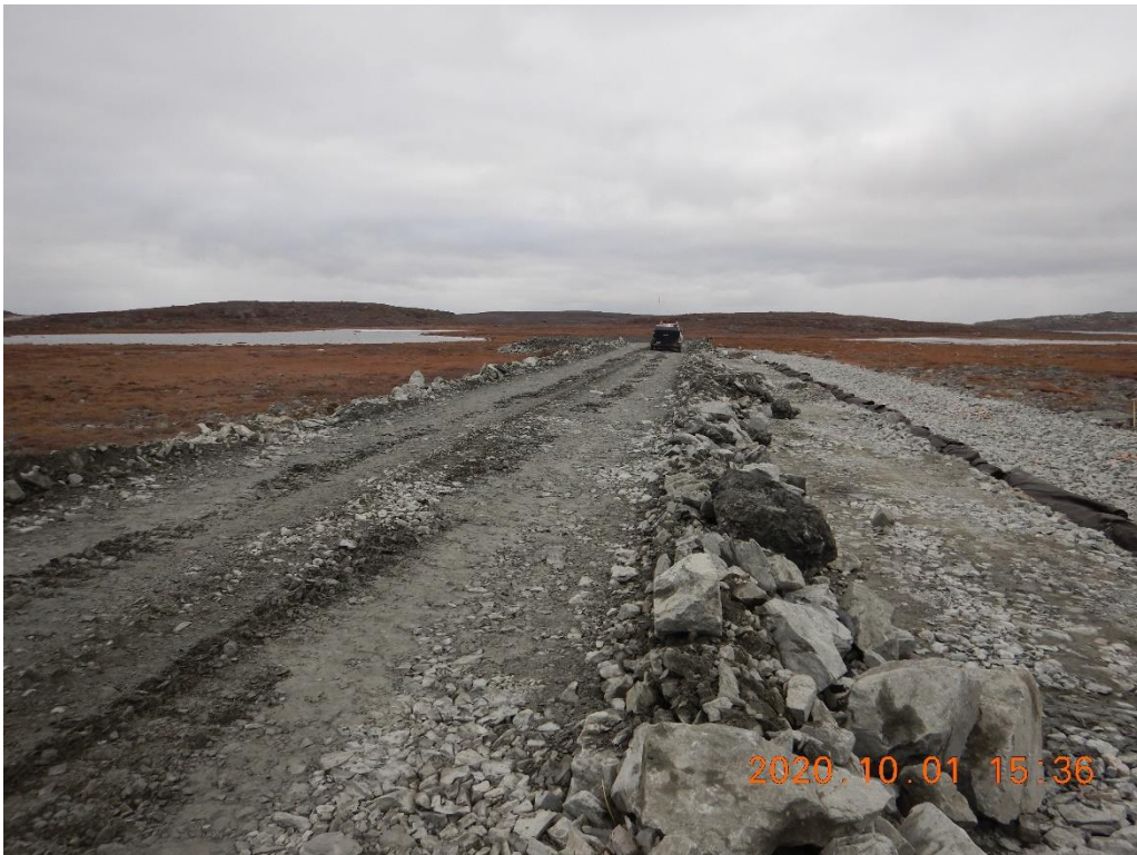
Photo 2. Final access road rockfill lift. Surface compaction with dozer and truck traffic. Adequate rolling surface. Looking North, STA 0+200
