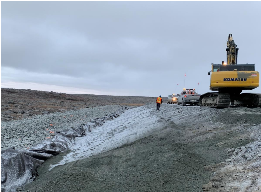
Figure 2: Fine filter placed between 0+162 and 0+230
