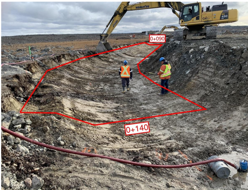
Figure 2: Foundation approval between 0+090 and 0+140
