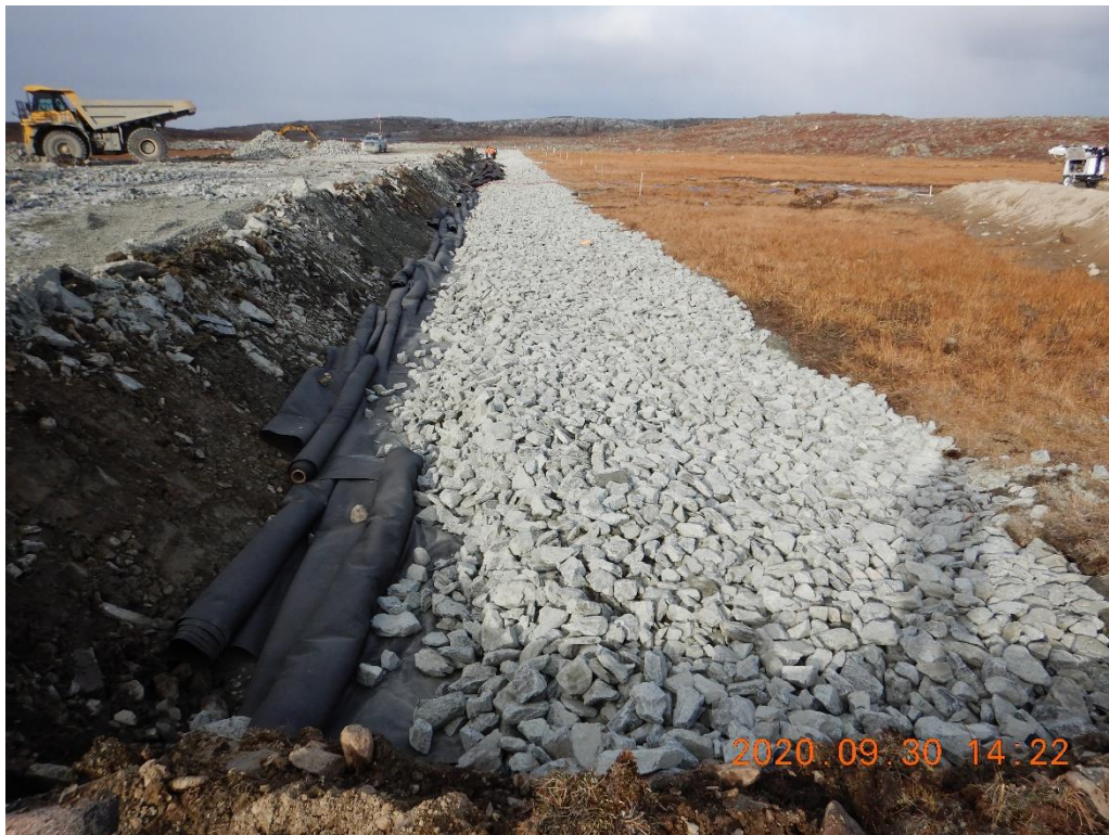
Photo 7. Rip rap placed to final grade on the invert and east slope, looking north from -0+015.
