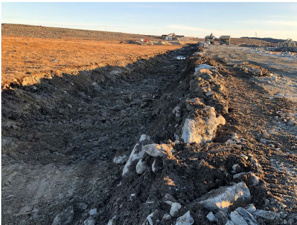
Photo 4: hammering of the first 400mm of frozen till, St.0+125 looking South. Clean up and assessment needs to be done.
