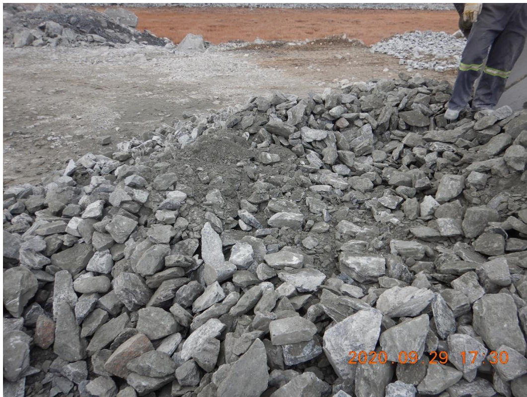
Photo 5: rip rap load containing a localized amount of finer material. This amount is rejected and tossed away. Such finer material shall not be placed in the channel. If it is so, it will need to be cleaned manually, to minimize risks of damaging the geotextile liner.
