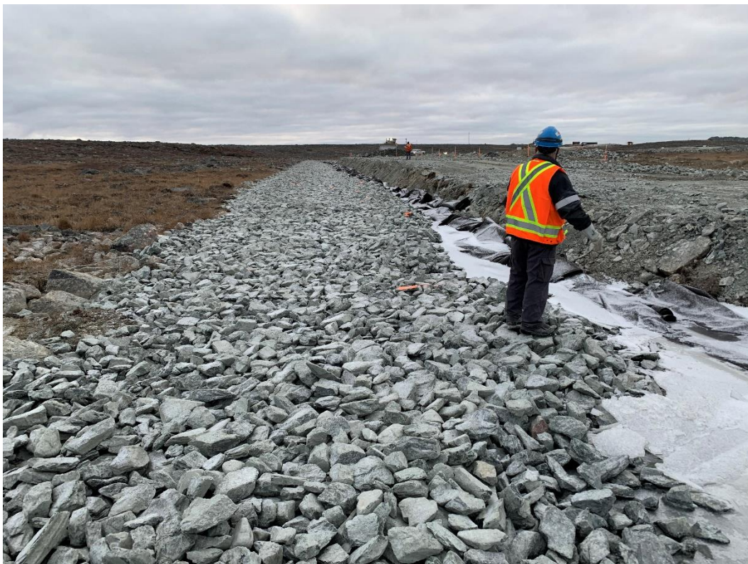
Figure 6: Riprap approval between 0+140 and 0+284.5
