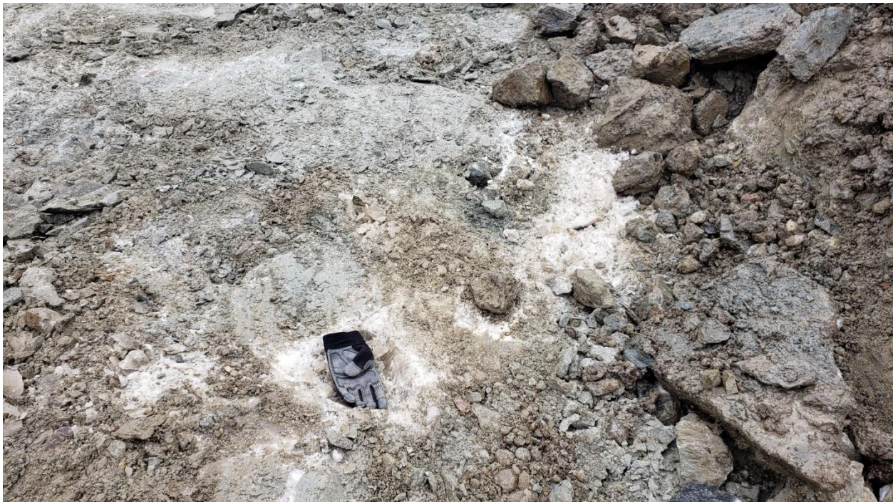
Photo 11: ice lens within an ice-rich till area, St.0+247. Ice was removed from the bottom of the excavation and under the downstream slope toe, right on the photo.
