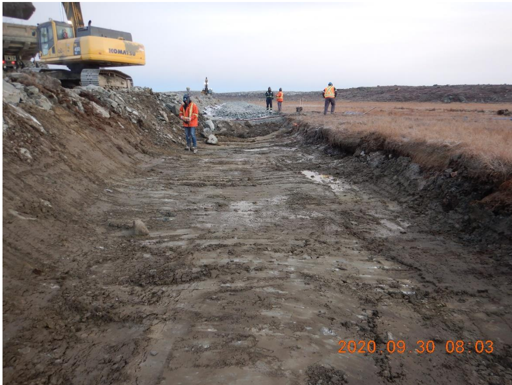
Photo 2. Bottom of the excavation from -0+015 to 0+029 after final clean up, looking north. Superficial thawed soil and water removed prior to backfilling FF.
