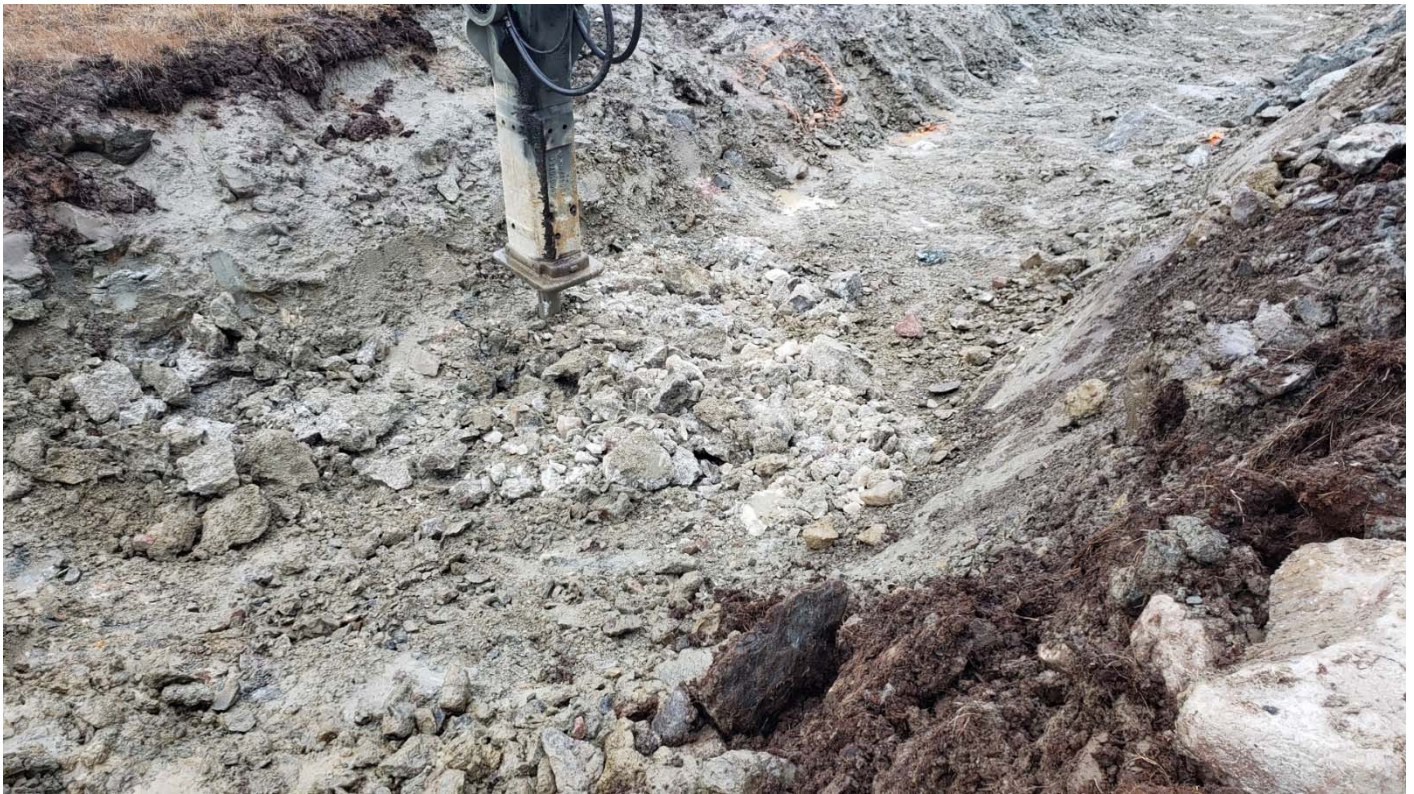
Photo 3: 2 nd pass of the removal of the ice rich till with hydraulic hammer, Sta. 0+260 looking South-East.
