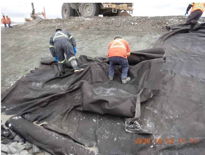
Photo 4. Geotextile placement at 0+150. Roll on the photo was partially damp and frozen
