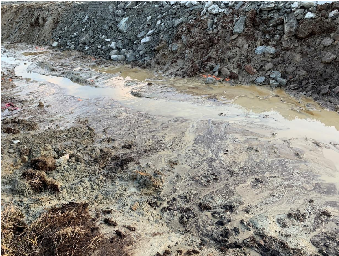
Figure 3: Ice-rich material at the bottom of the excavation
