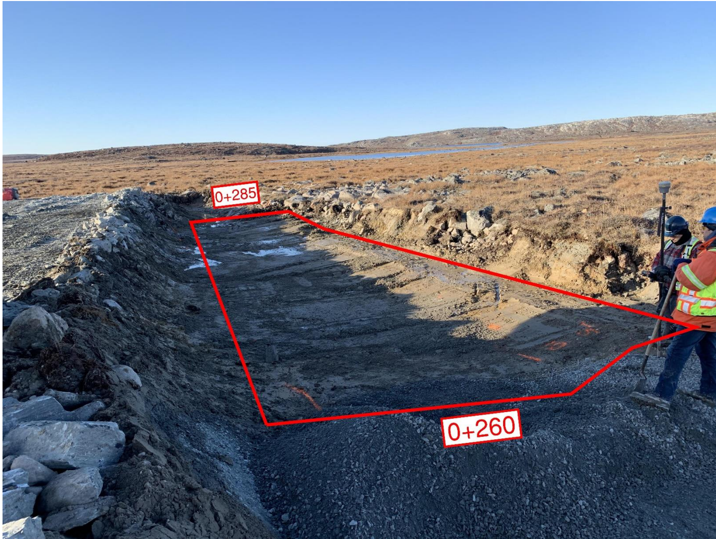
Figure 1: Foundation approval between 0+260 and 0+285
