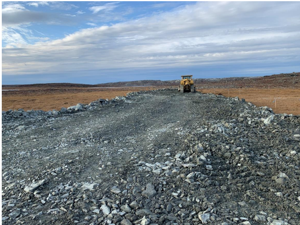
Figure 2: Visual gradation of the rockfill at the surface
