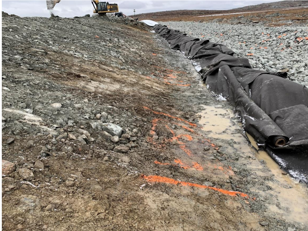
Figure 3: Soft spot identified
