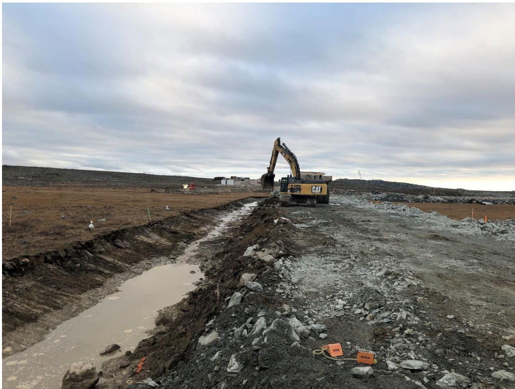
Photo 7: excavation St.0+150 looking South. First step of preliminary excavation near the shovel and final depth reached at bottom left, St.0+150 looking South-East.
