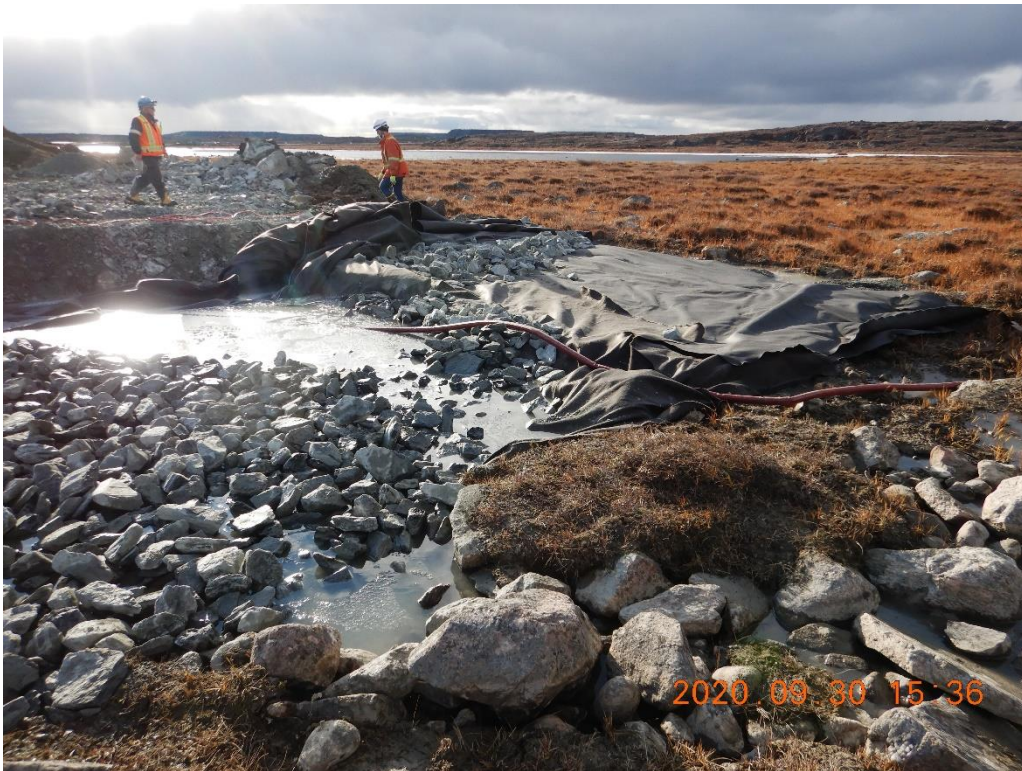
Photo 12. Two layers of geotextile placed on top of fine filter material (Photo 11). Rip rap placement ongoing on top of geotextile. Thin layer of rip rap will be placed to hold geotextile in place.
