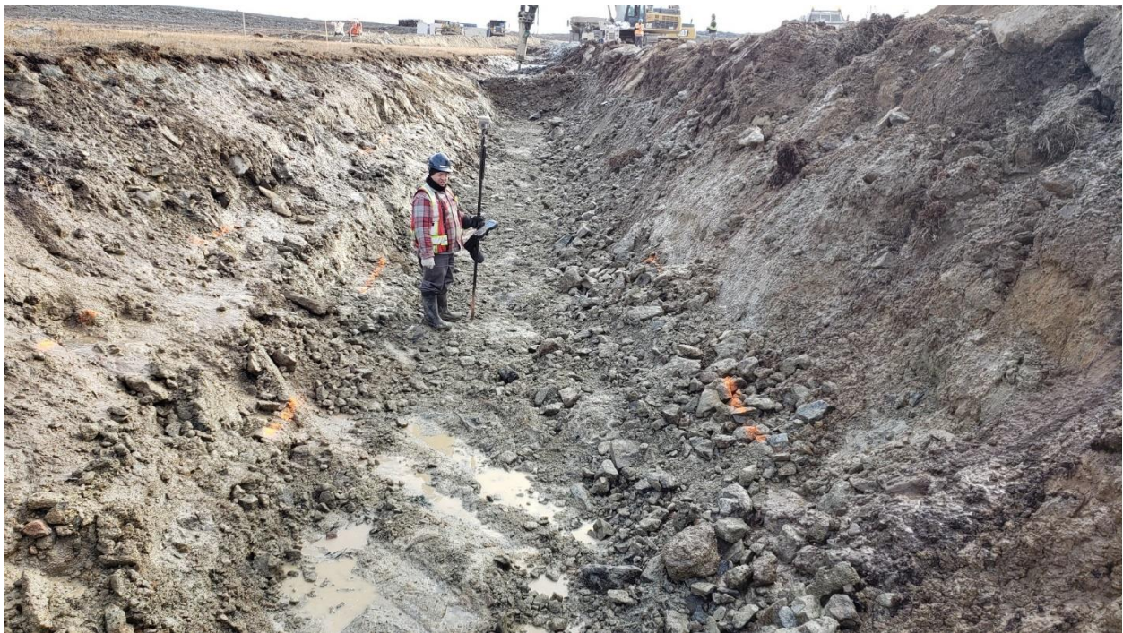
Photo 13: ice-rich till removal completed with the mechanical hammer, first 1200mm material removed, before backfilling it with esker, St.0+125 looking South-East.
