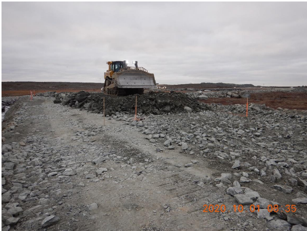
Photo 1. Rockfill placement for final lift of the access road along the west side of the channel looking south from around 0+200
