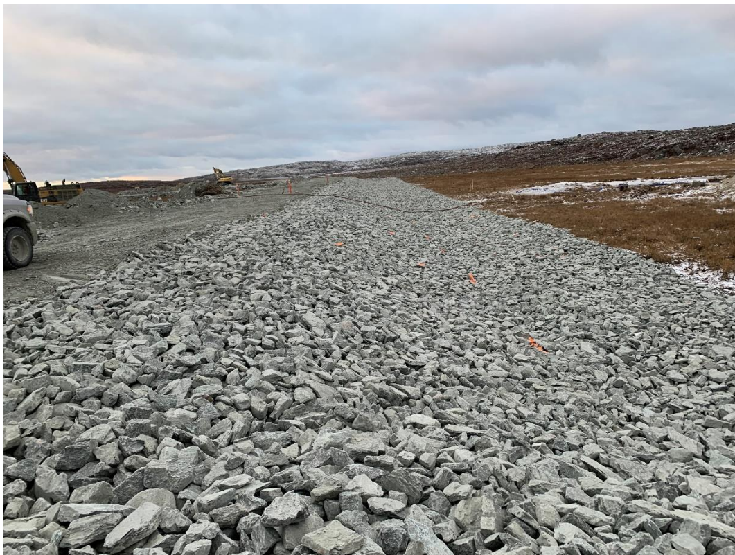
Figure 4: Riprap to final grade between 0-015 and 0+140
