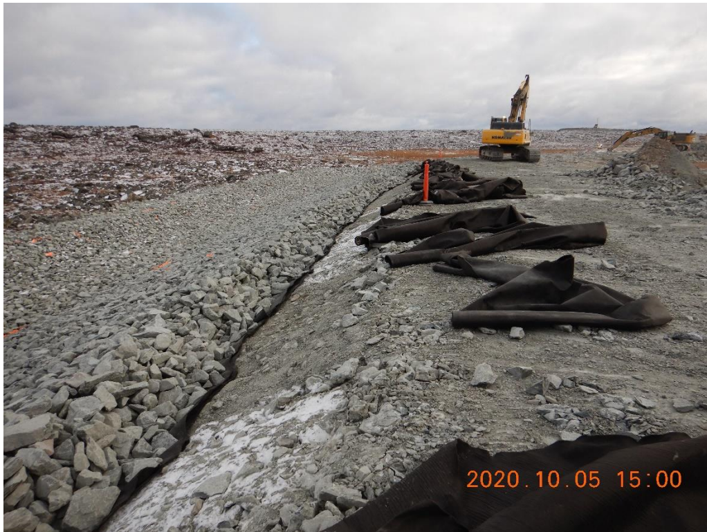
Photo 4. Exceeding geotextile removal, 0+200 looking South.
