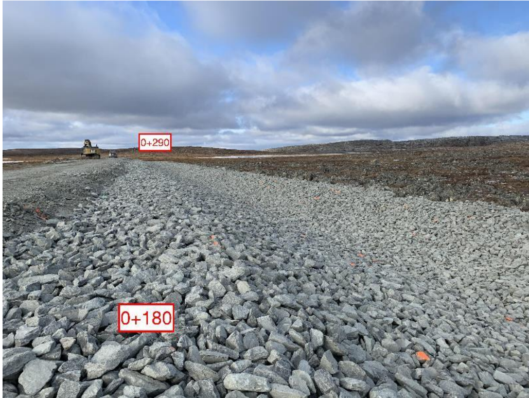
Figure 7: Riprap between 0+180 and 0+290
