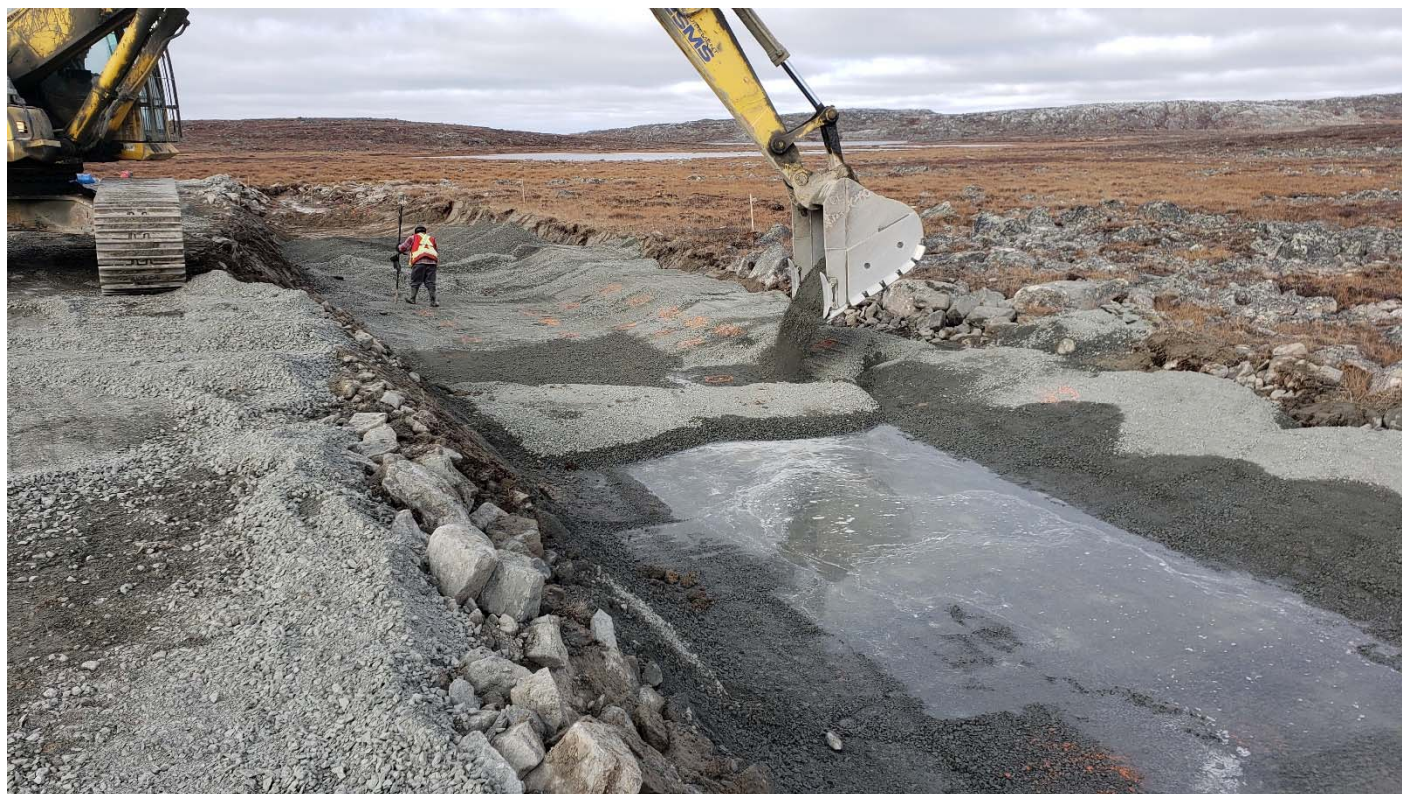
Photo 2: Fine filter placement on top of the esker, from St.0+200 looking North.
