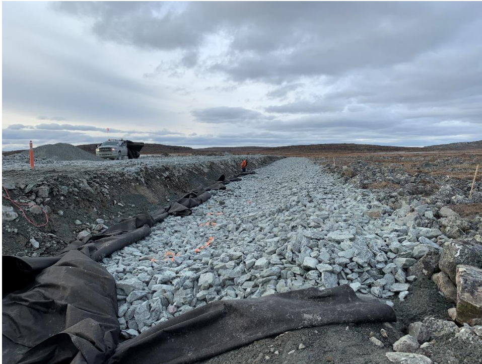
Figure 1: Riprap placement to grade between 0+155 and 0+284.5
