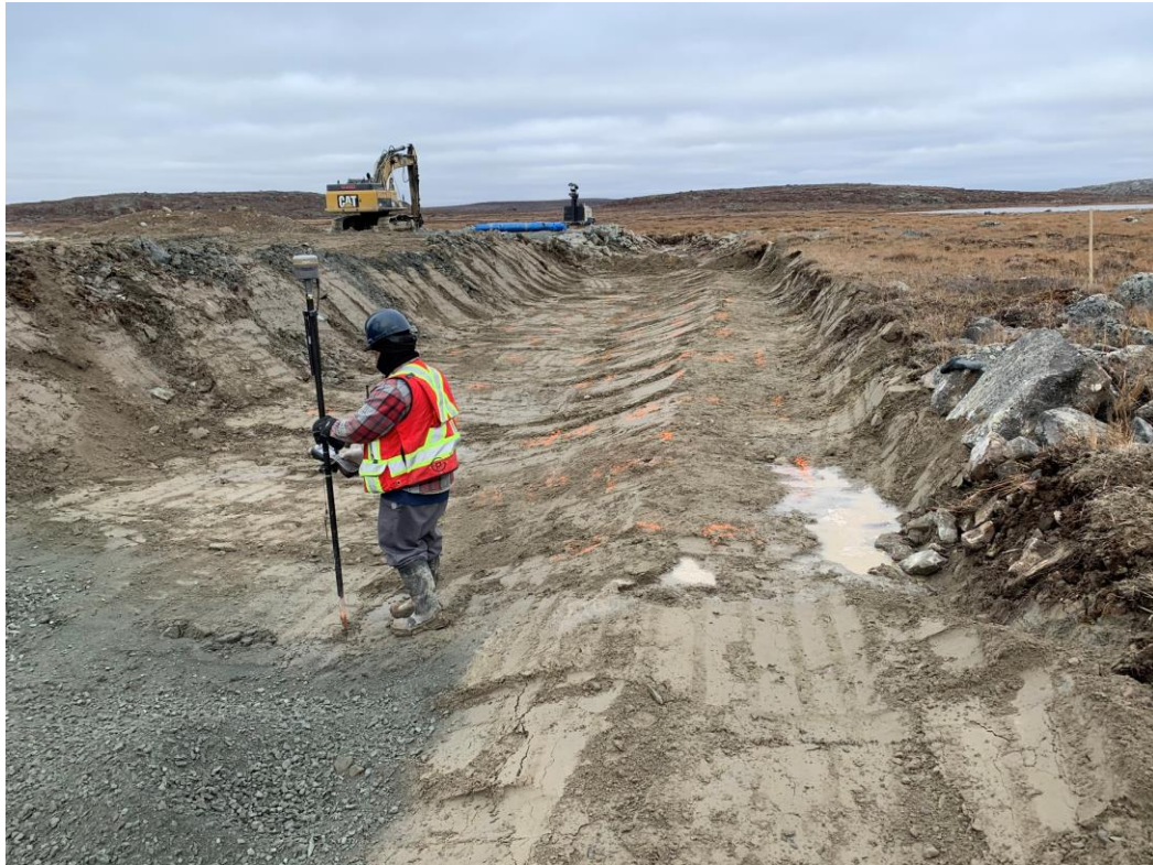
Figure 1: Foundation approval between 0+234 and 0+260
