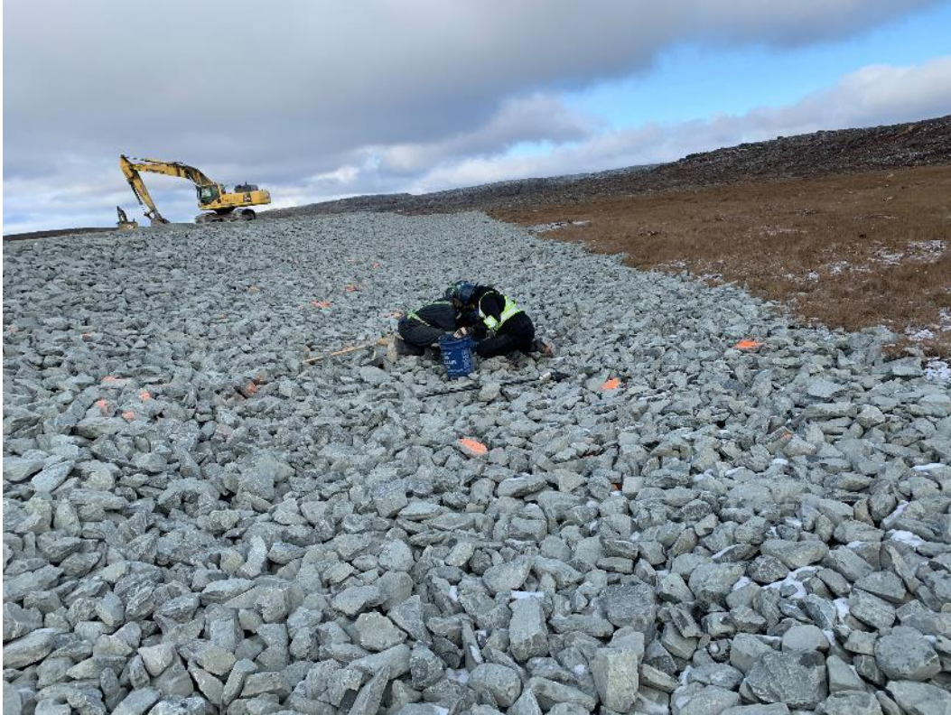
Figure 1: Fine material removal by hand
