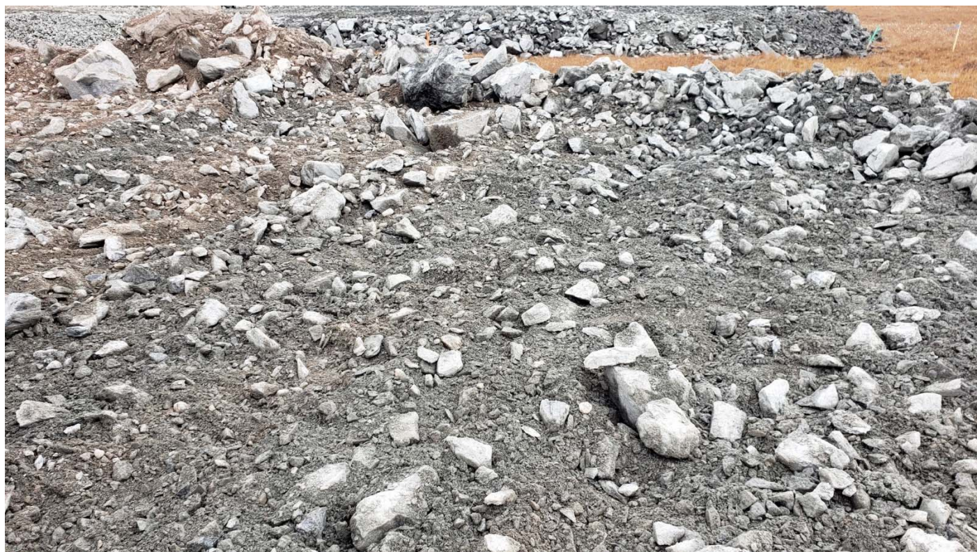
Photo 1: Close view of rockfill, at Station 0+005 to show grain size distribution of the material. Note: rockfill not compacted yet with haul trucks in this area as it is not connecting with the main berm seen on top of the photo.
