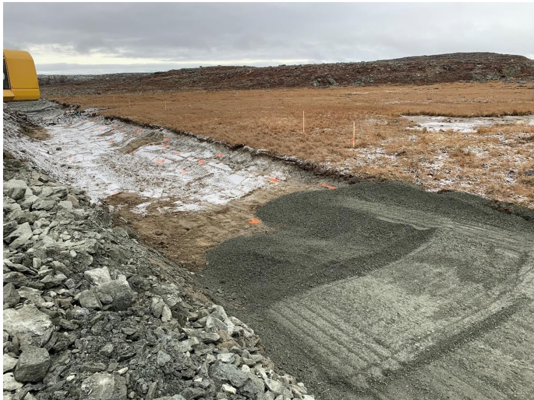
Figure 2: Fill placement in progress between 0+029 and 0+070
