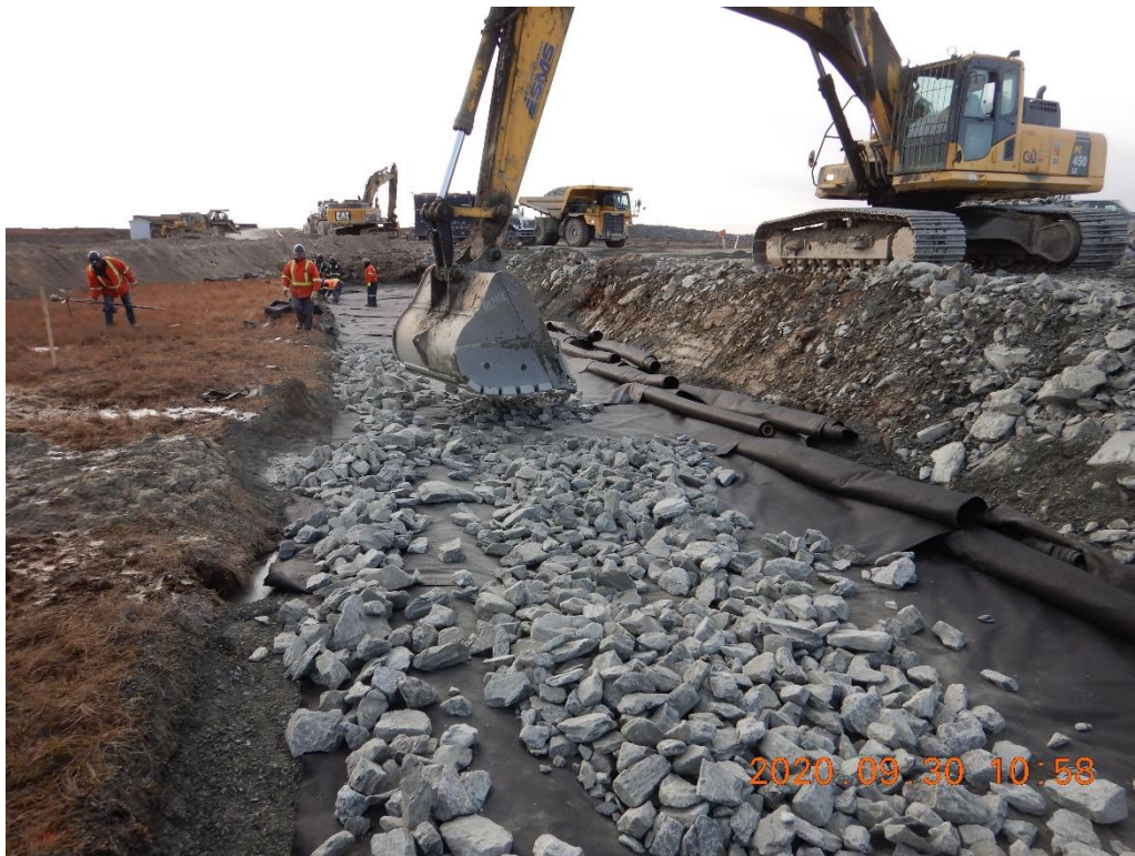
Photo 6. Rip rap placement, STA -0+015 to 0+032. Looking south
