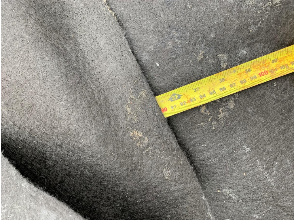
Figure 3: The geotextile overlaps were all above 600mm
