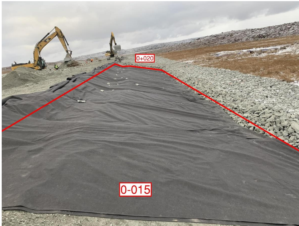
Figure 1: Geotextile between 0-015 and 0+020
