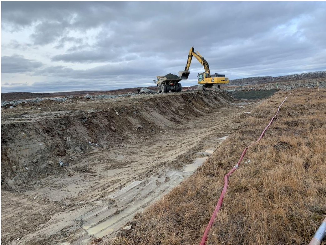
Figure 3: Foundation approval between 0+090 and 0+149
