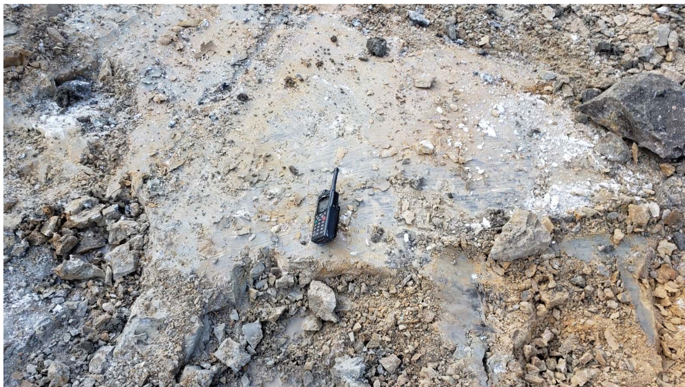
Photo 1: Frozen silty sand at the bottom of the excavation after material removal. Visually the material is ice-poor so it was accepted as is and covered with 2 layers of esker. Sample Ex-15 was taken for water content.
