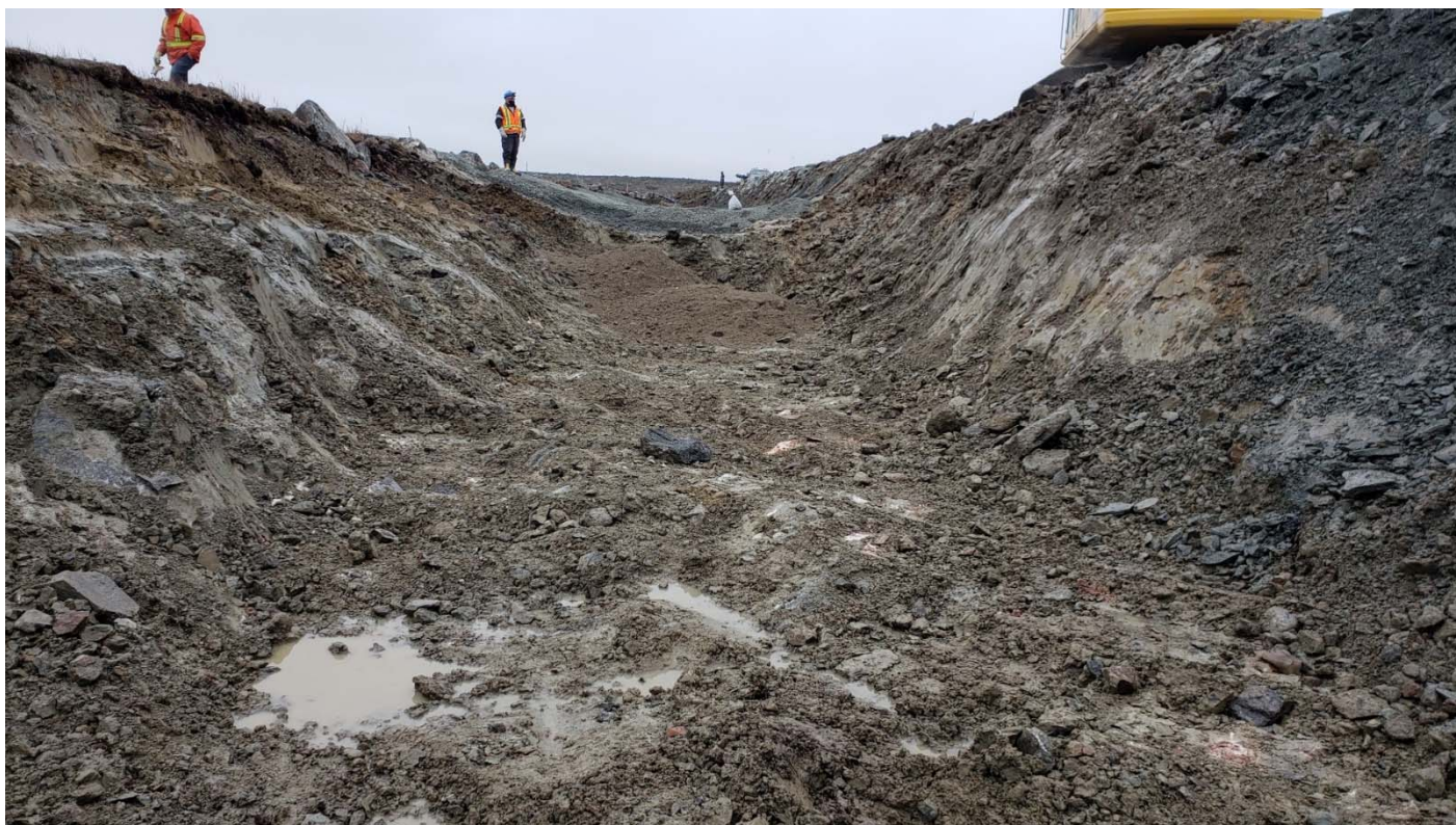
Photo 5: bottom of the ice rich section once all accessible till removed, St 0+255 looking S-E towards 0+235. Esker placement started by dropping loads of esker material with excavator and compacting it.
