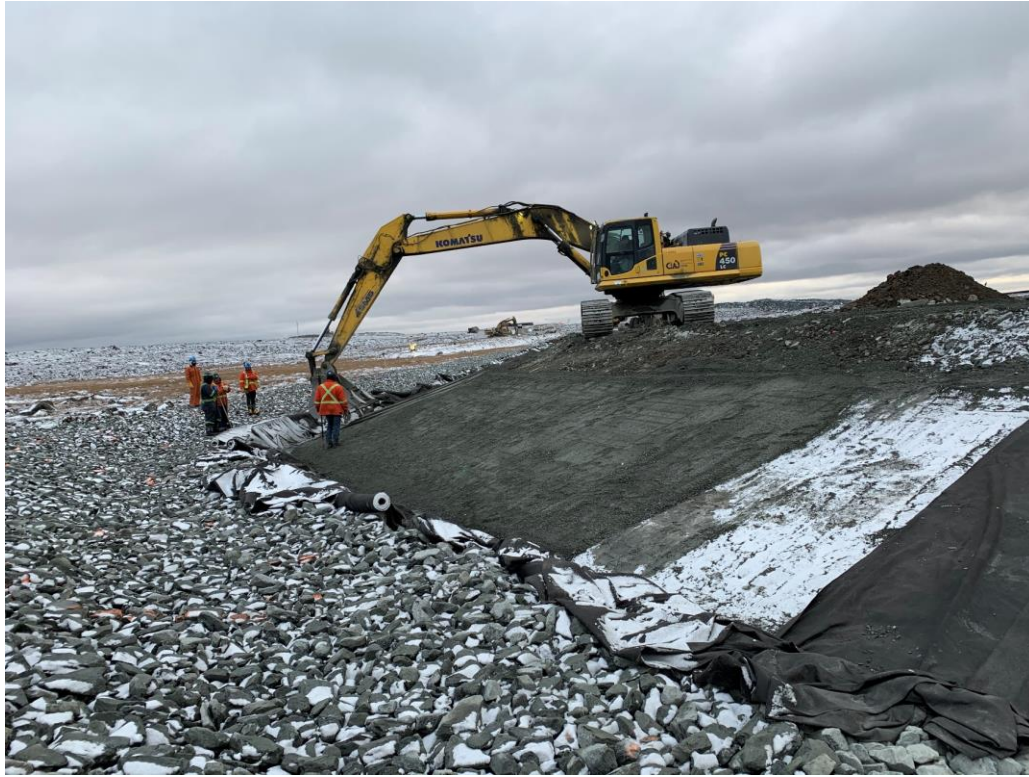
Figure 7: Fine filter approval between 0+140 and 0+155
