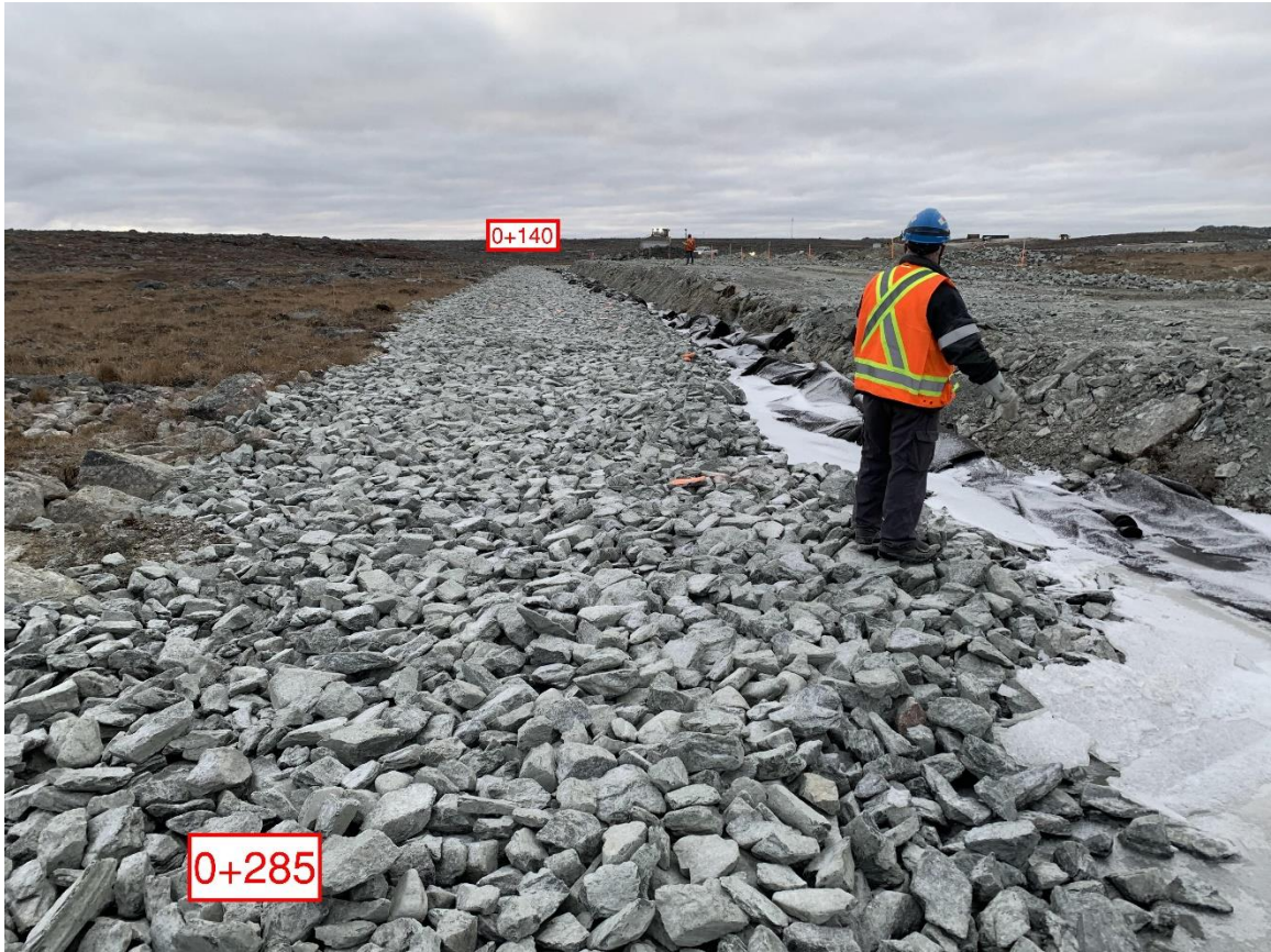
Figure 5: Riprap between 0+140 and 0+285
