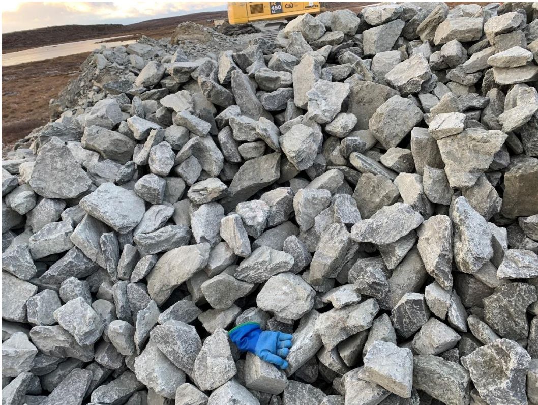
Figure 6: Riprap from the first half dumping process
