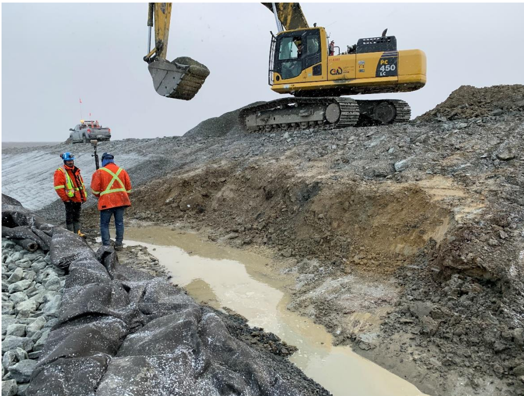
Figure 6: Ice excavated out of the foundation at 0+230
