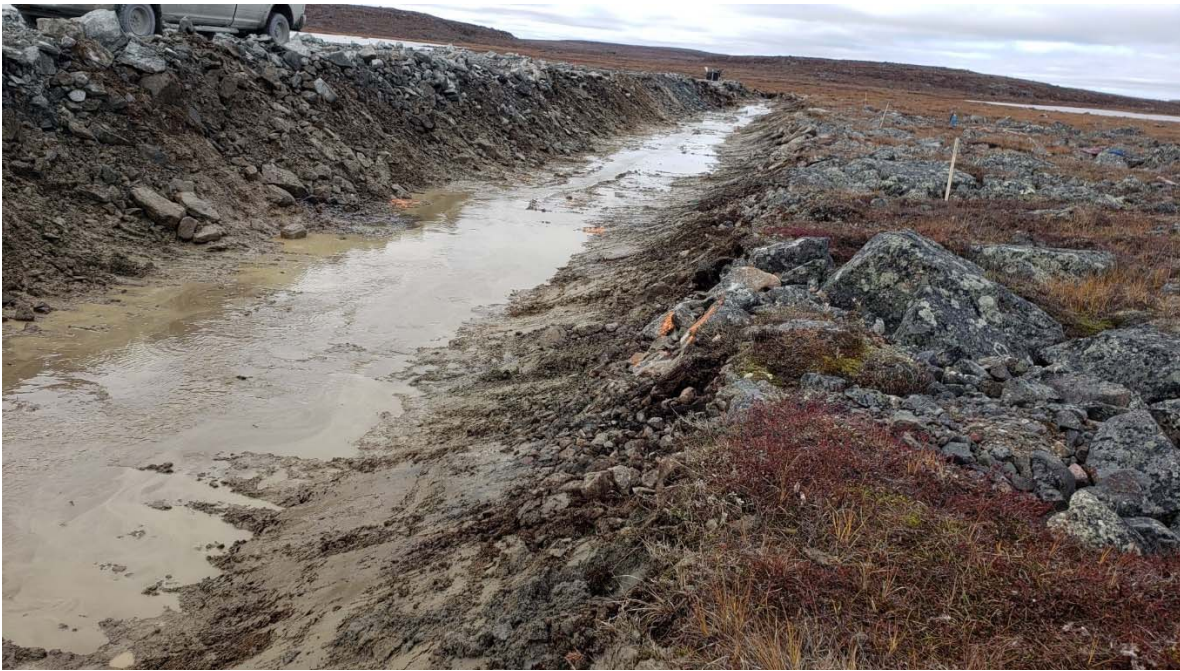
Photo 2: first pass of the excavation of the channel completed from 0+143 to +0281. Water from boulder fields along the channel and foundation still draining.
