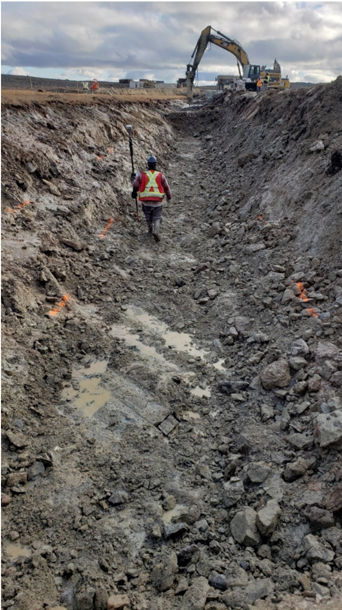
Photo 3: hammering of the frozen till to reach proper material in ice-rich sector 0+125 to 0+090, taken from St.0+125 looking South. With depth the till had gotten more ice-rich than at surface, ice lenses appeared in foundation (right). Excavation was stopped as it had reached maximum depth allowed for safety and was covered by fine esker material. Results of the water content of 3 till samples taken from that section, 20 (planned elevation), 24 and 25% (bottom of excavation), gradation on materials ongoing.
