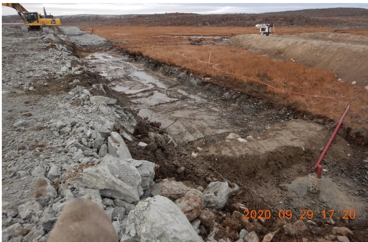
Photo 1: view of the bottom of the excavation, not final, at St.-0+015 looking North. Sump located at the upstream end of the channel at -0+015. Water in the excavation is coming from tundra runoff. Final excavation clean up to do prior to placing fine filter material.
