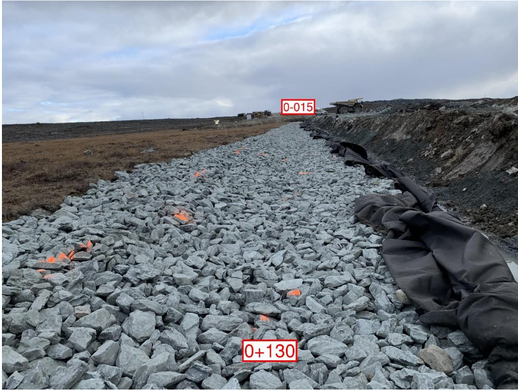
Figure 3: Riprap between 0-015 and 0+130
