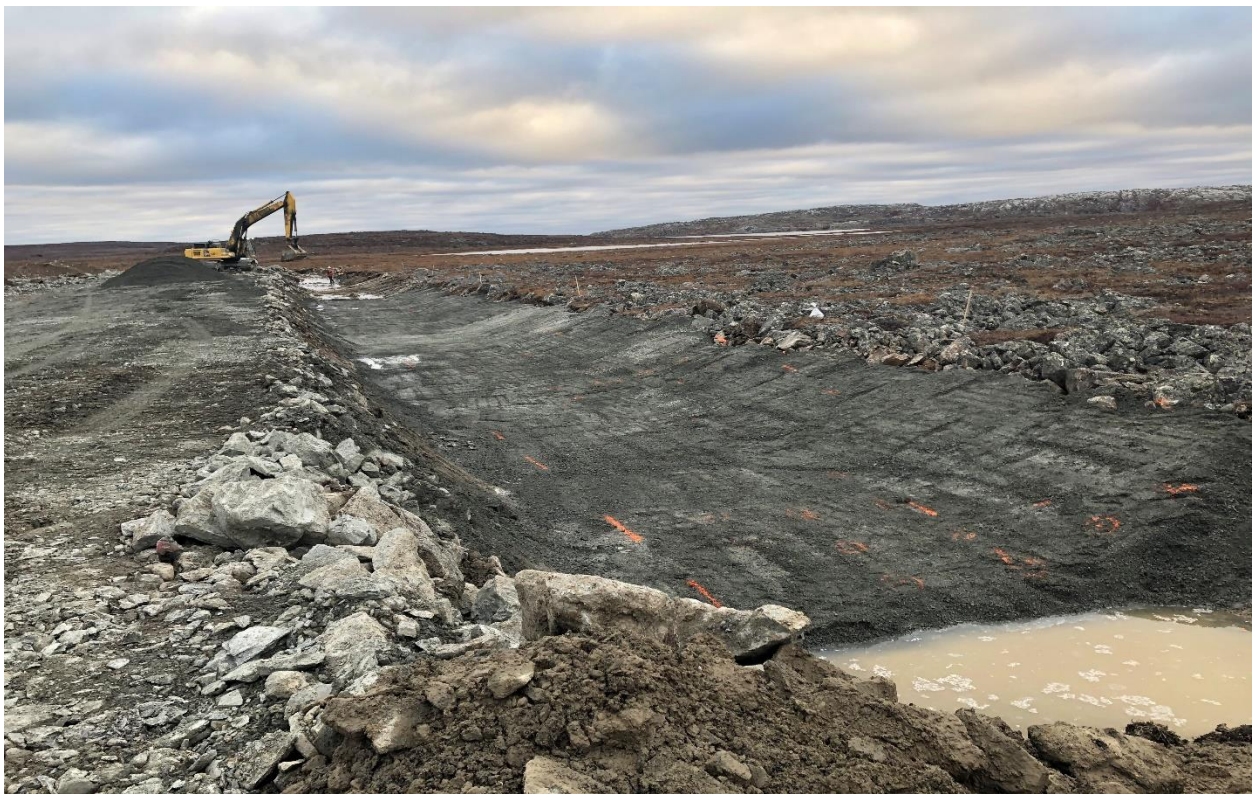
Figure 19: fine filter placement final approval before geotextile installation, St.0+140 looking North-West.
