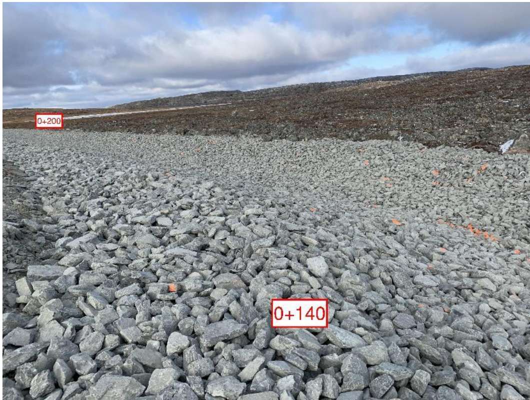
Figure 6: Riprap between 0+140 and 0+200
