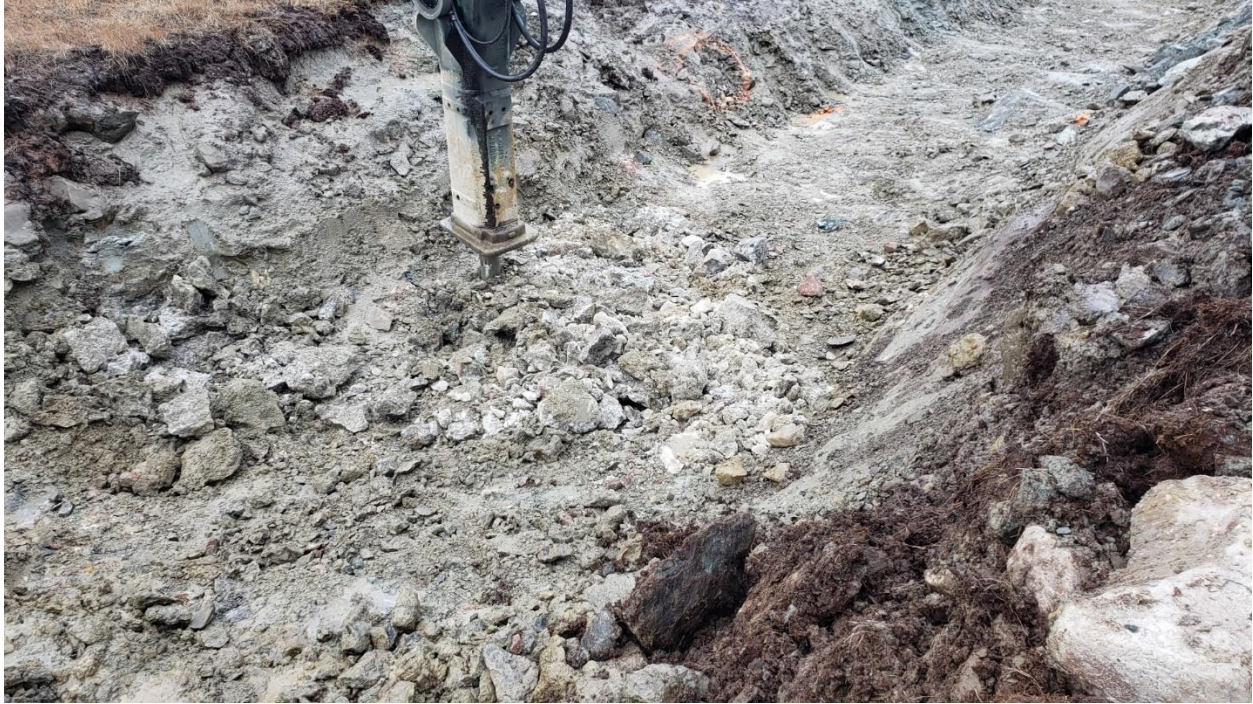
Photo 12: ice-rich till removal with a mechanical hammer, first 600mm material removal, St.0+125 looking South-East.
