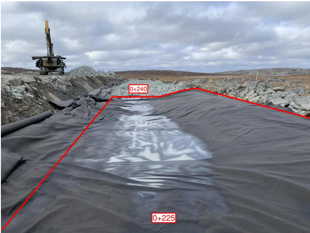
Figure 2: Geotextile between 0+225 and 0+240
