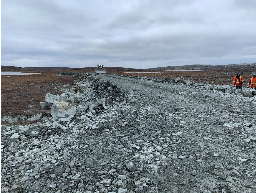
Figure 1: Final access road lift between 0+162 and 0+284.5
