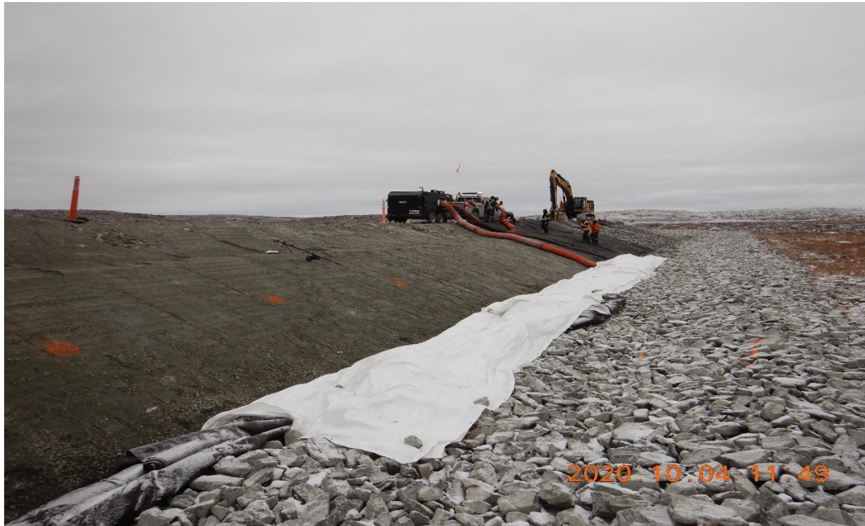
Photo 30: final fine filter placement in the downstream slope before geotextile placement, St. 0+070 looking North-West.
