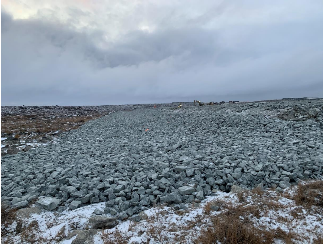
Figure 5: Riprap to final grade between 0+140 and 0+290
