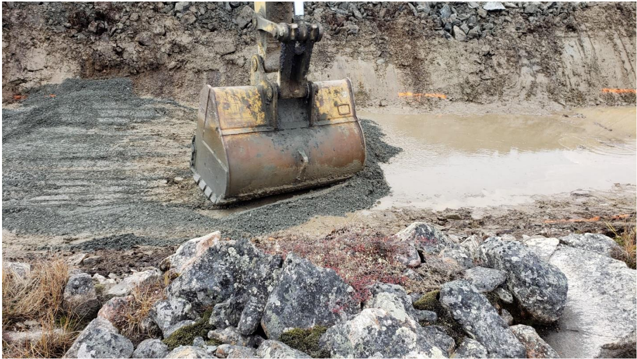
Photo 18: fine filter placement, pushing the water and mud out of the approved foundation before placement, St.0+240.
