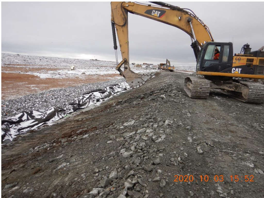
Photo 10. Remaining material from initial road lift being removed for the slope profiling. 0+070 looking south.
