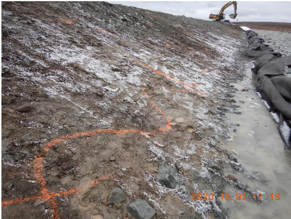
Photo 2. West slope at around 0+160. Zones with soft oversaturated material maked with spay paint, to be removed prior to FF placement
