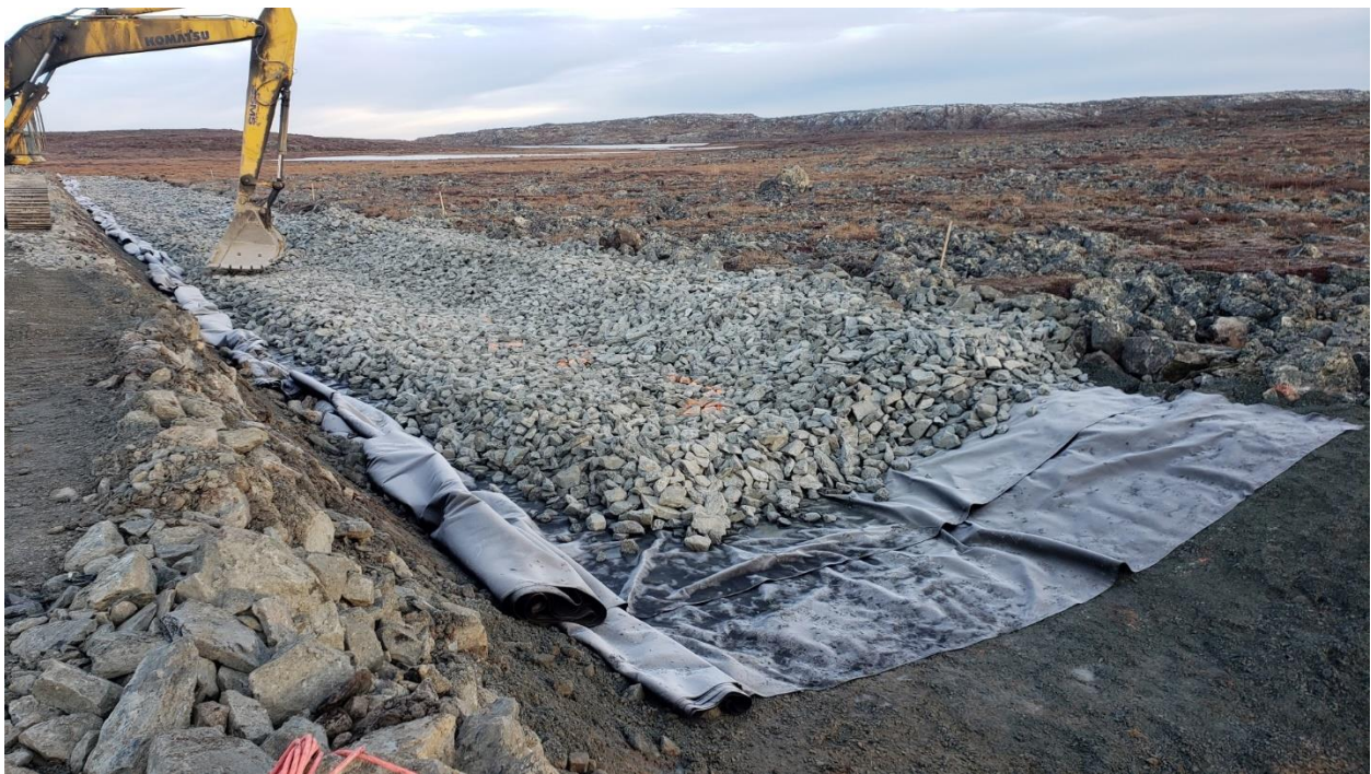
Photo 25: rip rap placement over the geotextile matching the natural topography on the upstream side, St.0+140 looking North.
