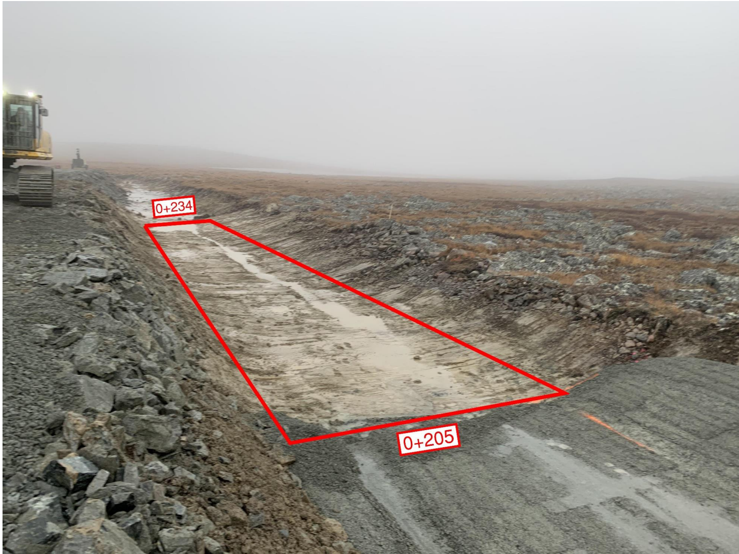
Figure 1: Foundation approval between 0+205 and 0+234
