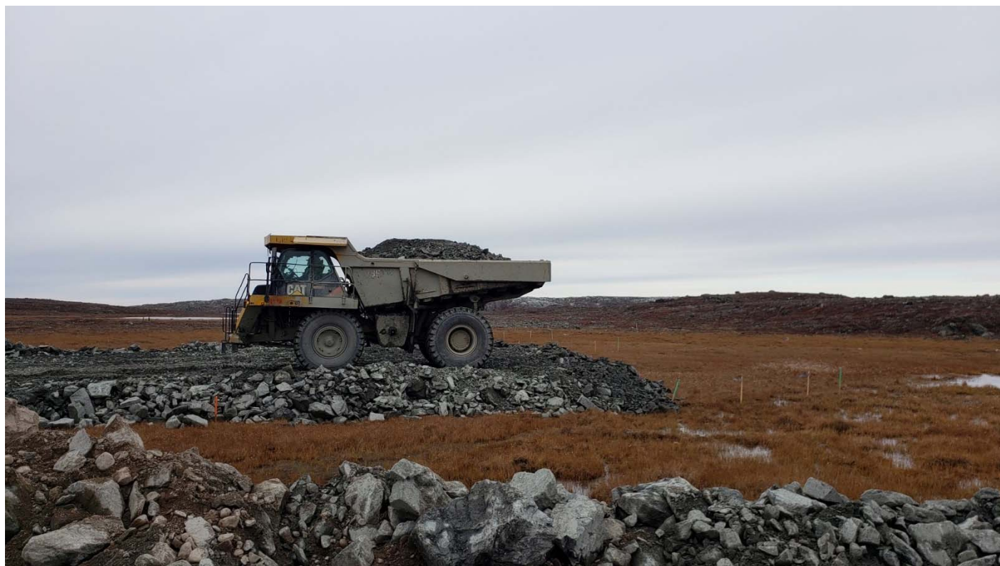
Photo 2: Construction of the d/s berm with rockfill, station 0+026. First lift slightly over the specified thickness as soft foundation encountered in the wet flat area between 0+000 and 0+125.
