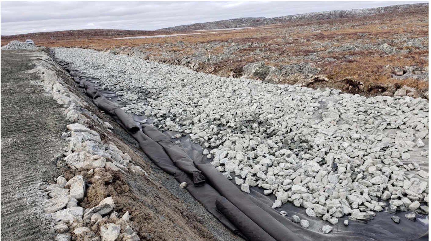
Photo 6: rip rap placement over the geotextile to hold it in place. Final riprap thickness to be adjusted and profiled, St.0+150 looking North.
