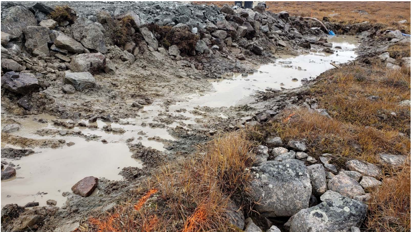
Photo 2: first pass of the excavation of the channel to drain surface water, 0+250 looking north at the sump at the end of the channel. \pm 0.5\text{m} of original tundra was removed on that picture.
