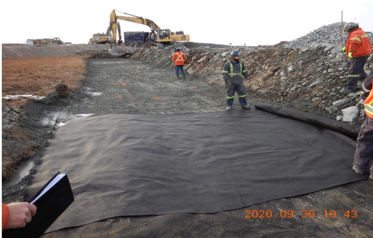
Photo 22: geotextile installation, St.0+050 looking South-East.
