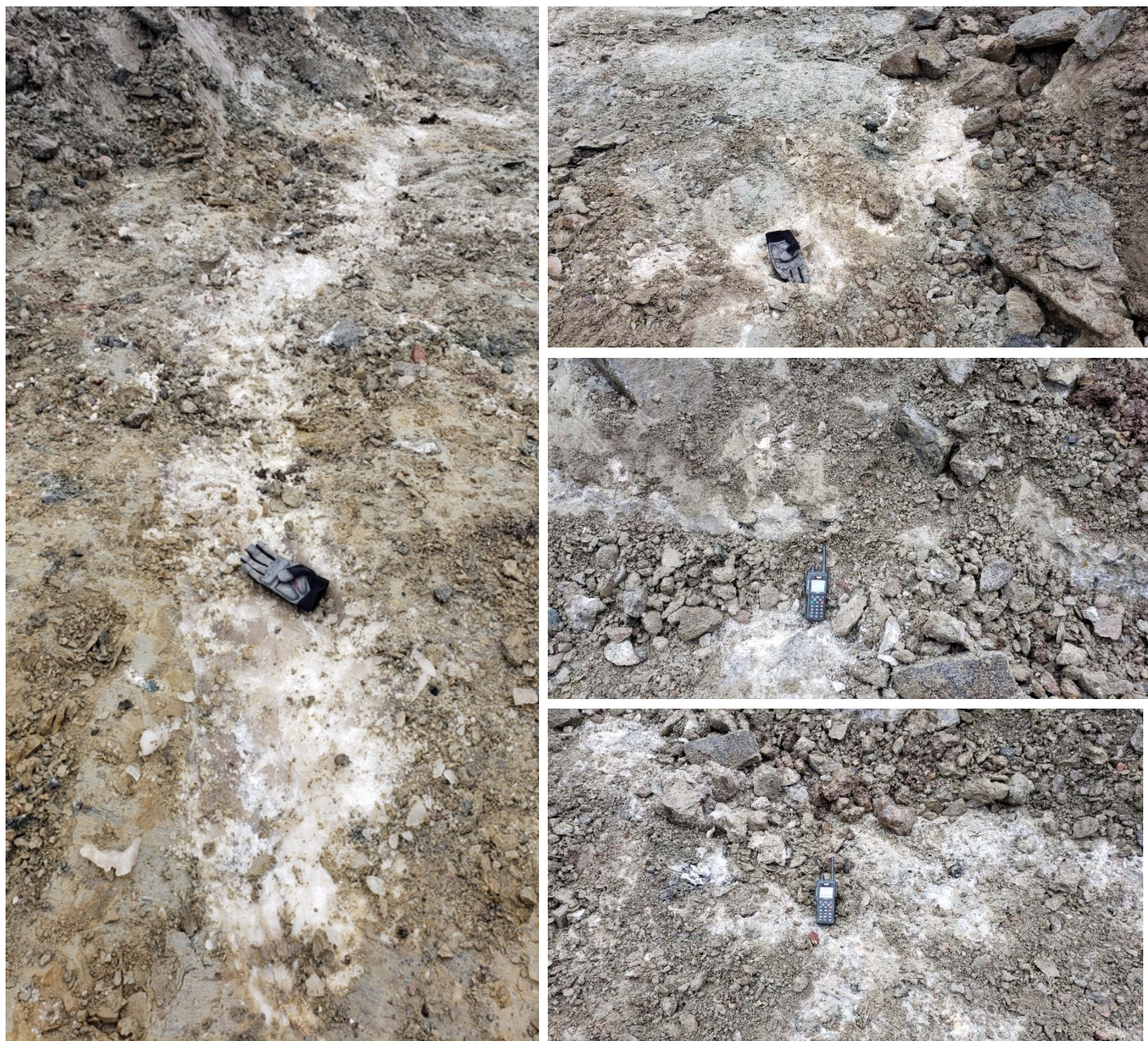
Photo 2: Ice lenses present after the first hammer pass at Station, Sta. 0+240 to 0+260.
