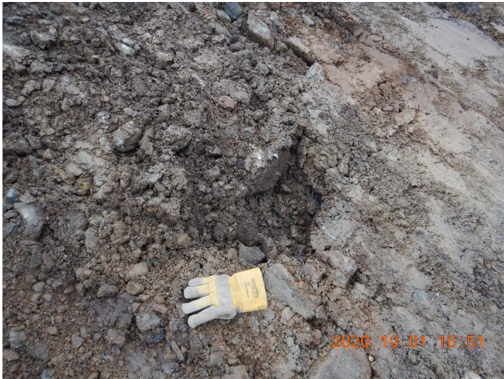
Photo 4. Ongoing slope excavation. Natural ground material. Till with gravel, sand, boulders and some organic matter in the upper portion. Material is dryer towards the top and more humid at the toe
