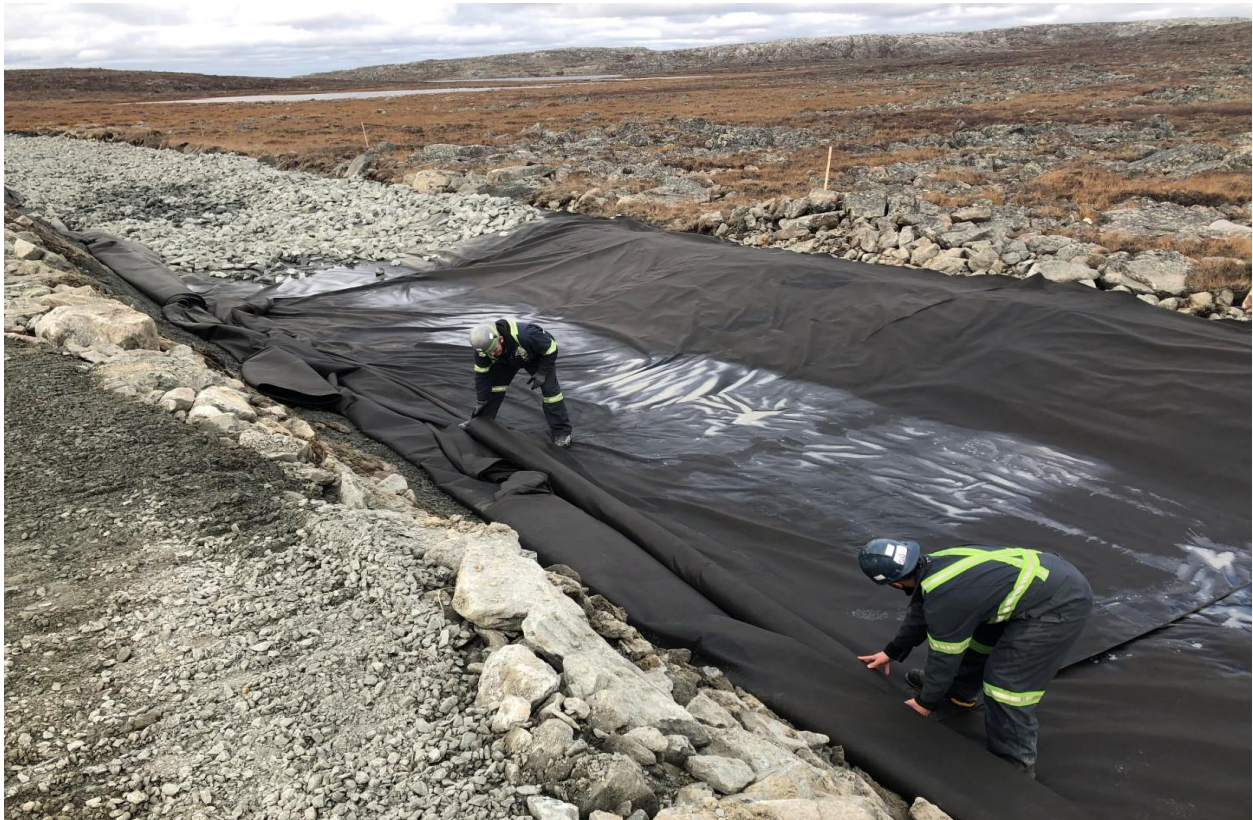
Photo 24: geotextile installation followed by rip-rap placement, St.0+200.
