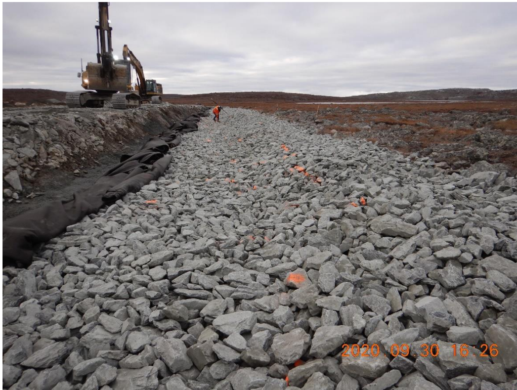
Photo 8. Final sloping, profiling and grading of the rip rap layer, invert and east slope. Photo taken around 0+160 looking north.
