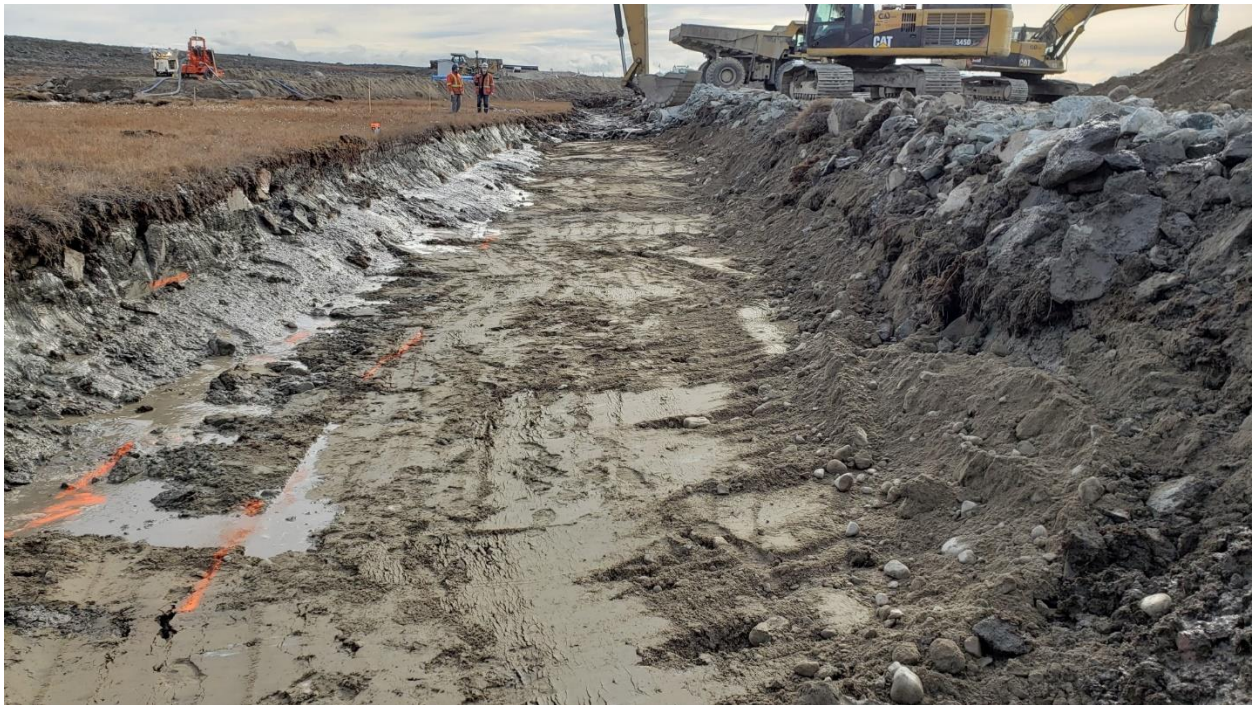
Photo 15: backfilling of the ice-rich till area 0+125-0+090 with compacted esker material completed to match planned channel bottom elevation, looking South-East.
