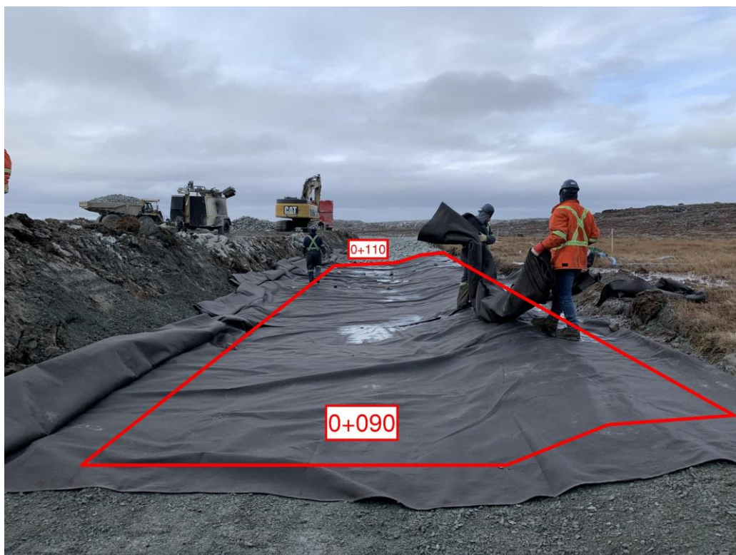
Figure 2: Geotextile between 0+090 and 0+110
