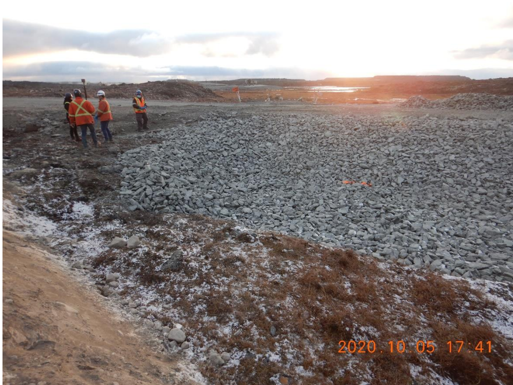
Photo 6. Finished upstream end of the channel with rip rap layer
