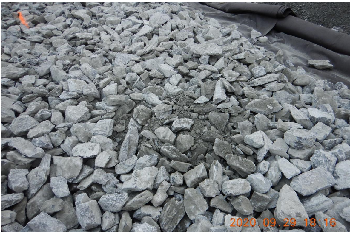
Photo 3: Localized excess of finer material in rip rap at 0+140 & 0+045 to be removed.
