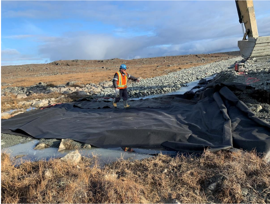
Figure 7: Geotextile placement at the downstream end between 0+284.5 and 0+290
