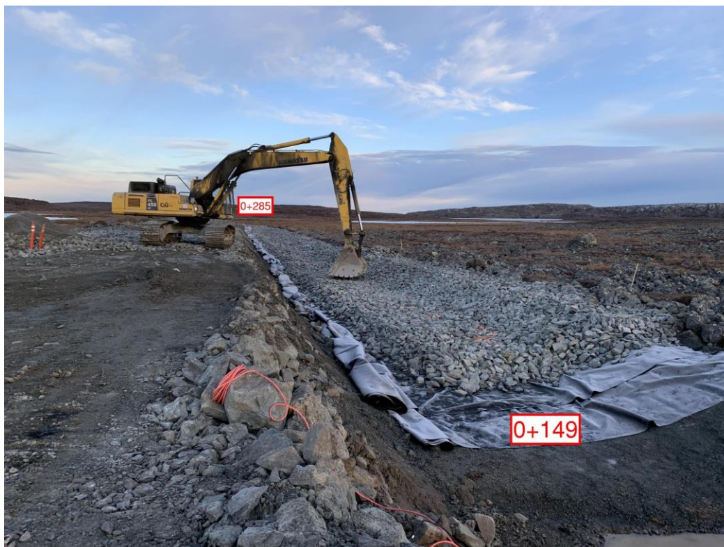
Figure 4: Global view of the geotextile between 0+149 and 0+285
