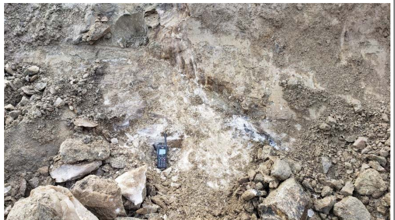
Photo 3: hammering of the frozen till to reach proper material in ice-rich sector 0+125 to 0+090, taken from St.0+125 looking South. With depth the till had gotten more ice-rich than at surface, ice lenses appeared in foundation (right). Excavation was stopped as it had reached maximum depth allowed for safety and was covered by fine esker material. Results of the water content of 3 till samples taken from that section, 20 (planned elevation), 24 and 25% (bottom of excavation), gradation on materials ongoing.
