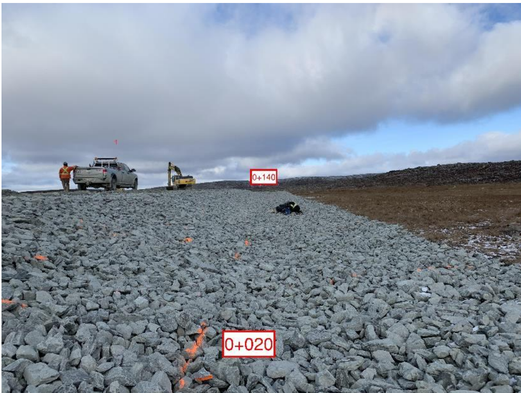
Figure 4: Riprap between 0+020 and 0+140
