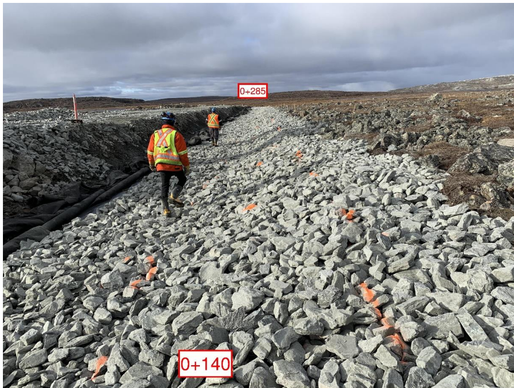
Figure 4: Riprap between 0+140 and 0+285
