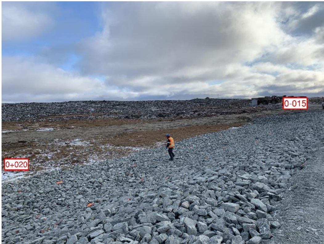
Figure 3: Riprap between 0-015 and 0+020
