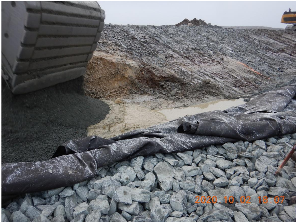
Photo 7. Fine filter placed in a way to push water further down the channel. Preliminary FF filling of the overexcavation where ice was found, STA 0+235
