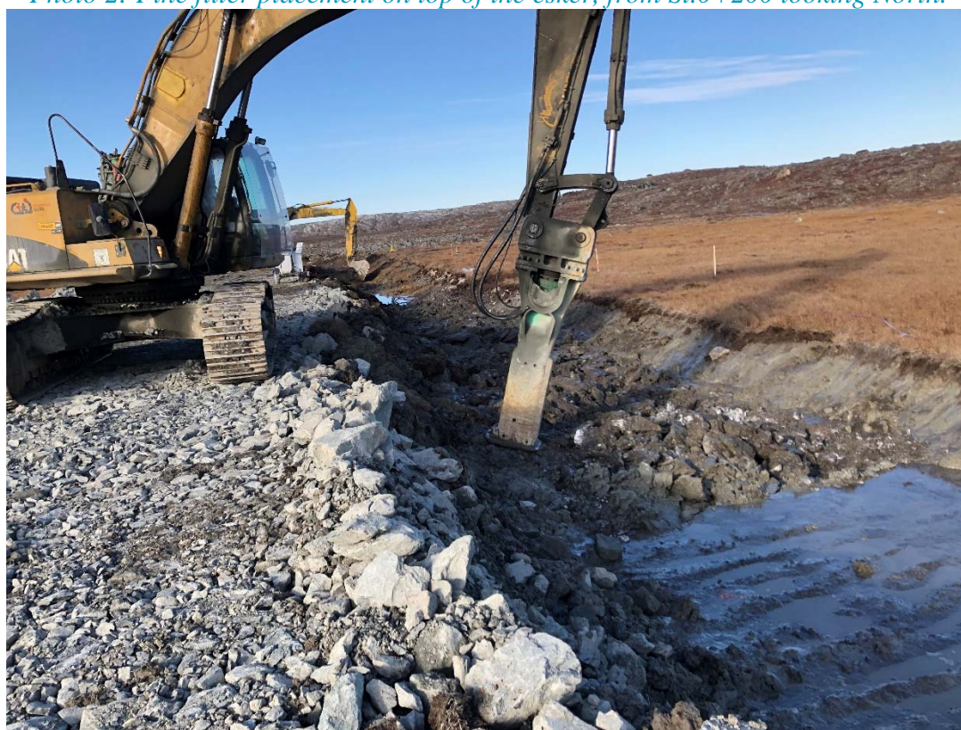
Photo 3: hammering of the frozen till to reach proper foundation grade in ice rich sector 0+125 to 0+090, taken from St.0+100 looking North.
