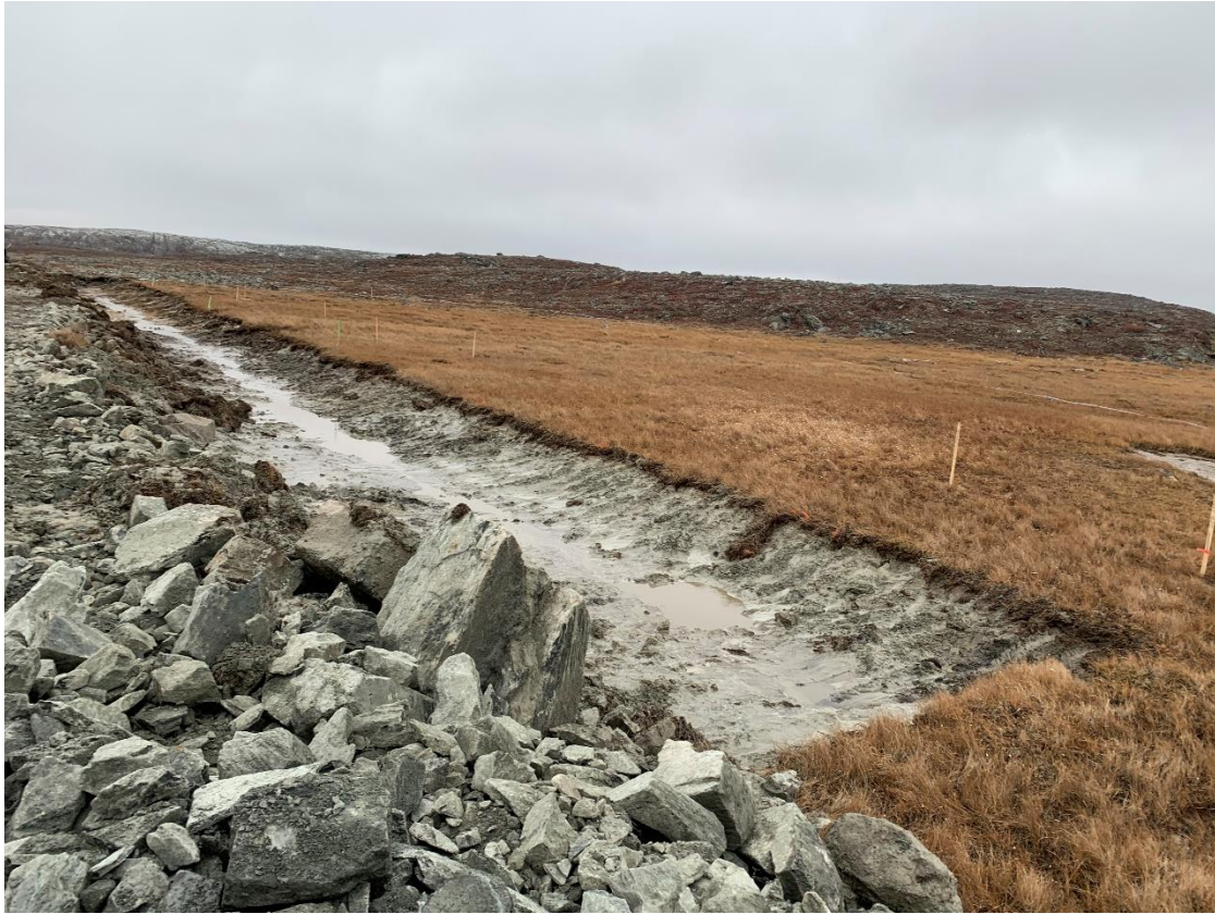
Figure 5: Preliminary excavation completed between 0+024 and 0+035
