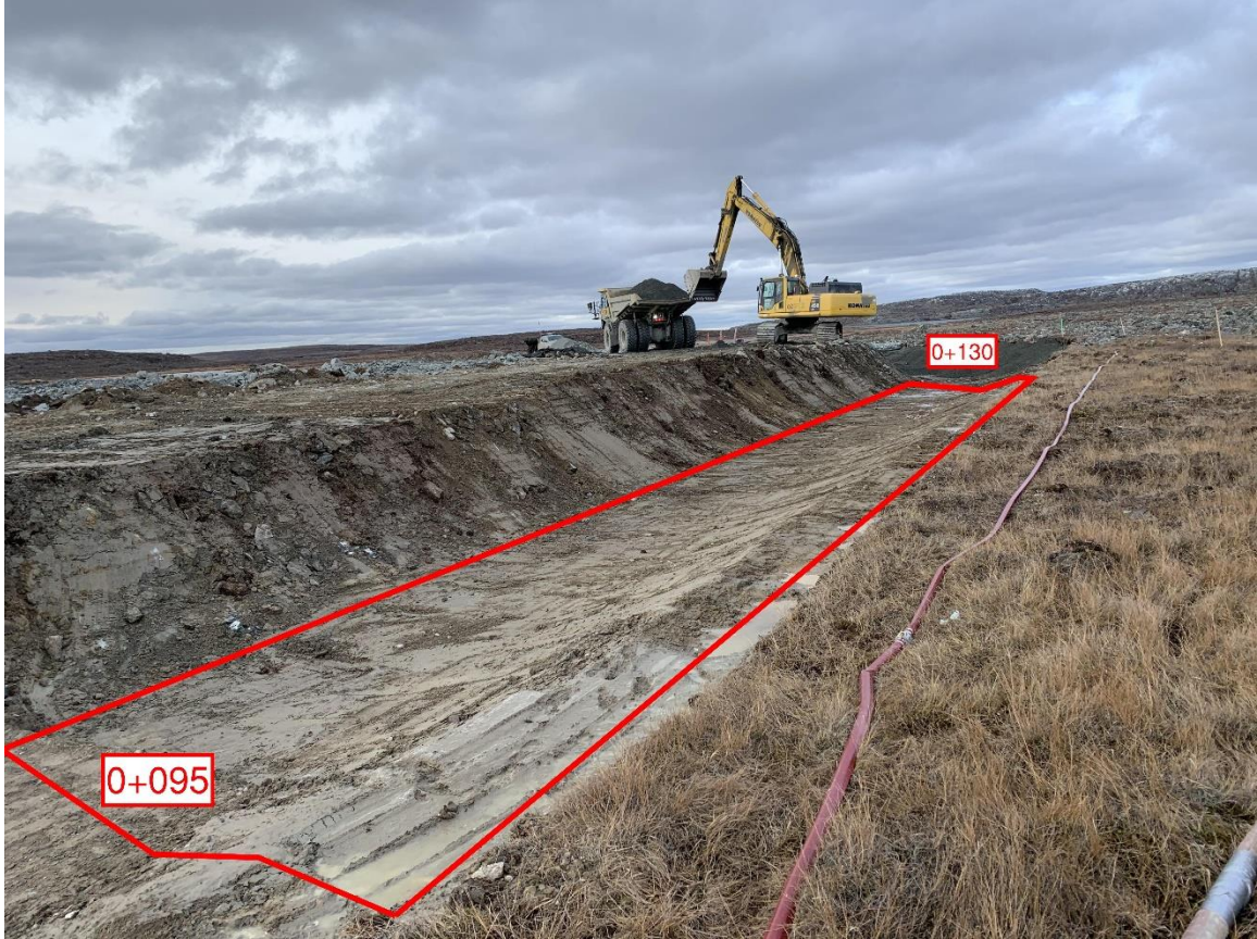
Figure 3: Foundation approval, different point of view
