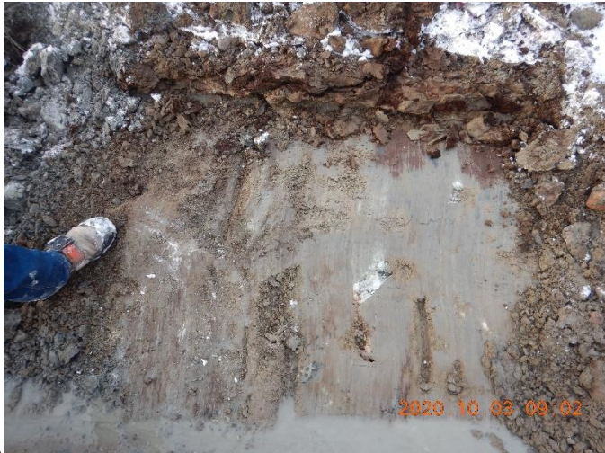
Photo 3. Foundation spot check STA 0+250, about 0.3m below grade. some ice visible at mm scale. Sample taken to confirm ice content.
