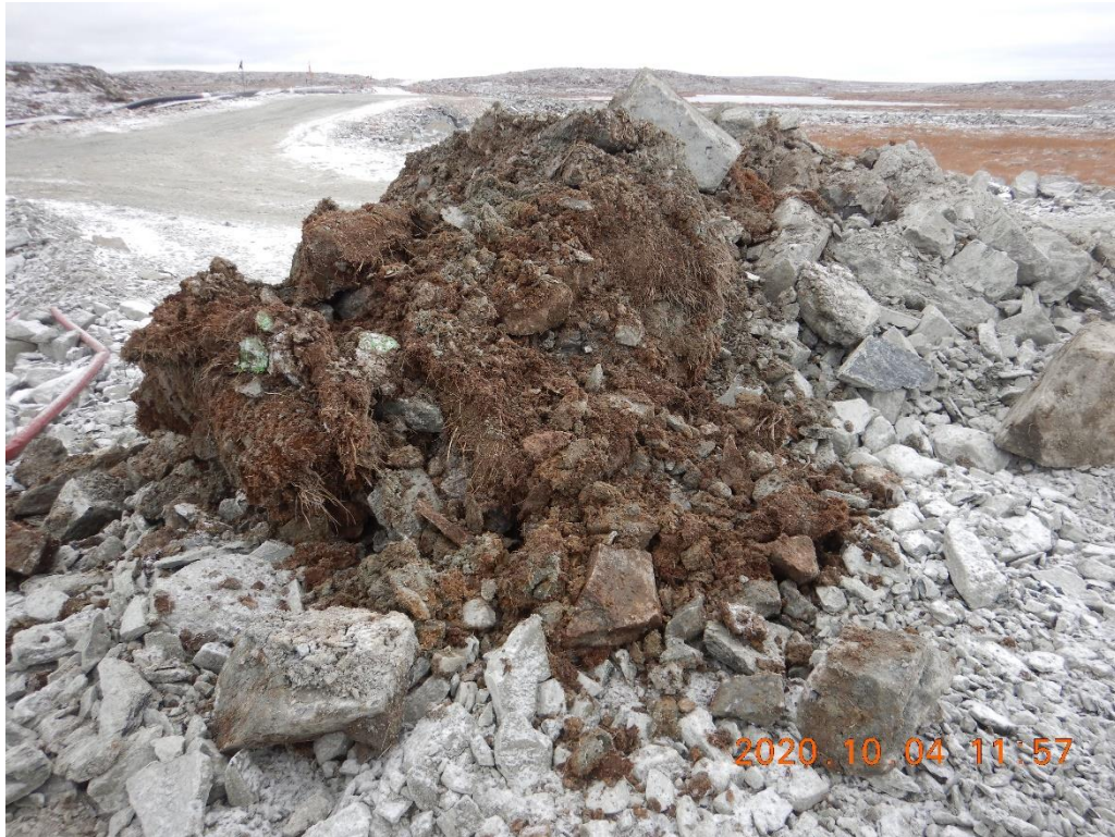
Photo 2. Organic matter removed from the foundation (west slope between 0+000 to 0+090)
