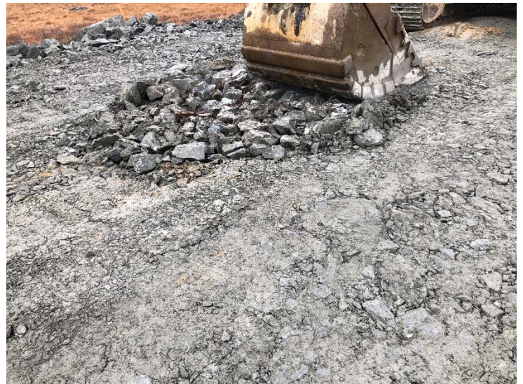
Photo 3: 1 of the 3 soft spots in the platform at St.0+225, overburden protruding through the rockfill. Soft materials were excavated and replaced with muck and compacted with the bucket of the excavator.
