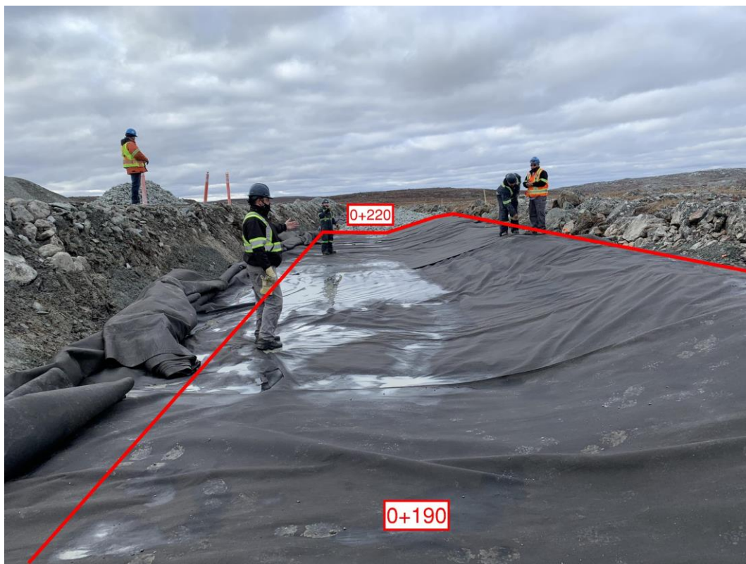
Figure 3: Geotextile between 0+190 and 0+220
