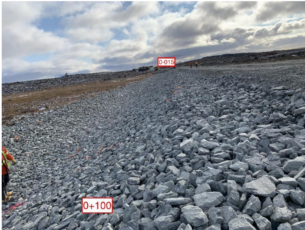
Figure 5: Riprap between 0-015 and 0+100
