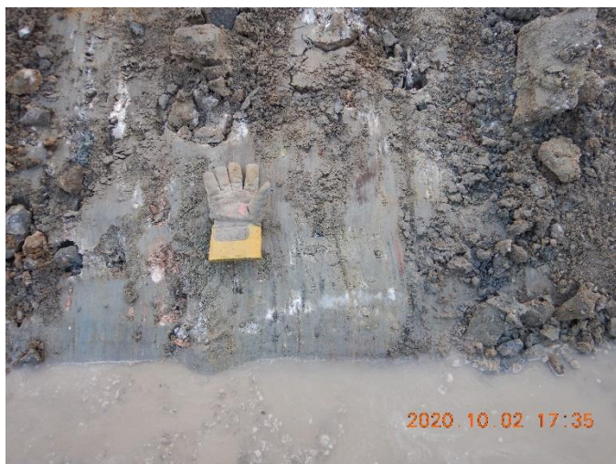
Photo 5. Ice lenses (A), ice pockets and ice rich material (B) observed between 0+230 and 0+240. All this material has been removed.
