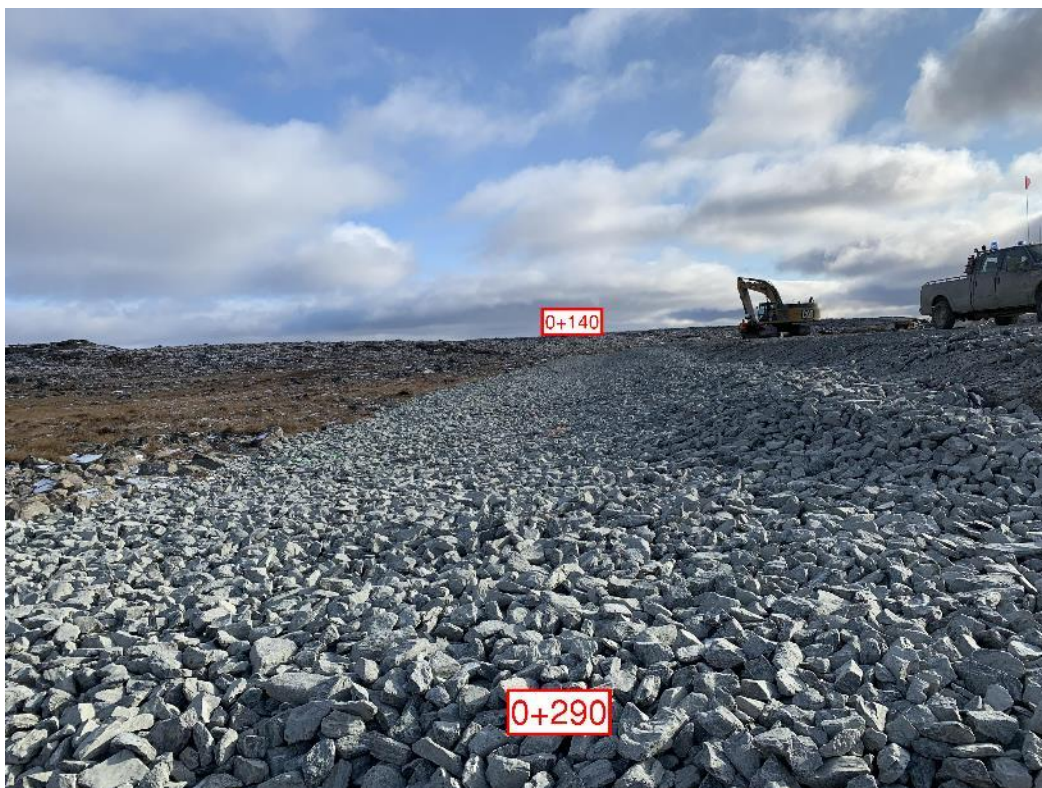
Figure 8: Riprap between 0+140 and 0+290
