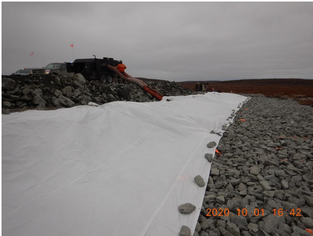
Photo 5. Tarps and frost-fighter installed at the downstream end of the channel to keep water and geotextile rolls above the freezing point.
