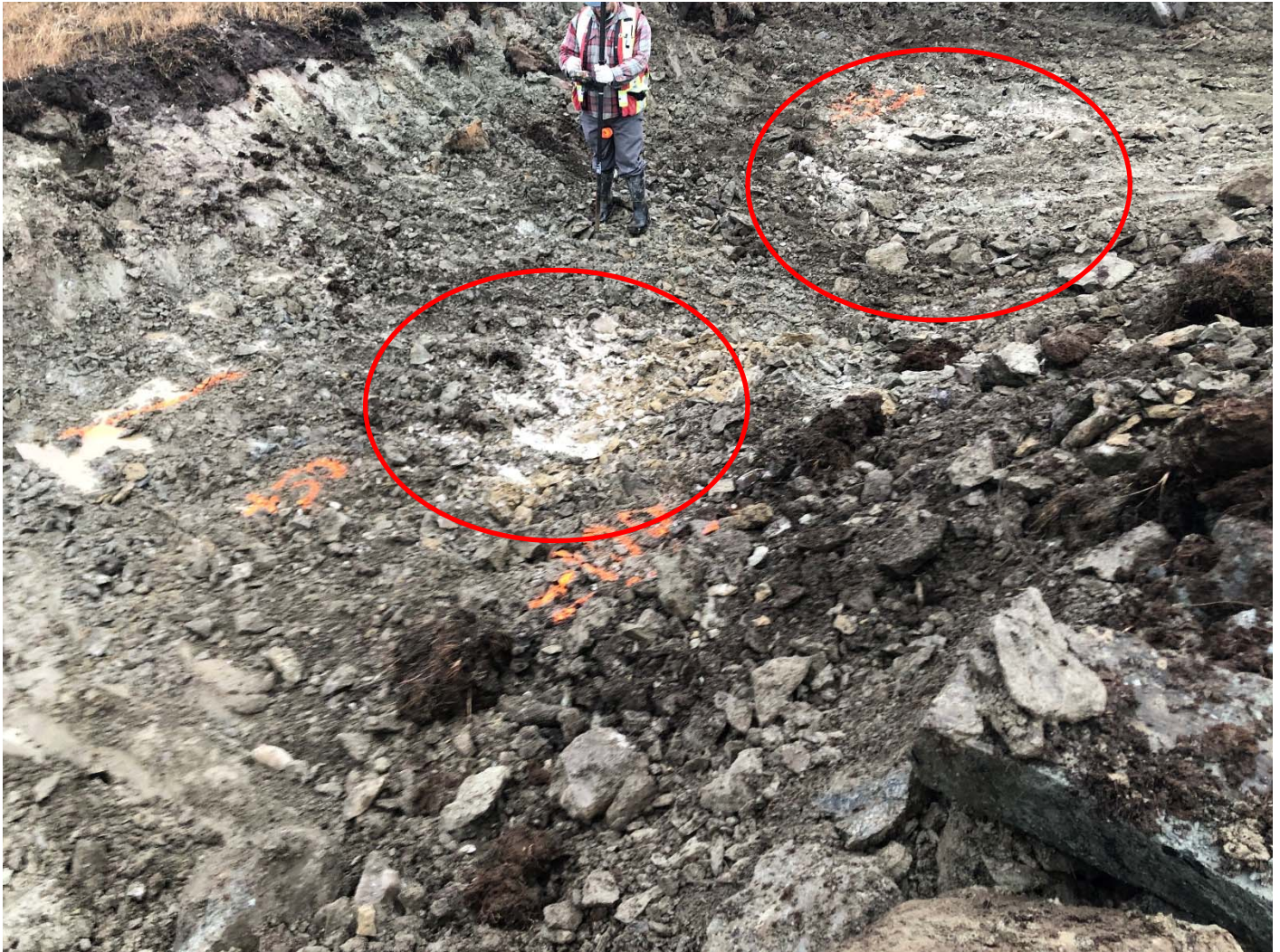
Photo 4: ice rich till in the foundation of the channel St. 0+245 looking North. Summary removal was completed without the presence of QA or QC. Ice situation will be reassessed tomorrow morning and complete removal will be performed if required, as per Specifications.
