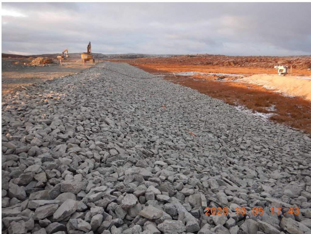
Photo 7. Finished rip rap placement, STA -0+010 looking North
