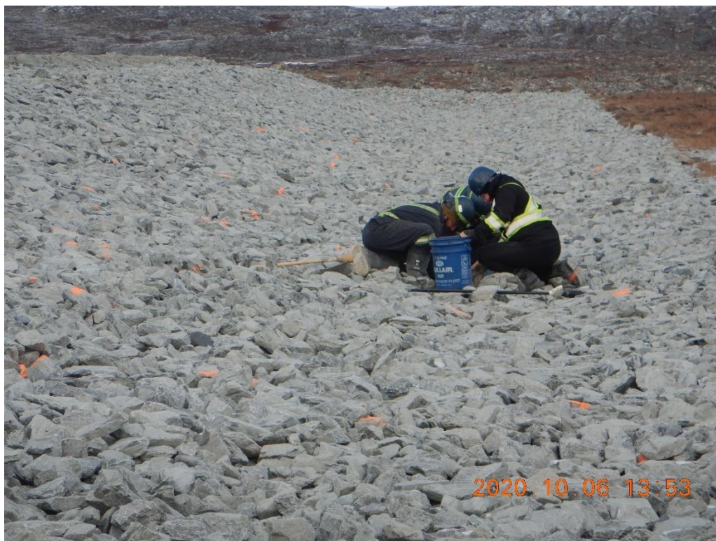
Figure 5. Rip rap fine particle cleaning by hand. A few bucket full of fines were successfully removed. STA 0+050 looking North.
