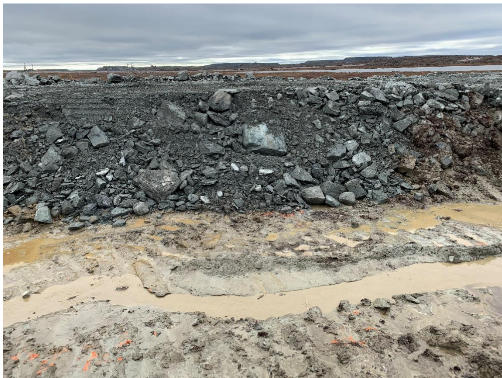
Figure 4: A ice lump has been removed and replaced by rockfill
