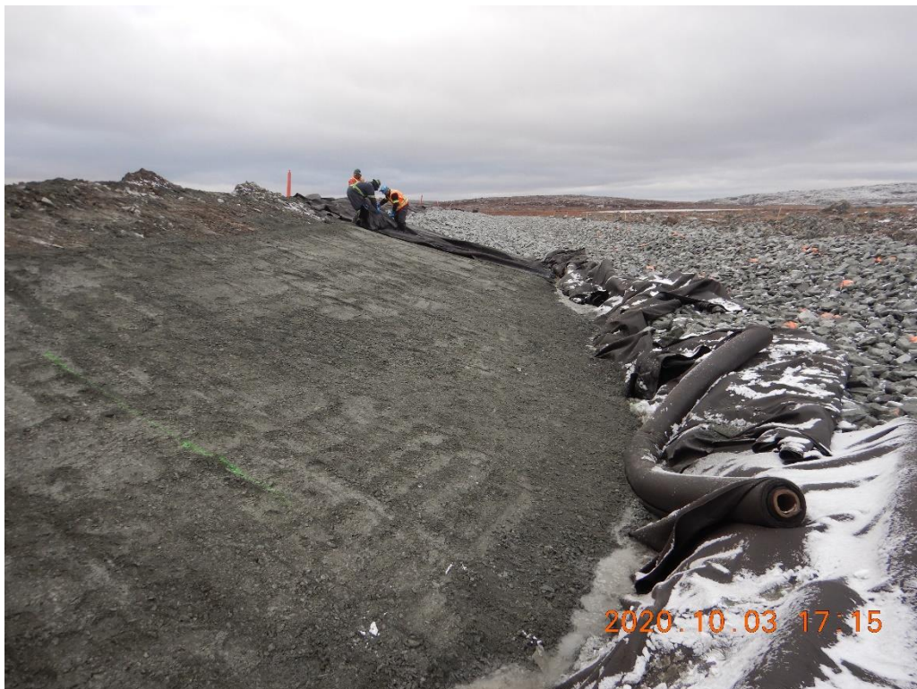
Photo 11. Geotextile being unrolled on the fine filter layer, 0+130 looking south
