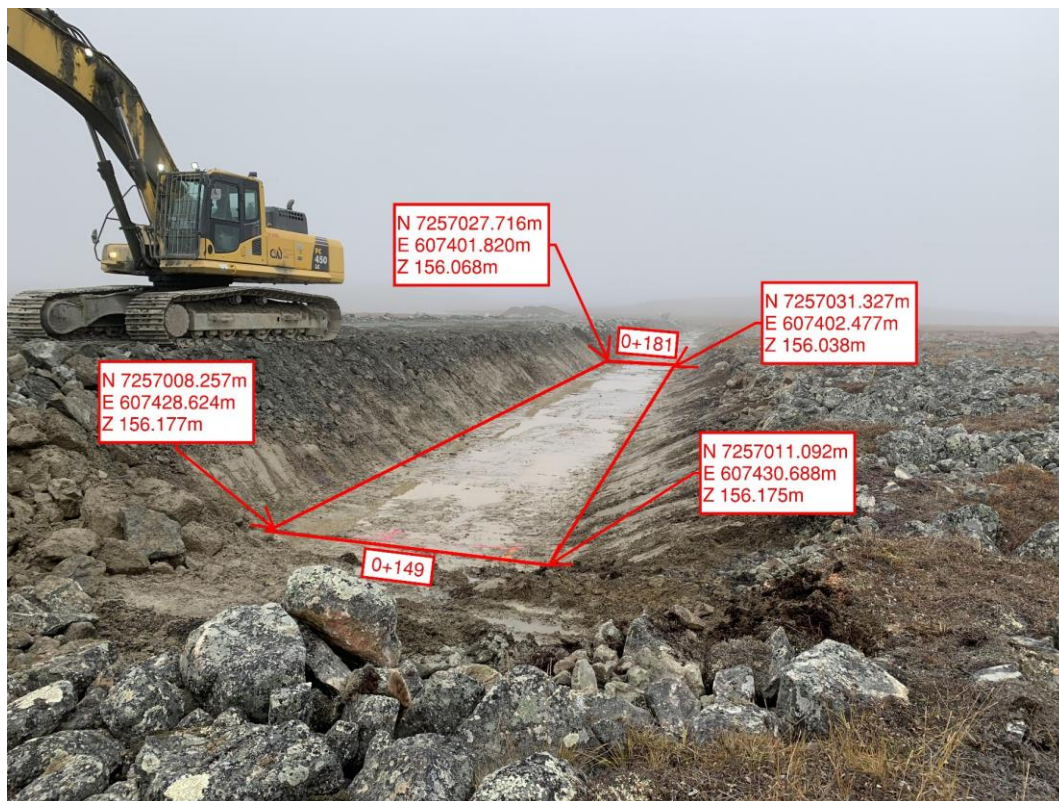
Figure 1: Foundation approval between 0+149 and 0+181
