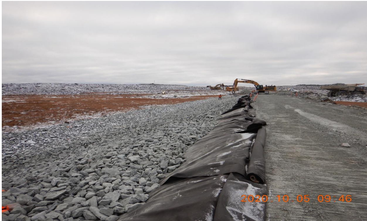
Figure 32: rip rap placement on top of geotextile in the downstream slope, St.0+100 looking South.
