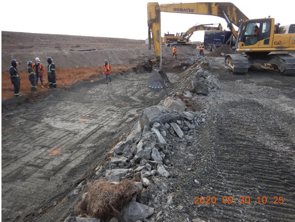
Photo 4. Completion of Fine filter material placement. Compaction with excavator bucket.
