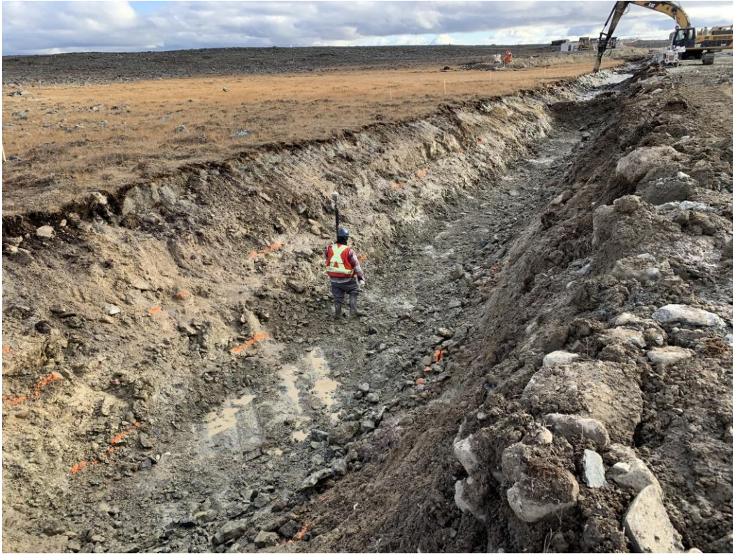
Figure 5: Ice removed (average thickness removed= 1.1m) between 0+090 and 0+125
