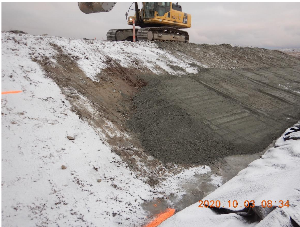
Photo 1. Fine filter placement at the downstream end of the channel. STA 0+250 looking north. Excess of snow was removed.
