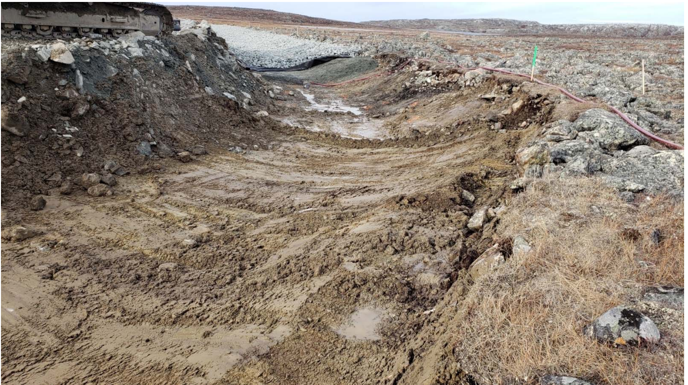
Photo 5: view of the thawed sand and gravel foundation from St.0+125 looking North to 0+150.
