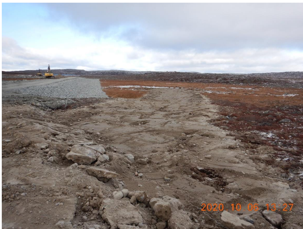
Figure 1. Temporary esker dewatering road removed
