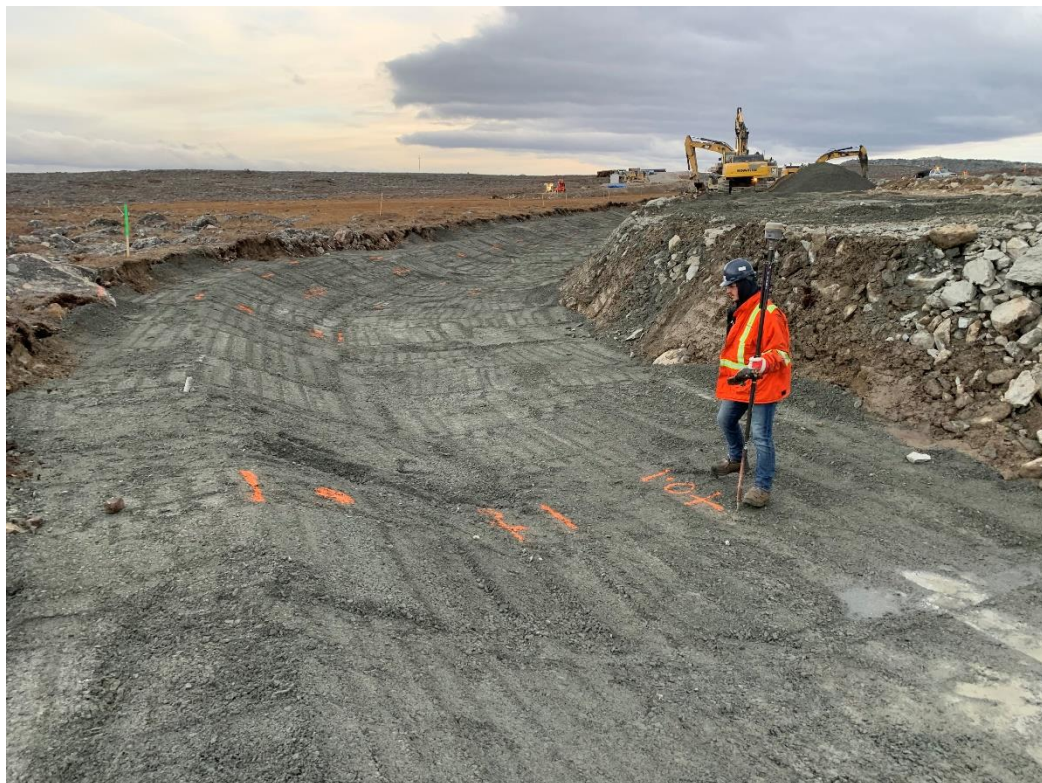
Figure 4: Fine filter fill between 0+090 and 0+149
