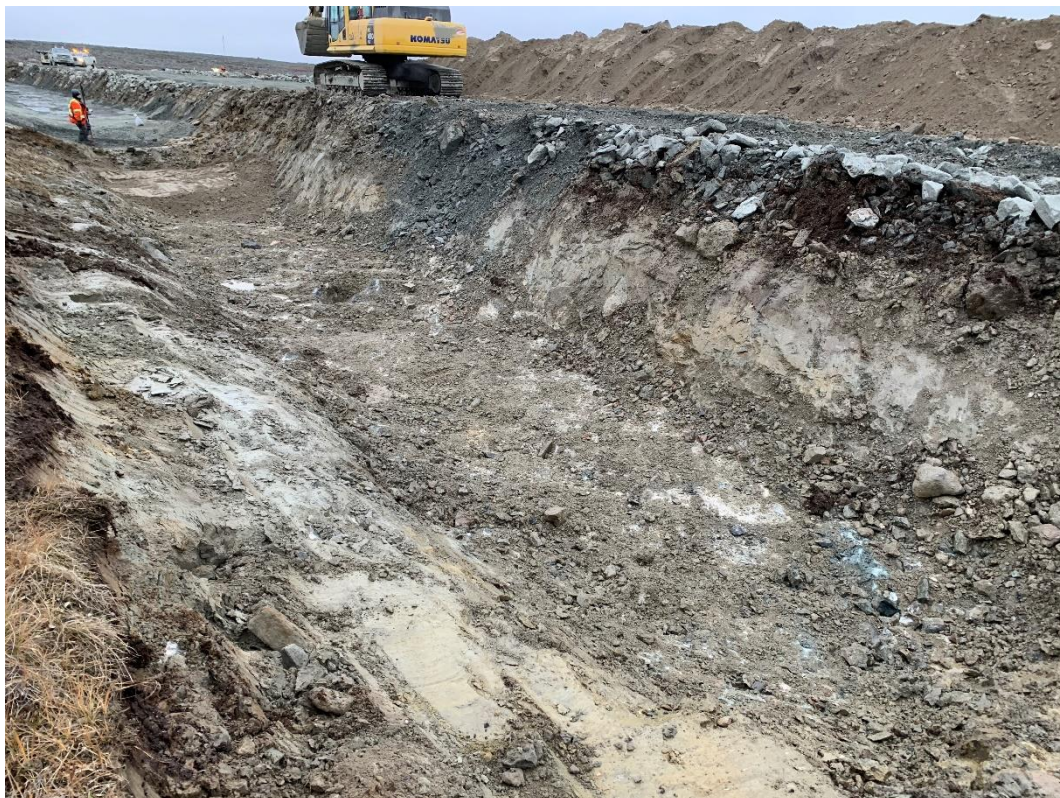
Figure 2: Ice removed between 0+235 and 0+261
