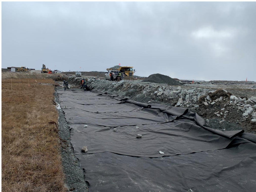
Figure 8: Geotextile between 0+029 and 0+070
