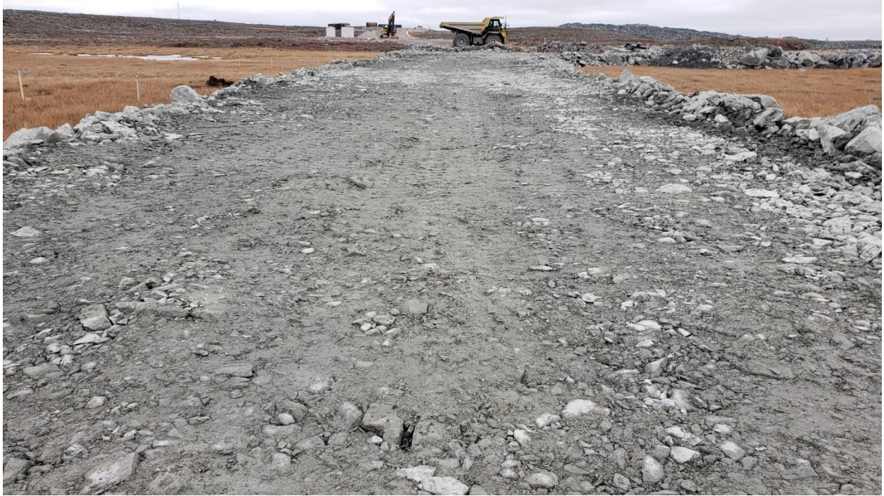
Photo 3: first lift of the downstream berm construction with ultramafic rockfill, St. 0+140 looking South.
