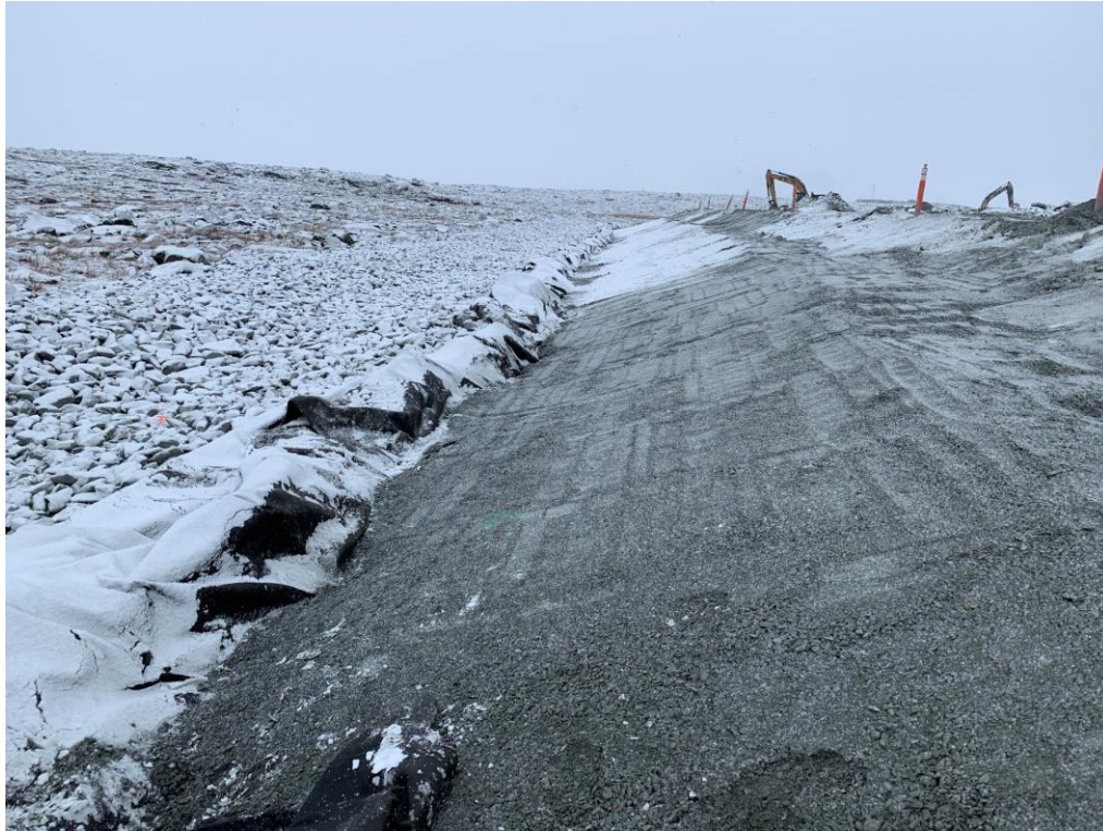
Figure 9: Fine filter approval between 0+160 and 0+220
