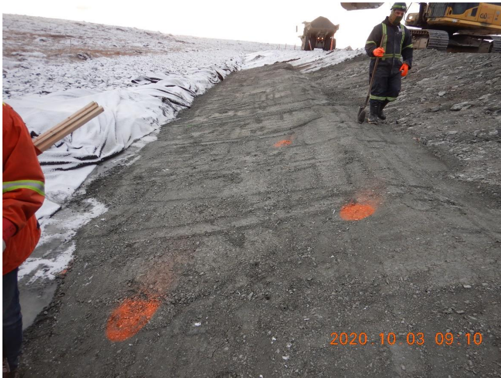
Photo 7. Fine filter layer at grade. From about 0+200, looking south
