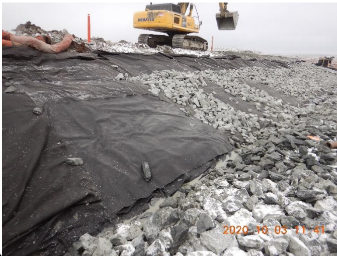
Photo 8. A) patch installed on the slope to cover the damaged geotextile. B) Close up on the damaged geotextile found the day before.
