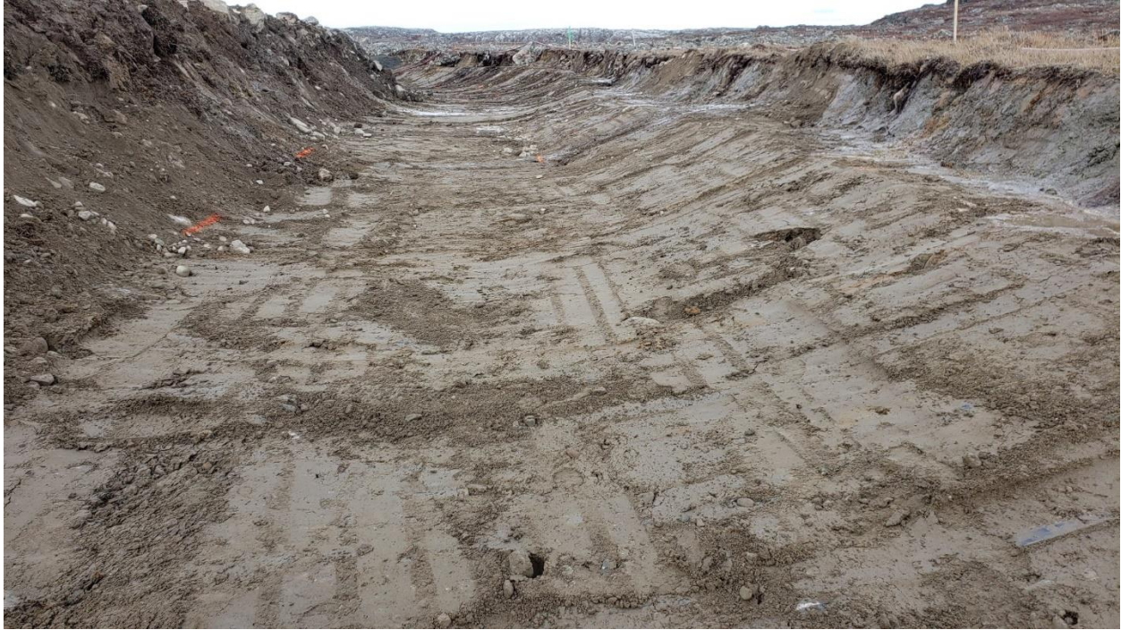
Photo 16: Approved foundation ready for the fine filter placement, St.0+090 looking North.
