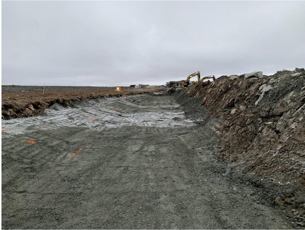
Figure 5: Fine filter approval between 0+090 and 0+149
