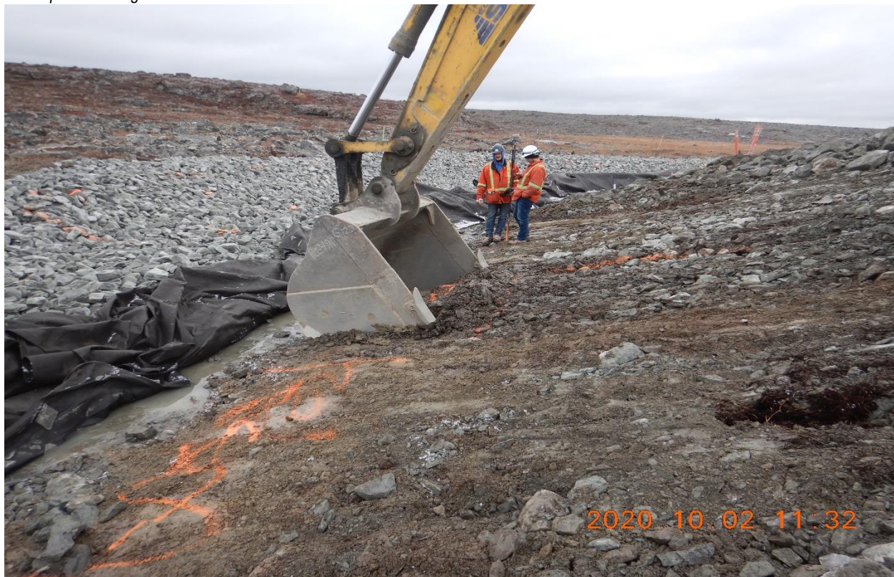
Photo 27: sloping of the downstream berm from foundation to top of platform, St.0+140 looking North-East.
