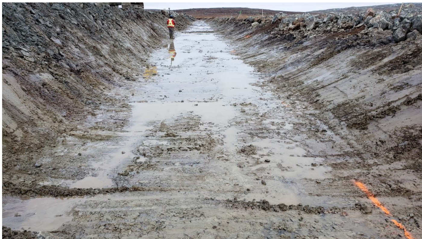
Photo 1: Foundation approved for the station 0+143 to 0+181. A final clean-up is done with the lip of the bucket then material is covered by 300mm of Fine Filter.
