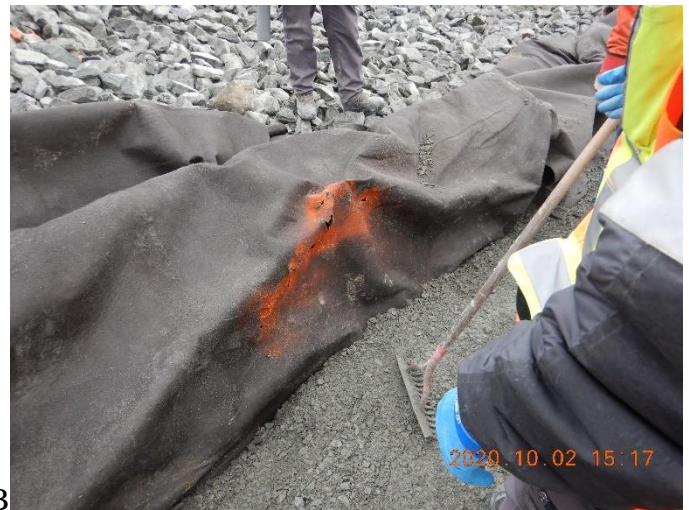
Photo 8. A) patch installed on the slope to cover the damaged geotextile. B) Close up on the damaged geotextile found the day before.
