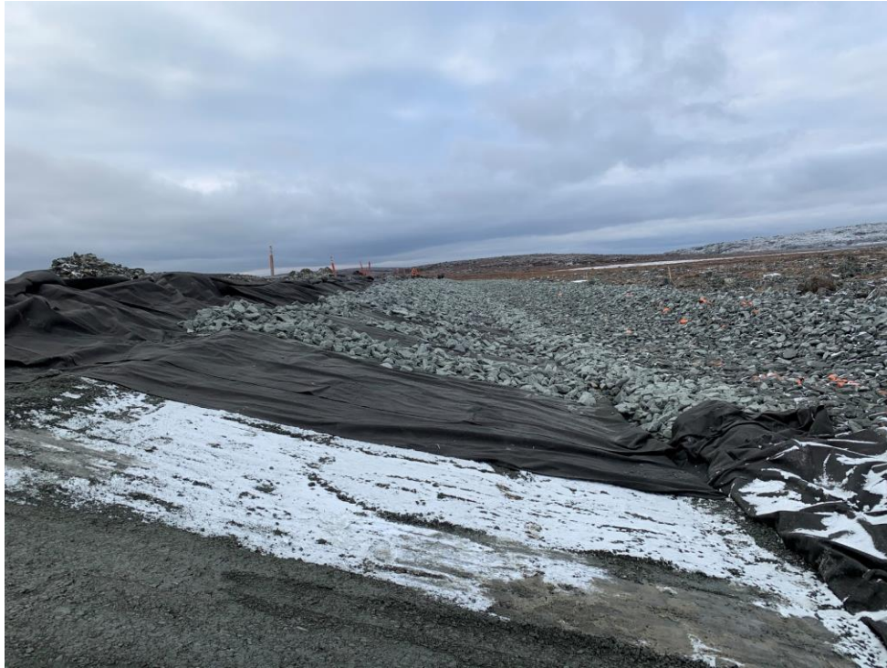
Figure 11: Geotextile and preliminary riprap between 0+160 and 0+284.5
