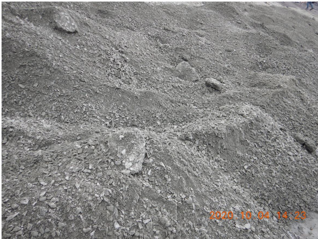
Photo 5. Fine filter with some chunks that were crushed during compaction.
