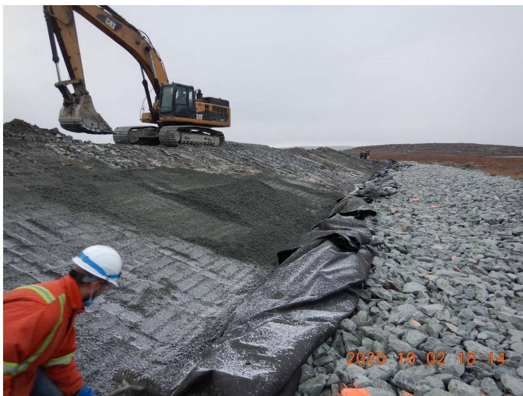
Photo 8. Fine filter placement, Looking north from around 0+225
