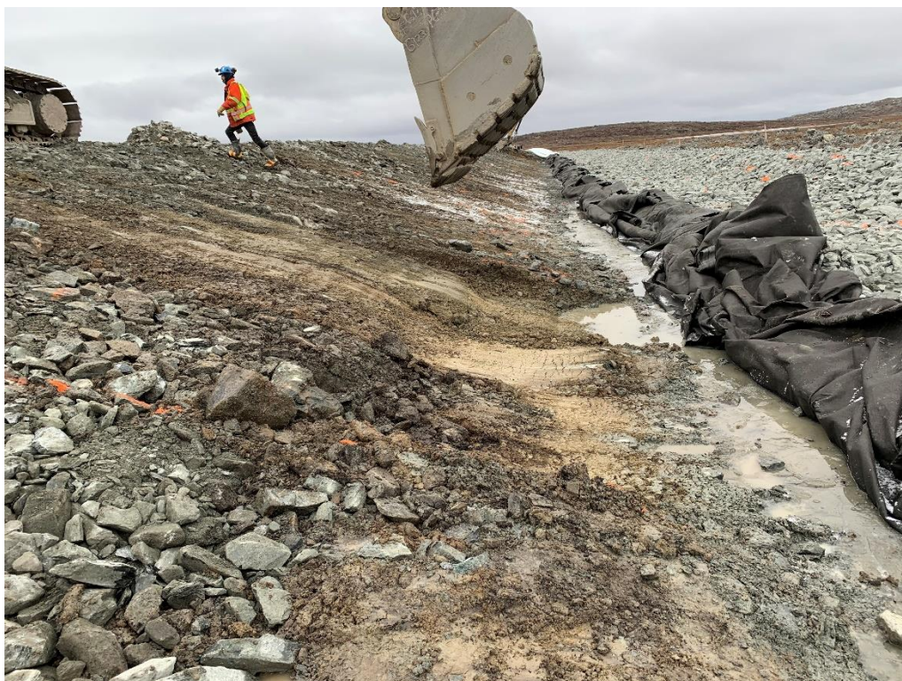
Figure 4: Soft spot excavated
