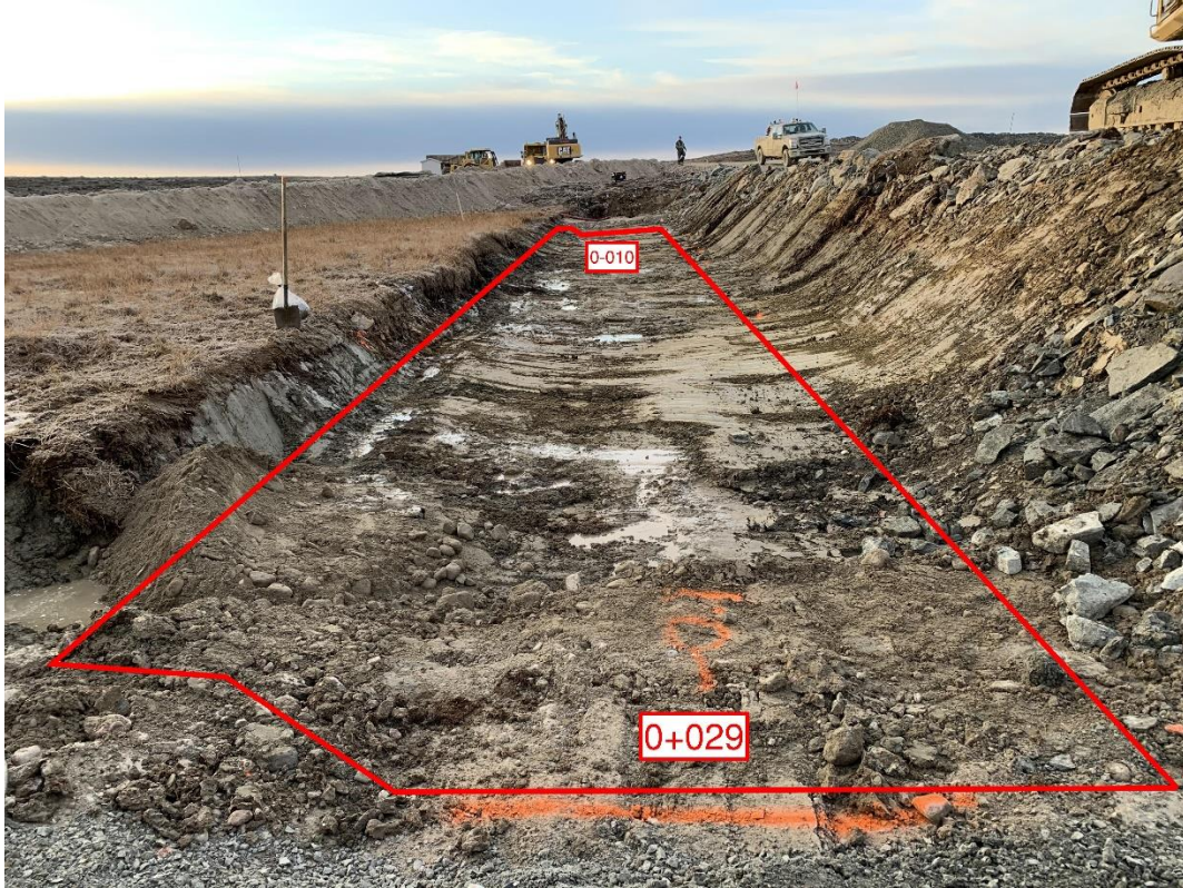
Figure 1: Foundation approval between 0-010 and 0+029
