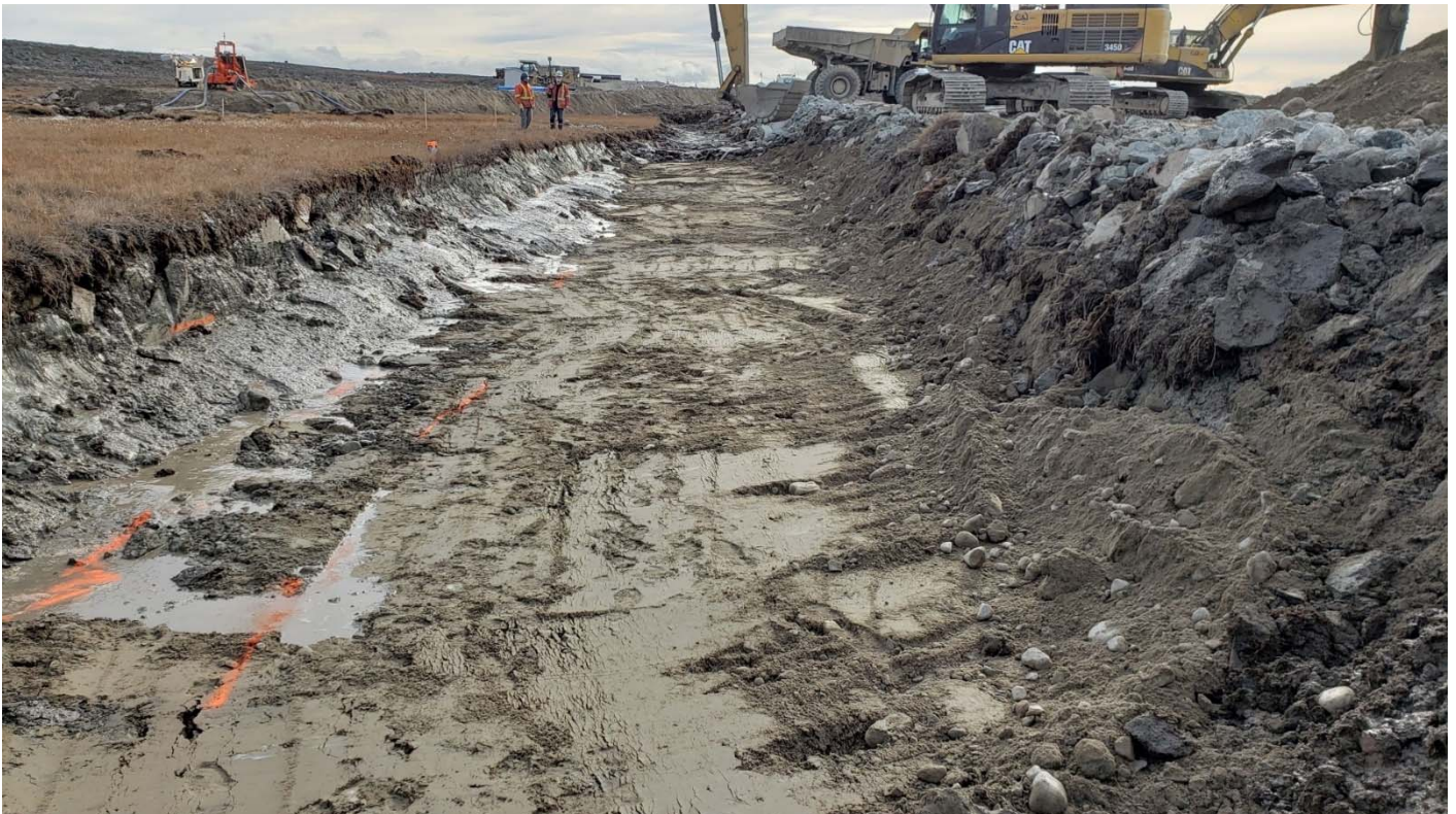
Photo 3: view of the same area after till placement, final grading ongoing.
