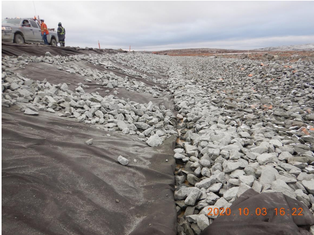
Photo 5. Rip rap placed to hold the geotextile on the west slope before completion of rip rap final layer. Visible on the photo is a fold in the geotextile at the toe of the slope, where the water within the geotextile remain frozen, because the rolls were on the invert side during sloping. Fine filter material underneath is at grade. As rip rap is placed in this zone, the geotextile levels to the top of the fine filter layer.
