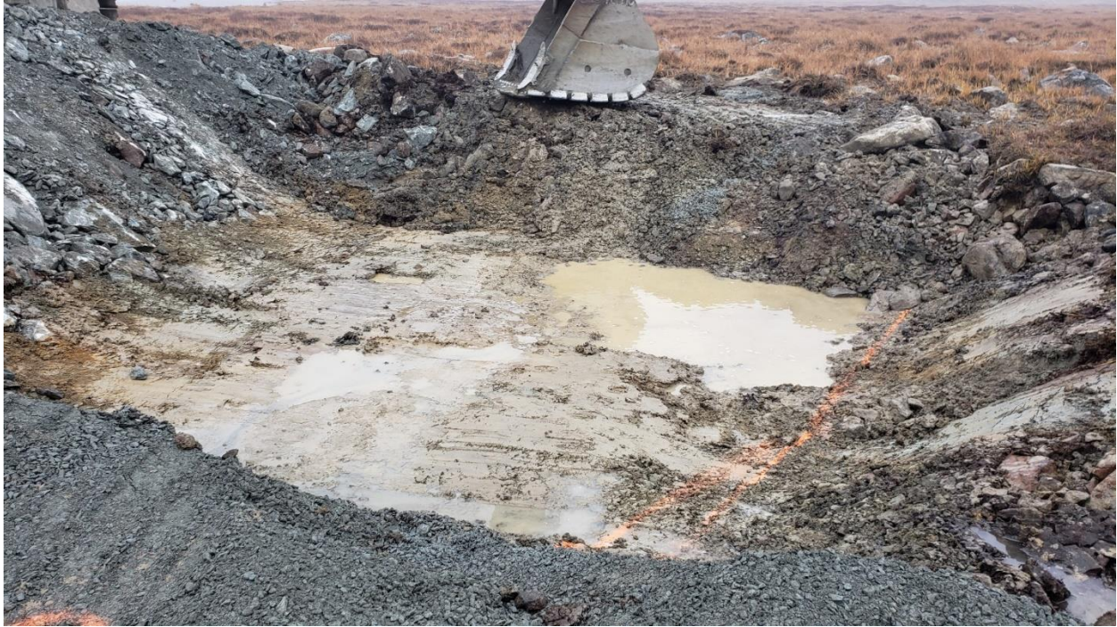
Photo 20: approved foundation of the energy dissipator following overburden excavation, looking at channel outlet.
