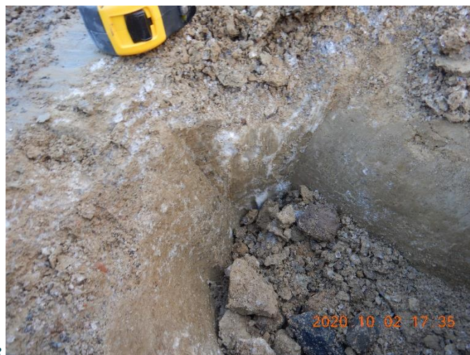
Photo 5. Ice lenses (A), ice pockets and ice rich material (B) observed between 0+230 and 0+240. All this material has been removed.
