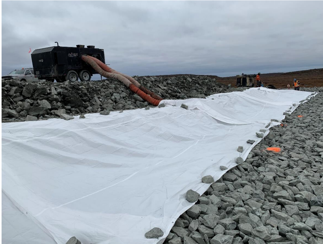
Figure 3: Heating provided between 0+235 and 0+284.5 to avoid freezing of wet geotextile
