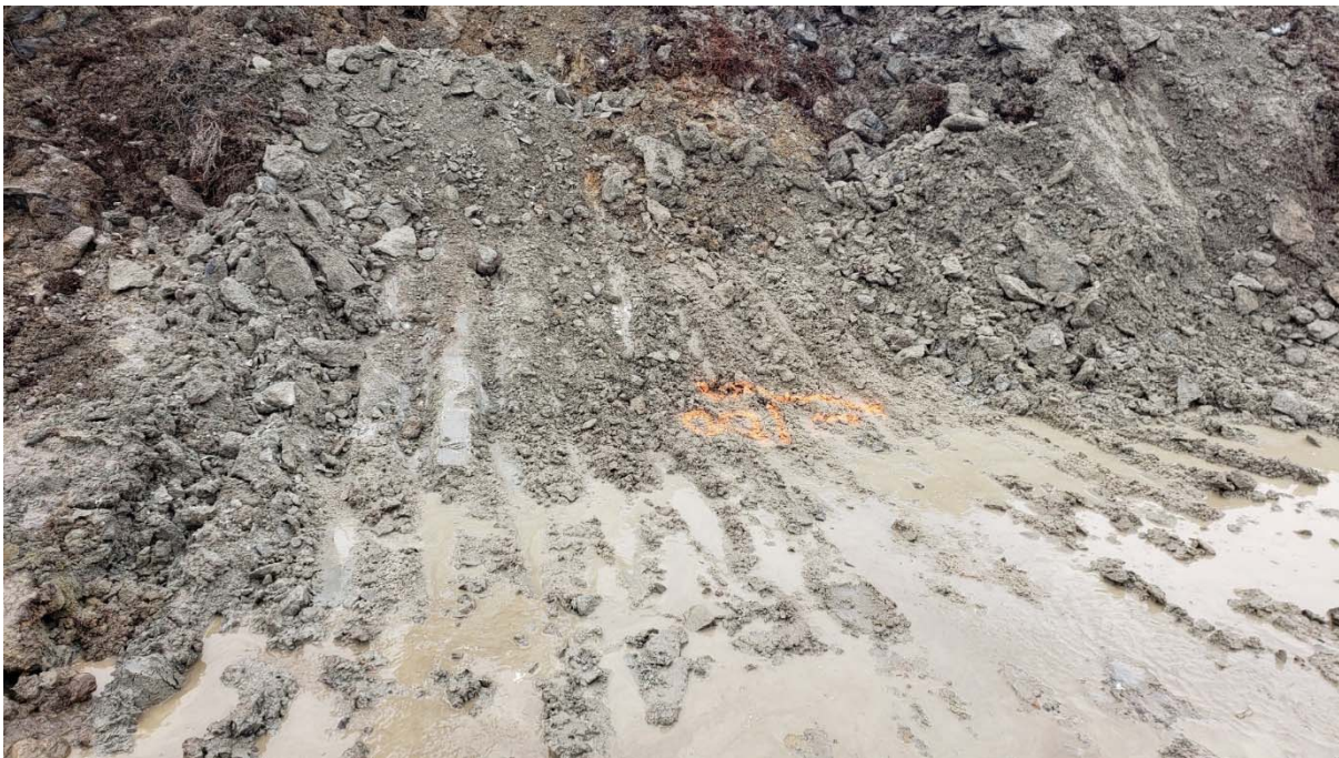
Photo 3: ice rich frozen till in the foundation of the channel between St. 0+235 and 0+260. Ice content sample revealed 93% water. Material to be excavated and replaced by esker in the next days.
