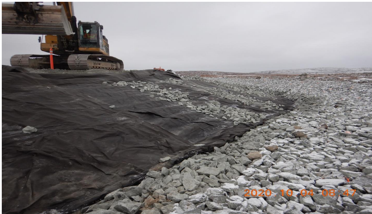
Figure 31: ballasting the approved installed geotextile with rip rap to prevent wind action, St. 0+125 looking North.
