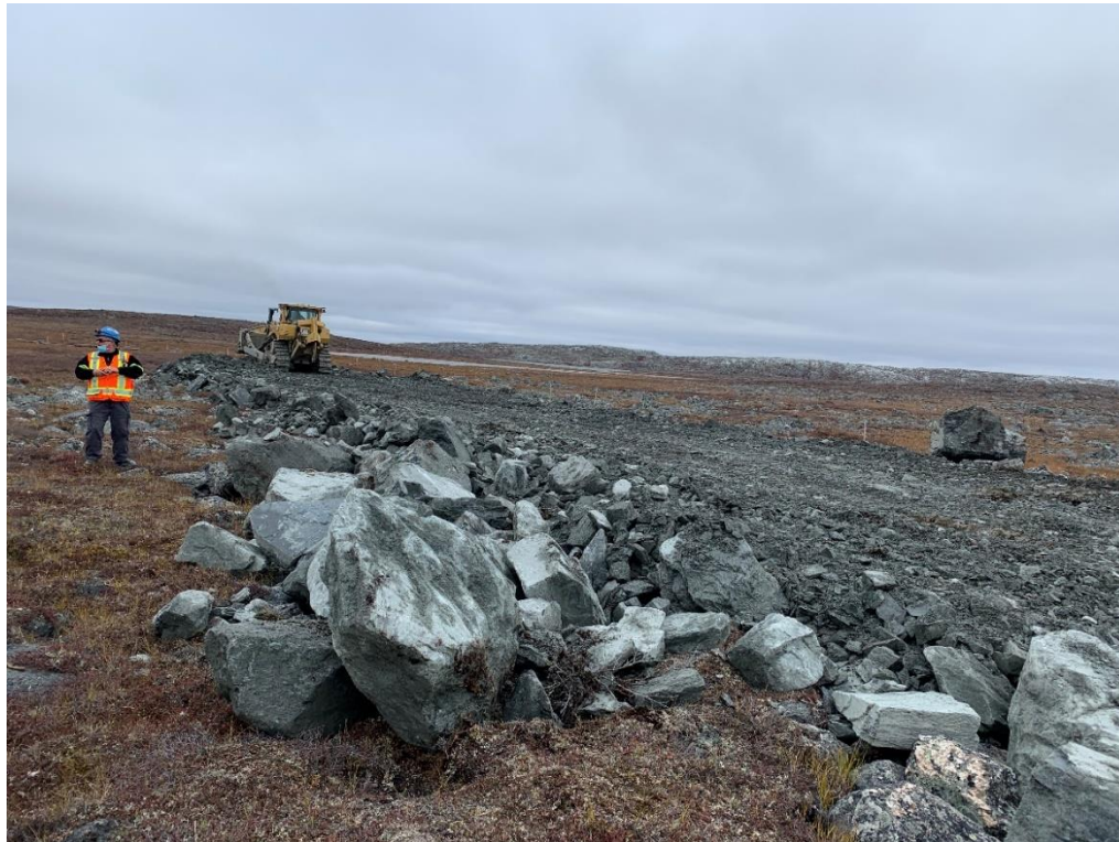
Figure 1: The larger boulders are discarded at each side of the access road
