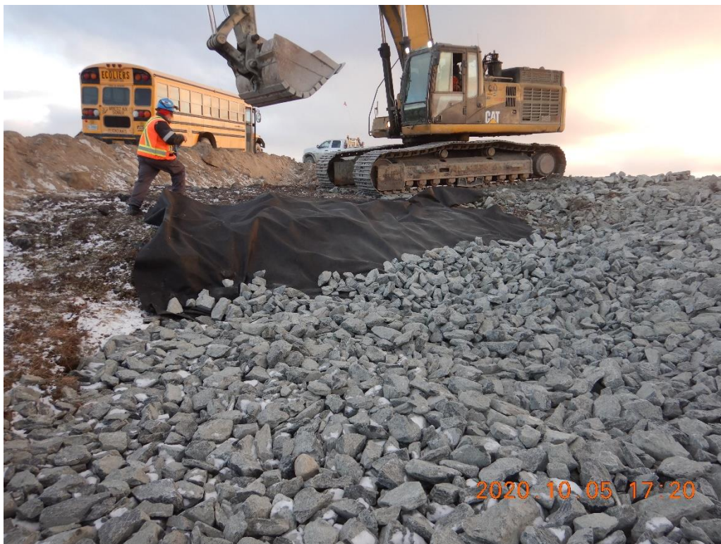
Photo 5. Geotextile placed over the natural slope at the upstream end of the channel.
