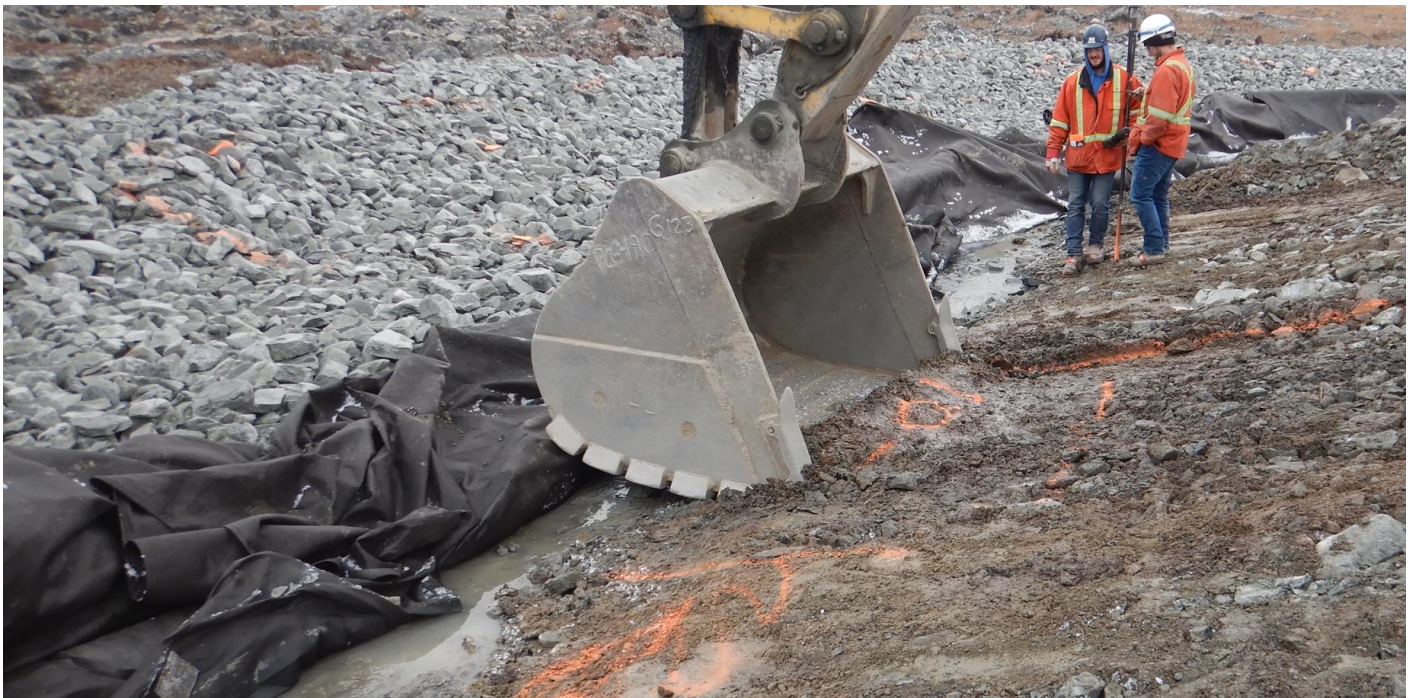
Photo 3. Soft oversaturated material starting to be removed by the excavator
