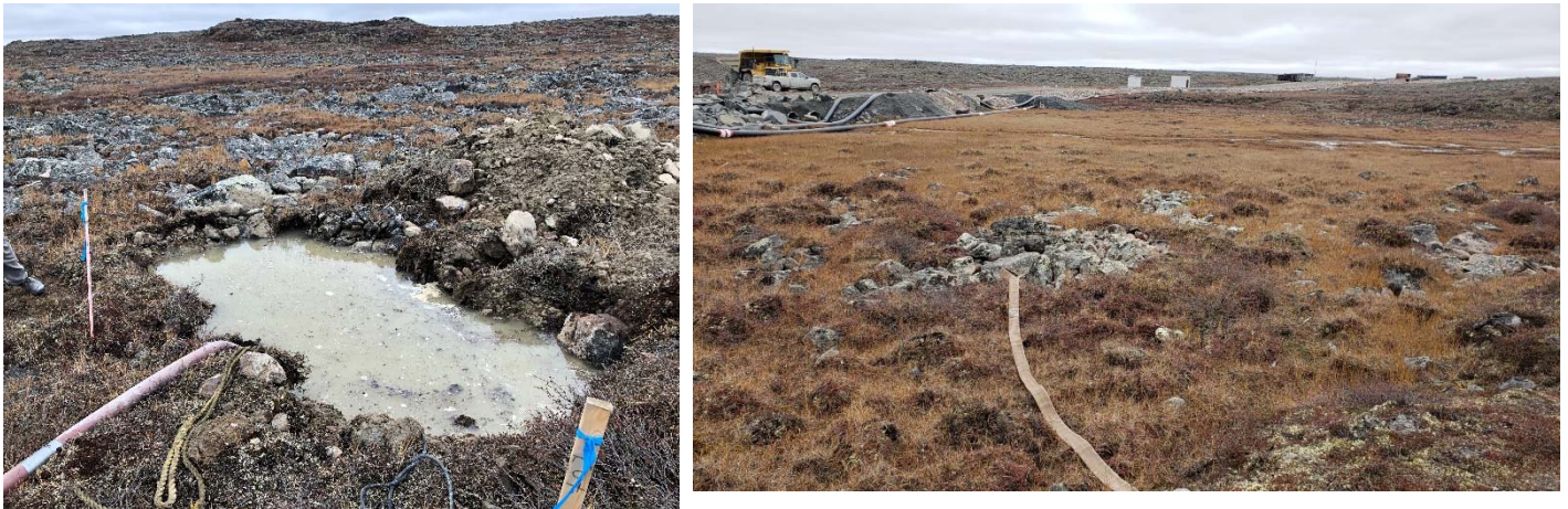
Photo 3: water management in the foundation. To drain the water contained in the boulder field to allow for a proper excavation, a sump was dug into the channel footprint and water redirected downstream of the Construction site. Pumping was effective to drain most of the boulder field after one night of continuous dewatering.
