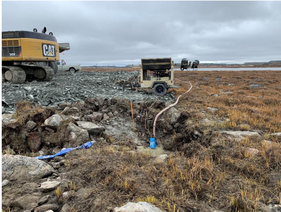
Figure 1: Sump downstream of the channel (approximately at station 0+290)
