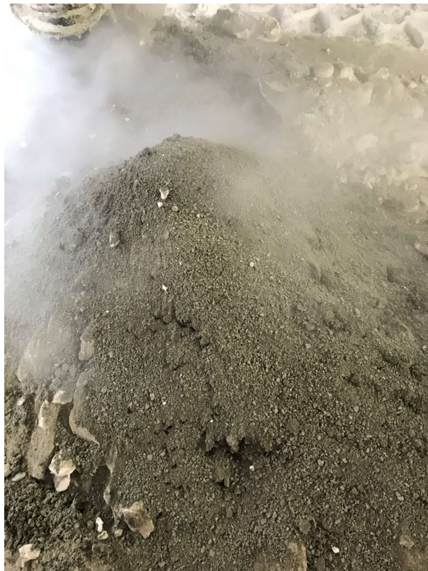
At S746.5, hole stayed dry during re-drilling of grouted hole
