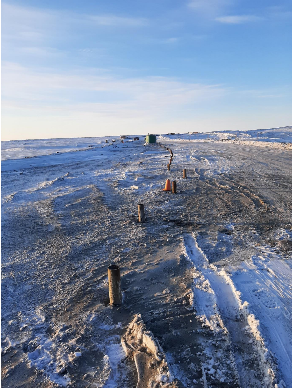
Photo4 : Installed casings, Looking west approx.from Station 425m
