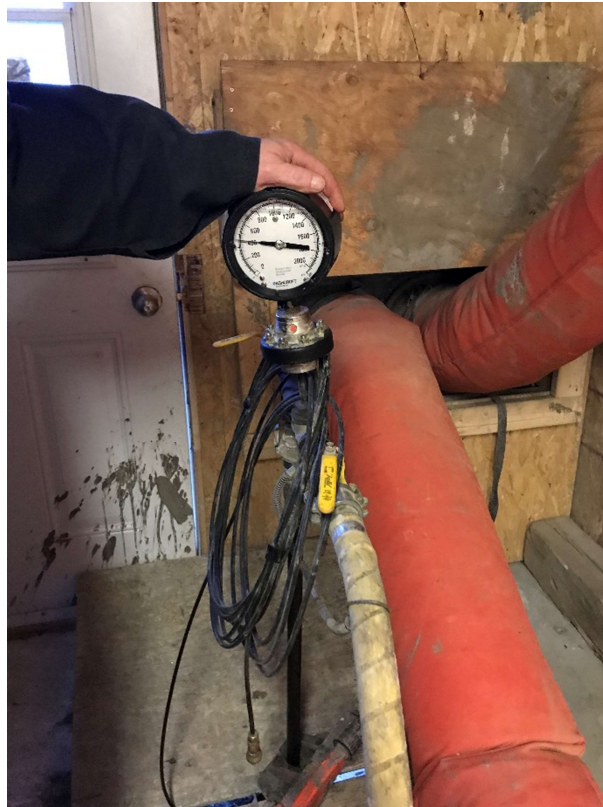
Packer installed and grouting in progress at S638.5
