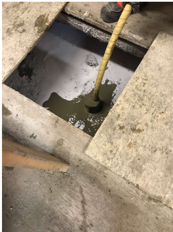
Hole backfilled after pressure refusal at T677.5
