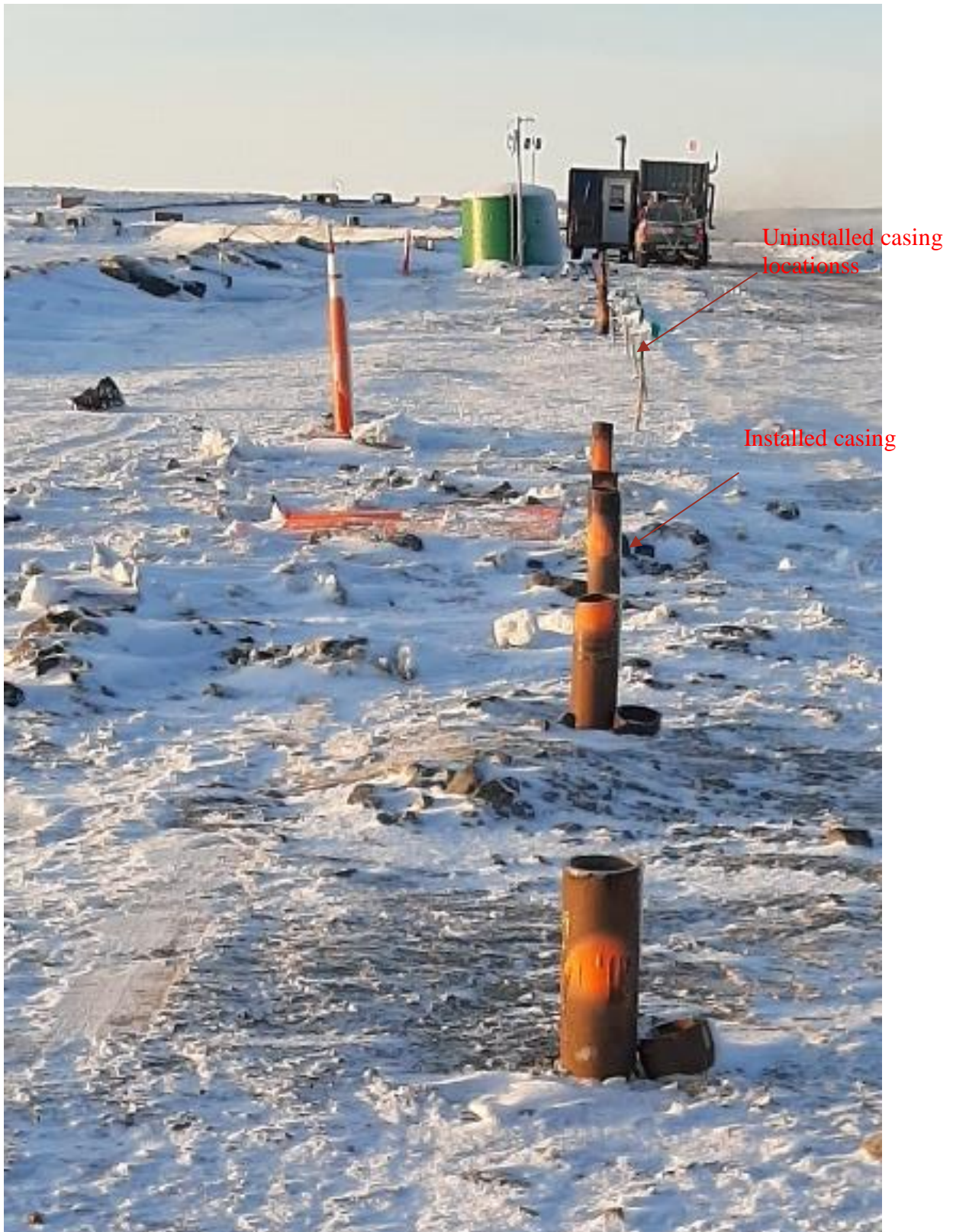
Photo1 : Looking west approx. from Station 735m, uninstalled casings (wood sticks with green flags) a little offset from the installed casings
