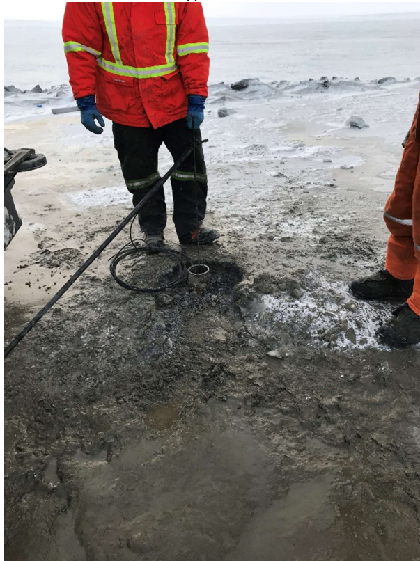
Pipe came out from packer during pulling with loader while packer still inside the hole at T719.5
