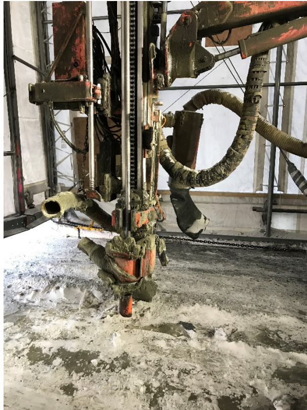
Drilling for 1.5 m into rock at S698.5
