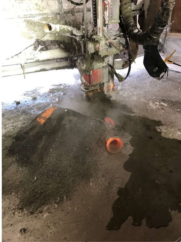
At S686.5, water encountered at 14.2 m during re-drilling of grouted hole
