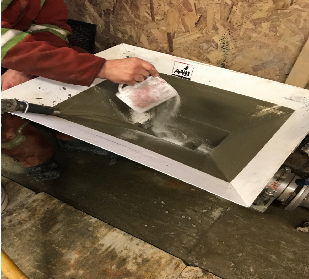
Adding Cellbex in the open throat pump
