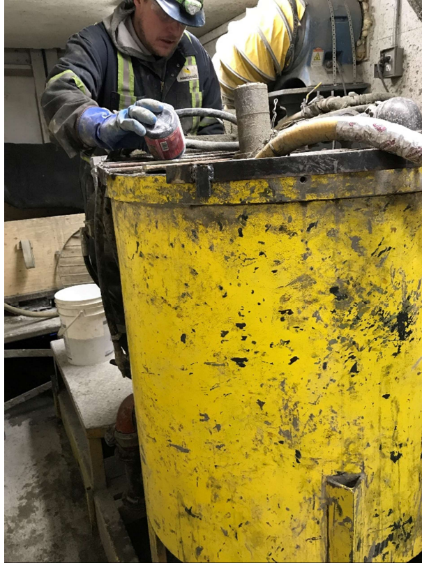
Adding celbex to the agitator tank for grout plug at T575.5
