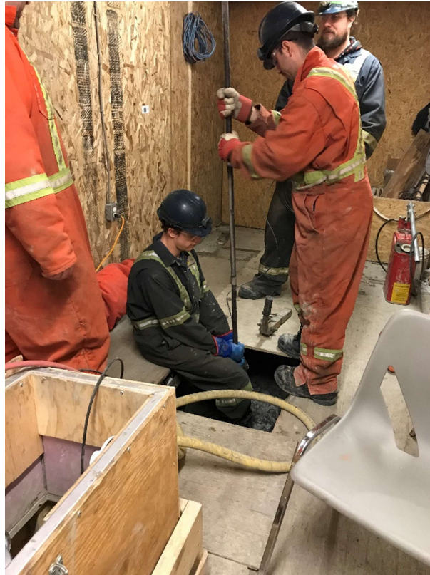
Installing Packer at S674.5
