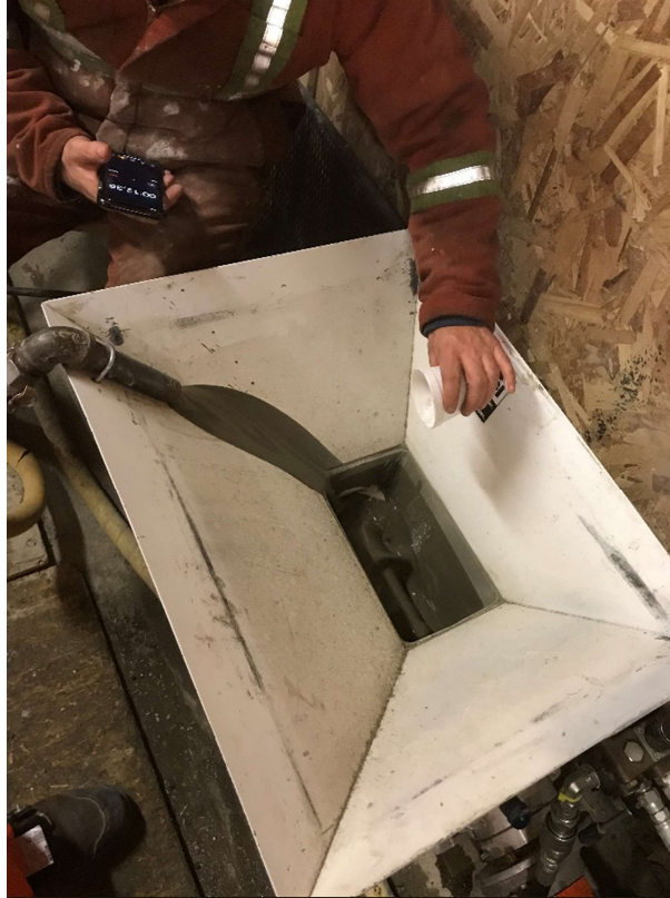
Adding celbex in open throat pump while looking at timer.
