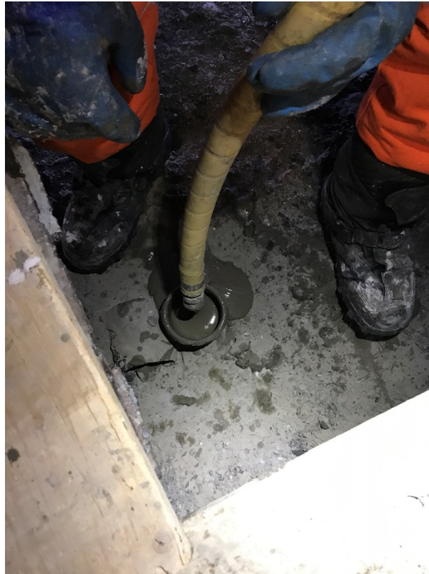
Backfilling P632.5 after re-grouting
