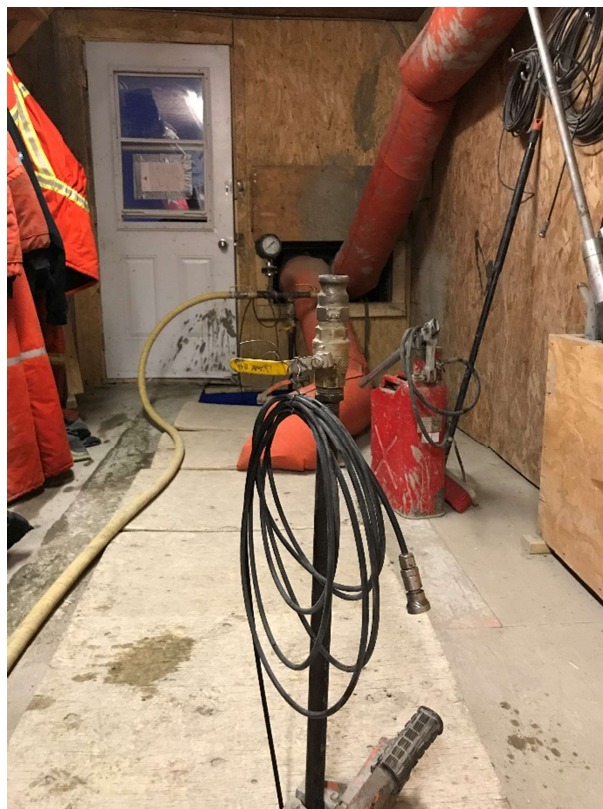
Packer placed at S626.5 while injecting at T629.5
