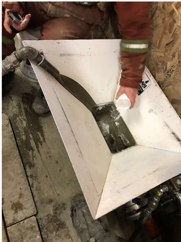
Adding Celbex through open throat pump at S746.5
