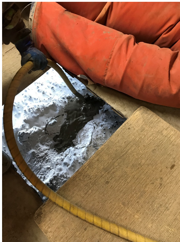
T197.5 backfilled after confirming grout elevation inside the casing
