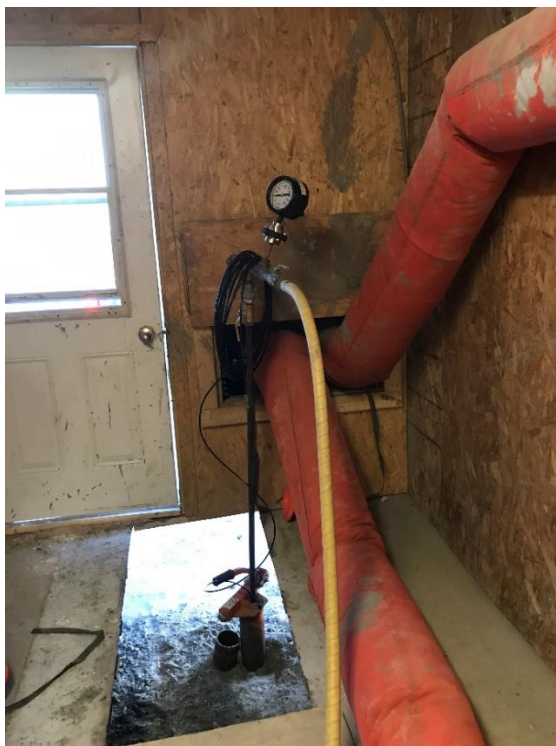
Photo2: Packer installed at T-749.5
