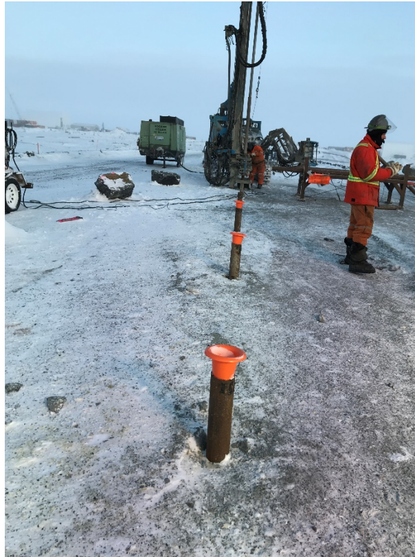
Figure 1: A photograph of the casing installation for downstream blanket
