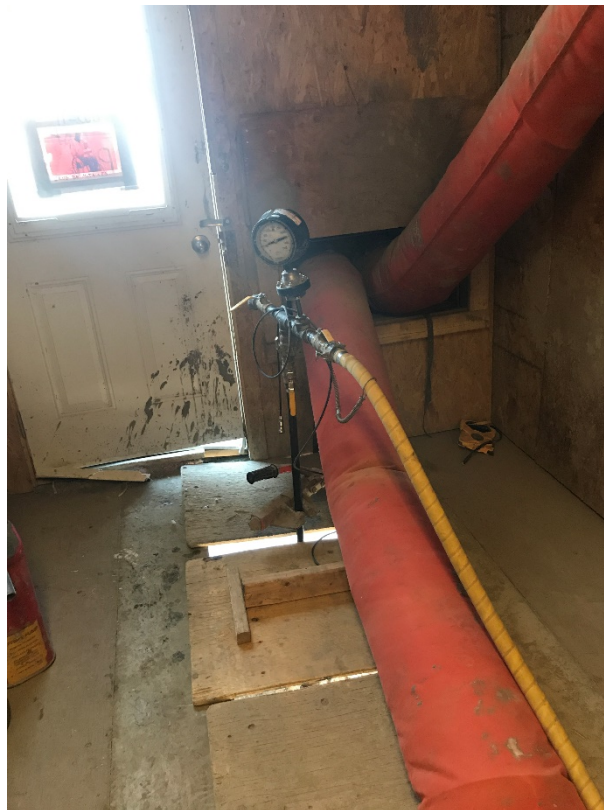
Packer installed at P368.5
