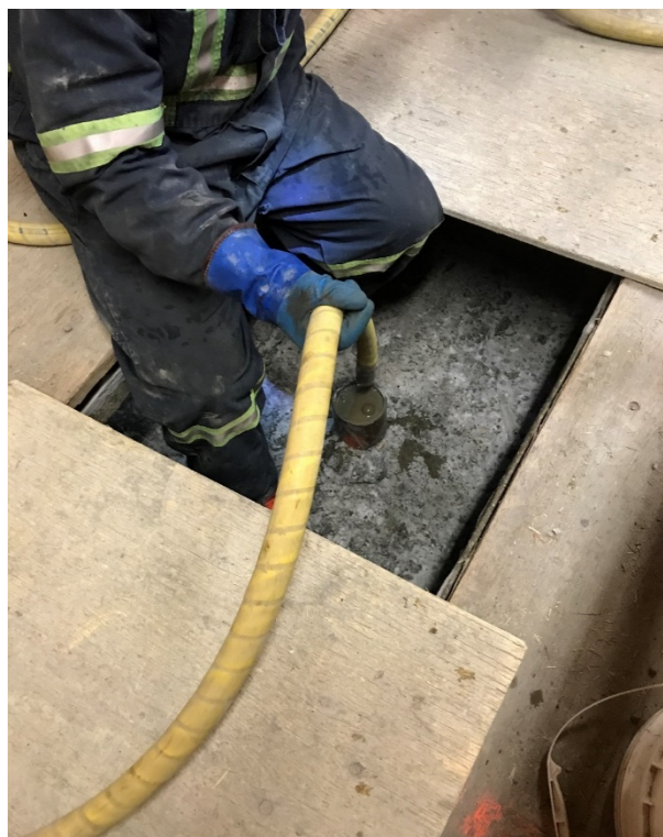
Photo 23: Backfilling hole after pressure grouting completed
