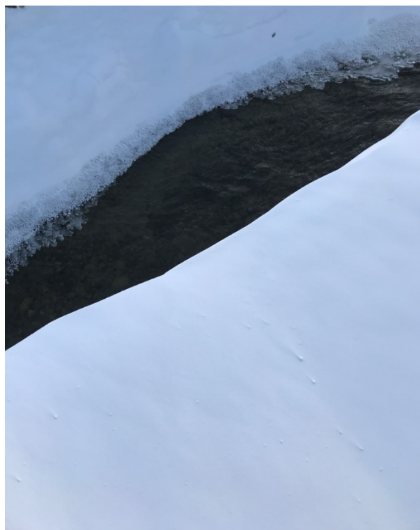
Photo 7: Seepage collection trench along downstream toe of dike
