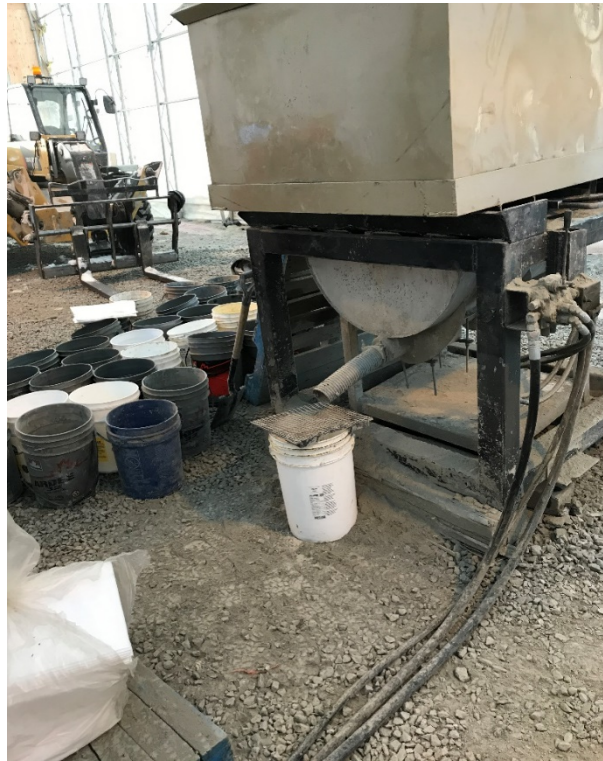
Photo 6: Cement screening and placing into 20 kg bucket
