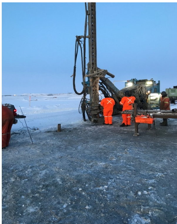
Photo 15: Casing Installation
