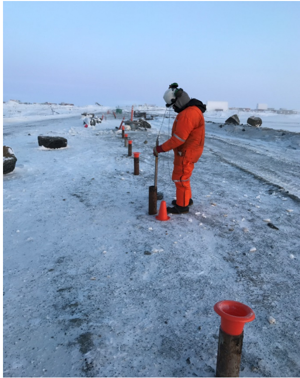
Photo 16: Checking Casing Installation
