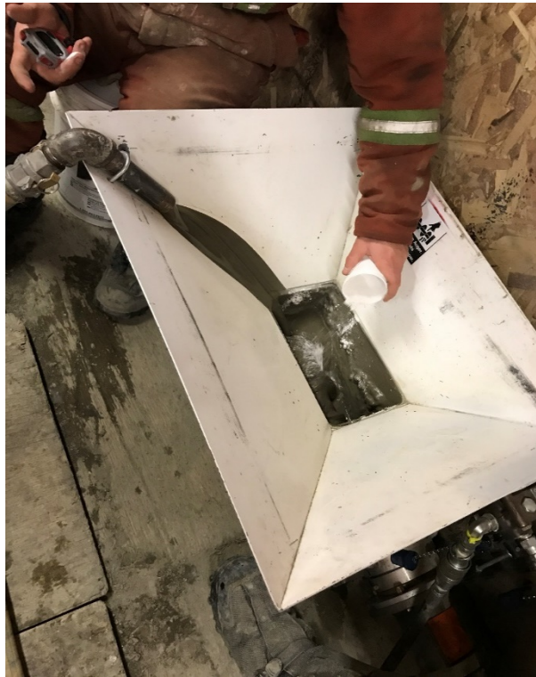
Photo 20: Adding celbex through open throat pump
