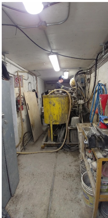
Photo 3: Inside view of the grout batching area
