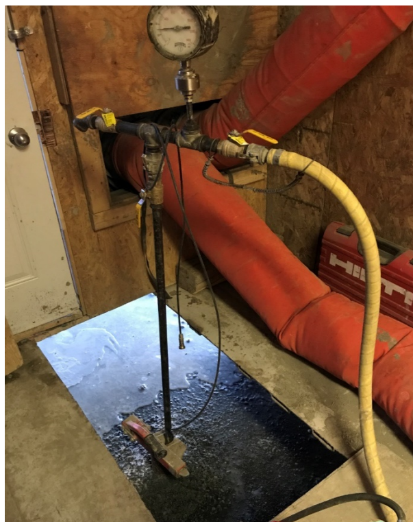
Photo 19: Set up of packer and collar gauge for blanket grouting
