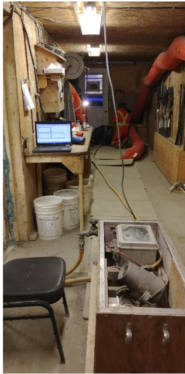
Photo 2: Inside view of the Injection unit
