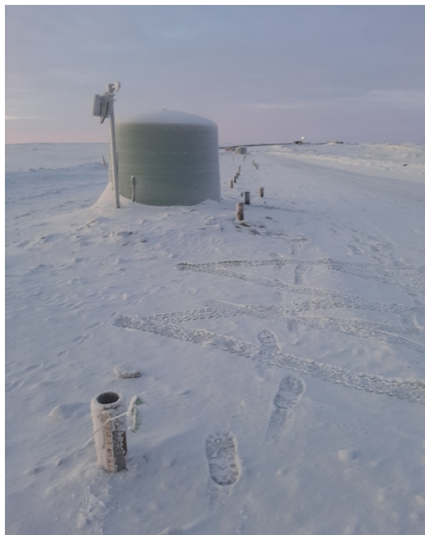
Photo 17: Casing installed showing casing offset from instrumentation cables
