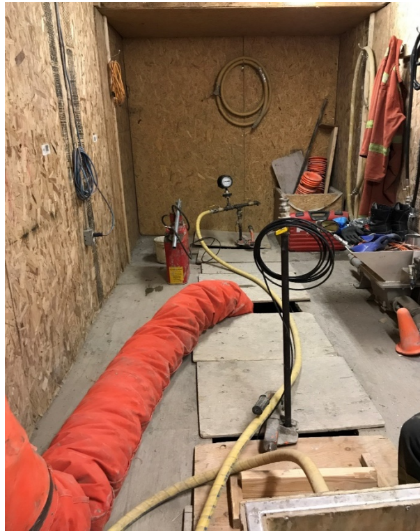
Photo 22: Setting up of dummy packer while grouting tertiary hole when adjacent secondary hole was not grouted yet
