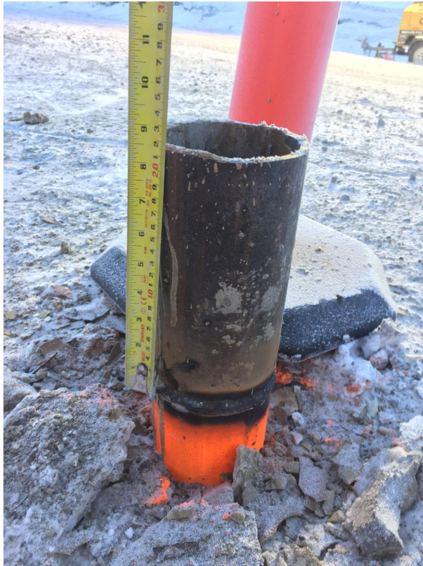
Figure 1: A photograph of the casing of primary hole #180 showing the ~200 mm welded tube on top of the casing
