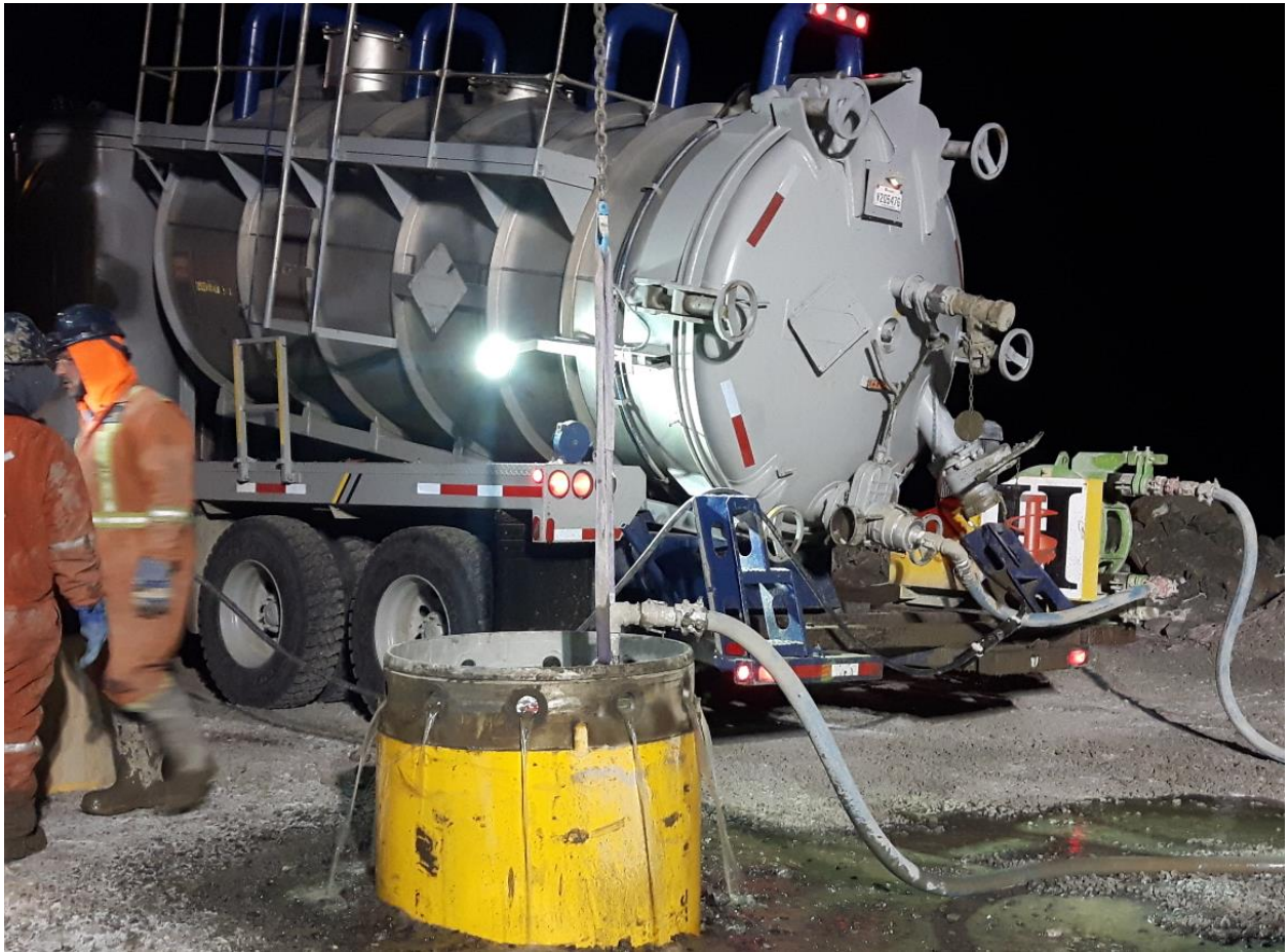
Picture showing slurry being pumped from truck to the piles
