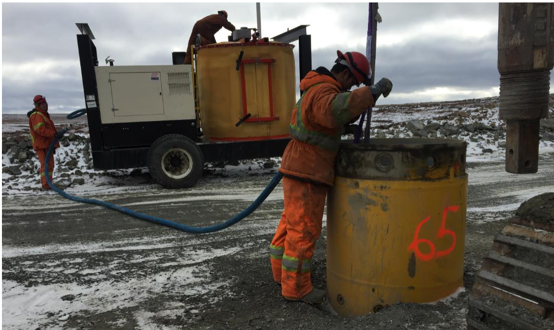
Figure 2 – CB Mix being Pumped to Primary Pile 065
