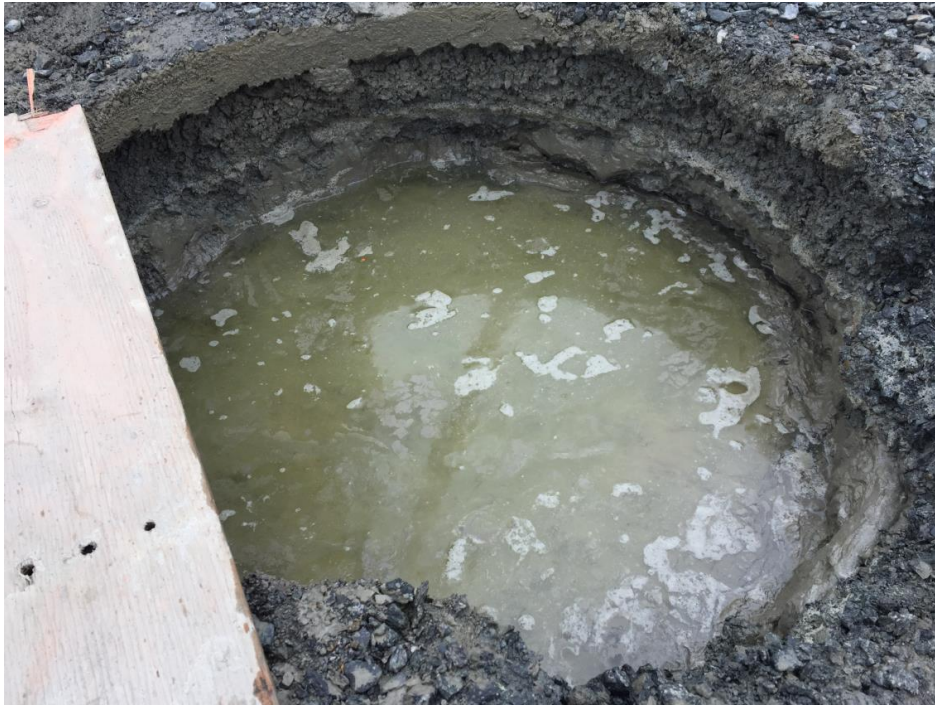
Figure 1 - Drop in Pile Height After Placement in Primary Pile 065: The pile was filled to the full elevation later on
