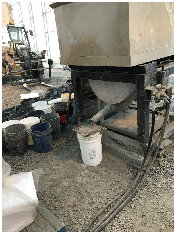
Transferring cement from big bags to 20 kg pails
