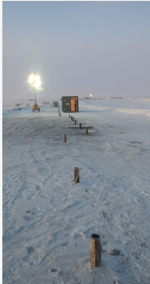
Casing offset due to buried instrumentations
