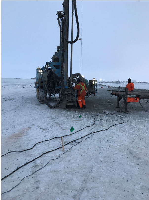
Casing instalation near west end of WTD
