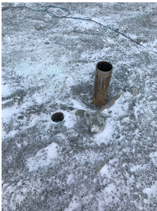
Casing relocated due to shoe broken at P488.5
