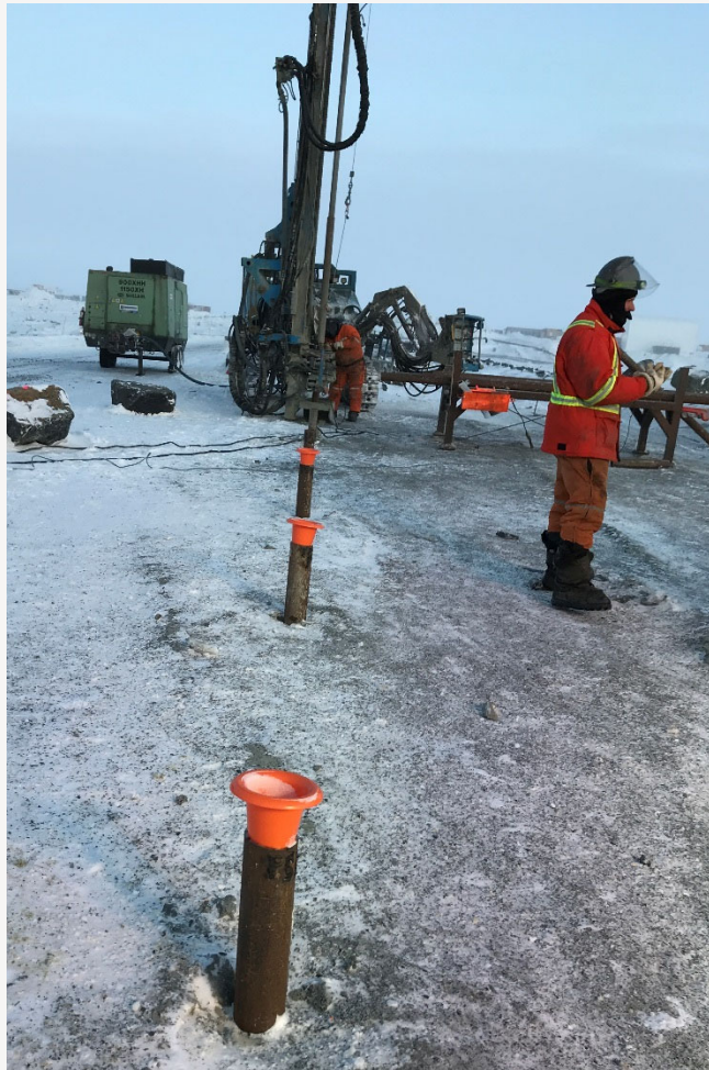
Installation of casings
