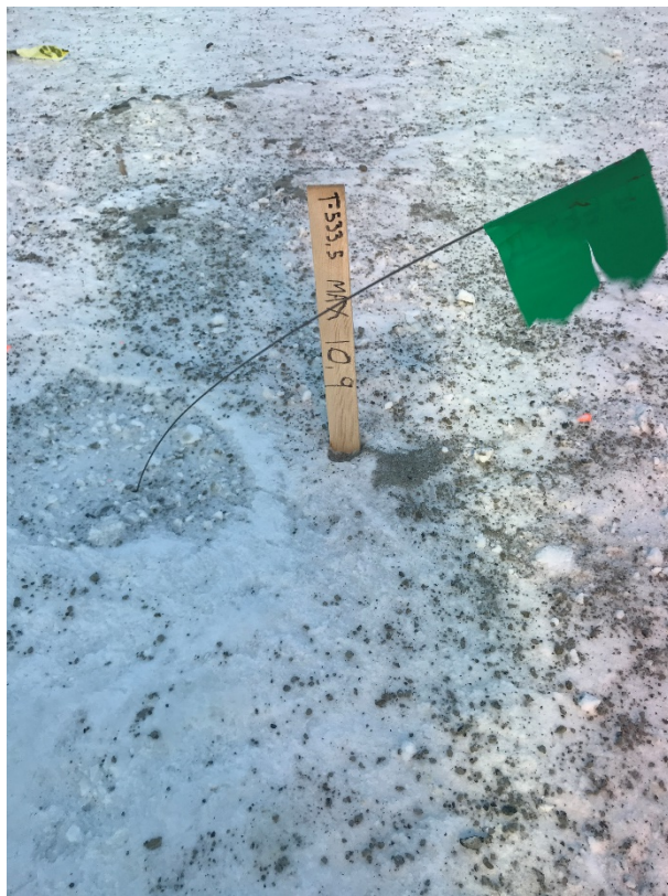
Borehole staked with expected bedrock depth and casing length
