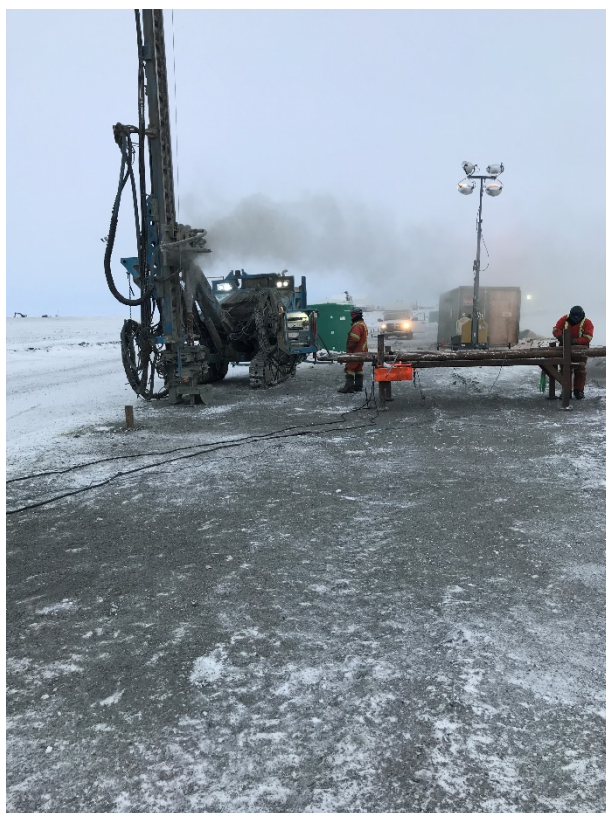
Casing installation in progress
