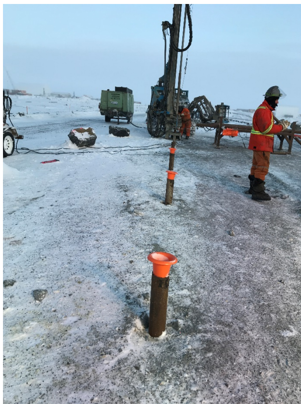
Casing installation in progress
