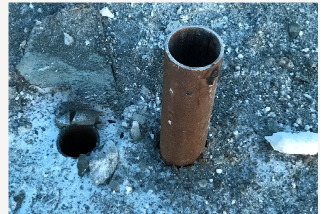
Drilling of new hole where obstruction occurred
