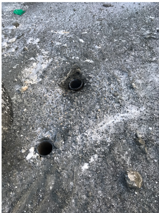
Casing shoe broken two time at T533.5 and casing installed in middle
