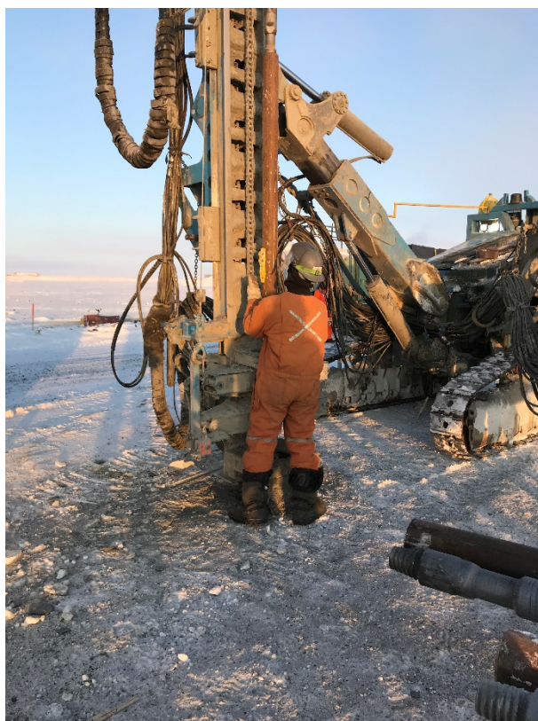
Checking casing alignment during installation
