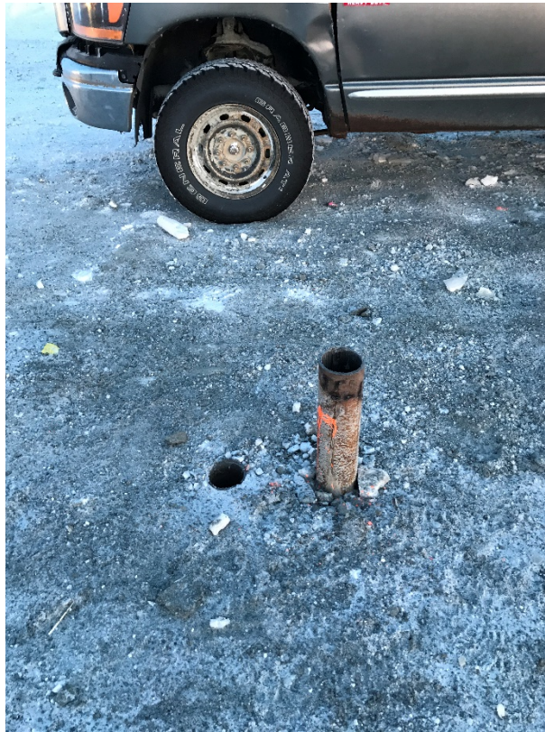
Casing relocated due to shoe broken at T521.5
