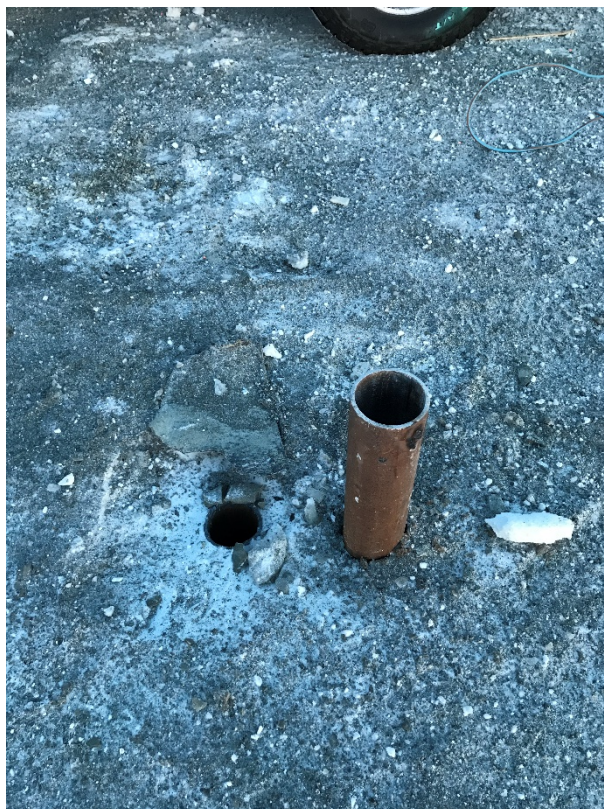
Casing relocated due to shoe broken at Q524.5
