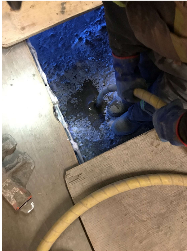
Backfilling T479.5 after confirming grout elevation within the casing
