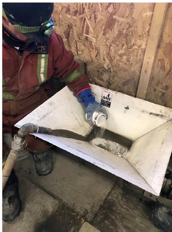
Adding celbex through open throat pump
