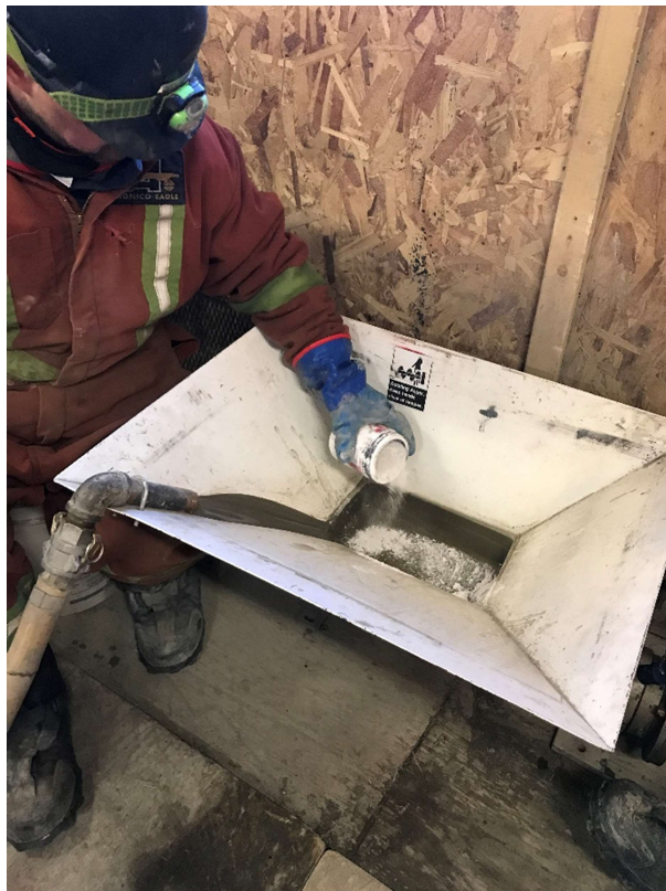
Adding celbex through open throat pump
