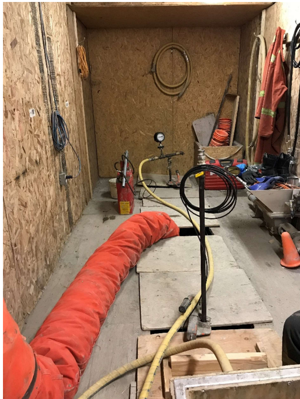
Packer installed at S614.5 while grouting T611.5
