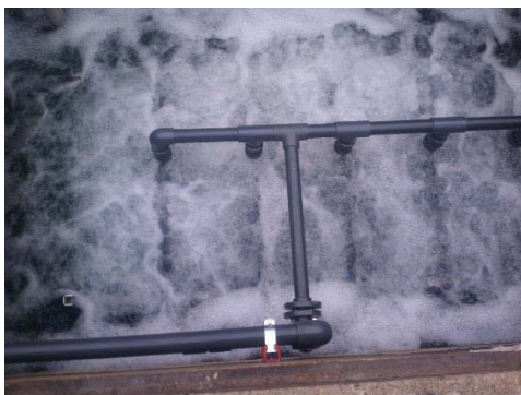
Proper air scouring in membrane tank
