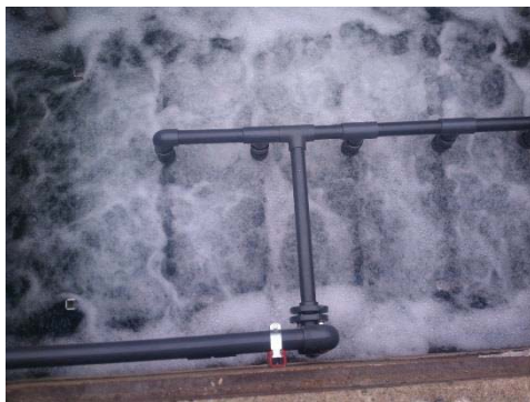
Proper air scouring in membrane tank
