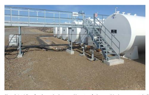
${\it Photo 3: Jet-A\ Transfer\ -\ Connection\ between\ shipper\ transfer\ hoses\ and\ Agnico\ permanent\ pipeline}$
