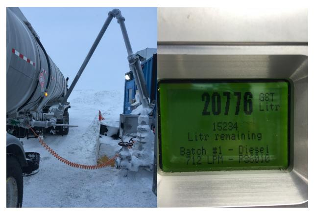
Photo 4: Agnico Eagle Ltd.'s Refueling Station – Loading arm and Scully System
