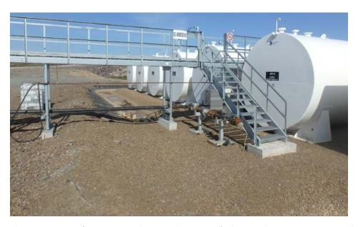
${\it Photo 2: Jet-A\ Transfer\ -\ Connection\ between\ shipper\ transfer\ hoses\ and\ Agnico\ permanent\ pipeline}$
