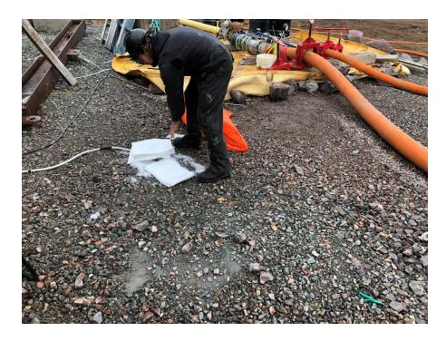
Photo 3 - Absorbent sheets applied on the contaminated area
