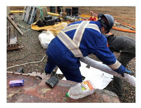
${\it Photo}~4~{\it -}~Absorbent~sheets~and~booms~applied~downstream~and~on~the~contaminated~area$
