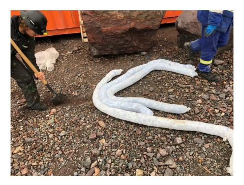
Photo 5 - Trench dug downstream of the spill to contain de spilled fluid
