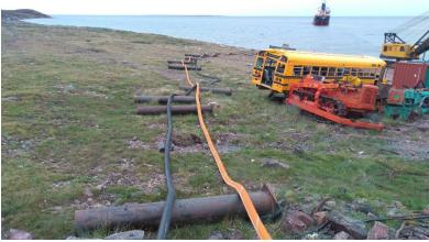
${\it Photo 1: Diesel\ Transfer\ -\ Connection\ between\ shipper\ transfer\ hoses\ and\ Agnico\ permanent\ pipeline}$
