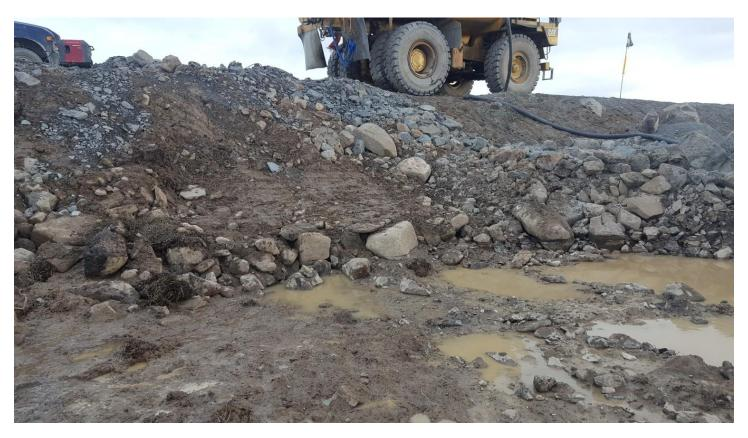
Upon completion of cleanup, excavated material was replaced with natural overburden material from stripping operation of the IVR pit, as part of the Whale Tail Pit Project Expansion, roughly located 7 km away.
