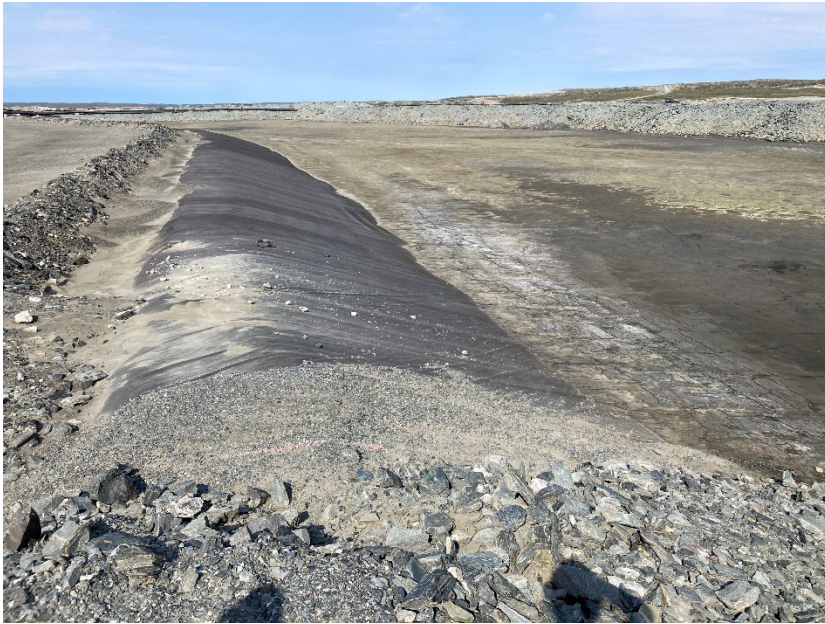
Photograph B4-09 Stormwater Dike
