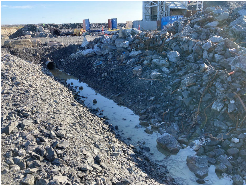
Photograph H12-4 UG Ore Stockpile Saline Ditch
