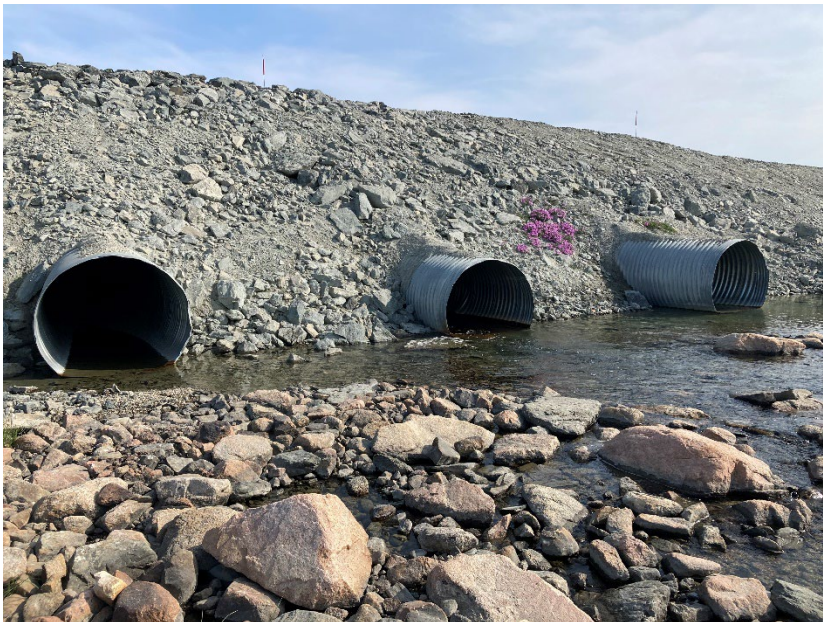
Photograph H1-02 Vault Road Culverts
