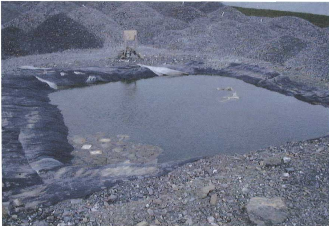
figure 1. Lined sump within the ore storage pad; 2000/07/11.
