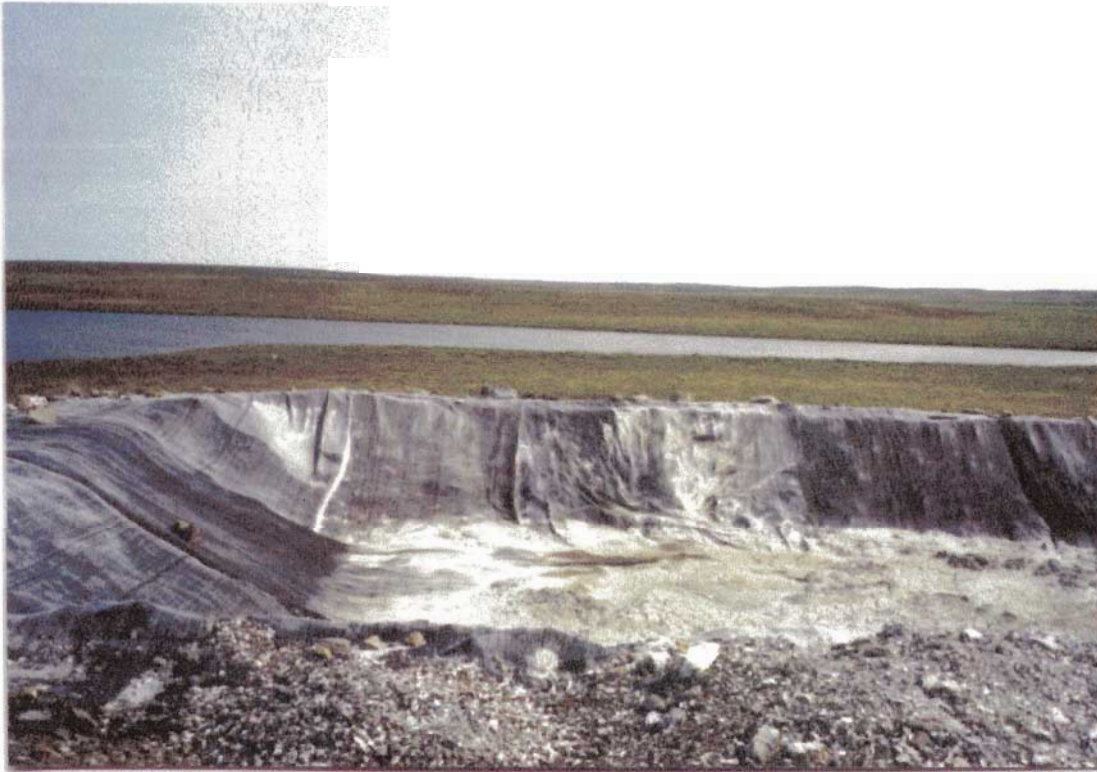
figure 5. Lined sump in periphery of the ore pad; 2000/07/20. (courtesy of NWB)
