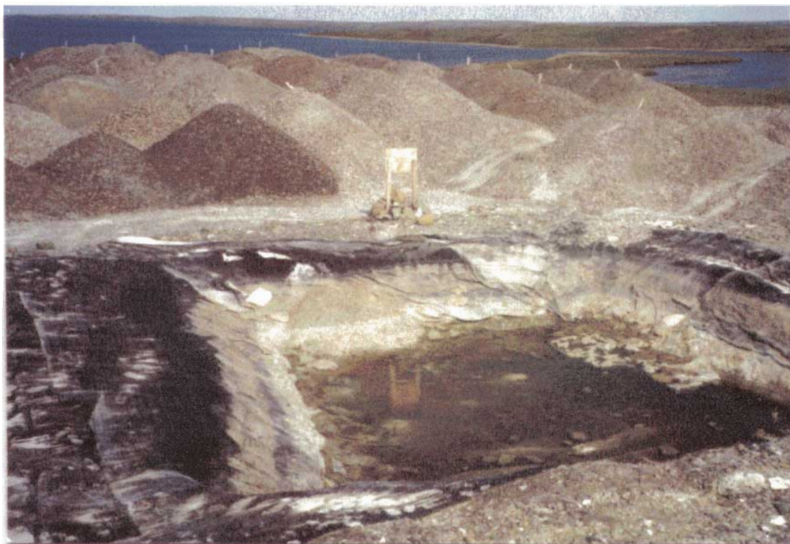
figure 2. Lined sump within the ore storage pad; 2000/07/20. (courtesy of NWB)
