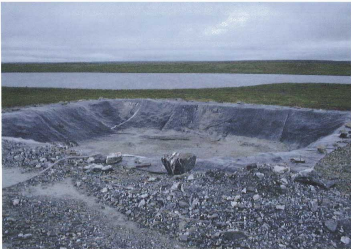
figure 4. Lined sump in periphery of the ore storage pad; 2000/07/11.
