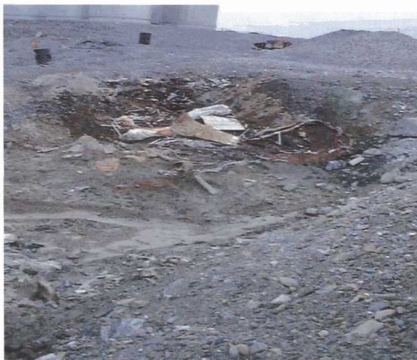
figure 3. Unlined sump in the periphery of the ore storage pad; 2001/08/12.
