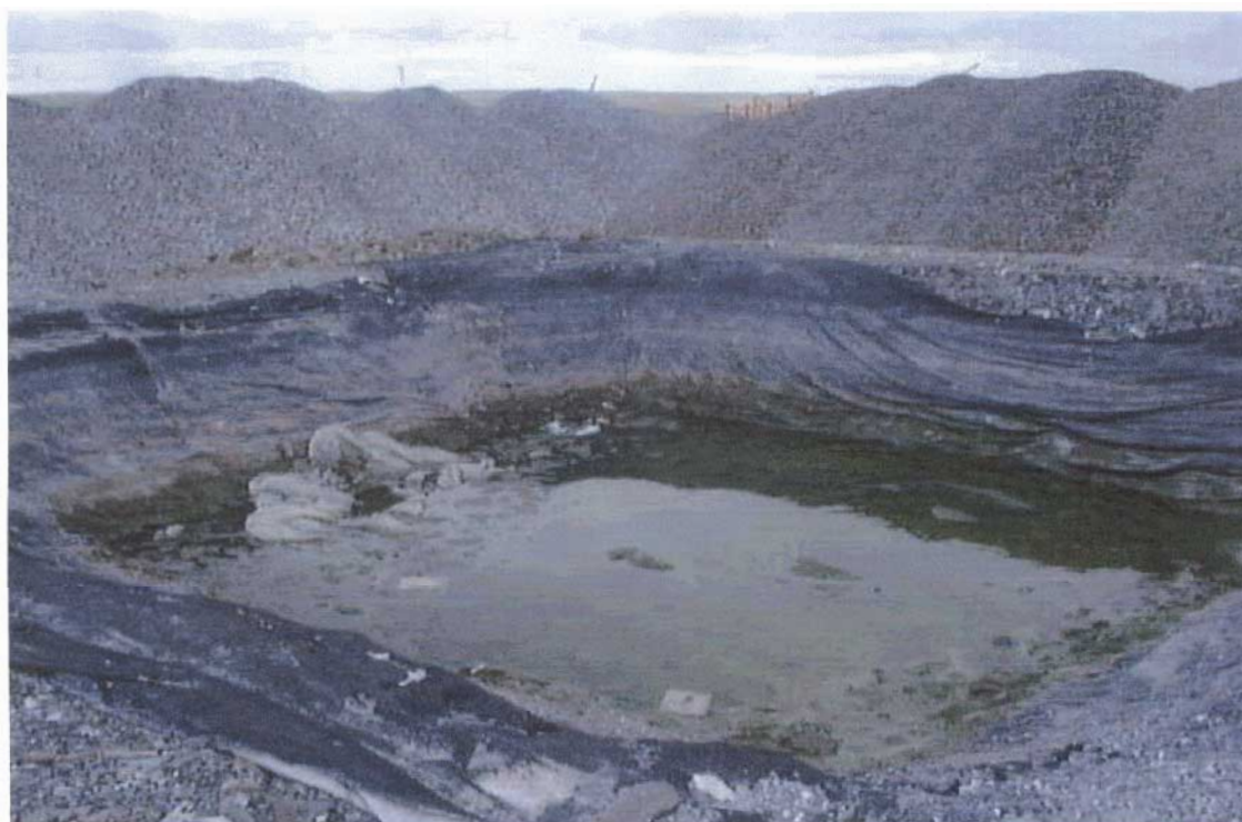
figure 2. Lined sump in the ore pad area, dubbed central holding pond; 2001/08/12.
