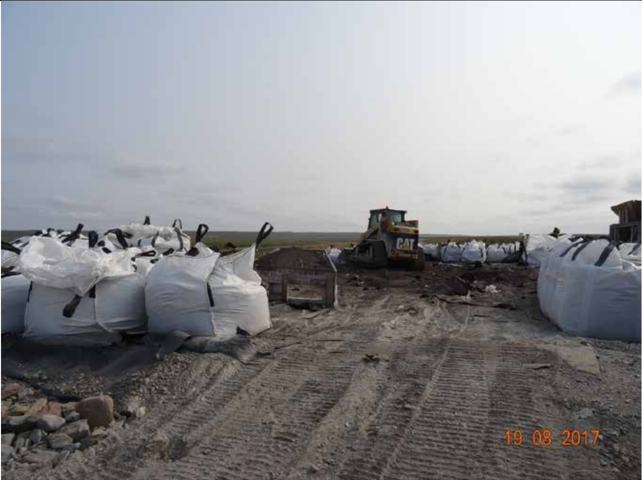
Description: Landfarm contents being bagged for winter backhaul to Doris.
