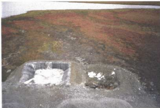
Settling Ponds at Boston Camp, August 31, 1999. Note northern pond is lined, and southern pond is unlined. Also note supersacks in southern pond.
