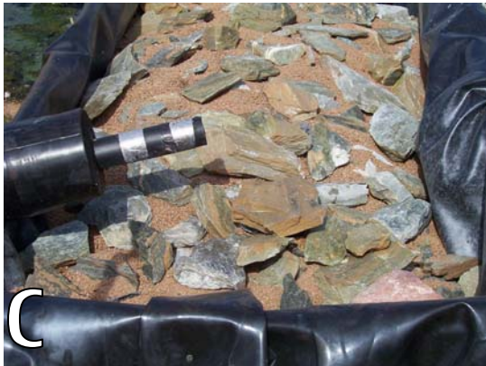
Photographs C & D: Photo C showing peat moss and corncobs laid over the gravel bed. Rocks were then placed on the peat moss and corncobs. Photo D showing the general location with corncobs spread to absorb sludge and remove odour emitting from the discharge area. The application was effective in reducing foul odour.
