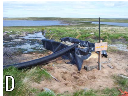
Photographs C & D: Photo C showing peat moss and corncobs laid over the gravel bed. Rocks were then placed on the peat moss and corncobs. Photo D showing the general location with corncobs spread to absorb sludge and remove odour emitting from the discharge area. The application was effective in reducing foul odour.
