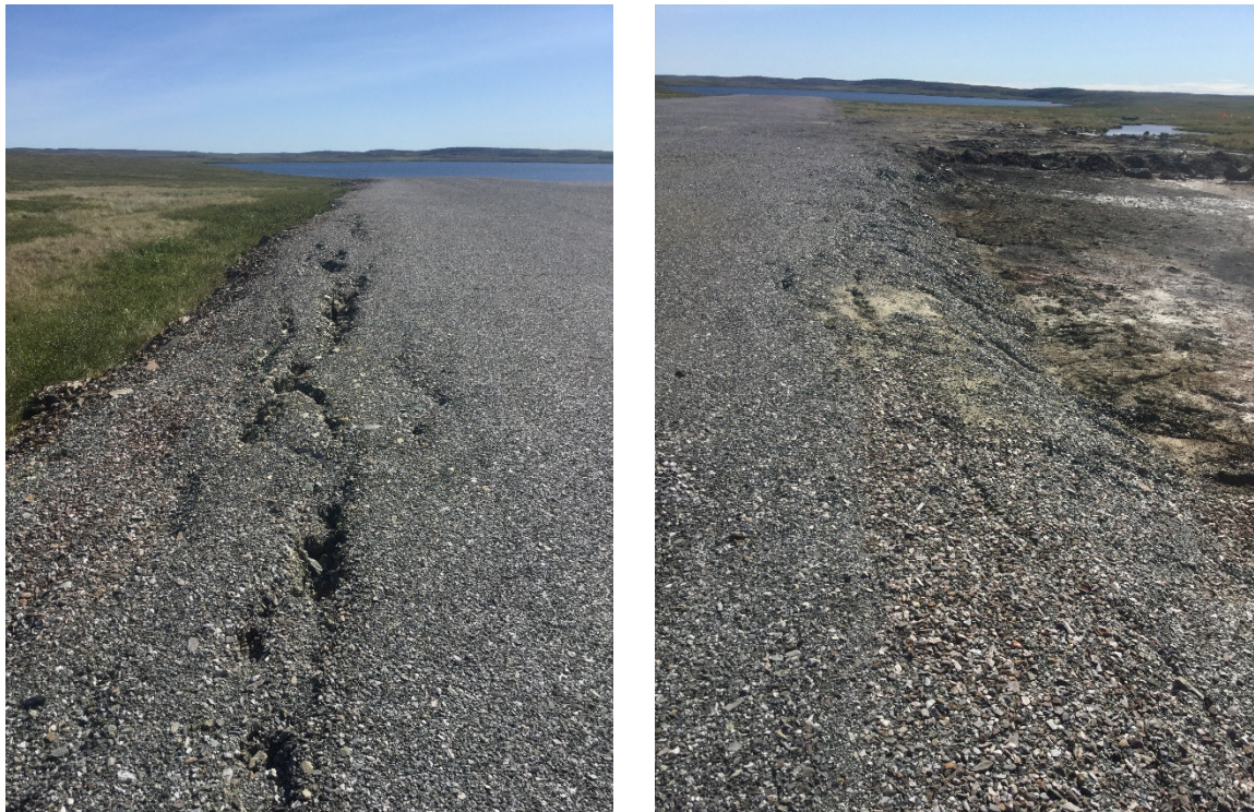
Photos 1 and 2: The left-hand photo shows some of the more extensive and wider shoulder tension cracks along the airstrip shoulder. The right-hand shoulder depicts some of the newer, but still extensive shoulder cracking.
