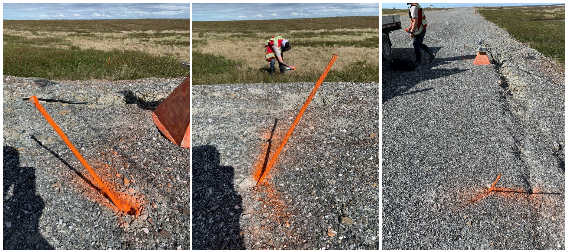
Photographs 1, 2 and 3: Fix survey monitoring pins installed in June 2020.
