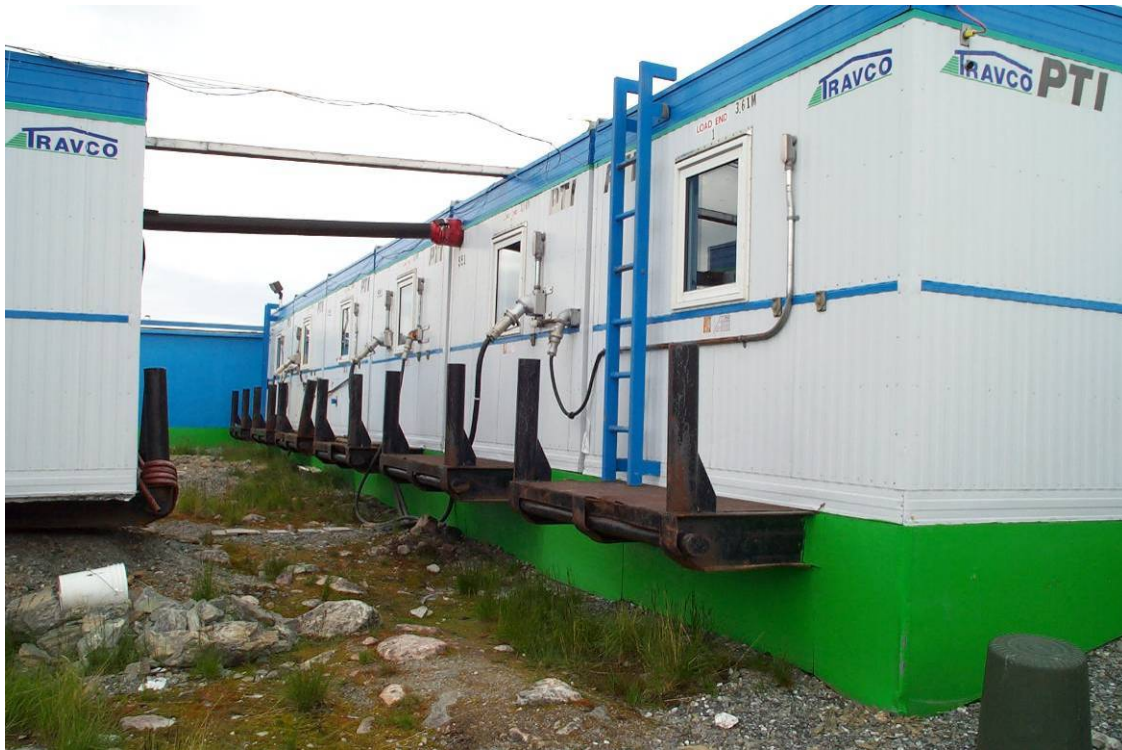
Photo 3: The accommodation complex trailers are installed on skids, which are leveled on the foundation pad by means of timbers (see note for Photo 1).
