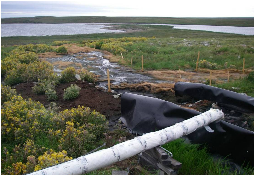
Photo 40: Drop box for the sewage grey water discharge. Note: the cocoa matting in the background.
