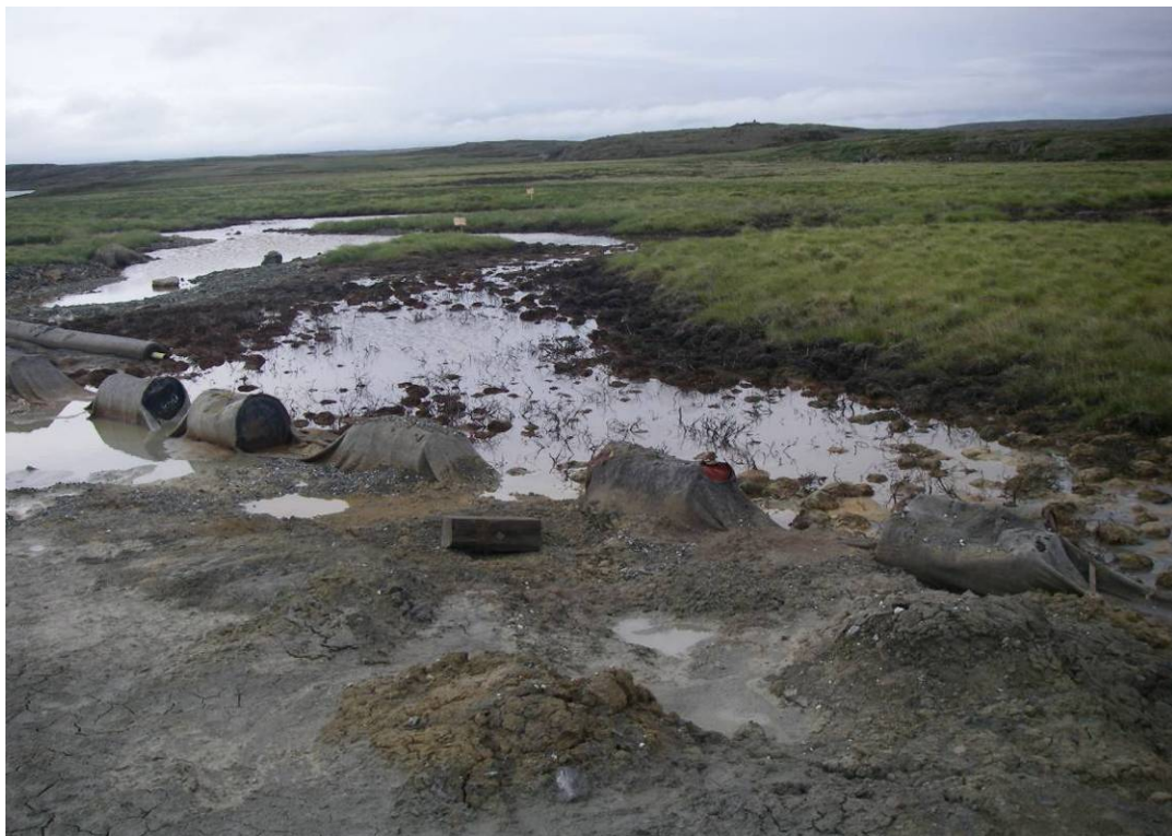
Photo 24: Drill cutting sedimentation pond outlet. Note: filter cloth is no longer functional.
