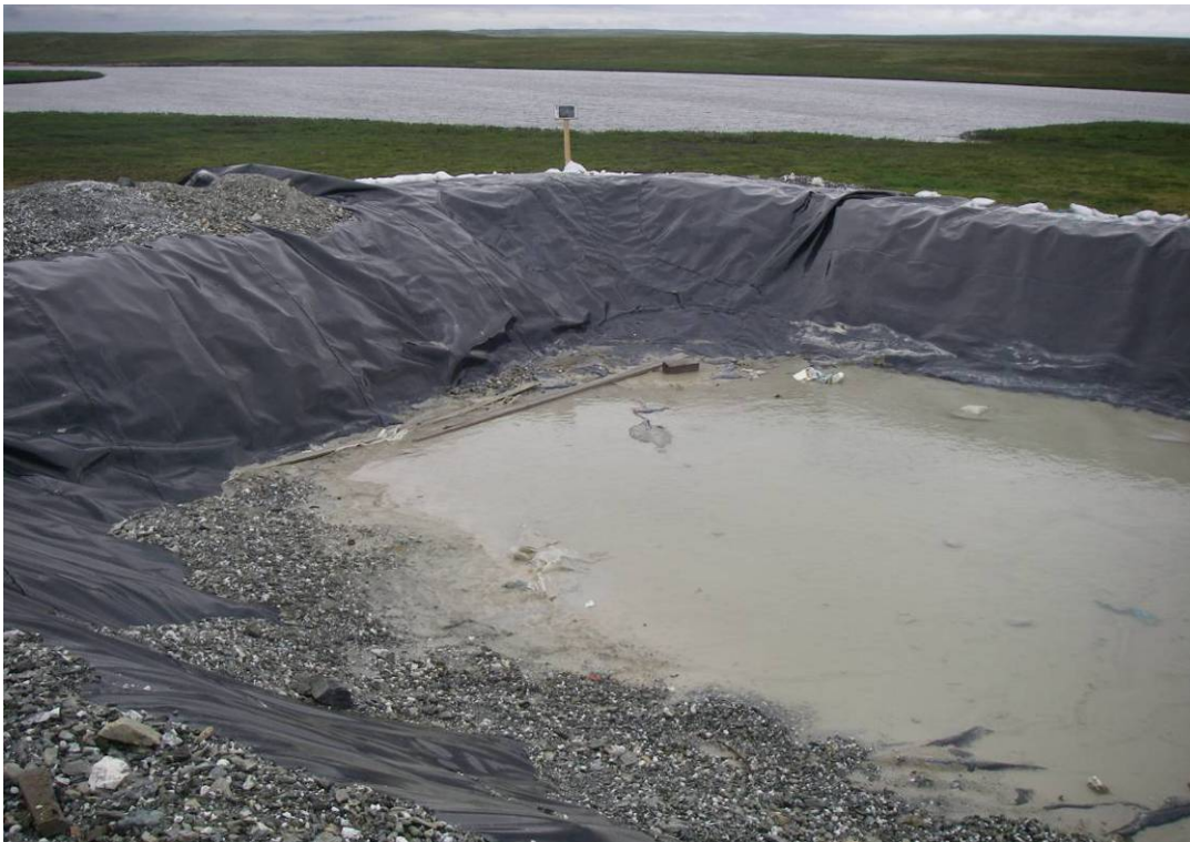
Photo 19: Note: wood debris, gravel and other sediment in base of sedimentation pond.
