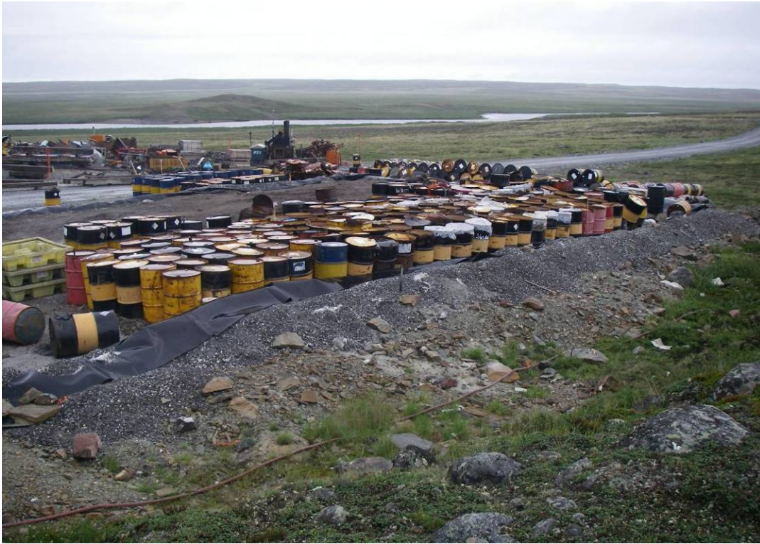
Photo 21: Fuel drums filled with contaminated soil stored on top of the soil filled landfarm.
