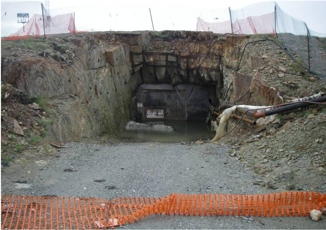
Photo 25: Portal entrance. Note: upper barricade needs to be repaired.
