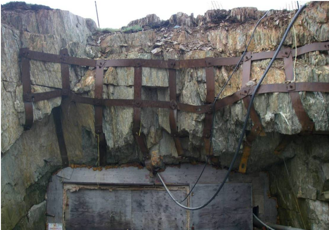
Photo 27: Steel mesh band and rock bolts supporting the portal access roof. Note: spalding rock will be a hazard should the roof support collapse.
