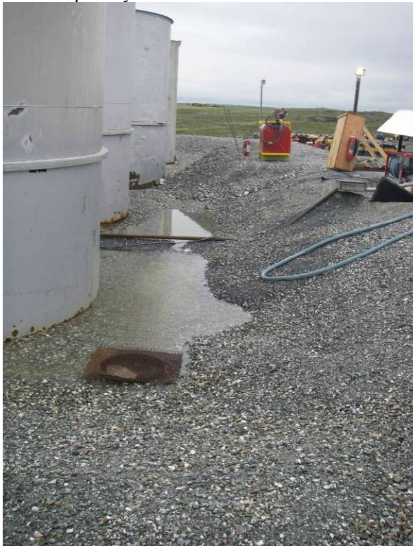
Photo 12: Ponded water in the primary tank farm. This suggests that the liner is performing as intended.
