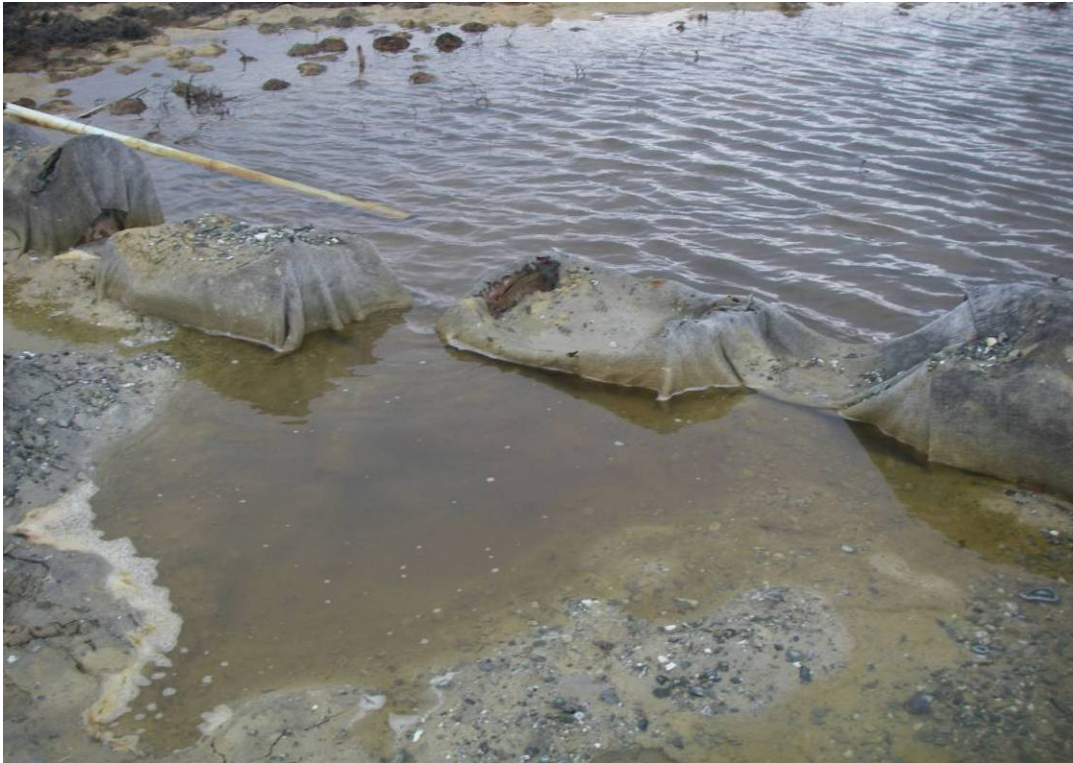
Photo 23: Drill cutting sedimentation pond outlet with geotextile filter cloth wrapped around old fuel drums. Water however by-passes this system which is in disrepair.
