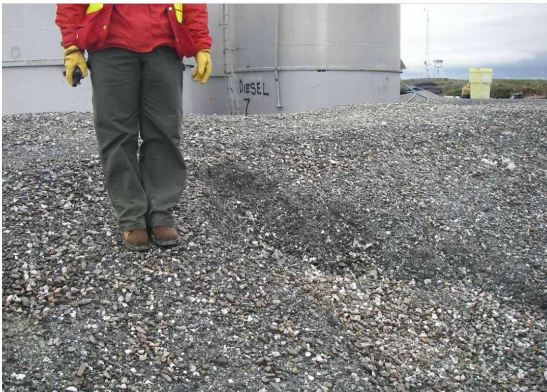
Photo 10: Surficial slip surfaces on the west face of the primary tank farm berm.
