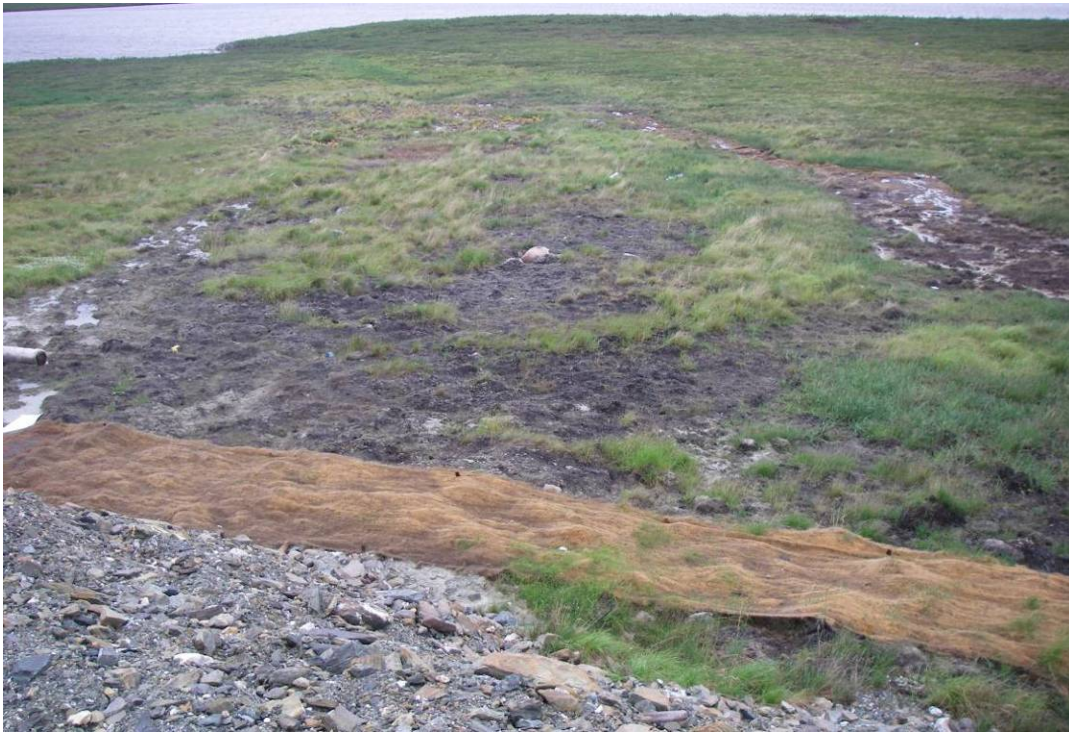
Photo 31: Cocoa matting placed on vegetation dieback areas to control erosion and promote revegetation. Note: damage from the drainage in the background.
