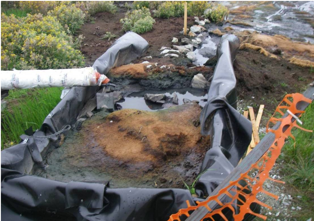
Photo 39: Drop box for the sewage grey water discharge.
