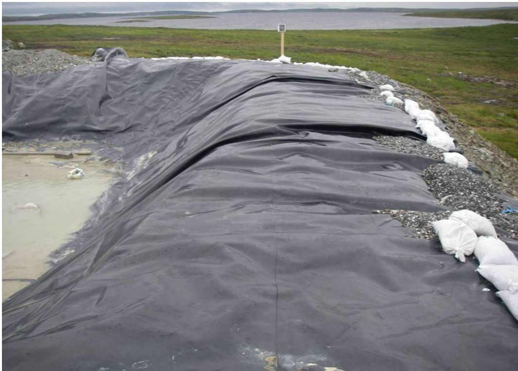
Photo 18: Sedimentation pond liner repositioned and repacked with sand bags.
