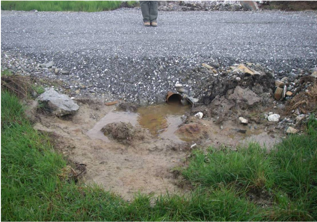
Photo 35: Pipe culvert outlet with no apparent drainage. This culvert is under the core storage area road.
