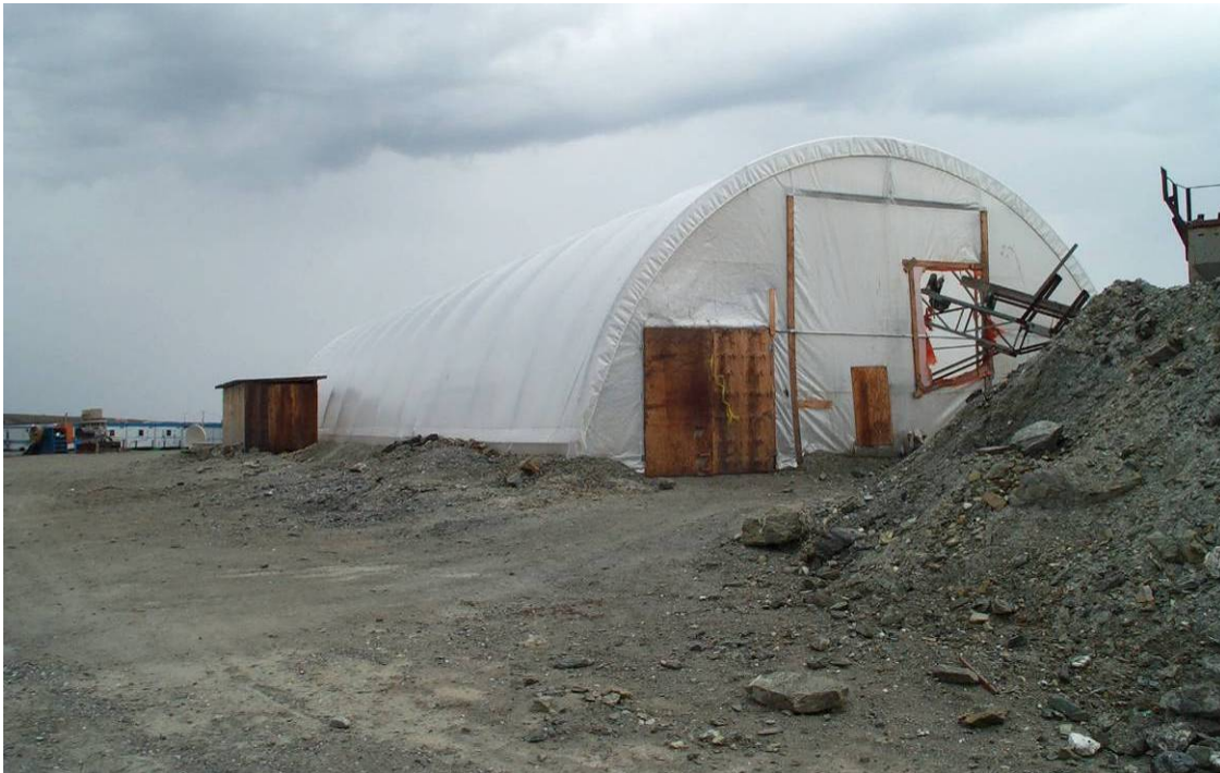
Photo 5: Heated sprung structure used to house the bulk sample crushing plant (see note for Photo 1). The crushing plant was dismantled and the structure is currently used for general storage and heavy equipment shelter.
