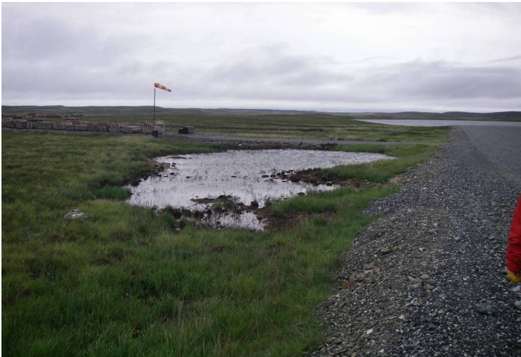
Photo 44: Large pool of standing water immediately adjacent to the airstrip. Ponding due to permafrost degradation at the old drillhole location.
