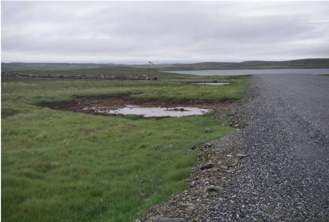
Photo 43: Permafrost damage and vegetation dieback at the historic drill hole location immediately adjacent to the airstrip.
