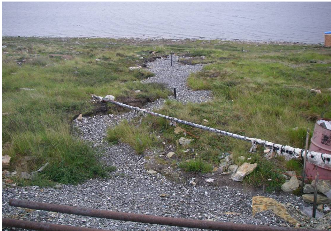
Photo 34: Repaired erosion gulley southwest of camp pad. Crushed ore material used for repair.
