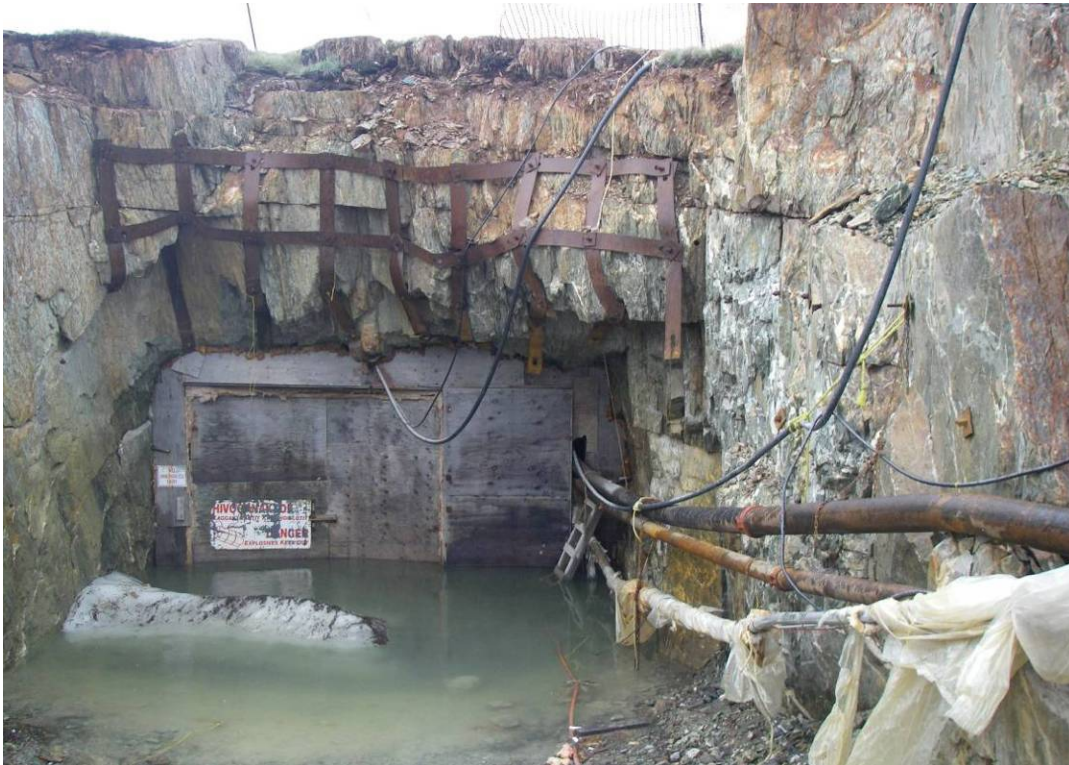
Photo 26: Portal entrance. Note: access warning sign is faded and the area is flooded at time of inspection.
