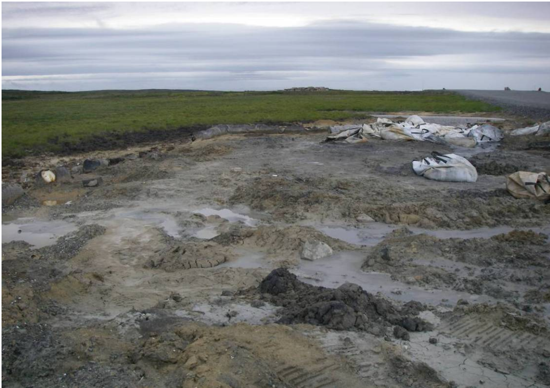
Photo 22: Drill cutting sedimentation pond.
