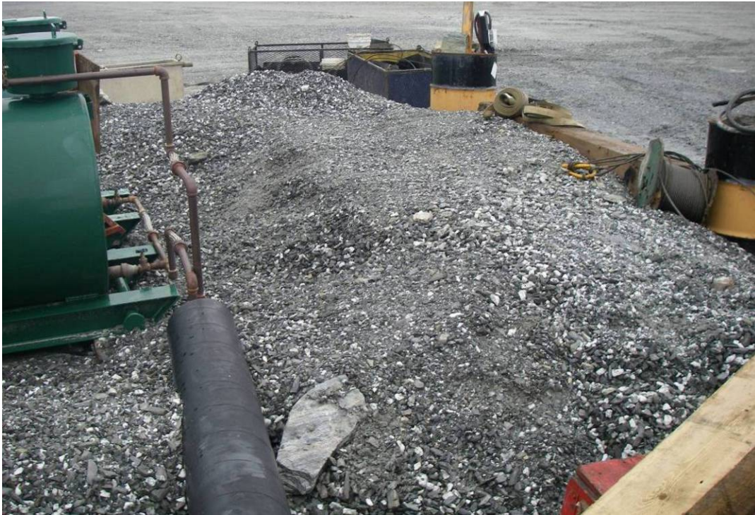
Photo 13: Diesel fuel tank supply to the camp powerhouse. Containment dike breaches have been repaired.
