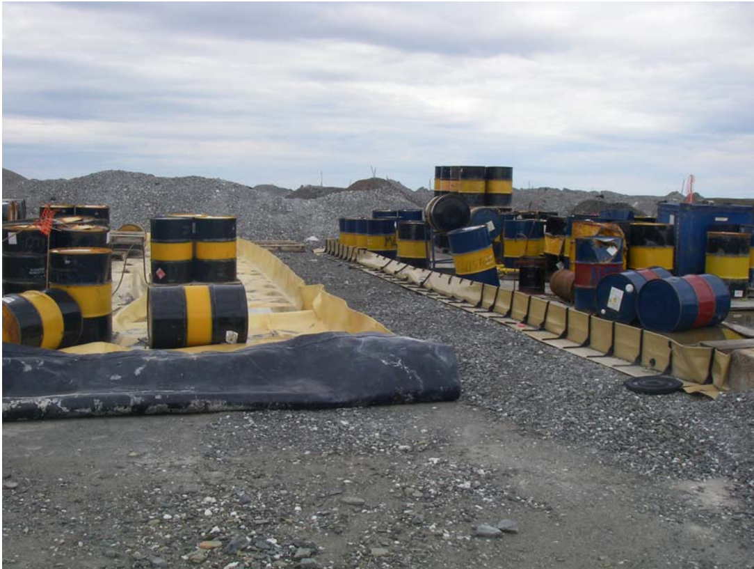
Photo 21: Another view of the collapsed secondary containment system wall, with another jet fuel stack and secondary containment system in the background.
