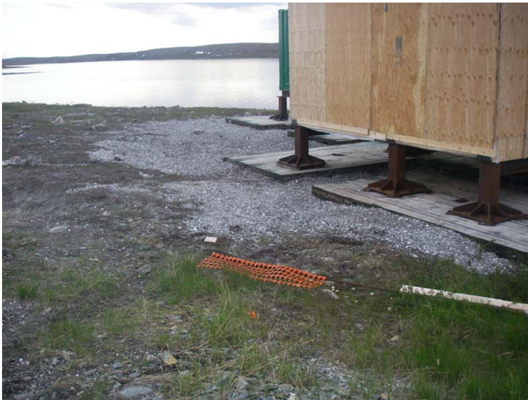
Photo 13: Close-up of raised foundation footings used on the new Boston Sewage Treatment Plant.
