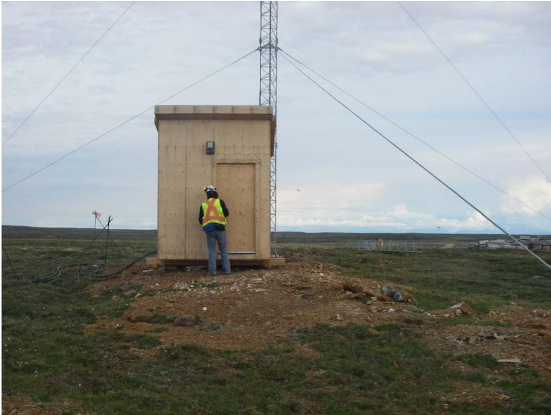
Photo 51: Enclosure for radio equipment installed on raised wooden foundation on rock outcrop.
