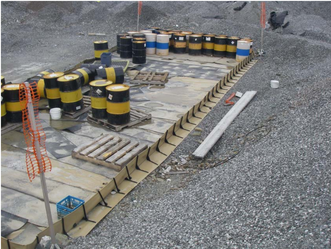
Photo 23: Another view of the secondary containment system used to store the jet fuel.
