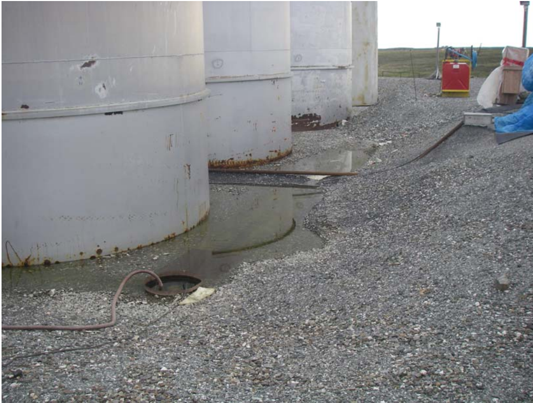
Photo 31: View of water ponded in the fuel tank farm. A trash pump is installed in the sump.
