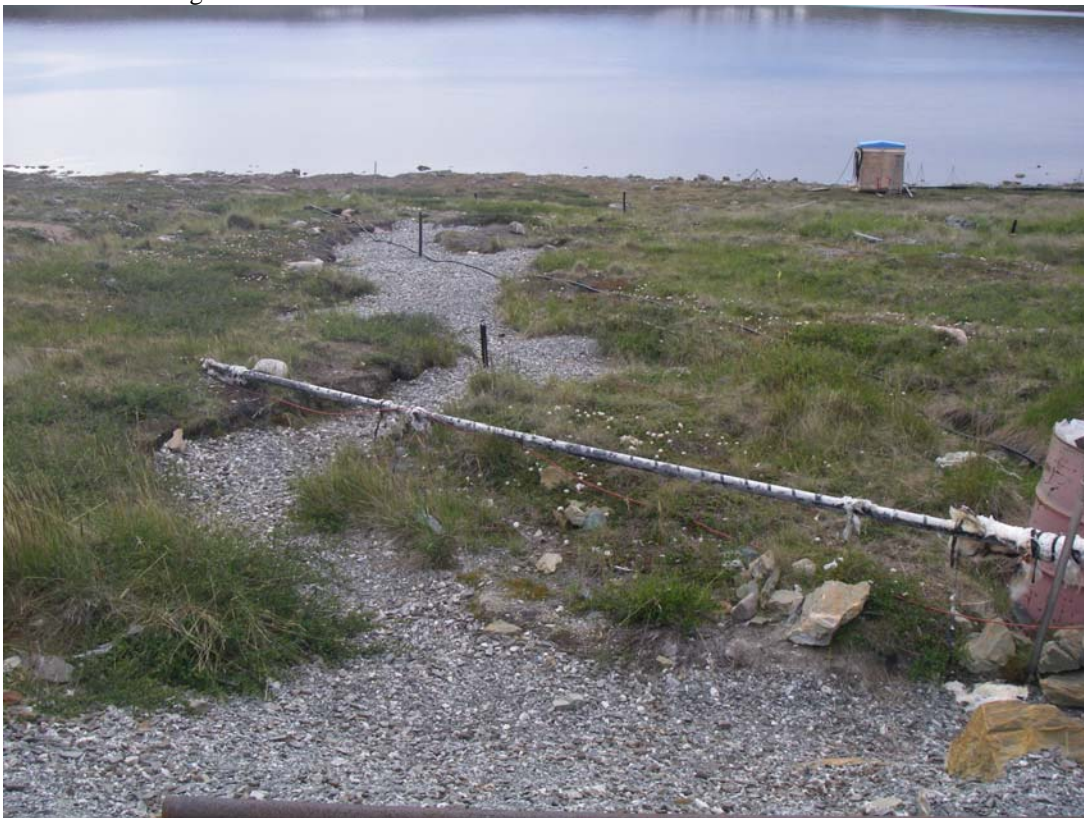
Photo 38: Looking west at an area of erosion and permafrost damage repaired by infilling with gravel.
