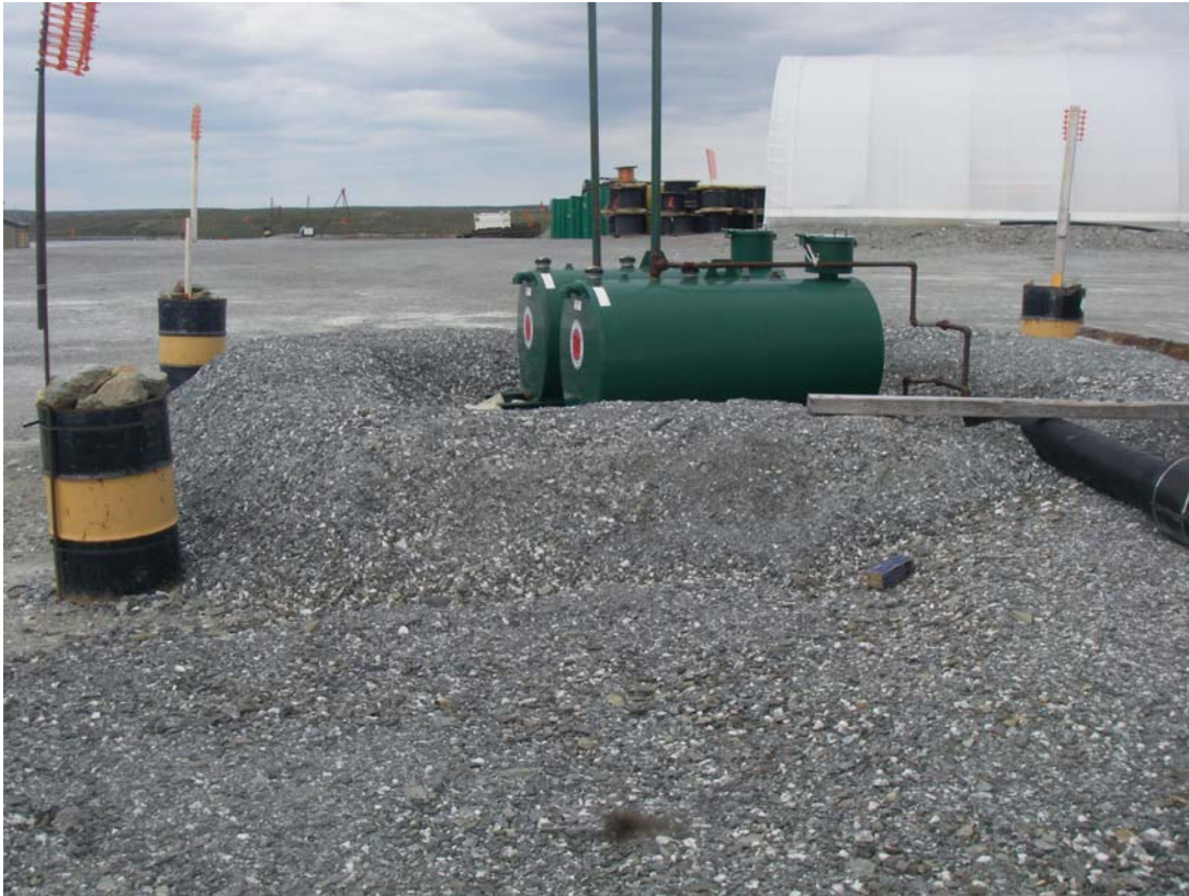
Photo 39: View of the secondary containment and fuel tanks (western section) supplying the diesel power generators.
