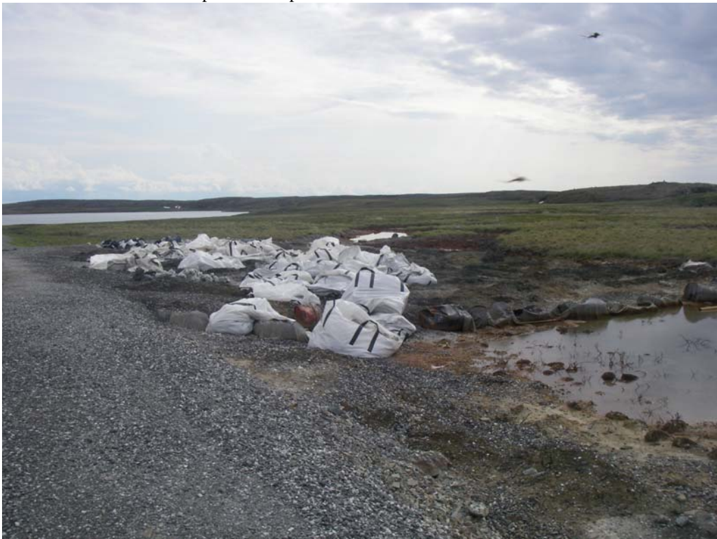
Photo 46: Close-up of permafrost damage immediately adjacent to the airstrip. The bags in the picture are filled with drill cuttings.
