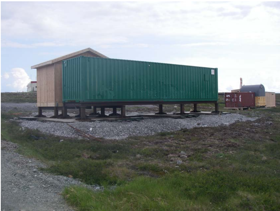
Photo 12: Thermal pad and raised foundation for components of the new Boston Sewage Treatment Plant.
