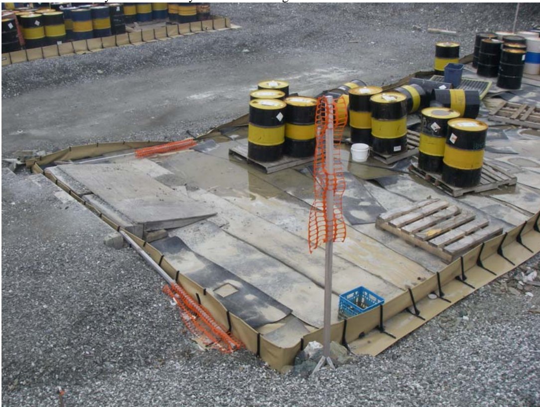
Photo 22: More jet fuel stored in a secondary containment facility. Note the access ramp constructed to facilitate loading and unloading of fuel.
