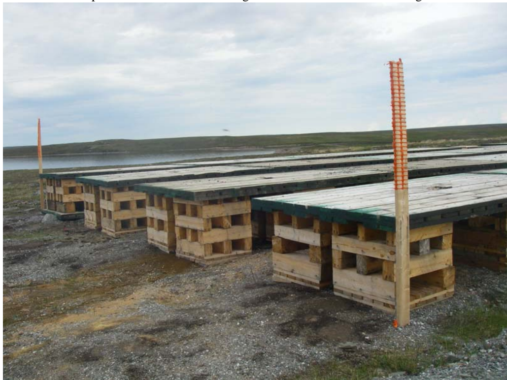
Photo 14: Lower end of the leveling foundation for the new Boston Sewage Treatment Plant.
