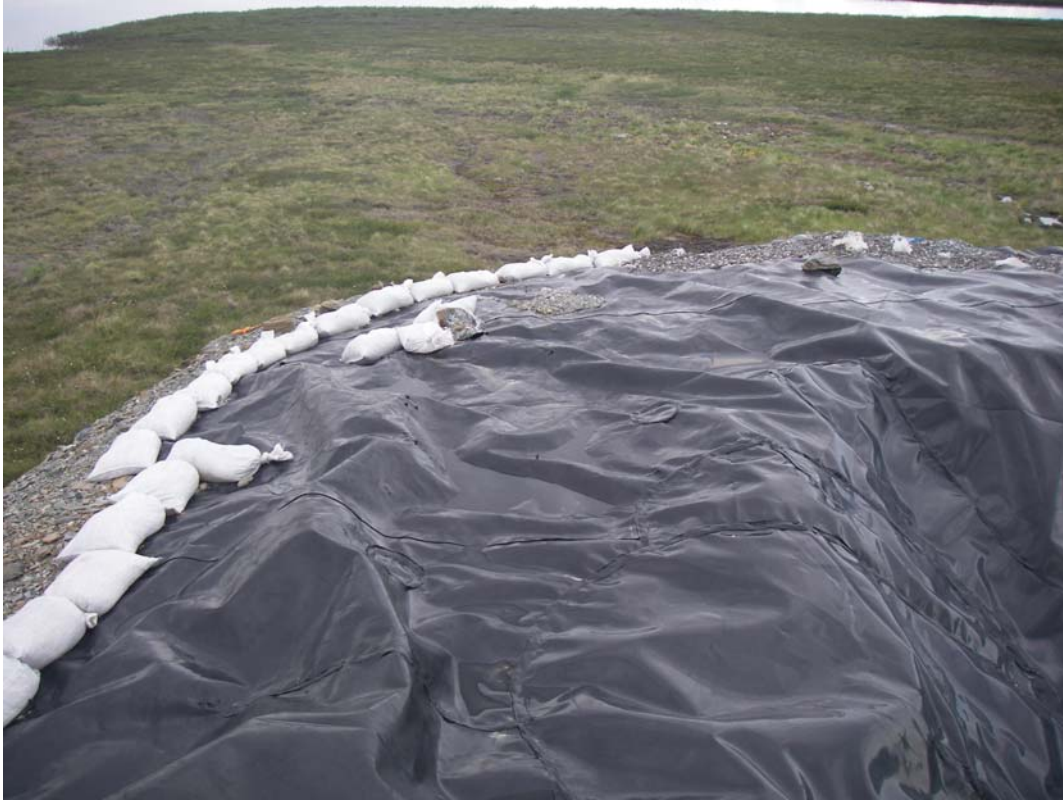
Photo 27: View of the sand bags used to anchor the liner for the setting pond.
