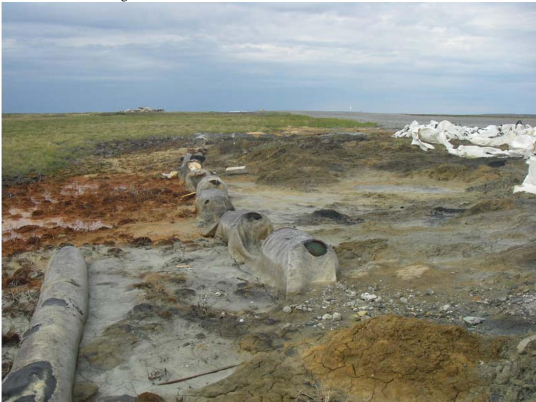
Photo 48: Looking north across the permafrost degradation area that has historically been used as a sediment pond. Note the use of geotextile.
