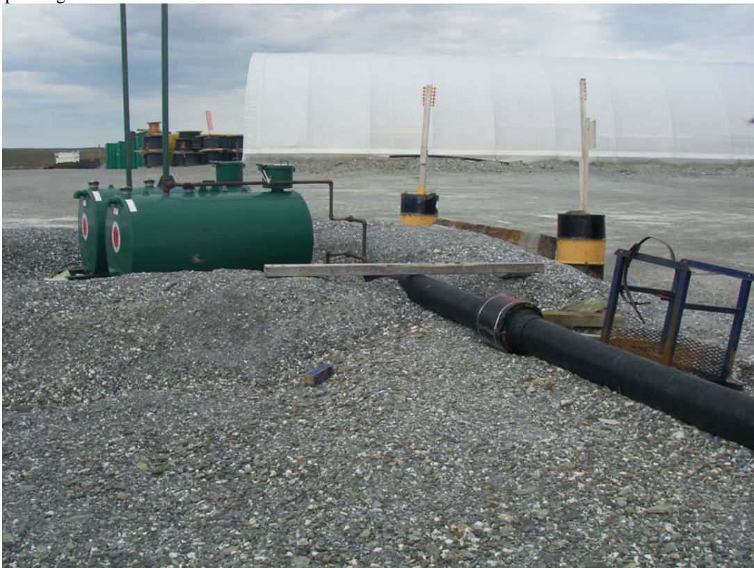
Photo 40: View of the secondary containment and fuel tanks (eastern section) supplying the diesel power generators.
