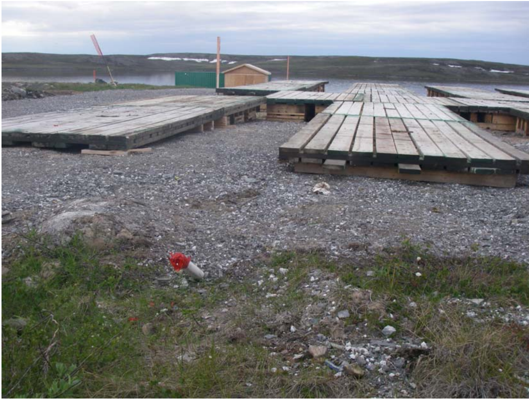
Photo 15: Upper end of the leveling foundation for the new Boston Sewage Treatment Plant.
