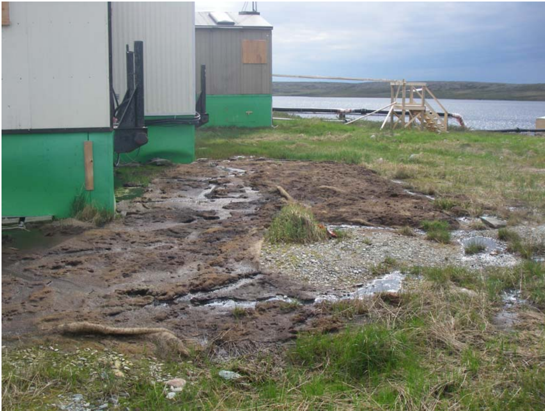
Photo 55: Area of permafrost degradation behind the administration office buildings.
