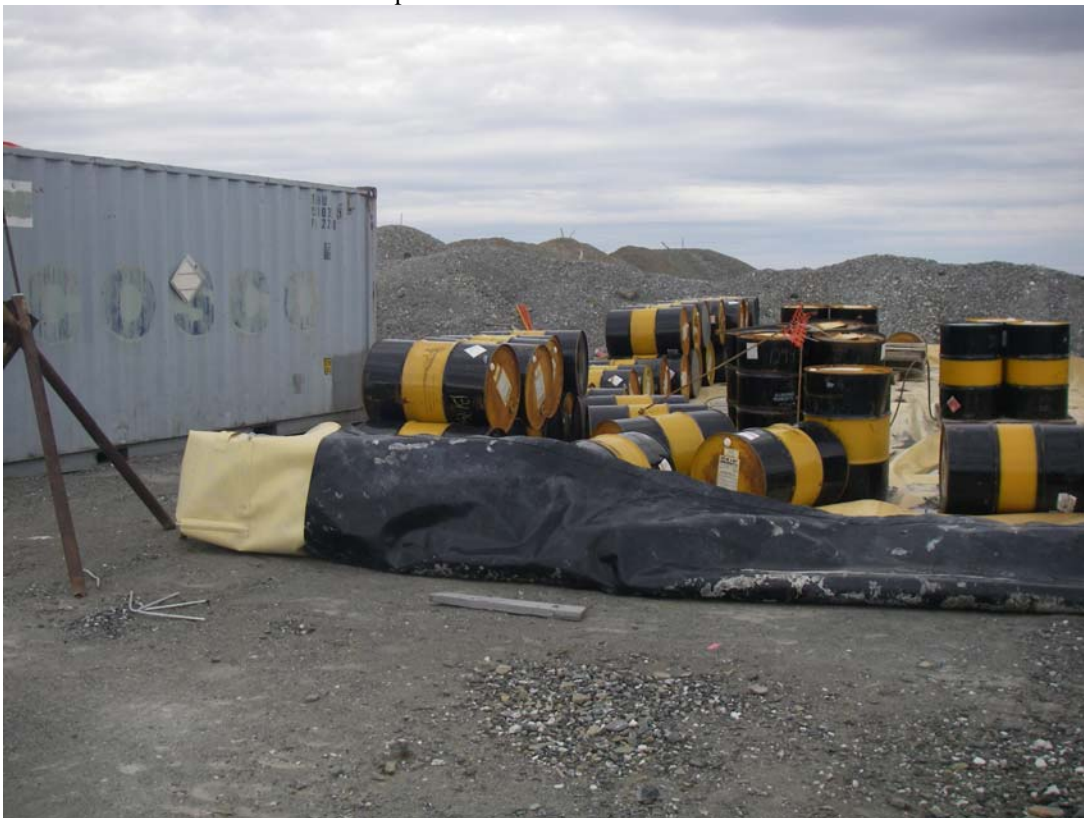
Photo 20: Jet fuel stored in secondary containment. Note one wall of the secondary containment has collapsed.
