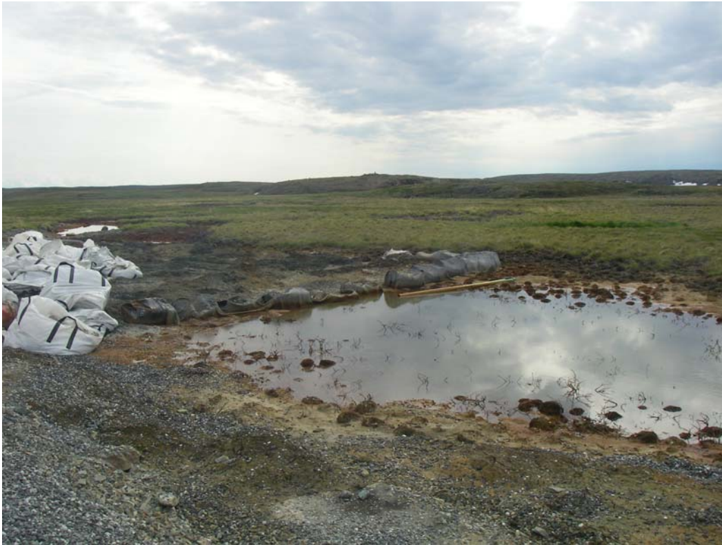
Photo 45: Close-up of extensive permafrost damage immediately adjacent to the airstrip. This area has been used as a sediment pond in the past.
