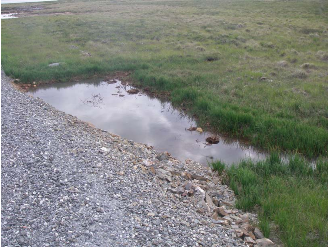
Photo 43: View of water ponded next to airstrip leading to permafrost degradation. The pond was created by drilling.
