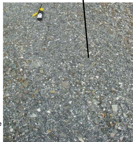
Tension cracks along the crest of the containment berm.
