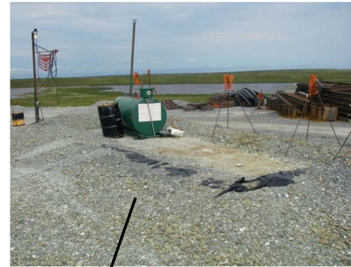
Secondary containment for fuel tank.
