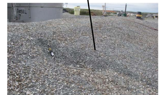
Erosion gulley on south outer containment berm.
