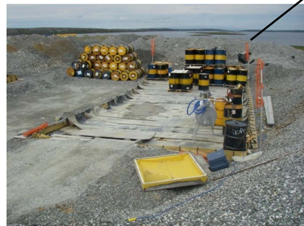
Looking north towards eastern most containment area. Note access ramp leading into bermed area.
