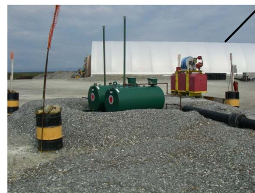
Secondary containment for fuel tanks supplying power house and workshop looking north.
