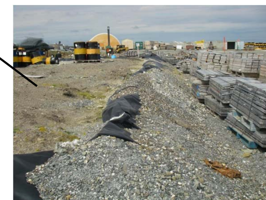
Exposed liner along the crest of the land farm east berm.
