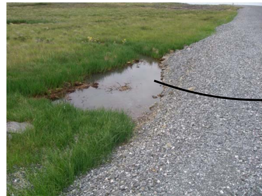
Permafrost degradation pond along west shoulder of airstrip.
