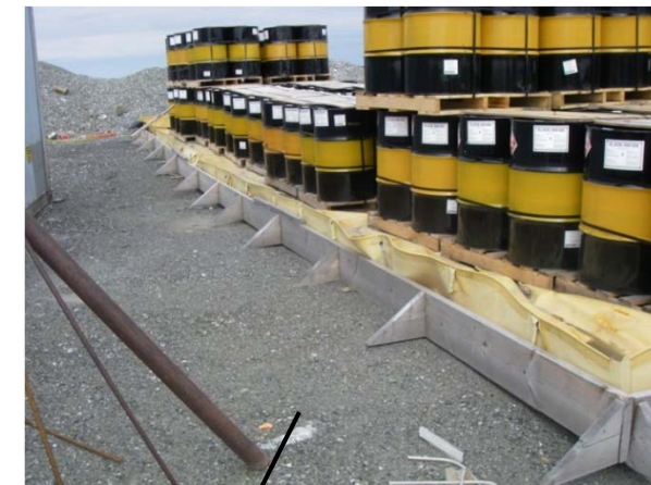
Containment berm supported by timber cribbing.
