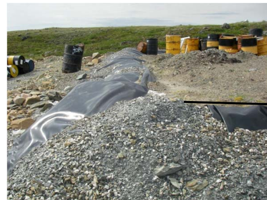
Exposed liner along the crest of the land farm south berm.
