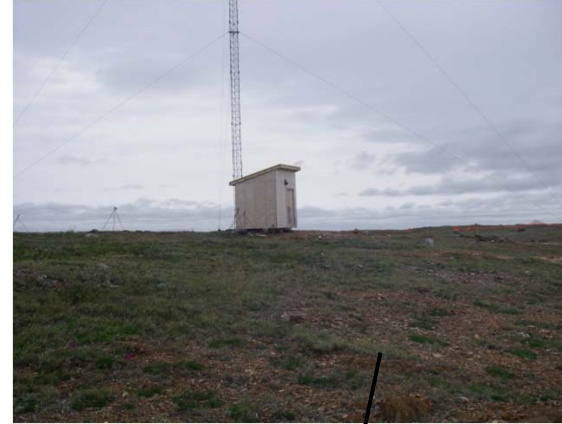
Looking southeast at enclosure for radio equipment installed on raised wooden foundation on rock outcrop.
