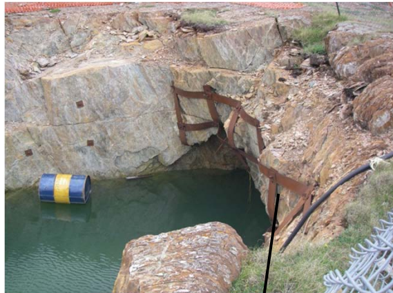
Rock bolted highwall above the portal.
