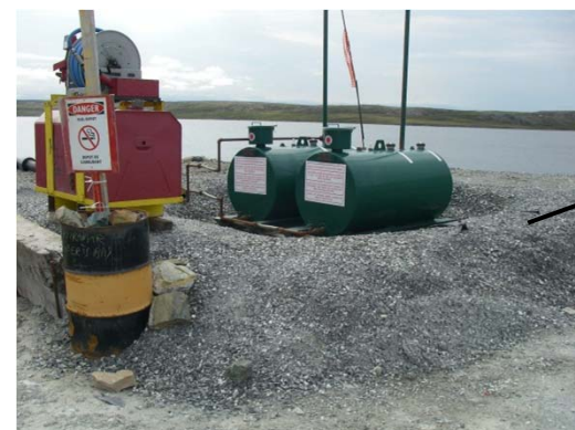
Secondary containment for fuel tanks supplying power house and workshop.
