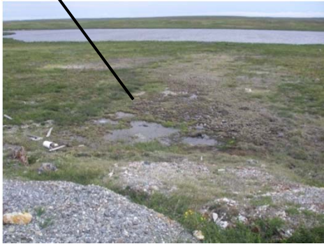
Ponding and vegetation dieback as seen at toe of camp pad.
