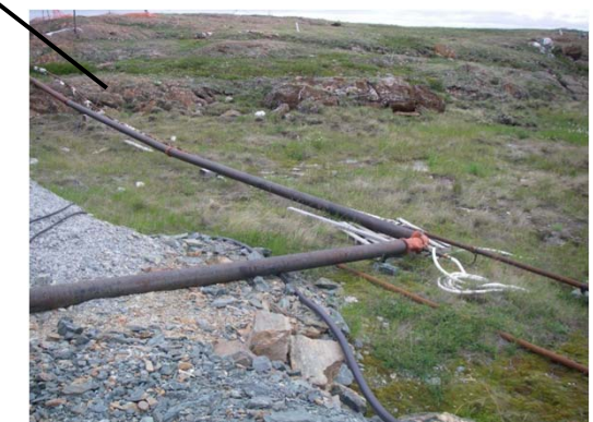
Fuel delivery pipeline to power house and workshop.
