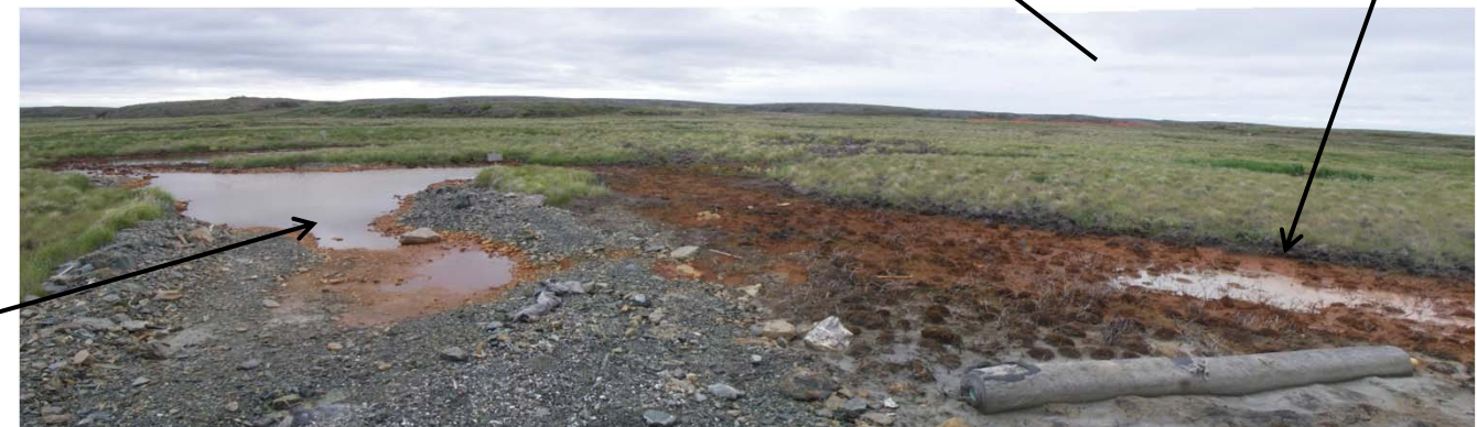
Large permafrost degradation and vegetation dieback area along west shoulder of airstrip.
