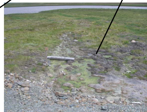
Signs of seepage from the settling pond.
