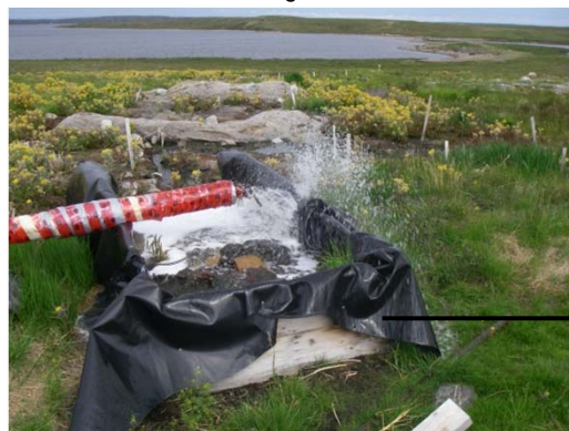
Diffuser for treated sewage effluent outflow.
