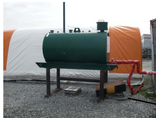
Fuel tank without secondary containment.
