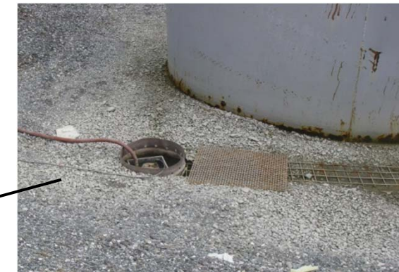
Sump with submersible pump in the northwest corner of the tank farm.
