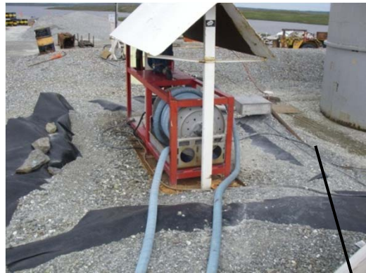
Fuel transfer pump on western containment berm.
