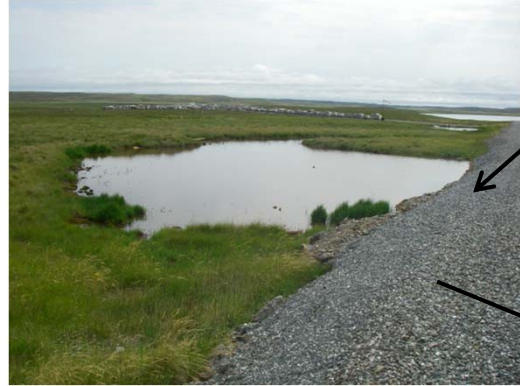
Permafrost degradation pond along east shoulder of airstrip
