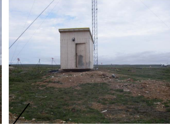
Looking northeast at enclosure for radio equipment installed on raised wooden foundation on rock outcrop.
