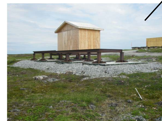
Thermal pad and raised foundation for components of the new Boston Sewage Treatment Plant.
