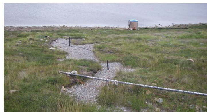
Looking west at an area of erosion and permafrost damage repaired by infilling with gravel
