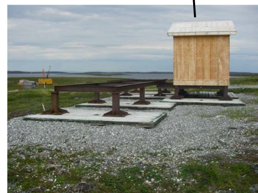
Close-up of raised foundation footings used on the new Boston Sewage Treatment Plant.
