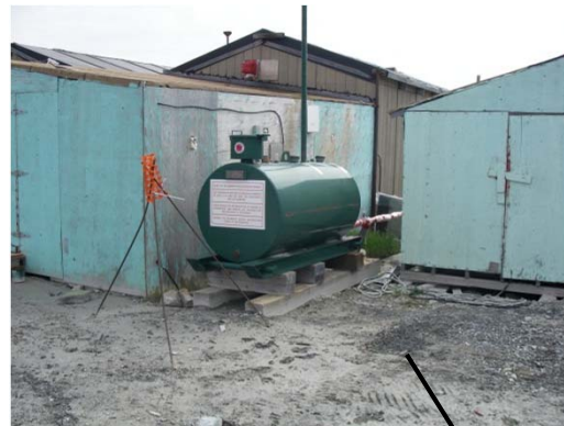
Fuel tank without secondary containment.
