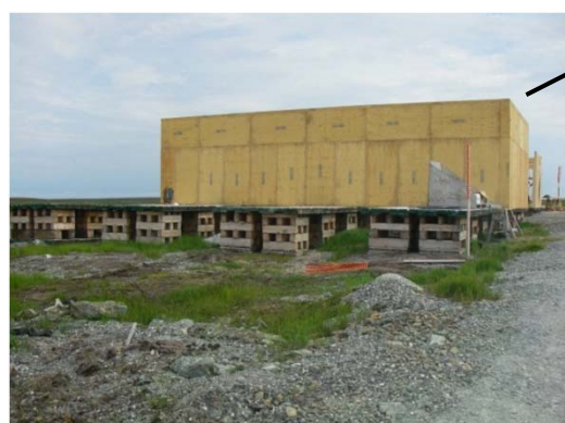
Lower end of the leveling foundation for the new Boston Sewage Treatment Plant.
