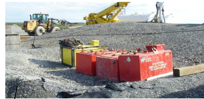
Air-transportable fuel tanks in secondary containment. Photo looking northeast
