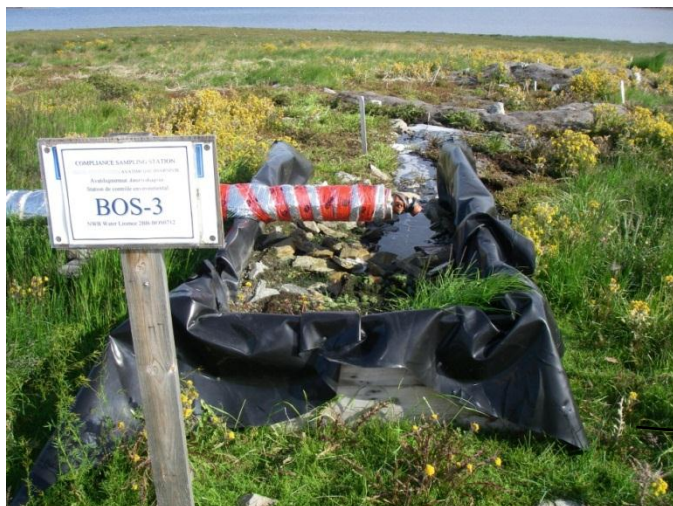
Diffuser for treated sewage effluent
