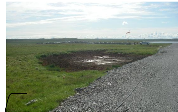
Permafrost degradation along east side of Airstrip
