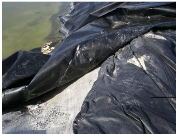
Closer look at tears and rips in the liner
