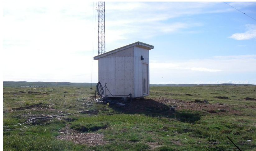
Enclosure for radio equipment installed on raised wooden foundation rock outcrop
