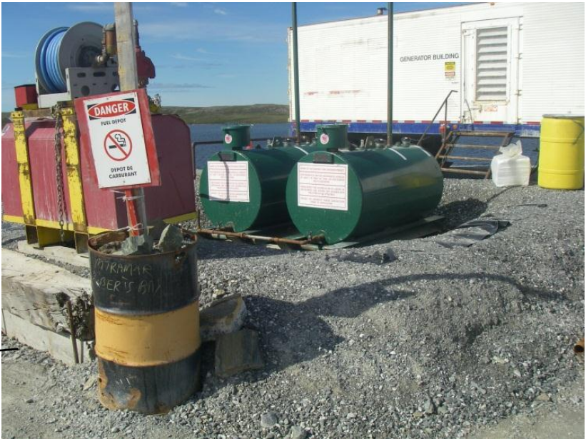
Secondary containment of powerhouse and shops fuel supply. Photo looking northwest
