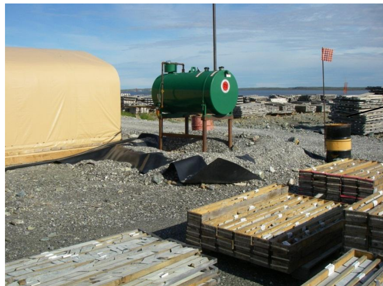
Fuel Tank with secondary containment berm on the east side of the complex
