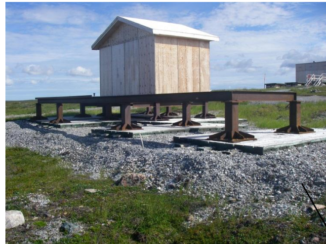
Close up look at thermal pad and raised foundations of new sewage treatment plant
