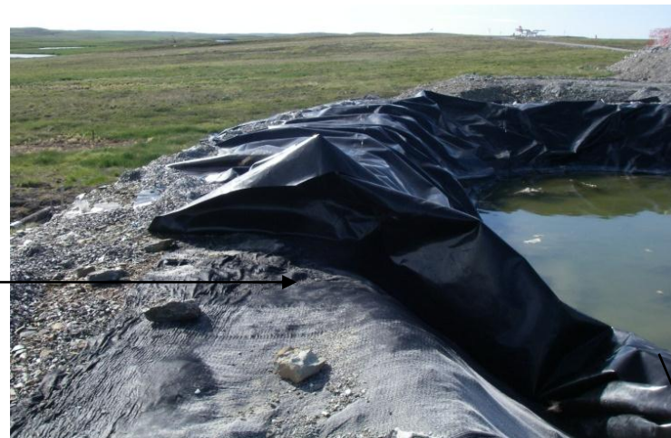
Folded portion of liner with tears and rips
