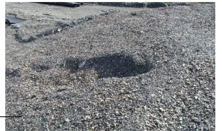
Settlement deformation of the north berm of the tank farm
