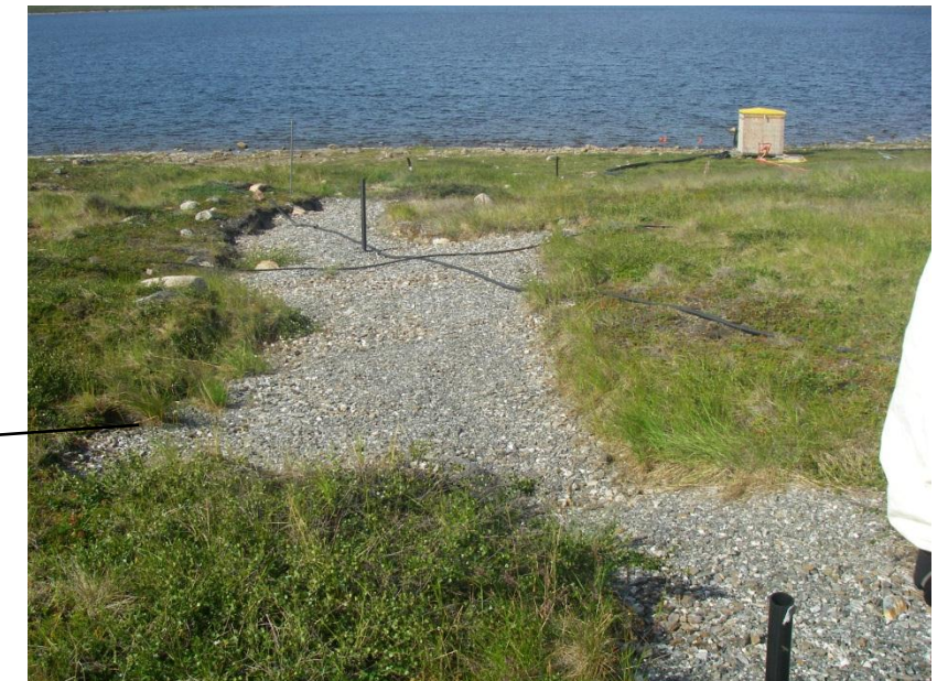
Trench on tundra filled with gravel
