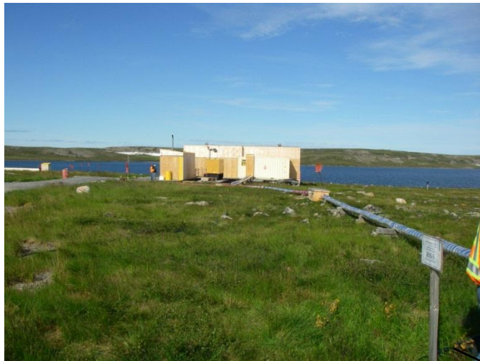
Pipe running from old sewage treatment to diffuser
