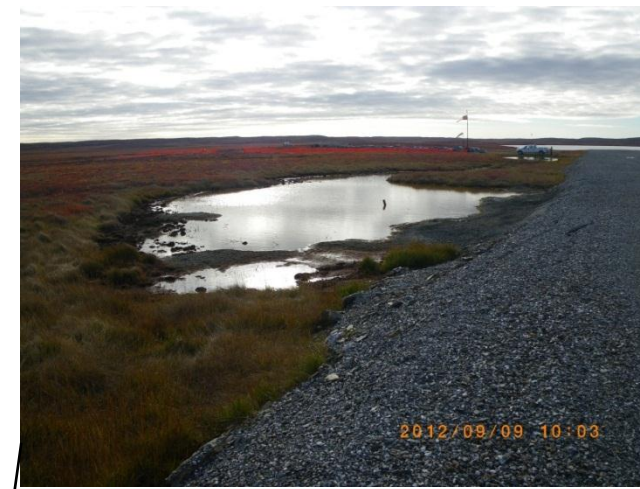
Permafrost degradation and ponded water
