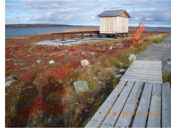
Thermal pad and raised foundation for the new sewage treatment plant
