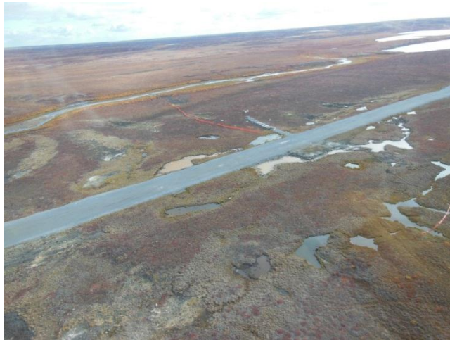
Aerial view of core box clean-up around core storage road/ drill cutting disposal and permafrost degradation along the airstrip perimeter – looking southeast
