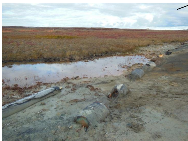
West side of drill cutting disposal area showing geotextile drapes over 45 gal. drums – looking northwest while on disposal area
