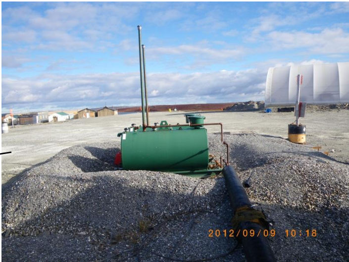
Side view of powerhouse/ shops fuel supply
