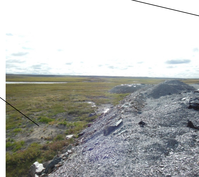
Seepage and vegetation die back at the toe of the rock fill pad by the Ore Stockpiles
