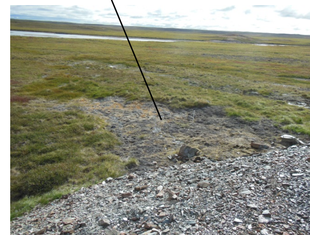
Seepage and vegetation die back along the toe of the Containment Pond
