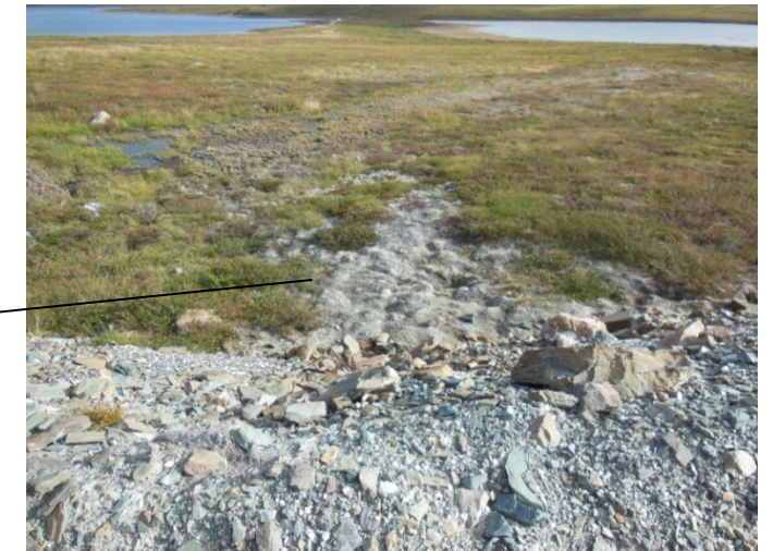
Seepage and vegetation die back at the toe of the rock fill pad at north end of the Ore Stockpiles
