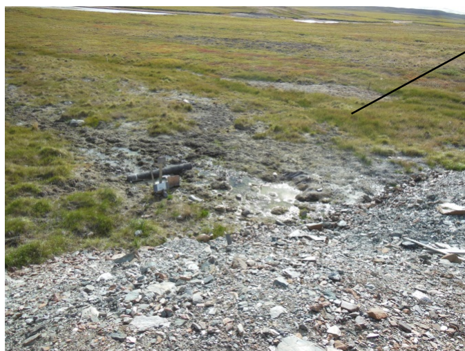
Seepage and vegetation die back along the toe of the Burn Pit
