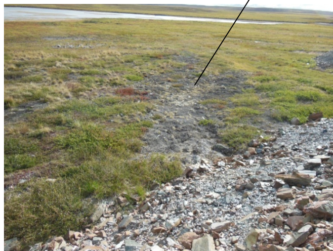
Seepage and vegetation die back at the south end of the Ore Stockpiles
