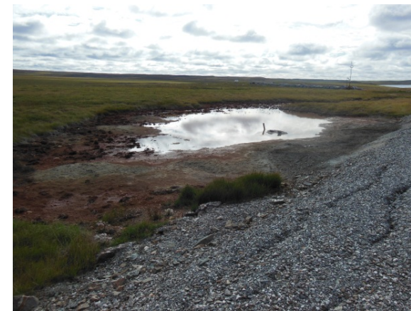
Permafrost degradation and ponded water along edge of the Airstrip
