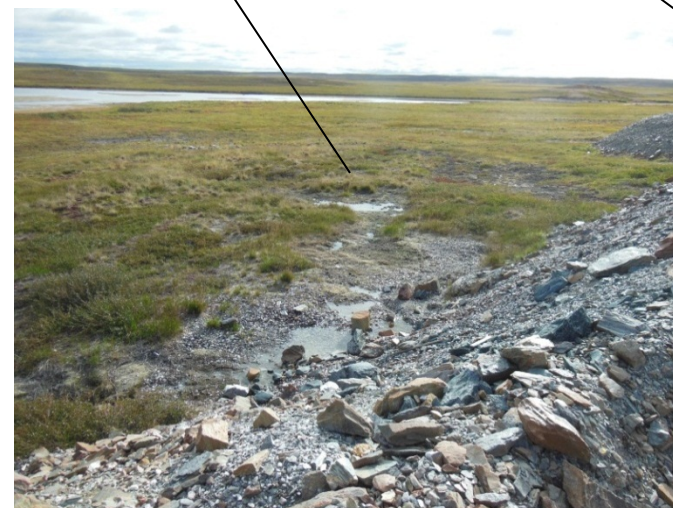
Seepage and vegetation die back at the toe of the rock fill pad by the Ore Stockpiles
