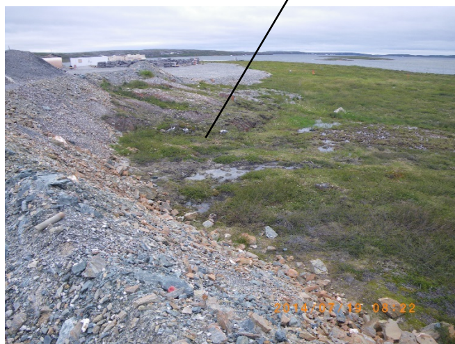
Seepage and vegetation die back at the toe of the rock fill pad by the Ore Stockpiles – looking north
