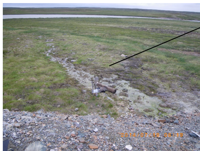
Seepage and vegetation die back along the toe of the Containment Pond – looking east
