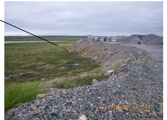
Seepage and vegetation die back at the toe of the rock fill pad at north end of the Ore Stockpiles – looking south
